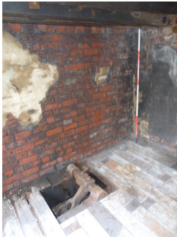
Plate 14: Looking south-east. Ground floor, east wall and brake-transmission lever.
