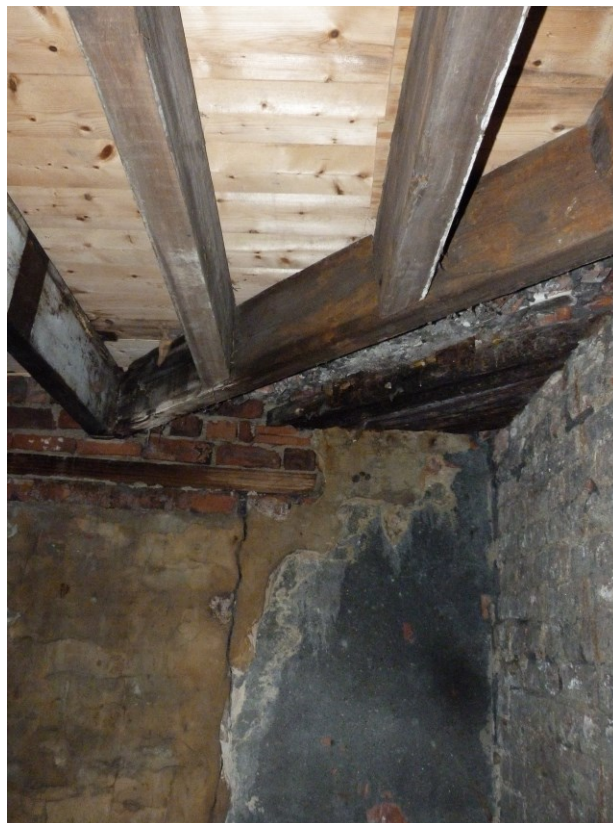
Plate 18: Looking south-west. Ground floor. Base of first-floor fireplace in ground-floor ceiling.
