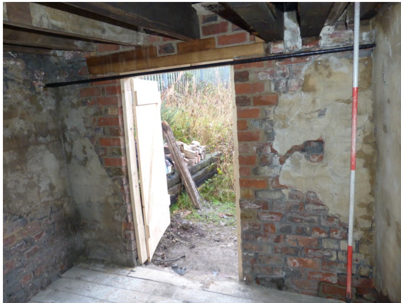
Plate 16: Looking north. Ground floor. North wall and restored doorway.
