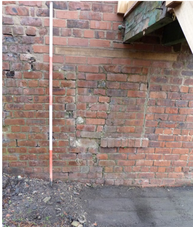
Plate 19: Looking north. South wall showing blocked window.
