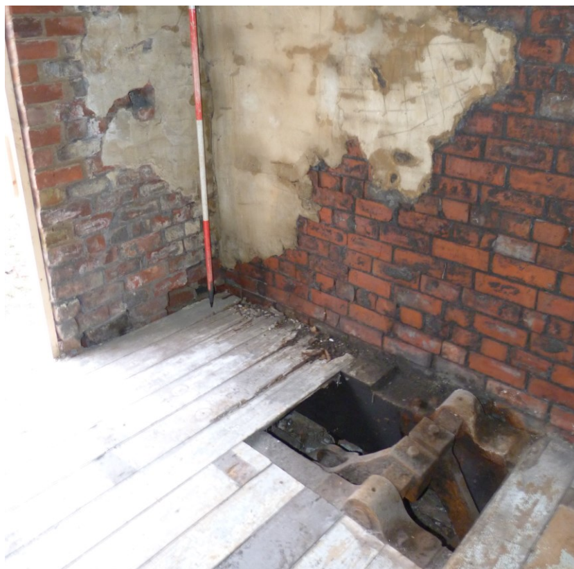
Plate 12: Ground-floor. Brake transmission lever cleared.
