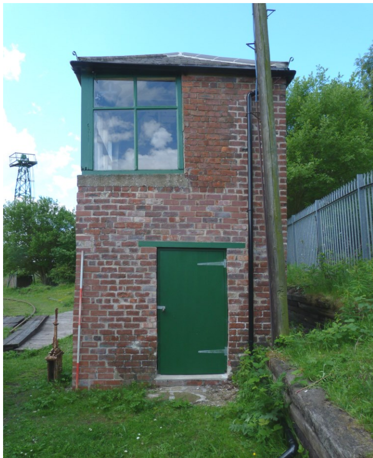
Plate 25: Looking south at new door and window.
