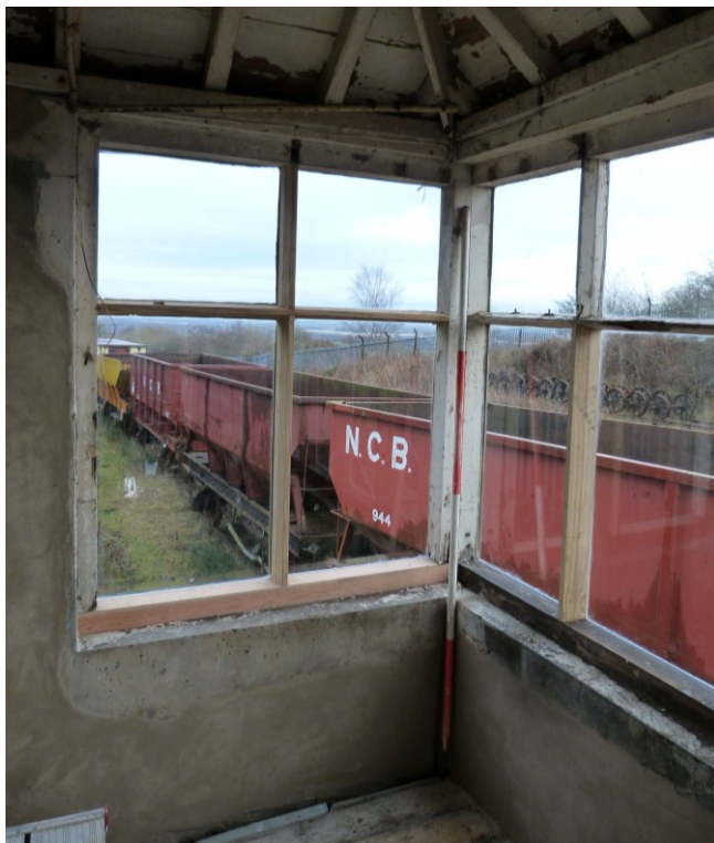
Plate 6: First floor. Looking north-east. Windows following conservation.
