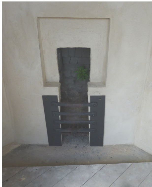
Plate 8: Hearth in south-west angle following conservation.
