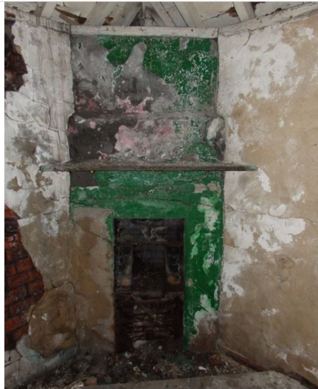
Plate 7: First floor. Looking south-west. Hearth in south-west angle before conservation.
