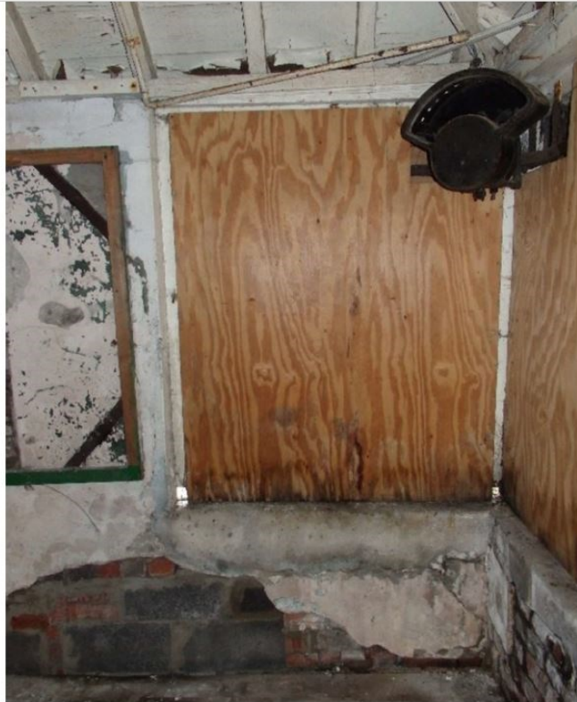
Plate 5: First floor. Looking north. Blocked windows before conservation.
