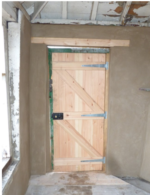
Plate 4: First floor. Looking south. Door in south-west wall after conservation.
