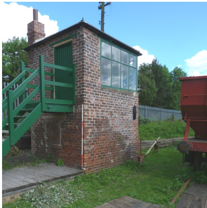
Plate 23: Looking north-west at platform, steps and windows.
