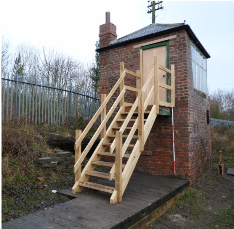
Plate 21: Looking north. External stair replaced.
