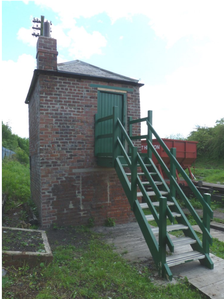
Plate 26: Looking north-east at new steps and door.
