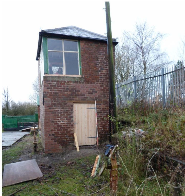
Plate 20: Looking south-west. Windows and door restored.
