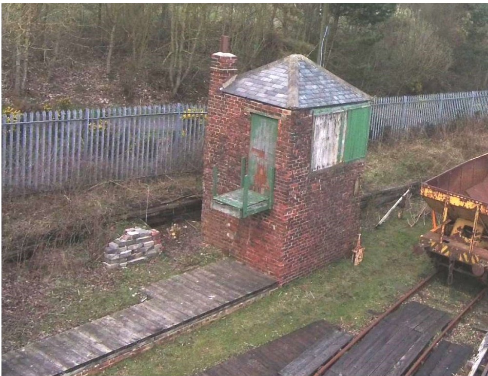
Plate 2: Brakeman's Hut from the south (Drone photograph by Doonan Architects 2018).
