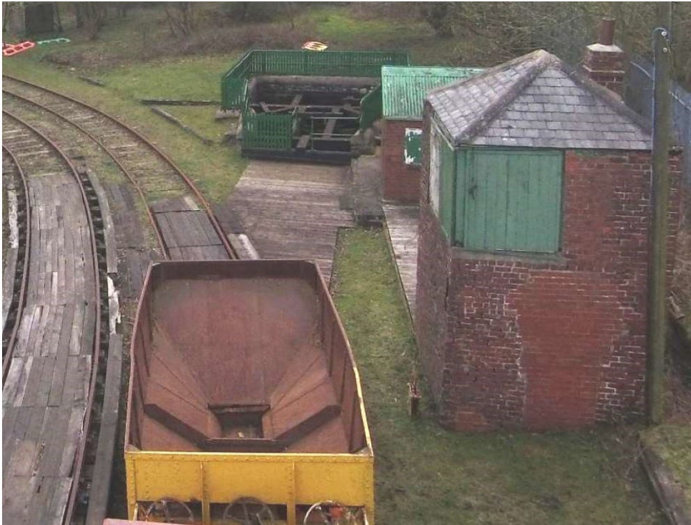
Plate 1: Brakeman's Hut from the north (Drone photograph by Doonan Architects 2018).
