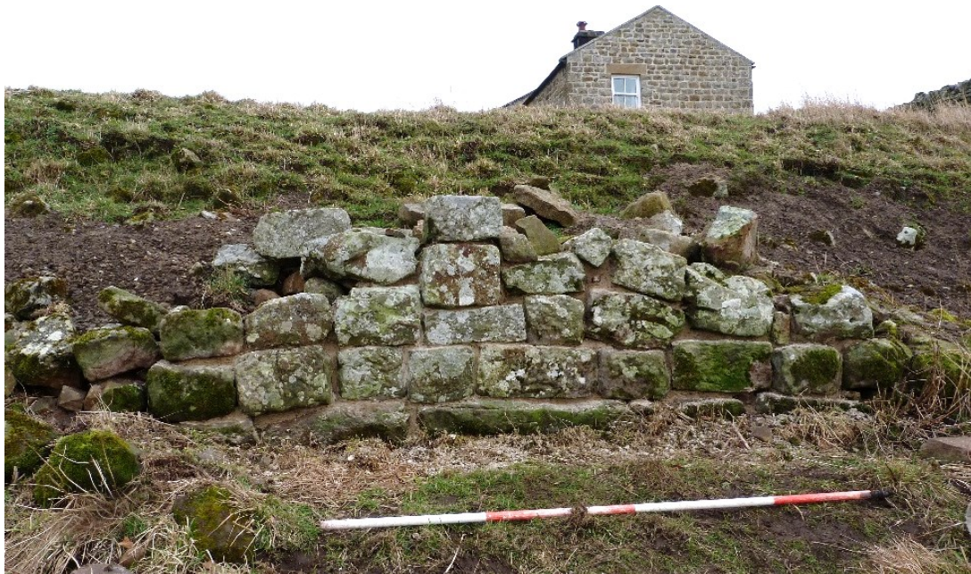
Plate 34: Block W7 during conservation, open joints have been deep tamped. Prior to turf capping. Looking east.
