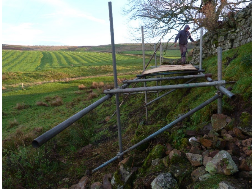
Plate 3: The north rampart, looking east. Platform constructed to take dropped stones for rebuilding.
