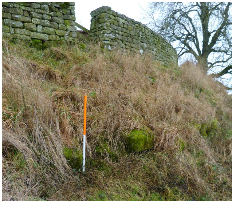
Plate 46: Block W23 (north) in autumn 2019. Facing stones re-bedded and corework above (W24) consolidated with turf and soil. Looking south.
