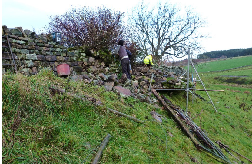
Plate 13: Loading stones on the platform for rebuilding. The east rampart. Looking north-west.
