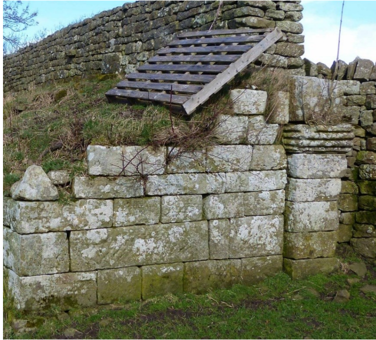
Plate 39: Block W16. The west gate. Pre-conservation with woody vegetation growing out of the upper courses of stonework. Looking north-east.
