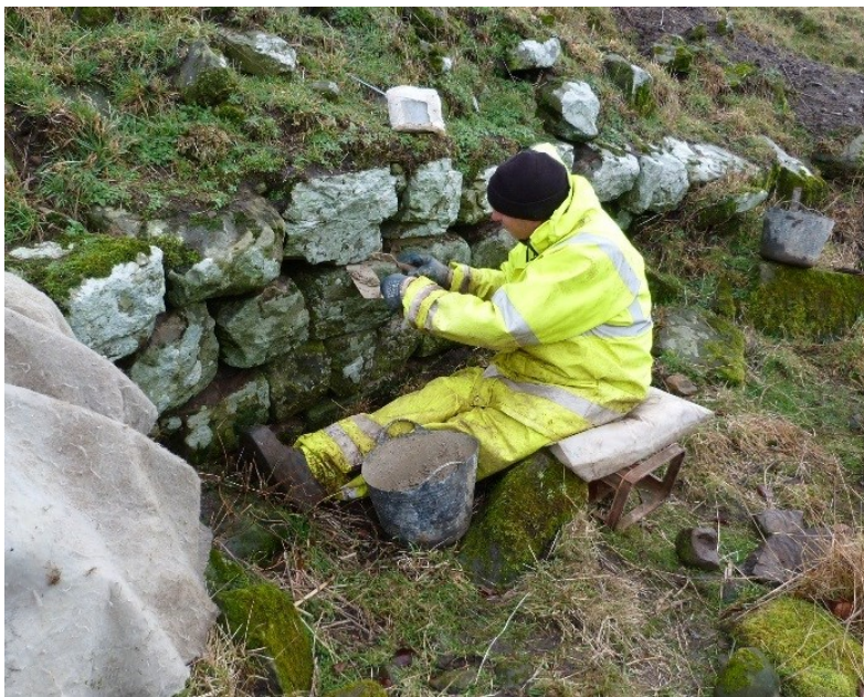
Plate 36: Mortar work on Block W9.
