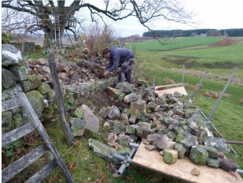
Plate 15: Taking down the wall at the north-east corner of the rampart. Looking north-west.
