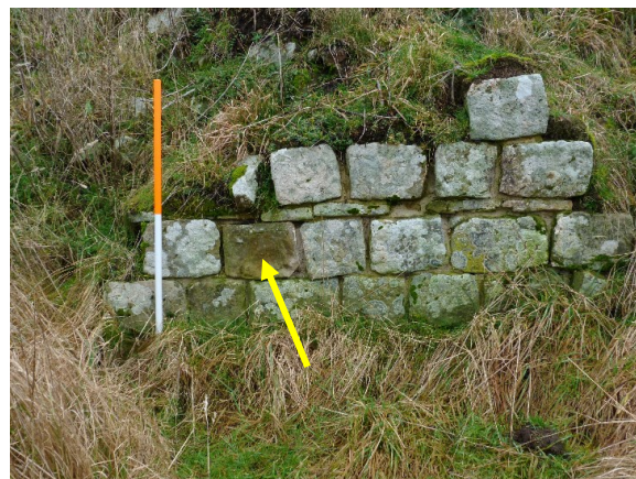
Plate 32: Block W2-3 following consolidation and turf capping. Arrow marks fallen stone recovered from base of wall which has been re-inserted.
