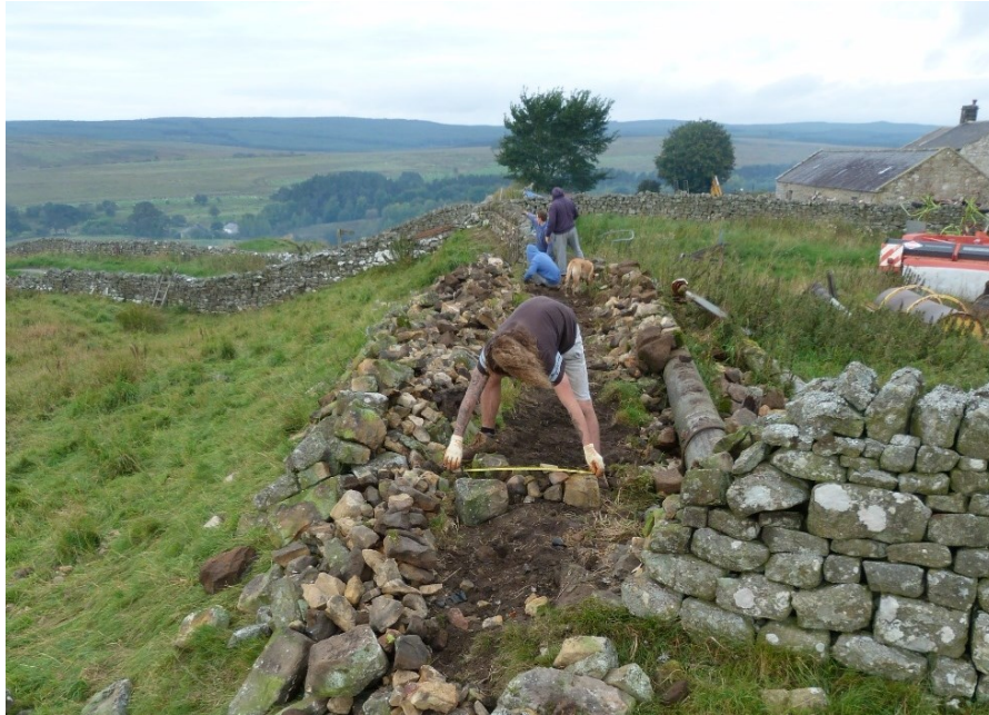
Plate 17: Measuring the width for the rebuilt wall S5. Looking west.
