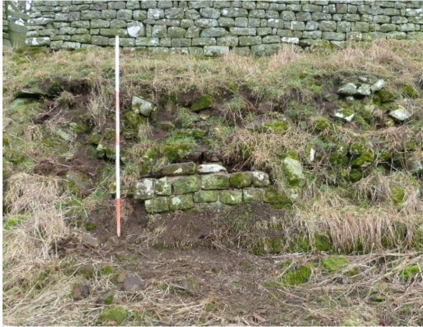
Plate 45: Block W23 (south) during consolidation, facing stones re-bedded and corework above and to right (W22 and W24) consolidated with turf and soil. Looking east.
