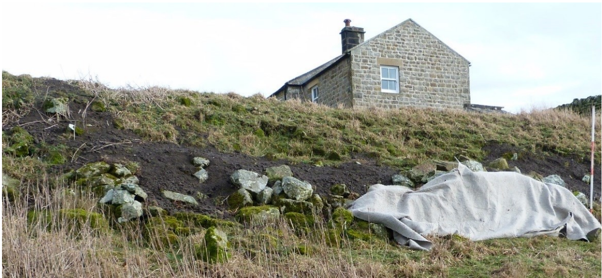
Plate 51: Block W8. Topsoil spread to stabilise and protect loose rubble. Looking east.
