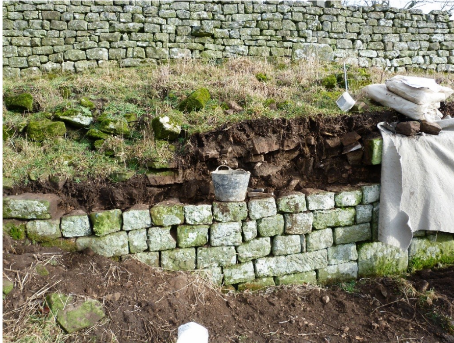
Plate 41: Block W19 North of west gate during conservation. Four courses removed exposing core. Looking east.
