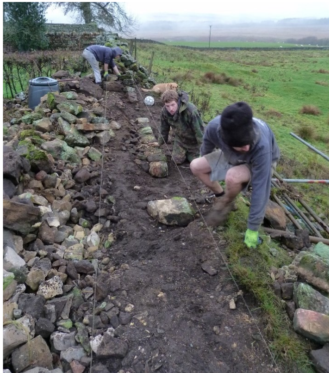
Plate 6: Laying out the line of the new wall along the north rampart. Looking west.
