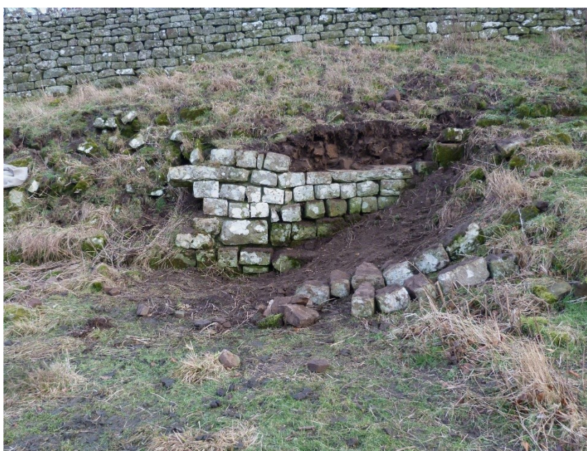
Plate 44: Block W21 during consolidation, a number of facing stones removed for re-bedding. Looking east.
