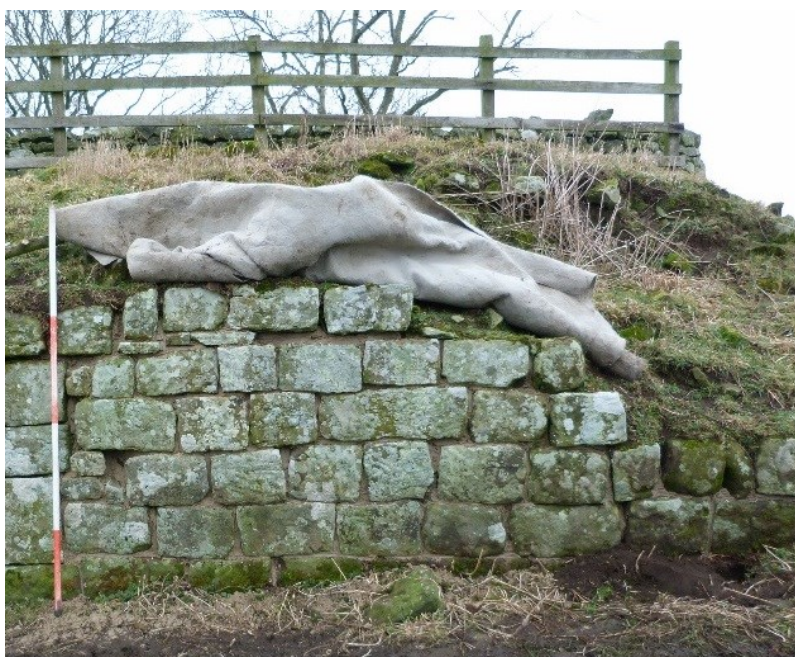
Plate 37: Block W13. Masonry south of the west gate during conservation. Open joints have been mortared. Looking east.
