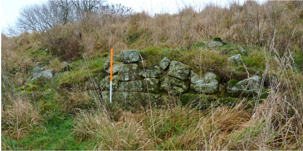
Plate 35: Block W7 following conservation and with turf capping added.
