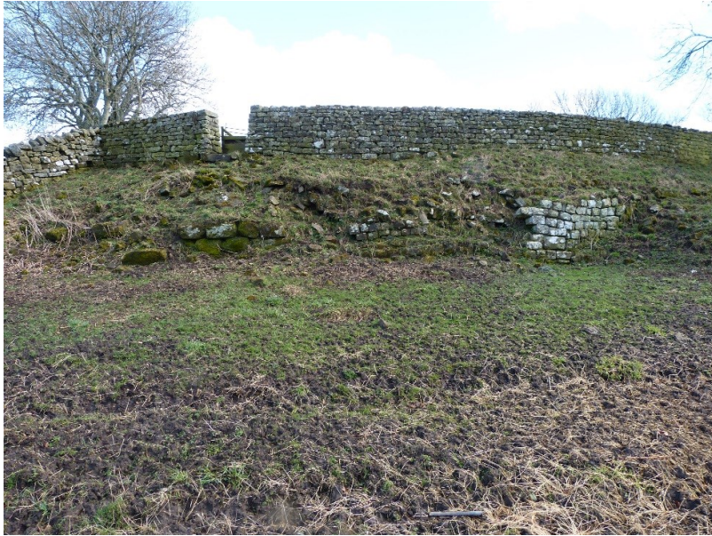
Plate 5: The north-west angle of the fort with standing facework and exposed core below a modern dry-stone wall.
