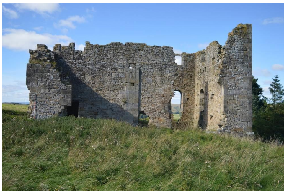
Plate 2: The engine house from the east. Much of the east wall has fallen since the 1970s, exposing in this picture the central longitudinal wall.
