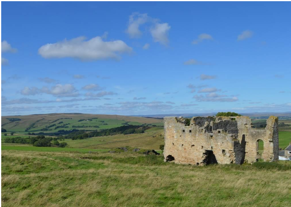
Plate 1: The engine house in its landscape. Looking north-west.
