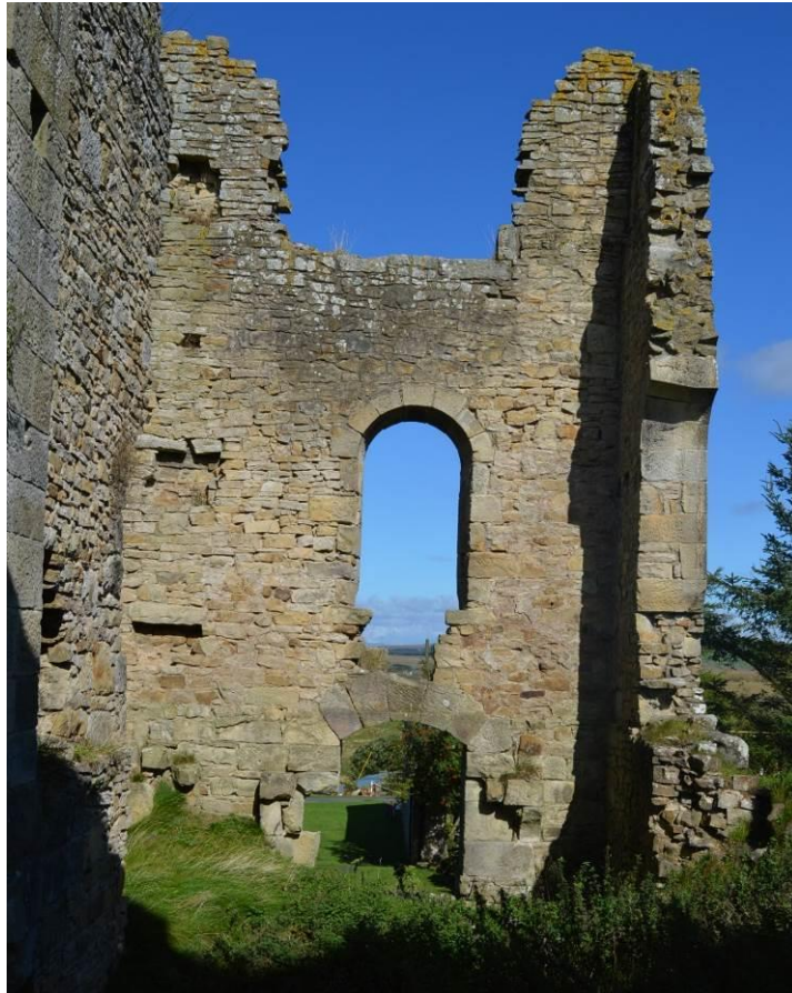
Plate 5: Looking at the inner face of the north wall of the engine house, the east wall to the right mostly fallen.
