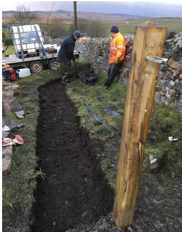
Plate 38: The slot completed. Looking north.
