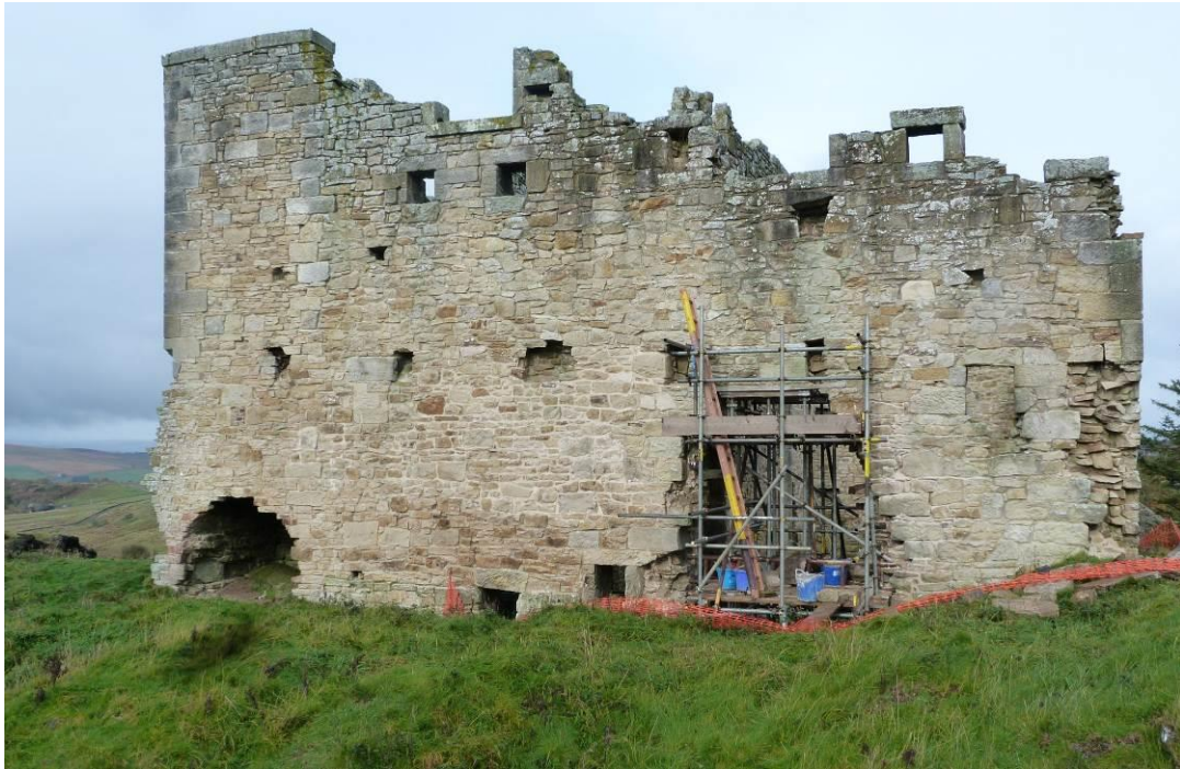
Plate 27: South wall of the Engine House. Scaffolding in place in 2018.
