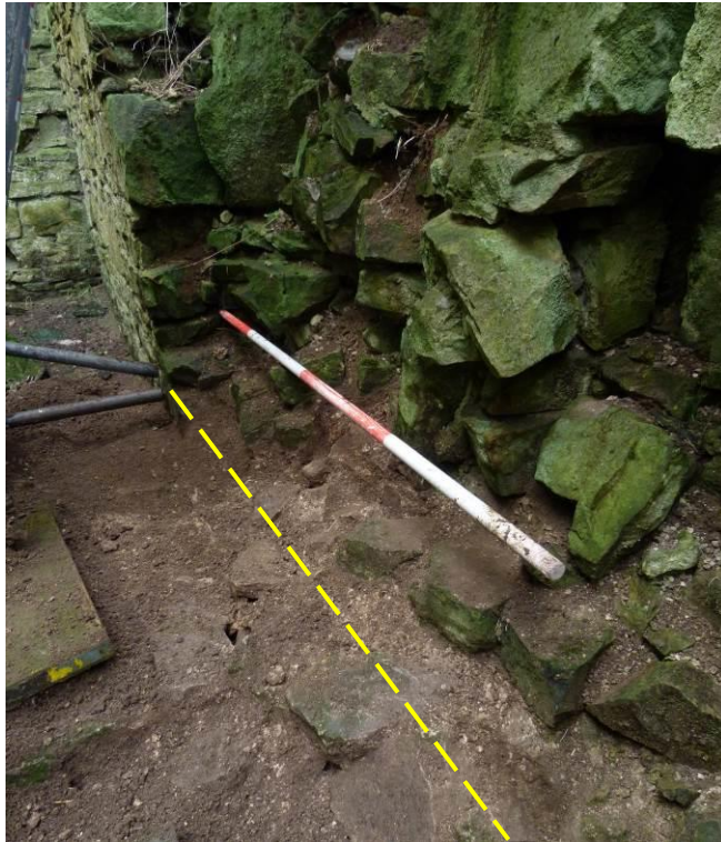
Plate 18: Inside the western half of the Engine House. The west wall following clearance of rubble down to solid core. Broken line shows line of wall face.
