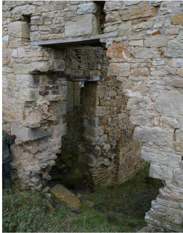
Plate 25: Opening in the south wall of the Engine House in 2017.
