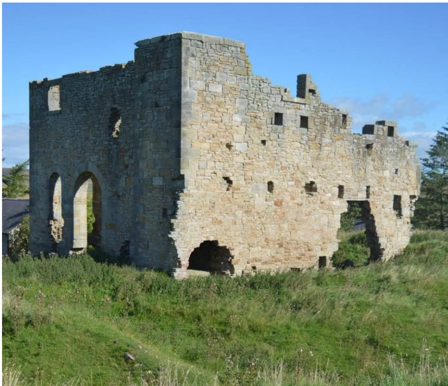
Plate 2: The engine house from the south-west in 2017. A square chimney forms the corner of the building.
