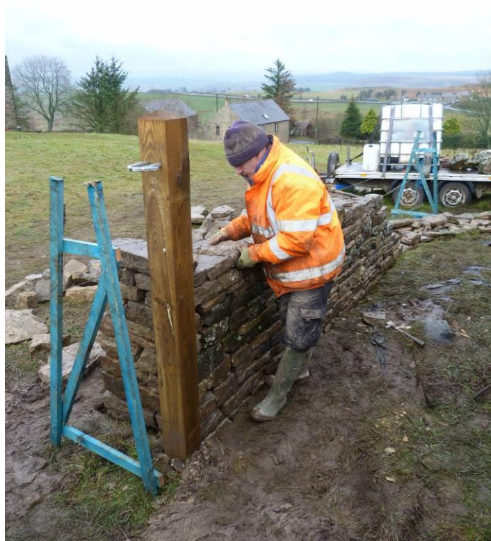
Plate 40: Working on the wall.
