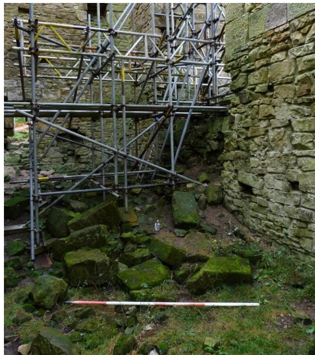
Plate 17: Inside the western half of the Engine House. Looking south at the west wall and tumbled stone below fallen arches. 2m scale.
