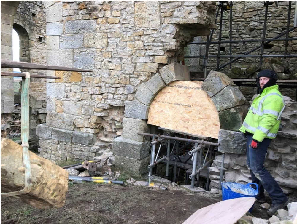
Plate 12: West face of Engine House. Centring in place, voussoirs going in.
