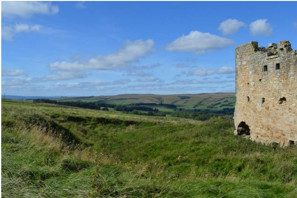
Plate 4: Part of the south face of the engine house from the south-east, looking across the former boiler house.
