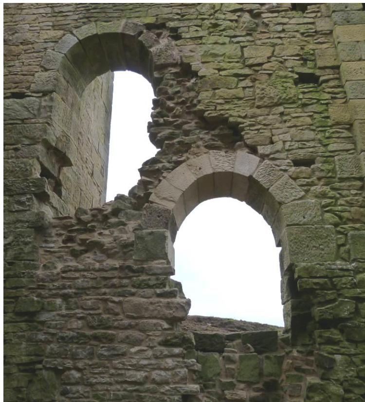
Plate 21: The rebuilt south end of the west wall. Looking west.
