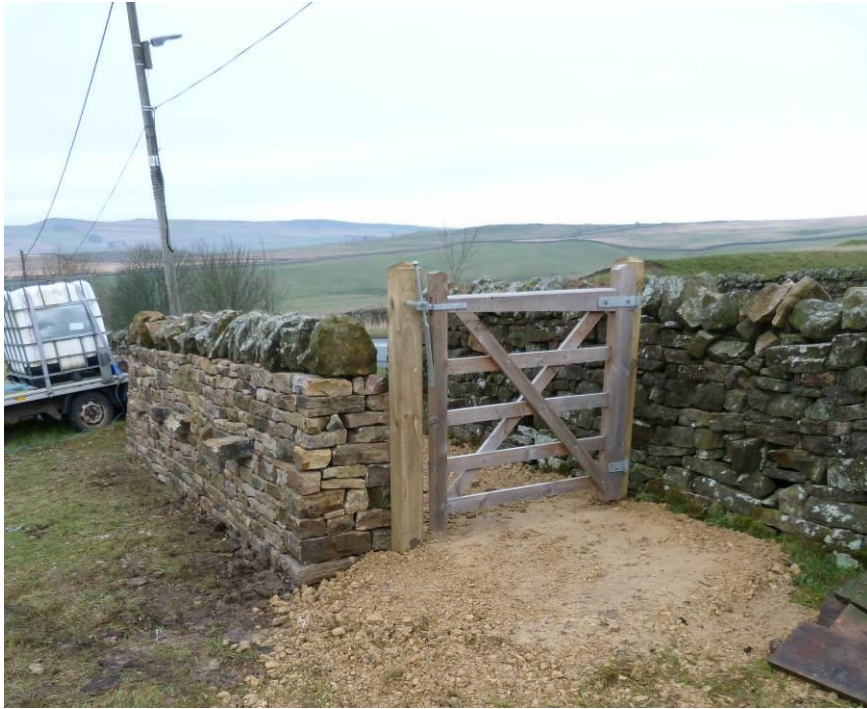
Plate 41: Entrance completed with crushed stone walkway.
