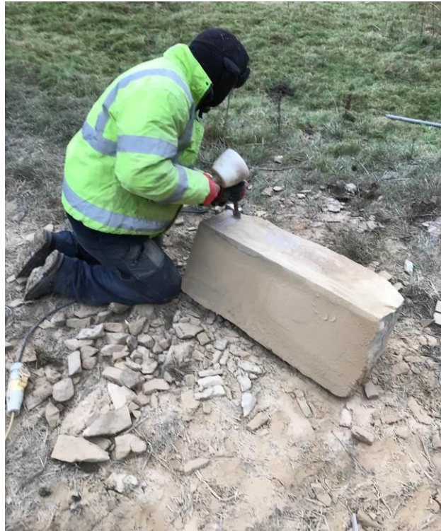
Plate 8: Mason working on a voussoir for its re-insertion Into an opening.
