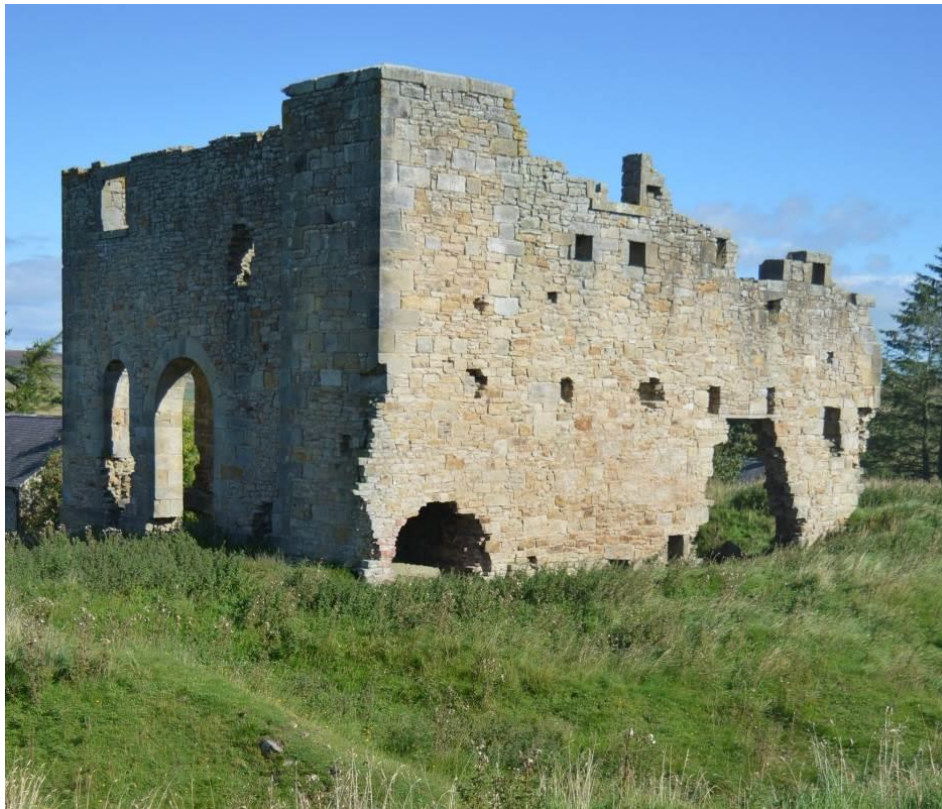
Plate 1: The engine house from the south-west looking across the turf-covered depression, formerly the boiler house for the steam-powered blowing engines within the house. A square chimney forms the corner of the building.
