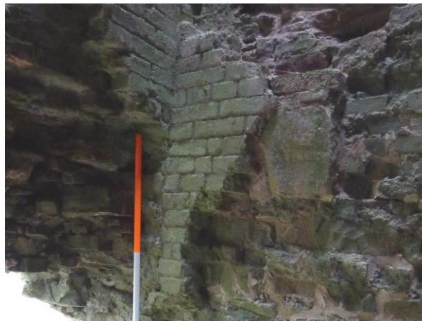
Plate 23: Repointing in the chimney flue.
