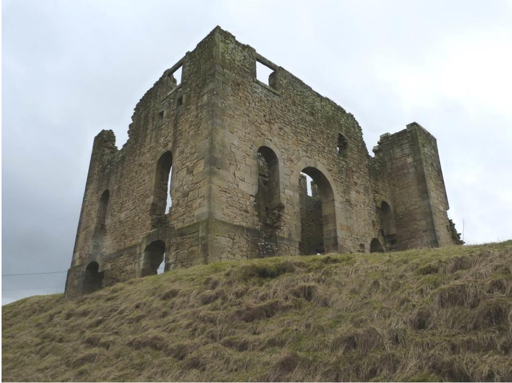
Plate 3: The engine house from the north-west in 2020. The building is set above a steep slope falling to the north.
