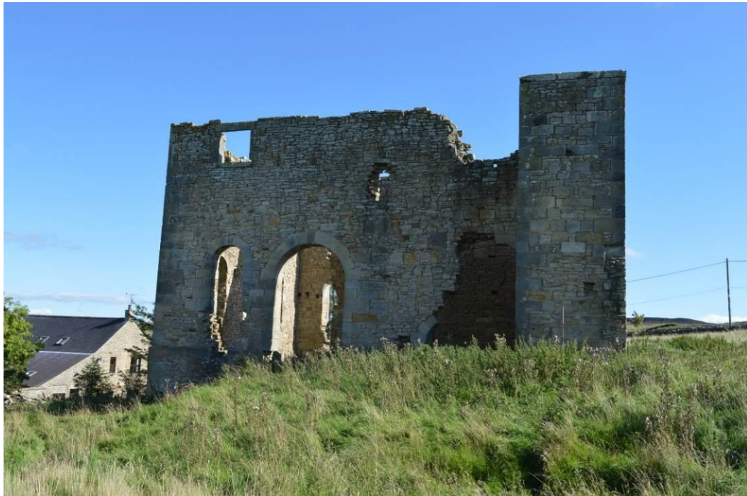
Plate 4: The engine house from the west in 2017 showing the tumbled arches to the left of the chimney.
