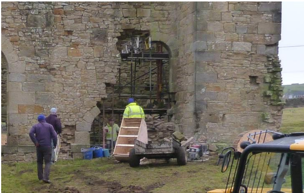
Plate 11: West face of the Engine House with timber centring being brought in to rebuild fallen arch.
