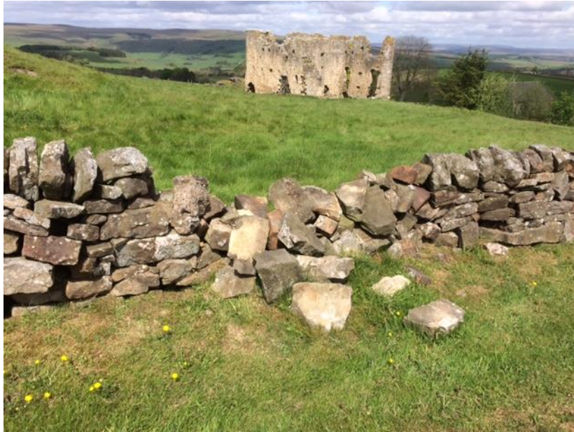
Plate 35: Ridsdale Ironworks 2017. Tumbled area of drystone wall along the A68, the location of the new gated access. Looking north-west (courtesy Lydia Speakman).
