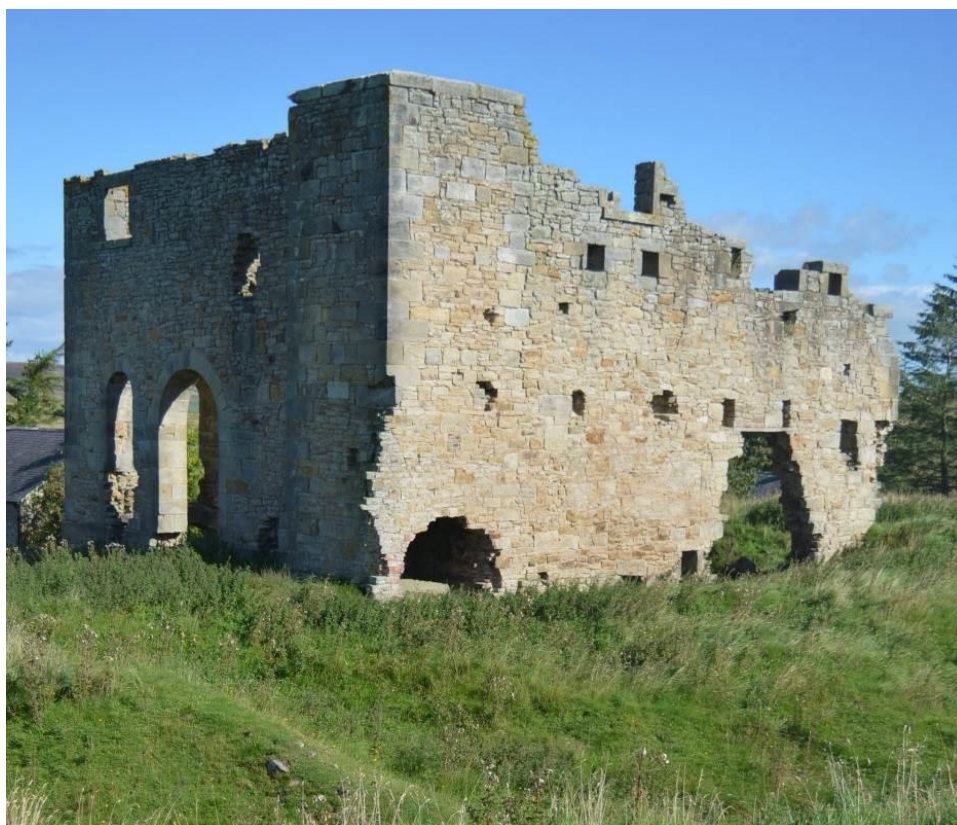
Plate 1: The engine house from the south-west looking across the turf-covered depression, formerly the boiler house for the steam-powered blowing engines within the house. A square chimney forms the corner of the building.
