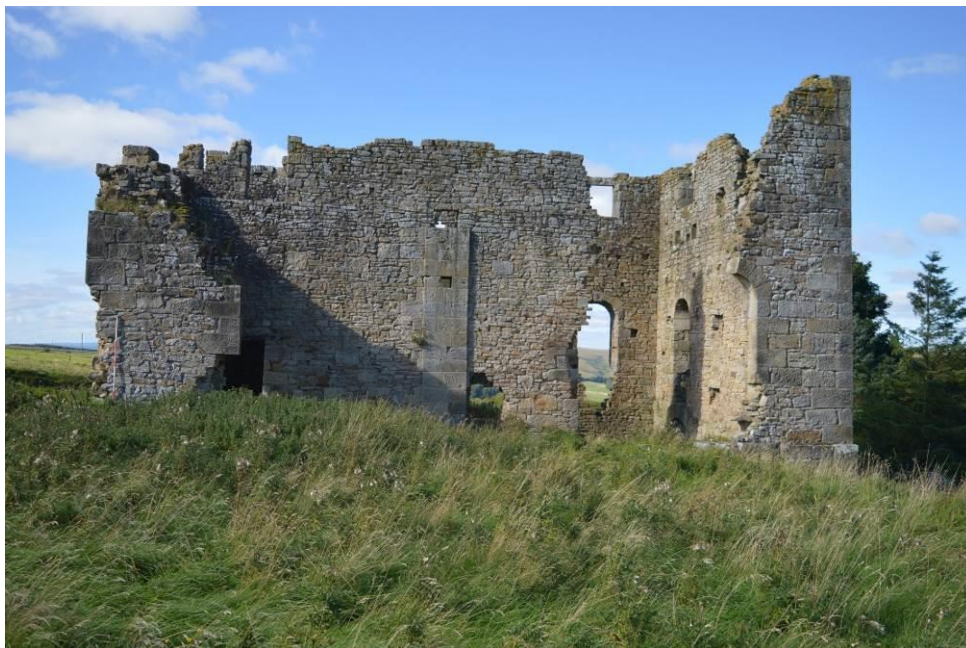
Plate 2: The engine house from the east. Much of the east wall has fallen since the 1970s, exposing in this picture the central longitudinal wall.
