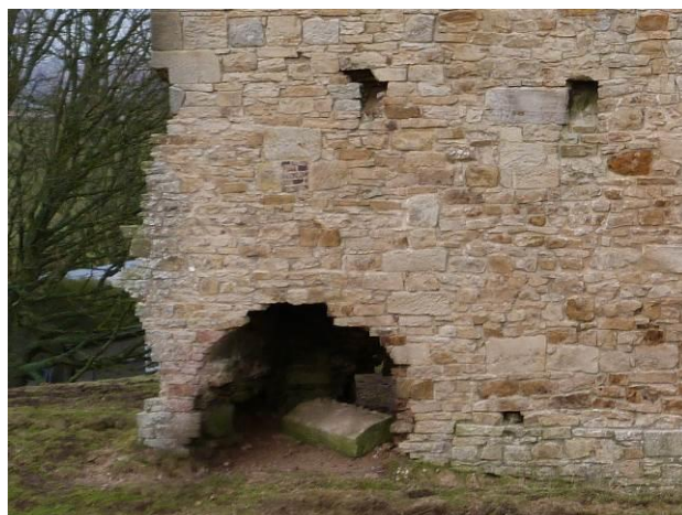
Plate 24: Work completed on the opening and the adjacent walls.
