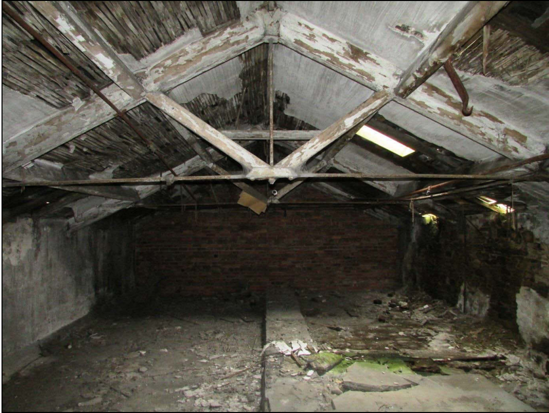
Plate 75 Office Block third-floor. The later southern elevation is visible at the rear, as well as the single span roof incorporating both iron and timber
