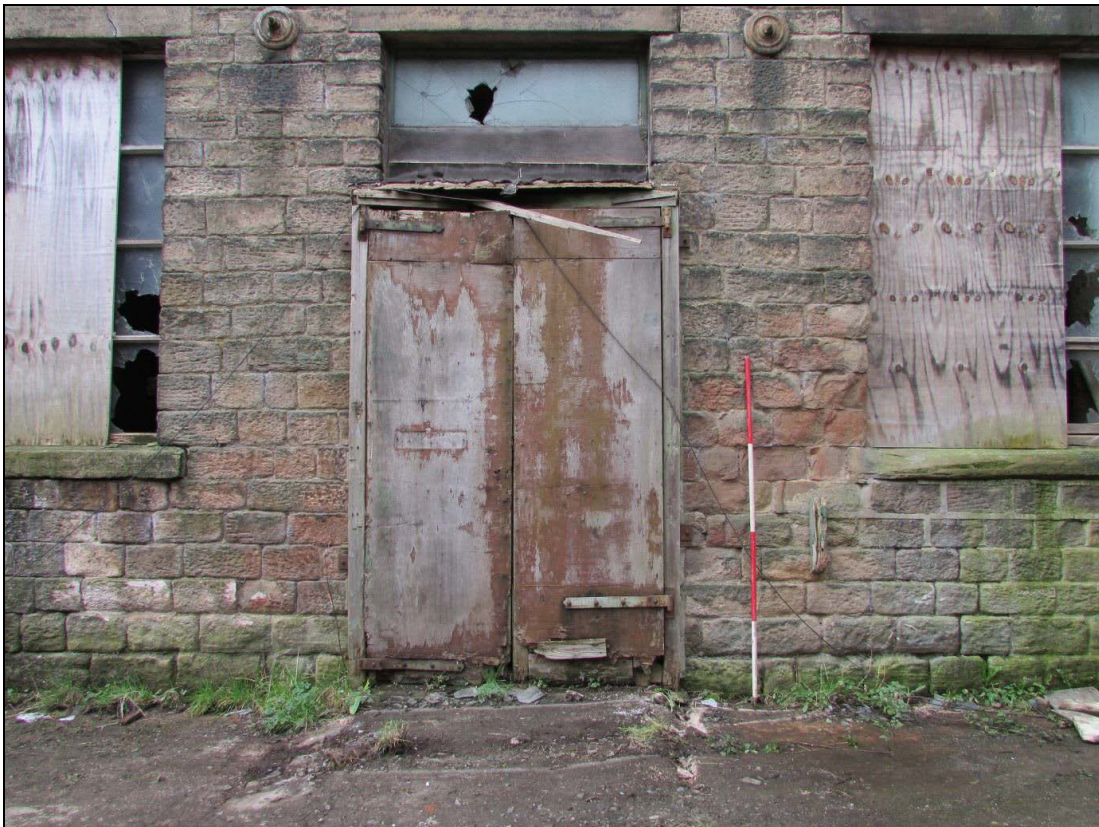
Plate 3 Window on the ground-floor of the mill, later modified into a door
