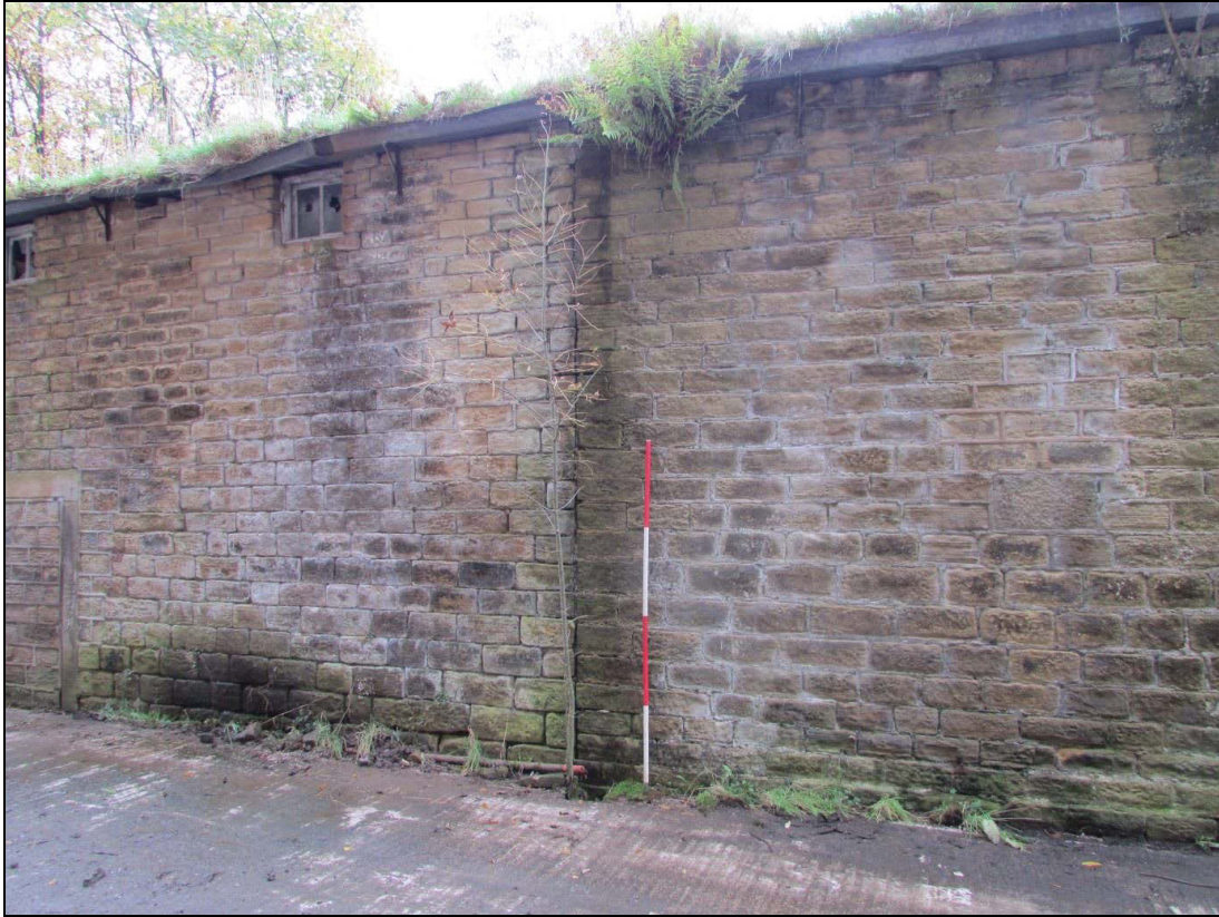
Plate 81 Butt joint between the east (left) and middle (right) sheds
