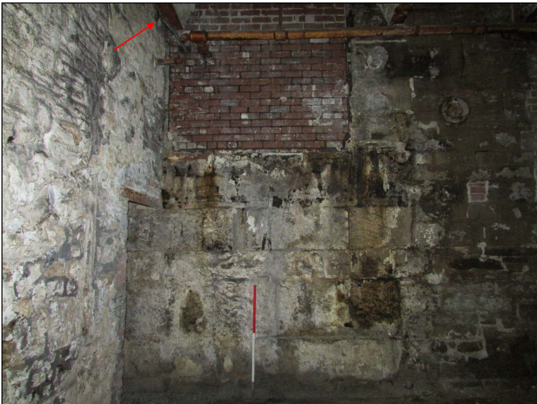
Plate 43 Blocked footstep bearing, with part of the later ceiling visible (the beam (arrowed) abuts the brick blocking)
