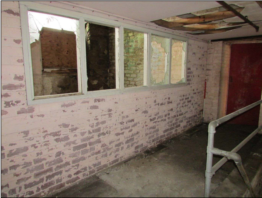
Plate 51 A later brick sub-division on the second-floor of the engine house
