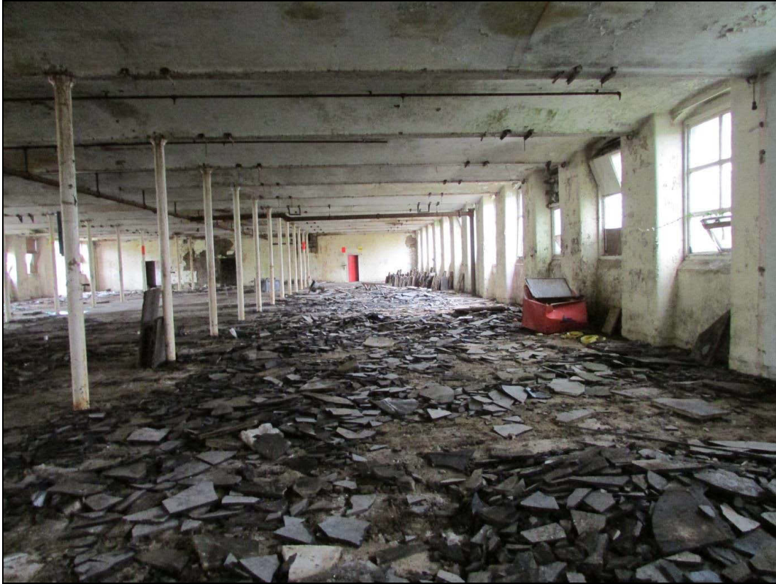
Plate 18 Visible on the beams within the ceiling are two lines of lineshaft hangers, which helped power the machinery
