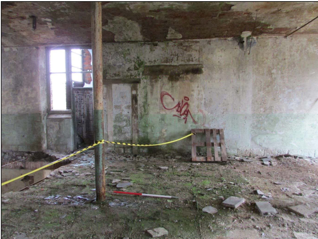
Plate 25 The later entrance to the privy tower extension is evident to the left, with two former entrances blocked to the right
