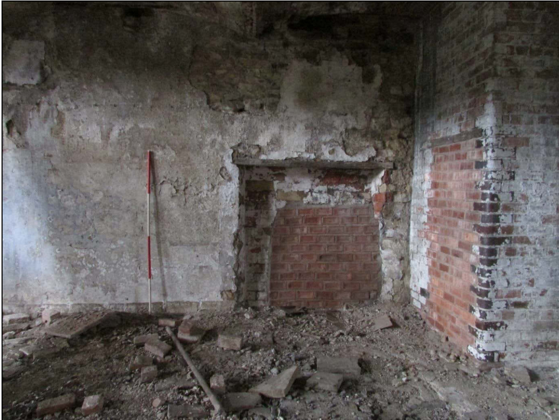
Plate 61 Blocked recess on the third-floor of the engine house. To the right is the blocked entrance into the void
