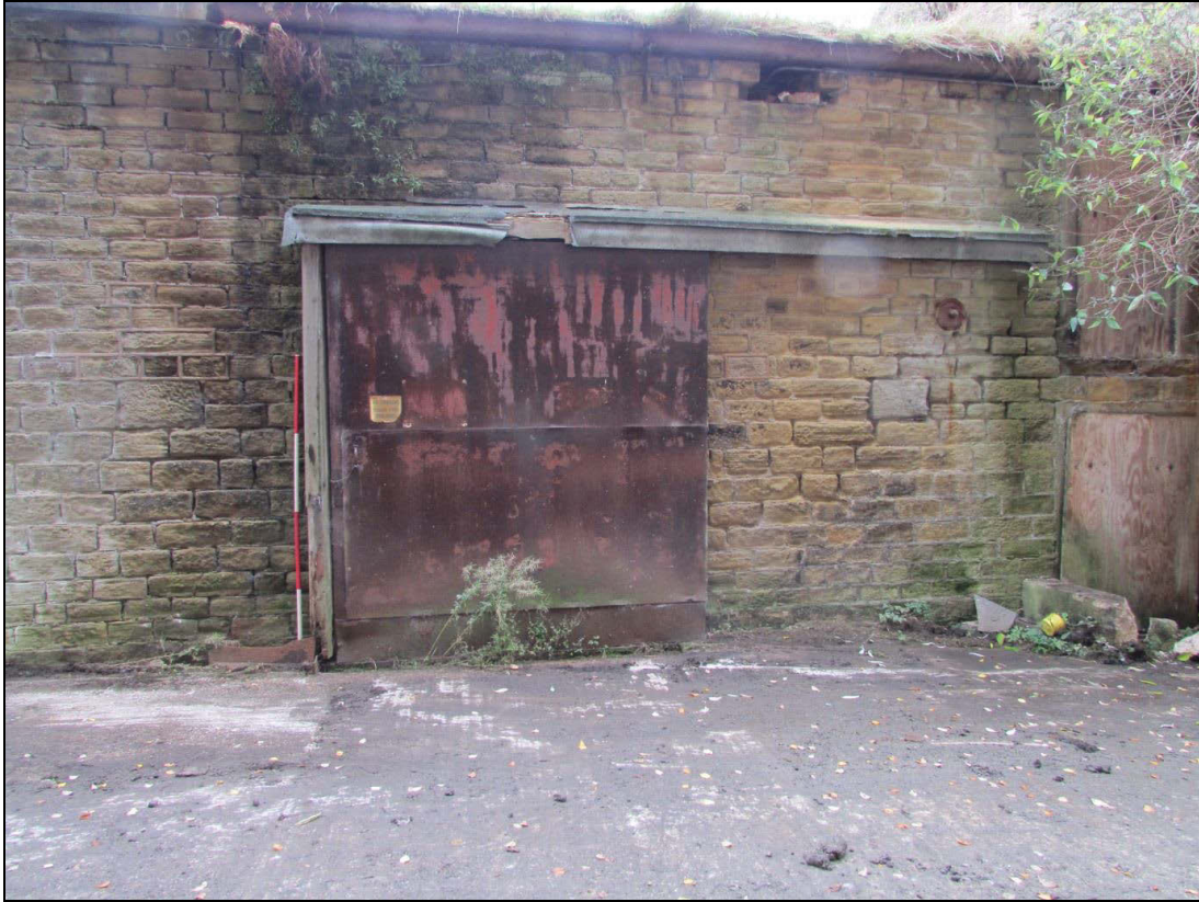
Plate 83 A later inserted door in the middle shed
