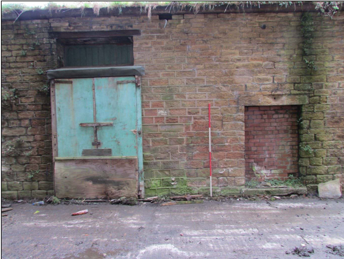
Plate 77 A door was inserted into the northern elevation of the east shed (left) and a window was also blocked at a later stage
