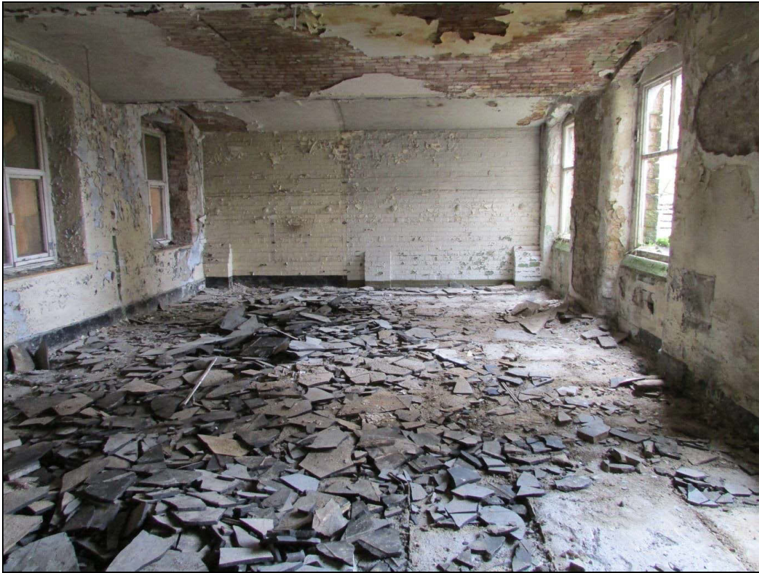
Plate 71 General shot of the Office Block first-floor
