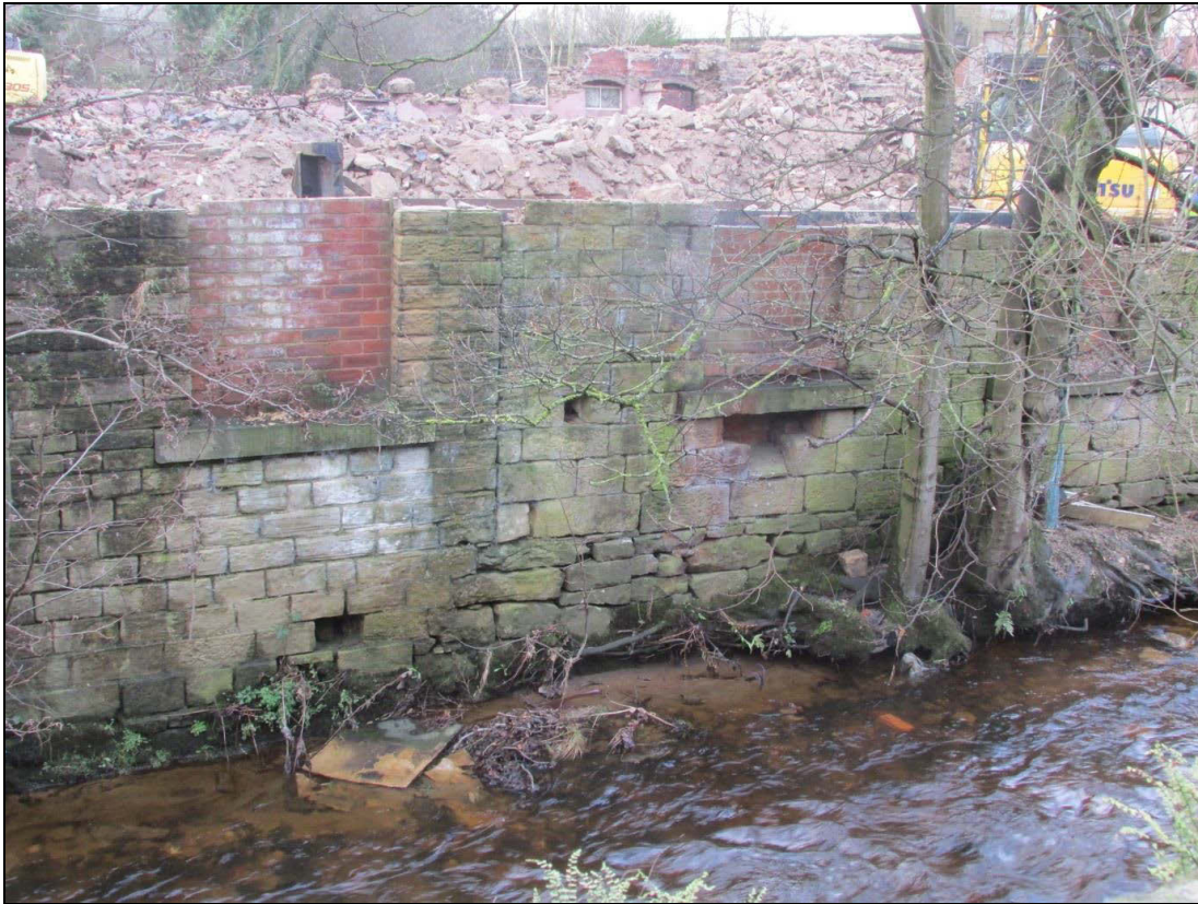
Plate 82 The butt joint between the earlier shed (east) and the later shed (west) is clearly visible, as well as where the later shed partly used the drystone foundations of the earlier building
