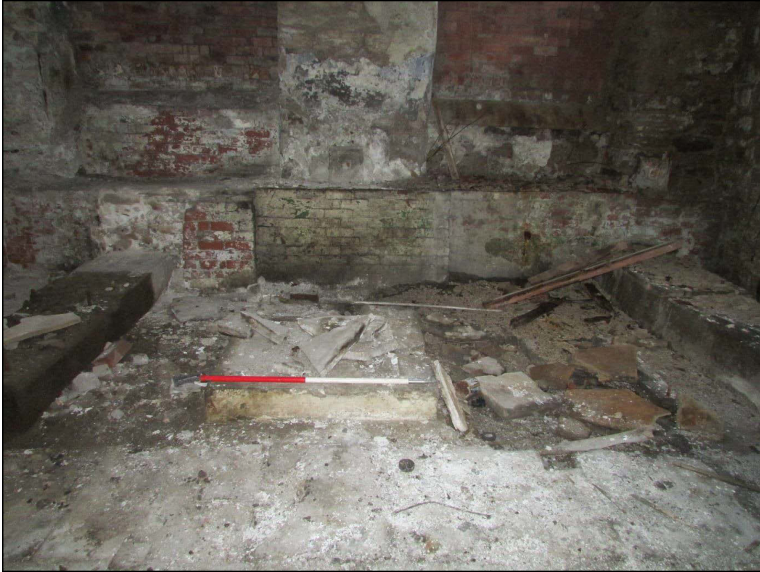
Plate 45 Stone or concrete bedding for later electric motors
