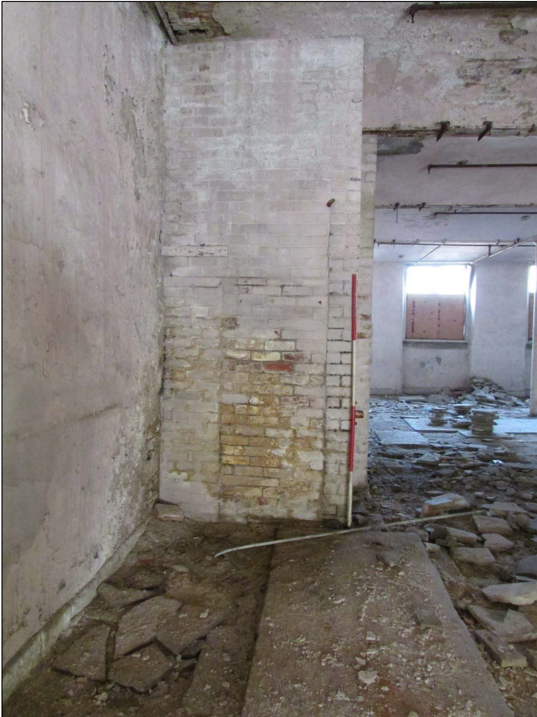
Plate 52 Blocked entrance into a later sub-division, creating a void behind which could not be accessed
