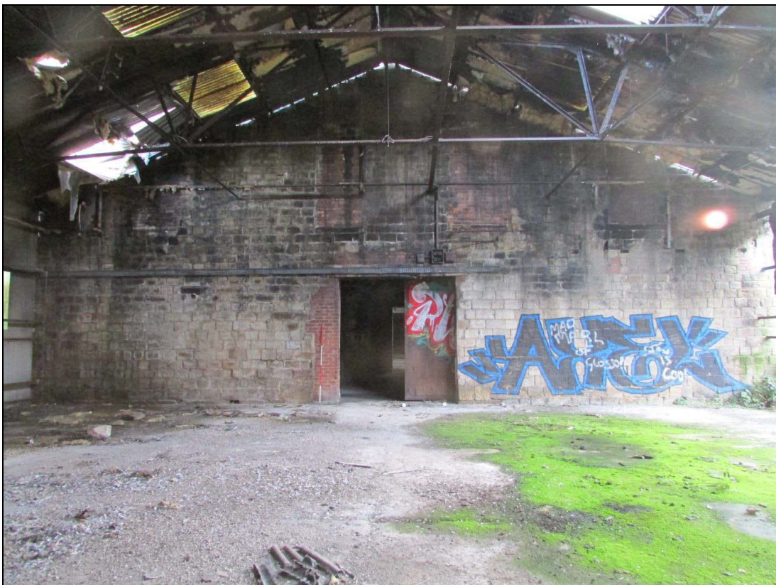
Plate 33 Close up of inserted ground floor entrance and blocked entrances on the first-floor
