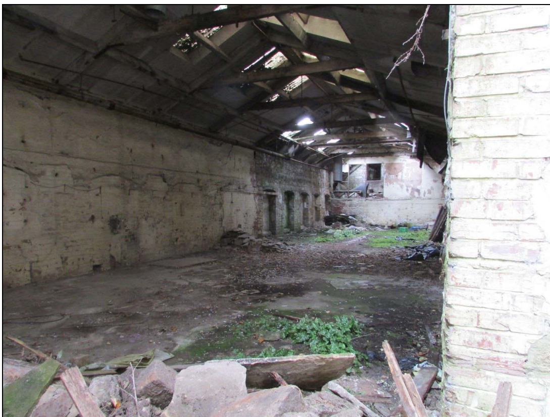
Plate 80 General view of the interior of the eastern and middle sheds. A machine made brick and timber division is visible in the background. Also visible are the former windows which were blocked subsequently
