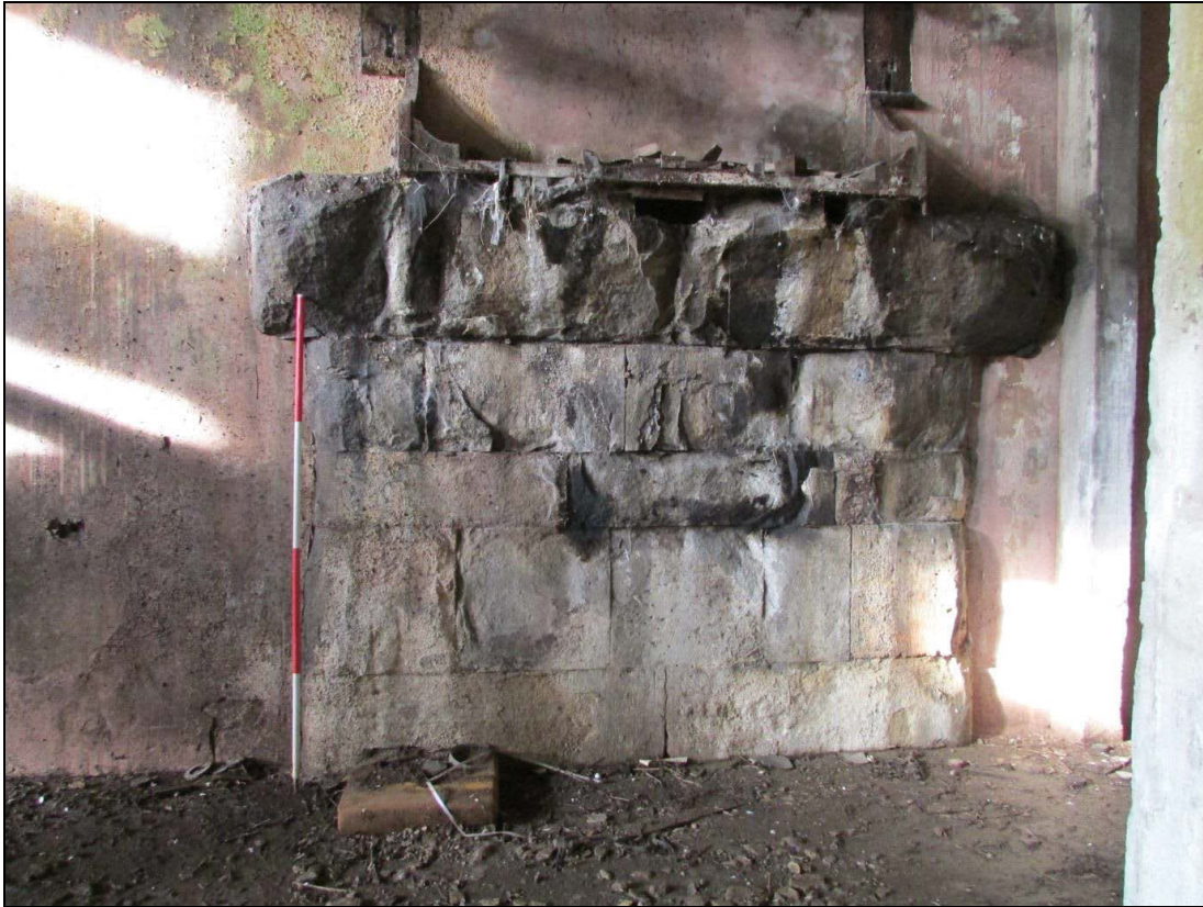
Plate 11 Projecting stone pier supporting footstep bearing for driveshaft
