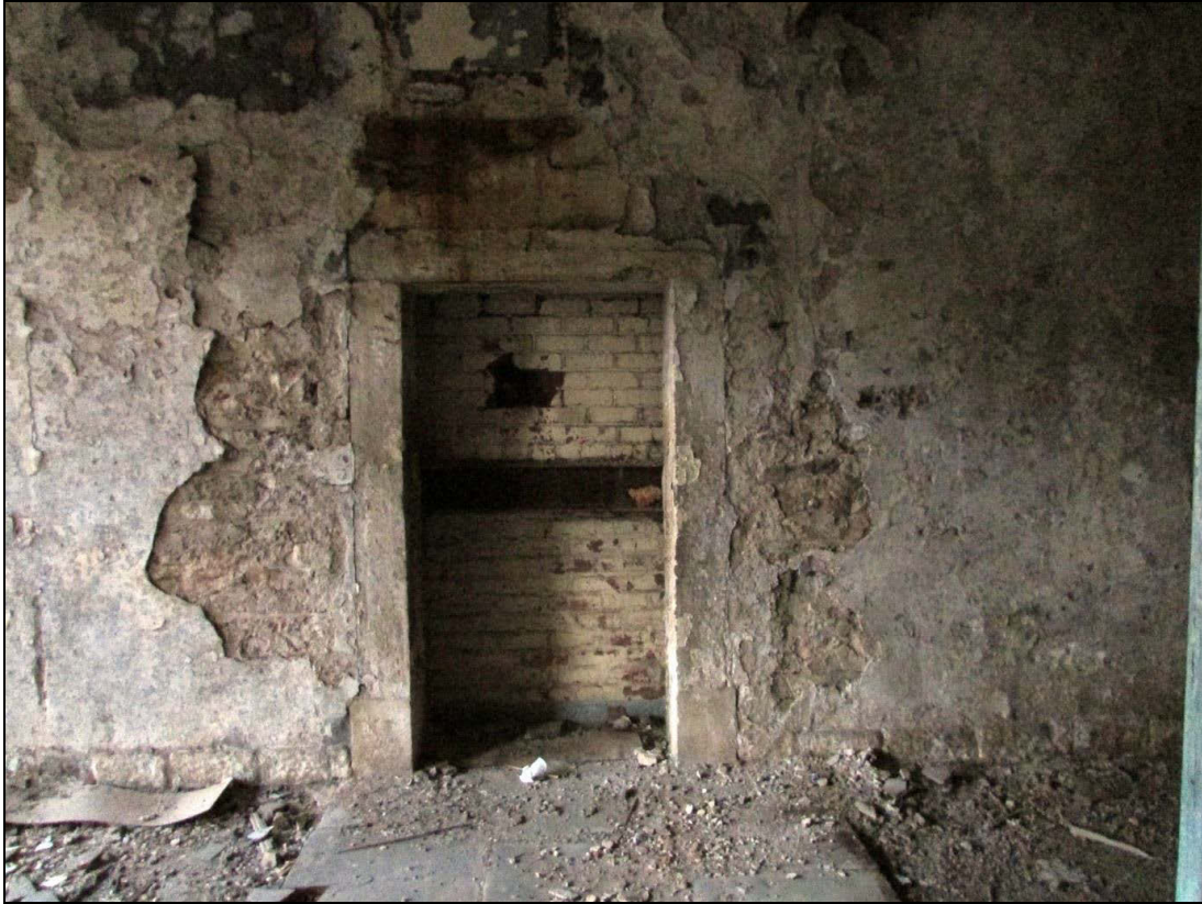
Plate 50 Blocked entrance which would have connected the engine house with the other spinning mill
