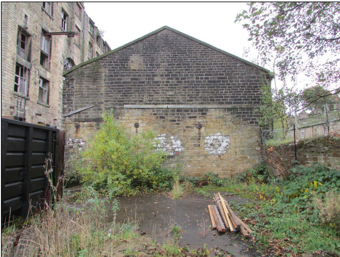
Plate 85 Western elevation of the west shed. A blocked entrance/window can be seen in the top left corner as well as the outline of where another shed abutted
