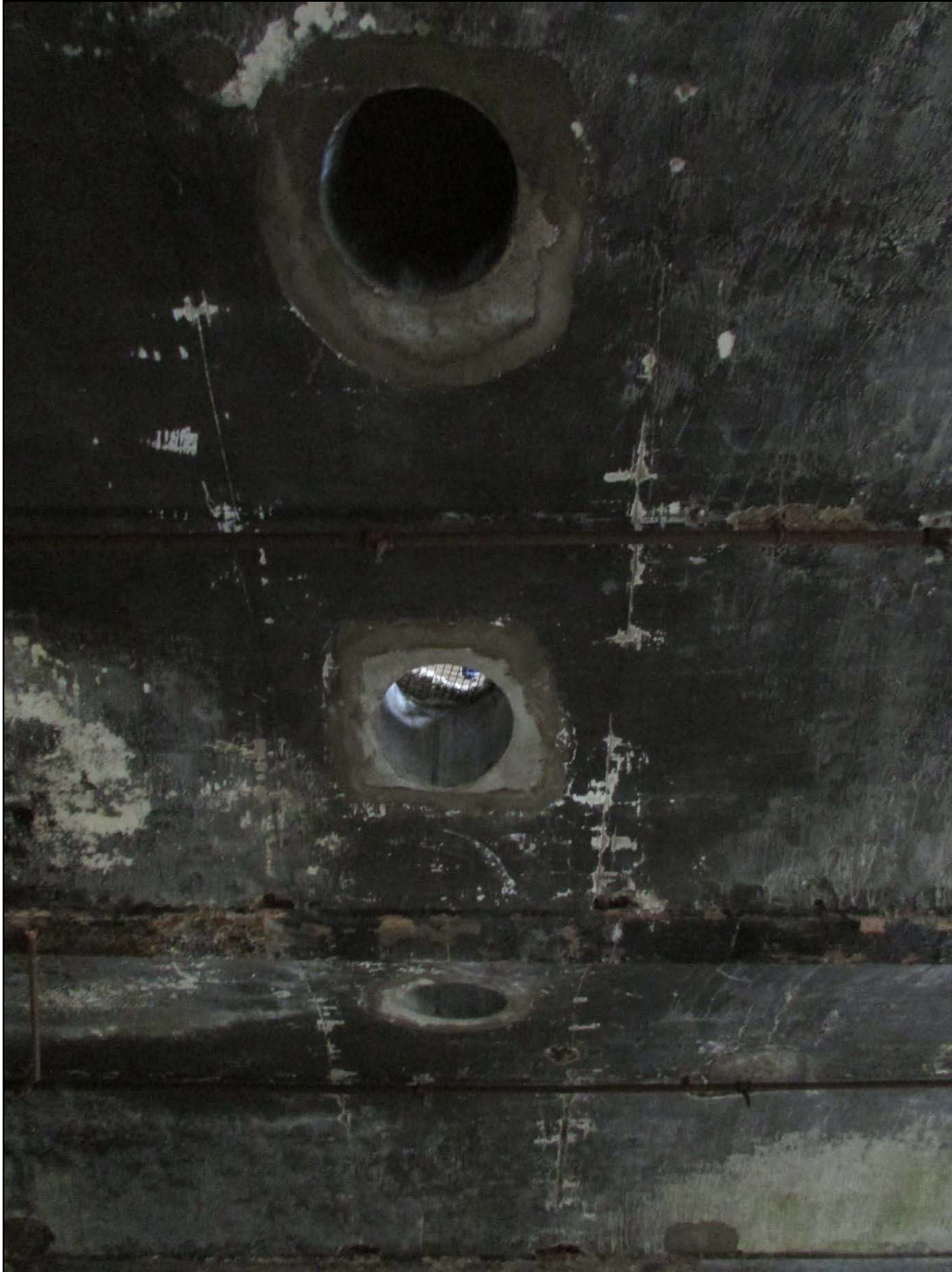
Plate 15 Small circular apertures inserted at a later date into the first-floor ceiling
