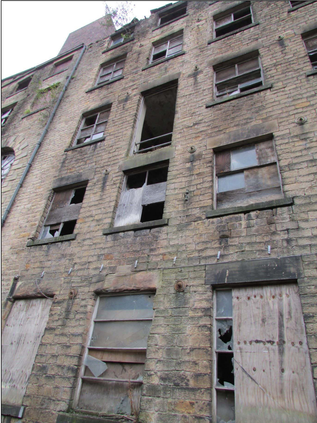
Plate 2 The modified second-floor window (in the middle)
