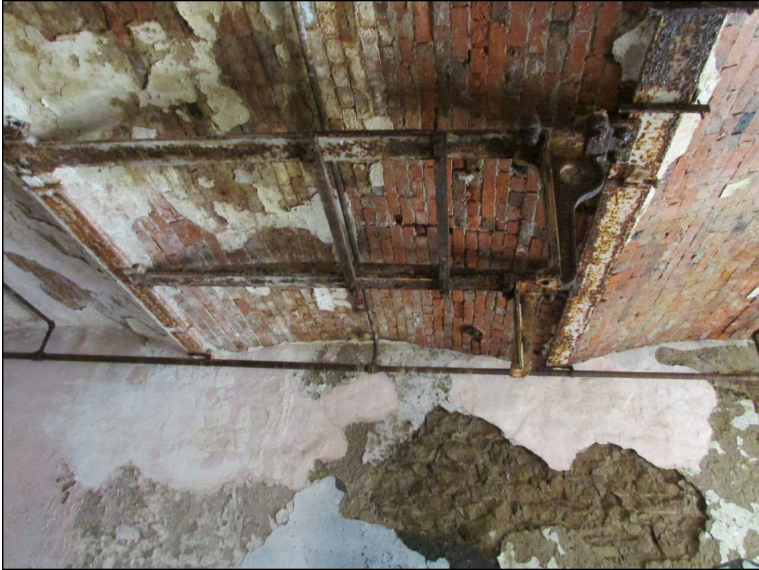
Plate 54 Original metal fixtures associated with goods movement, fixed to the ceiling
