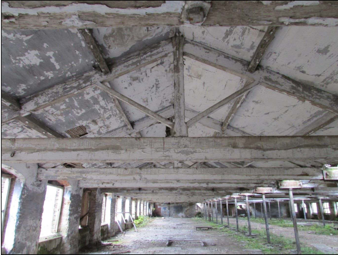
Plate 29 One of the three pitches spanning the roof showing the king post style structure
