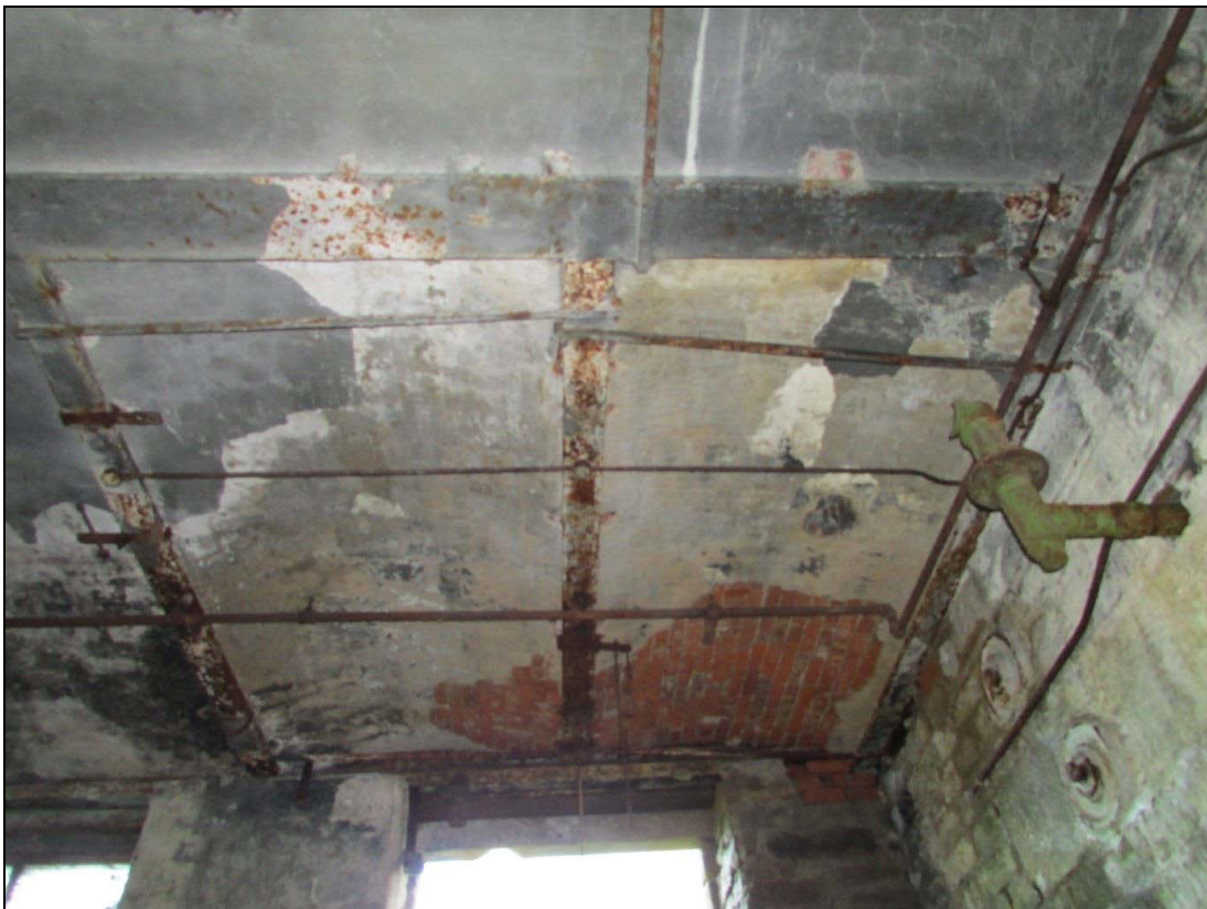
Plate 46 Fireproof arched ceiling located above the stone/concrete beds
