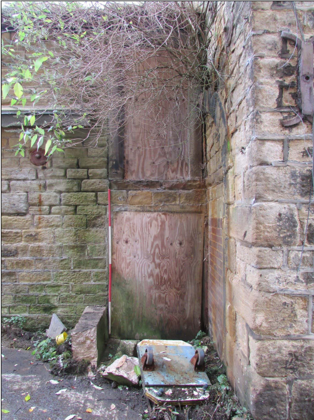
Plate 84 Boarded entrances into the middle shed
