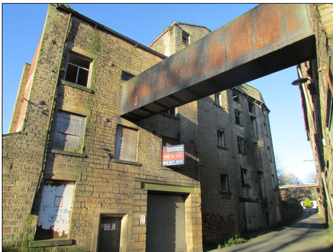
Plate 64 Eastern elevation of the office block, with the later metal walkway visible (access was not possible during the survey – this photo dates to December 2014)
