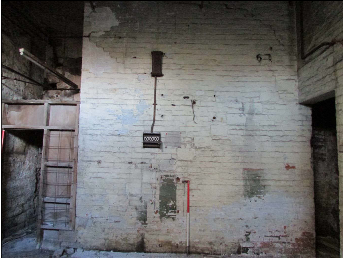
Plate 44 Later staircase inserted into the engine house
