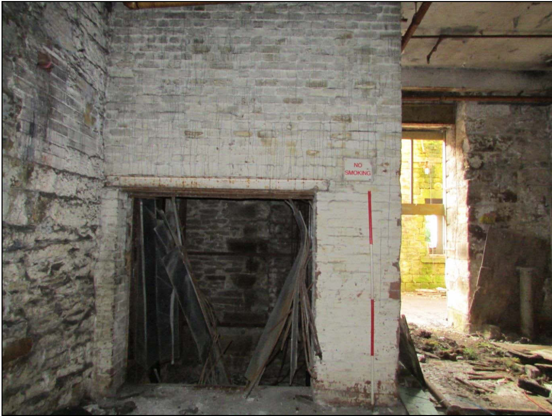
Plate 42 Later 20th century lift shaft inserted into the engine house
