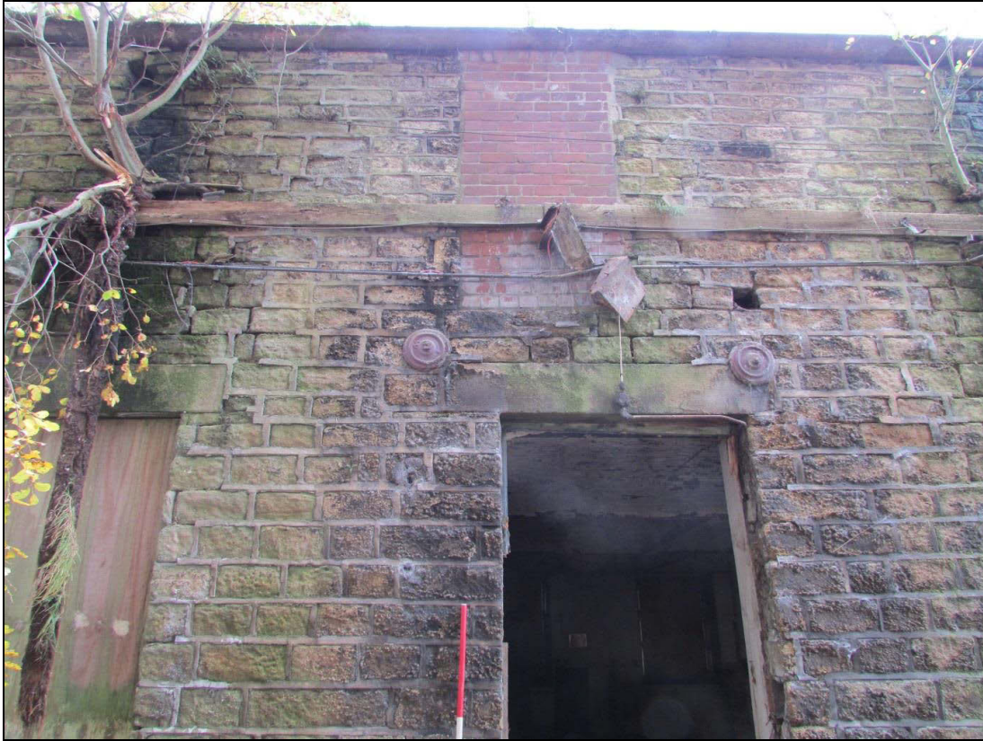
Plate 87 A possible blocked window is visible above the entrance to the west shed
