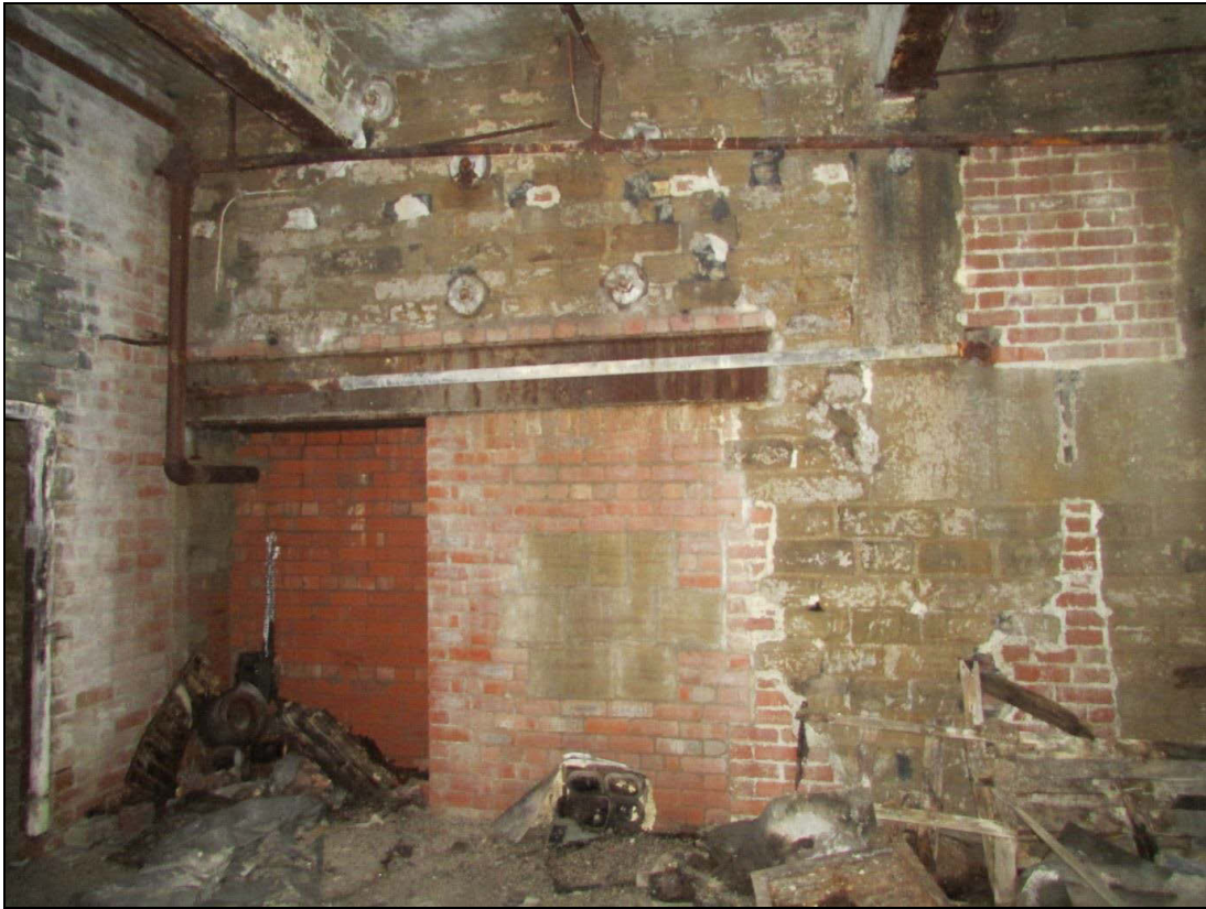
Plate 48 Later inserted doorway, which was then blocked and a blocked footstep bearing for another upright shaft (see also Plate 16 for the bracket on the other side of the gearing wall)
