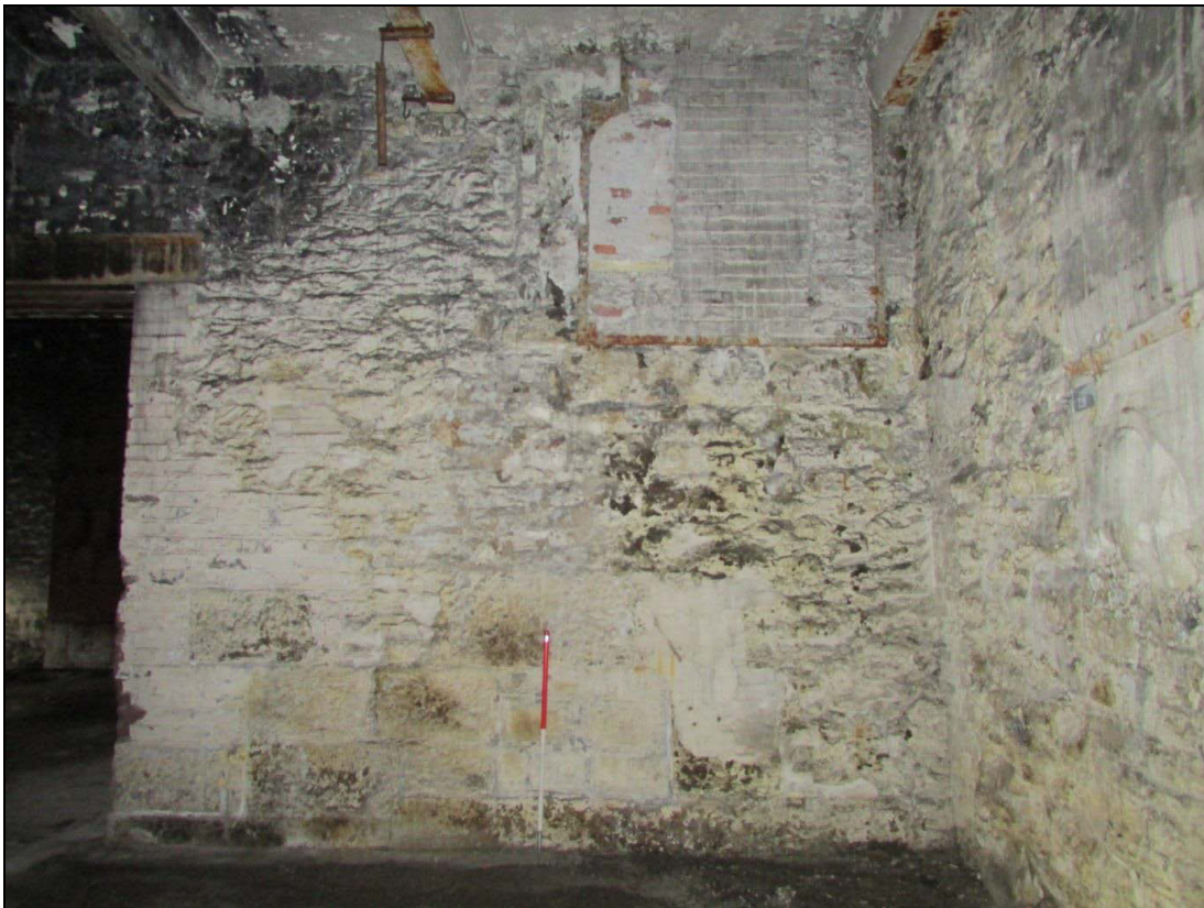
Plate 38 Although plastered over, the dividing wall of the engine house consists of mixed stone coursing types, including random rubble and coursed ashlar blocks. Also shown is a bearing box for the power transmission
