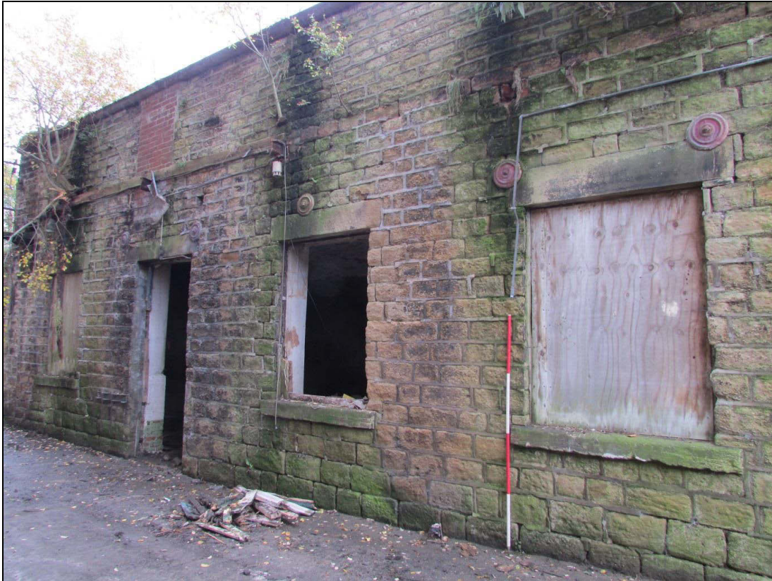
Plate 86 General view of the west shed northern elevation
