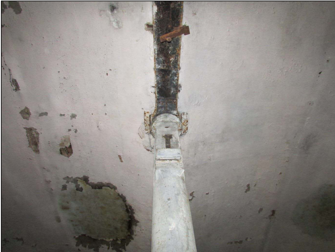
Plate 8 Close up of a column with a bolting face, supporting the line shaft
