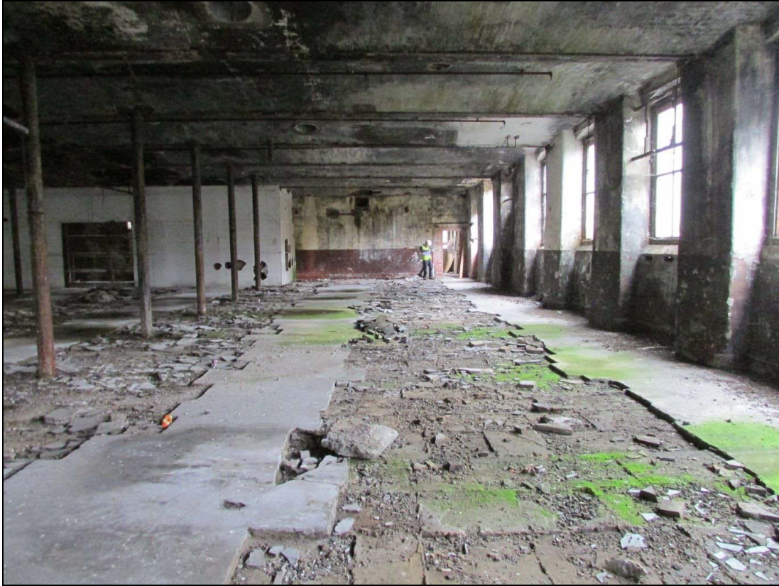
Plate 13 Robbed out flagged flooring on the first-floor
