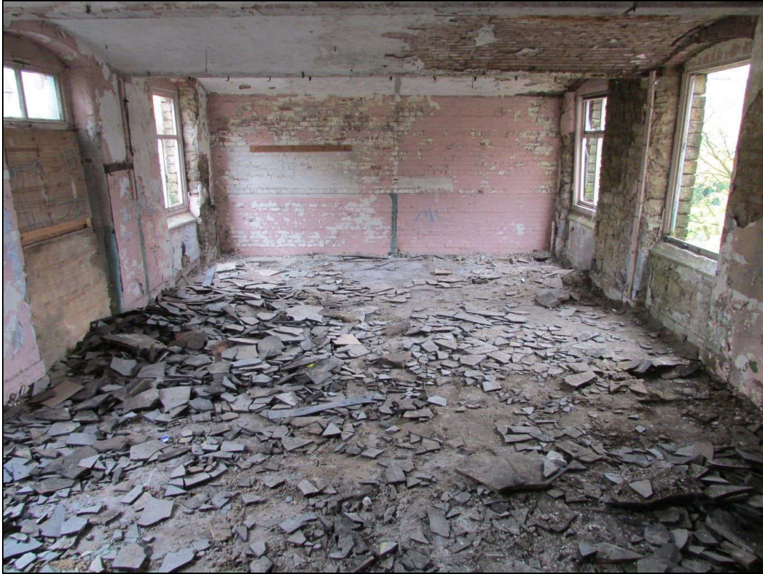
Plate 72 General shot of the Office Block-second floor
