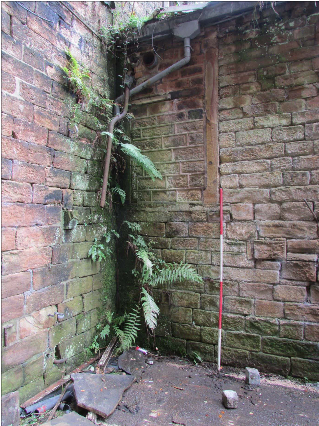
Plate 76 Blocked window within the northern elevation of the east shed
