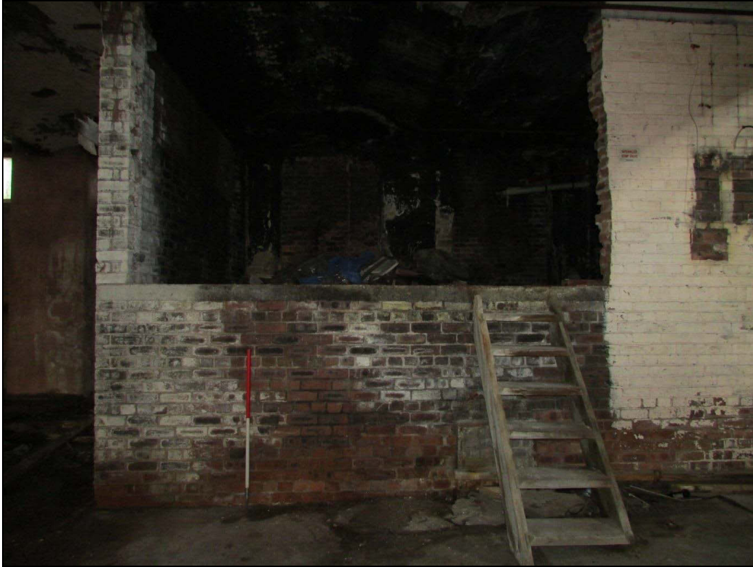
Plate 9 Later machine made brick sub-divisions in the north-east corner of the mill included this storage area and a toilet block to the east
