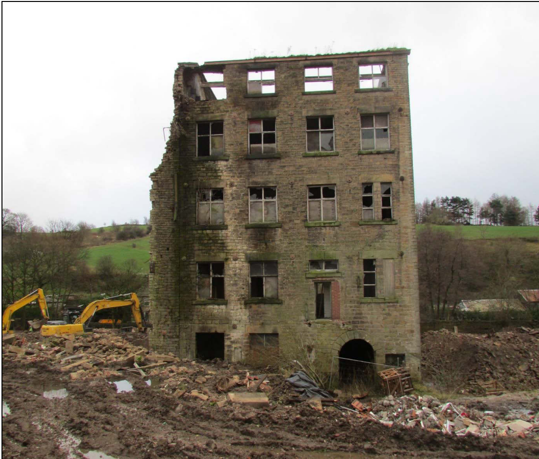
Plate 34 Northern elevation of the engine house
