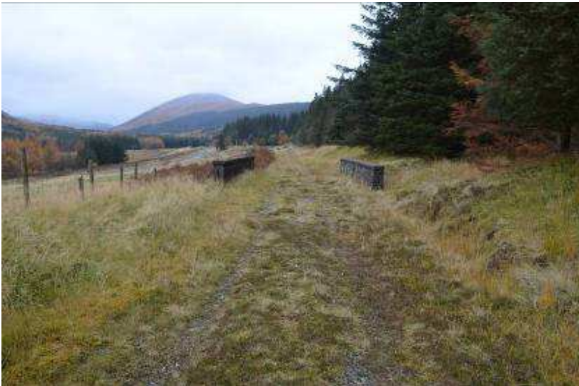
Photo 76: Section 4 general photograph.
