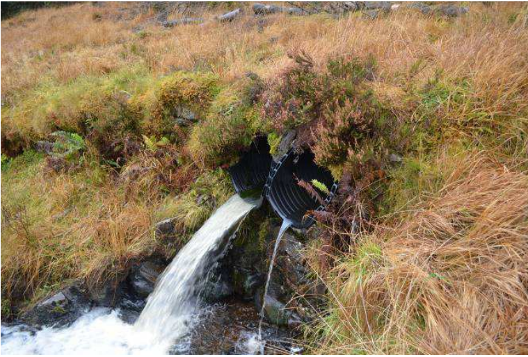
Photo 107: Culvert/Bridge [09] with modern pipes inserted.
