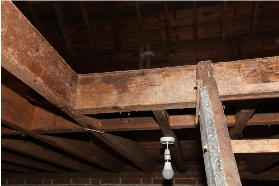
Illus. 11. A detail from the west of the granary's ladder trap showing the apparently original tenons of the framing joists. The trimmer supporting the ladder is through-tenoned and pegged at both ends.
