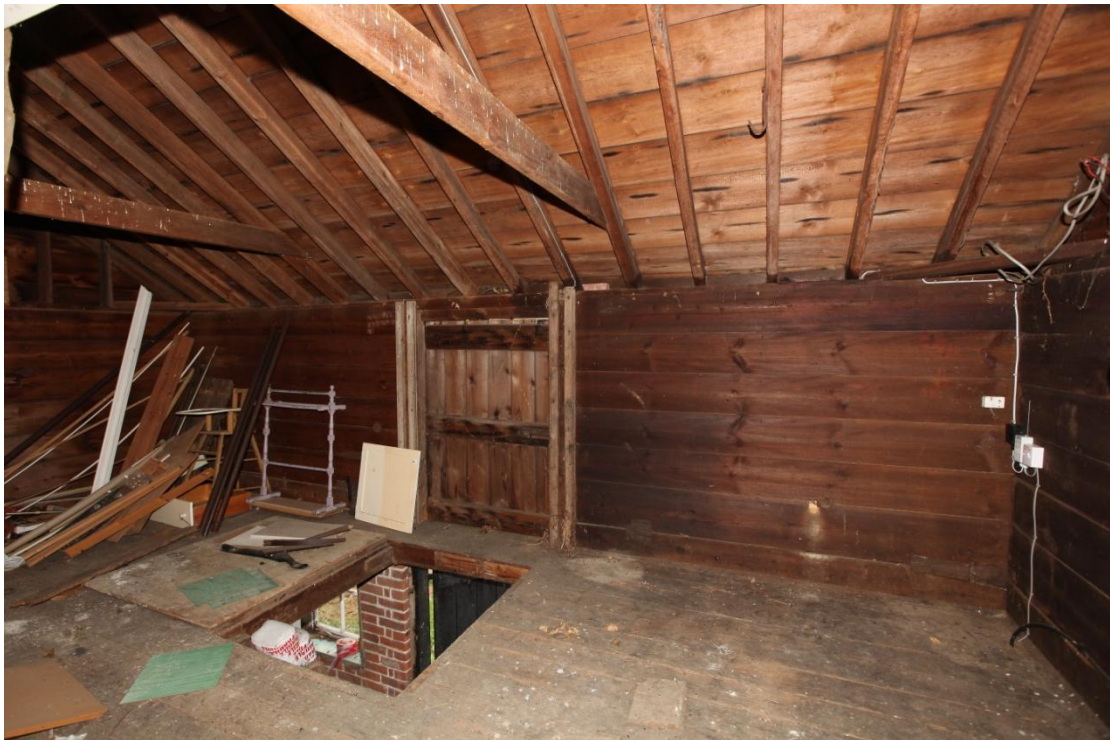
Illus. 12. The western interior of the grain loft showing the vertical grooves for missing bin partitions flanking the loading door. The interior is clad in deal boards with later staining and the original softwood roof structure consists only of coupled rafters with a ridge board and two nailed collars.
