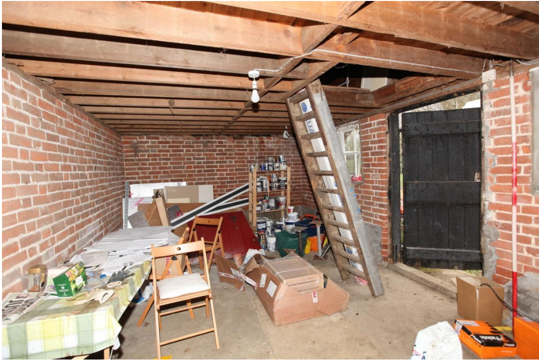
Illus. 9. The lower storey of the granary from the north showing its featureless interior with a concrete floor and ceiling of tall-sectioned softwood joists. This space was probably used for the milling and storage and animal feed.
