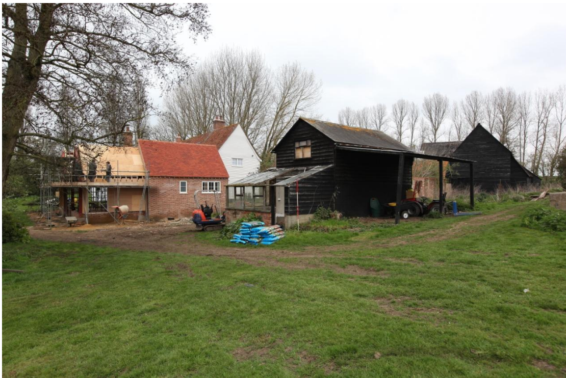
Illus. 2. A general view of the site from the south-east showing the slate-roofed granary (1) in the centre with the house (2) and aisled barn (3) to the left and right respectively.
