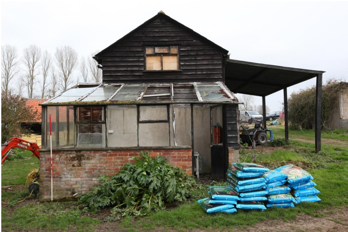
Illus. 4. The granary (1) from the south showing the 20th century lean-to greenhouse against its gable and the 20 th century tractor and implement shelter projecting from the rear (eastern) wall to the right.
