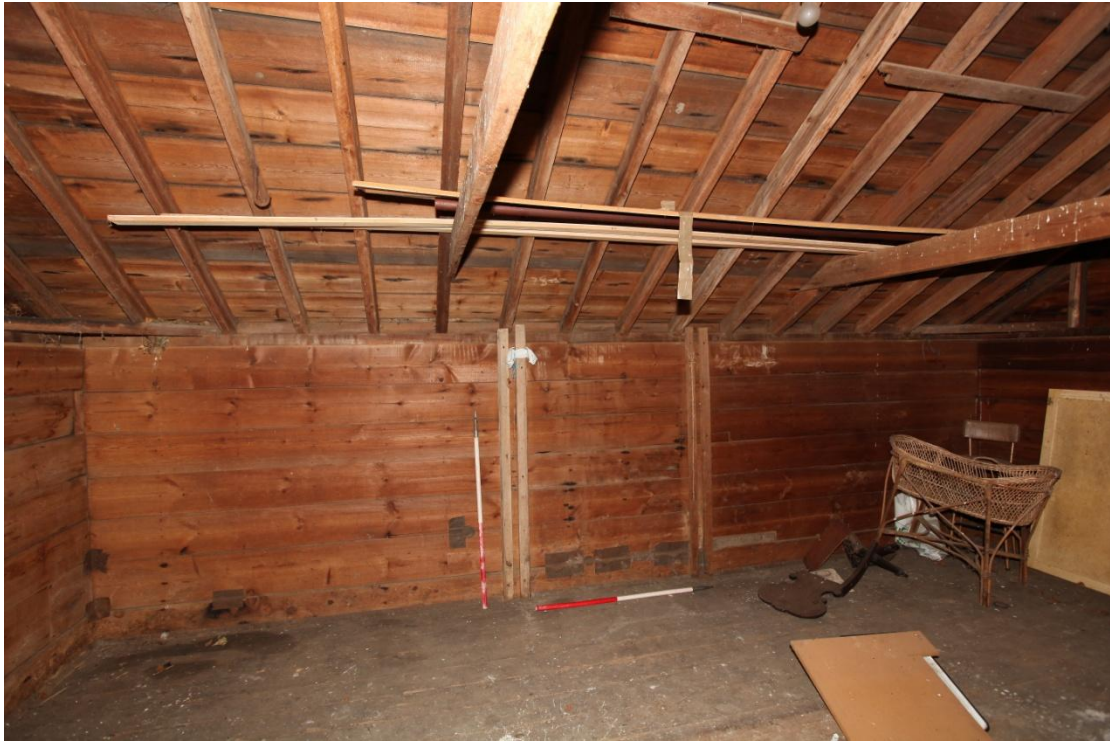
Illus. 13. The eastern interior of the grain loft showing the vertical grooves for missing bin partitions opposite the loading door.
