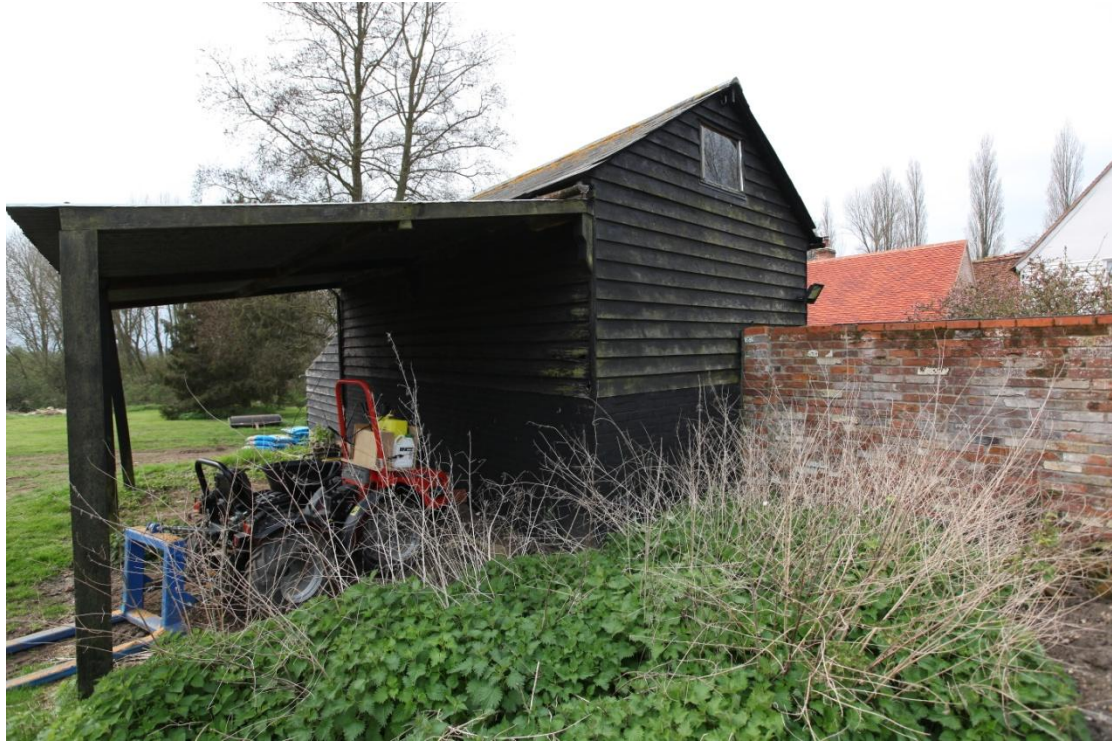
Illus. 7. The granary from the north-east showing its tarred northern gable and the 20th century lean-to implement shelter against its rear wall.
