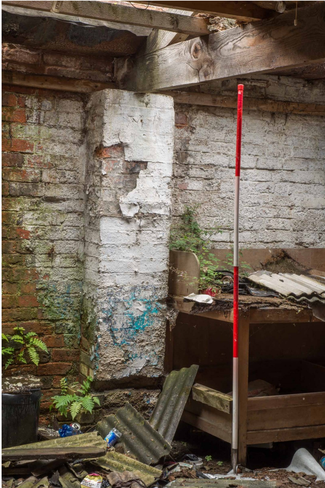
Figure 17. Wall shaft supporting the Drying Shed roof.
