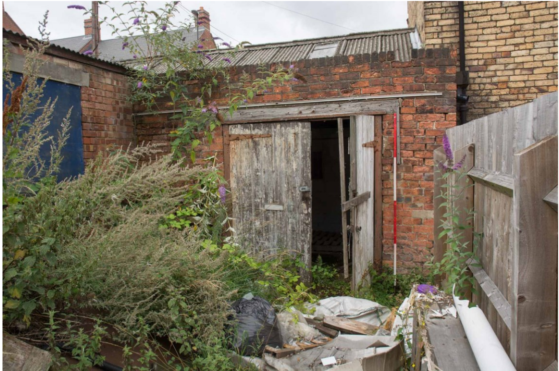
Figure 13. The Drying Shed entrance, looking west.
