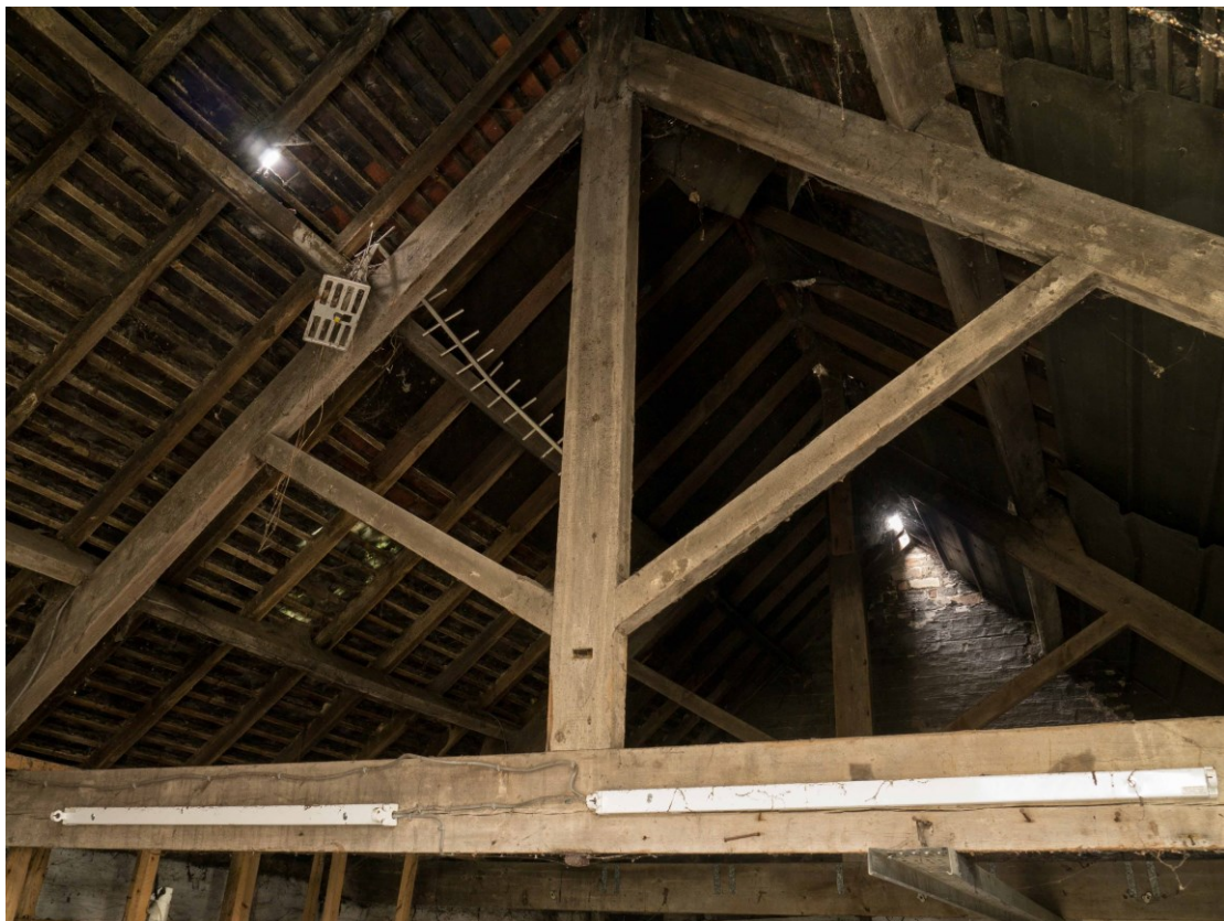
Figure 19. Roof truss of the Saggar House.
