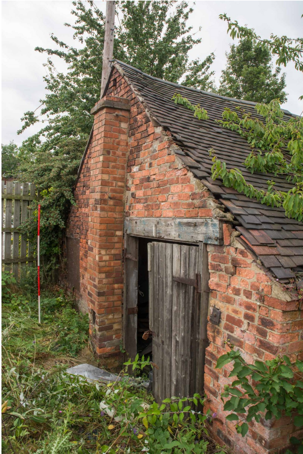
Figure 14. The Sagar House, looking south-west from the yard.
