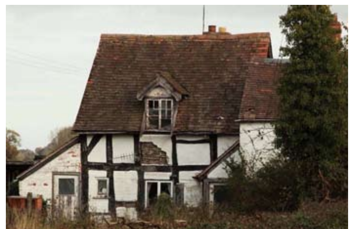
Wattle and daub. Photograph © Worcestershire County Council.
