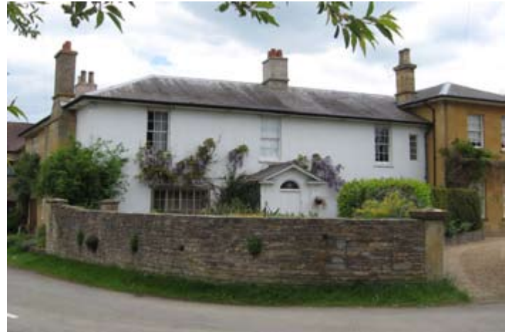
A late Georgian façade on a potential 16th or 17th century house (indicated by the off centre chimney stack). Deep eaves, sash windows and a pedimented porch. White stucco at the front, with Cotswold ashlar at the side, and a slate roof.
