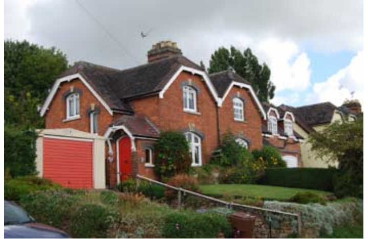
Red brick cottages, associated with the Amphlett Estate. Dated 1872 - 73. The roof is half hipped and the ground floor has blue brick forming a four-centered arch opening above windows.
