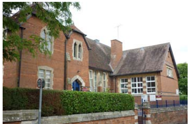
This school with attached house, in Crowle, reflects the influence of the Gothic style in mid 19th century design. Photograph © Worcestershire County Council.
