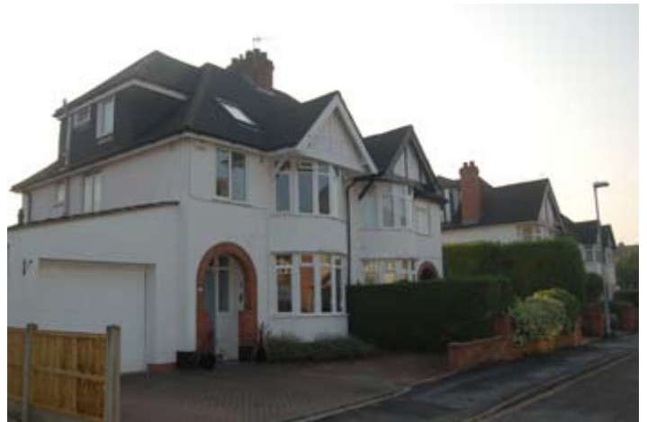
A pair of typical 1930s, semi detached houses with their simple plan form, round bay windows and arched porches. Photograph © Worcestershire County Council.
