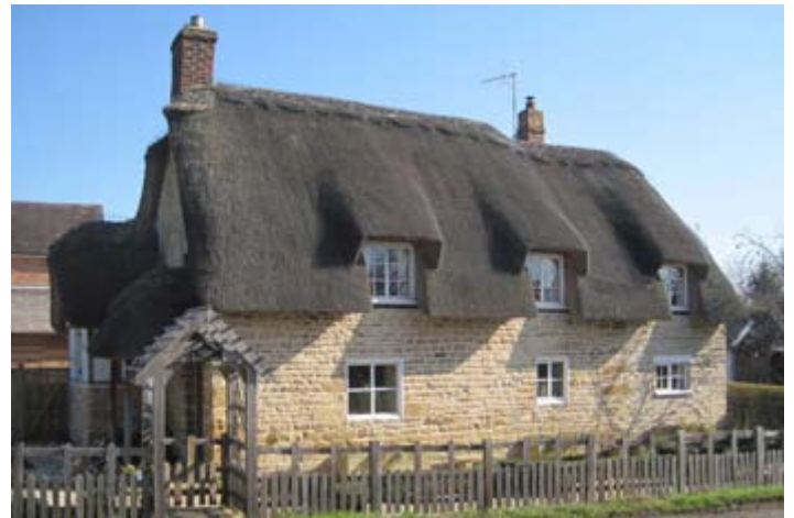
A thatched cottage constructed of coursed limestone.
