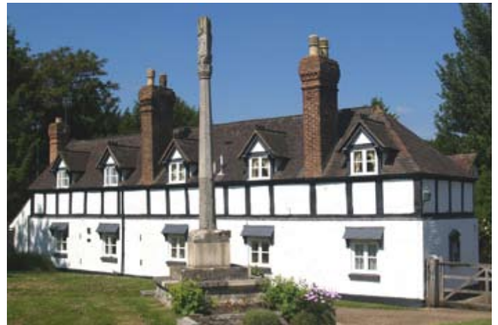
Almshouses in Hanley Castle. Possibly mid-19th century with 18th century remains. Brick with a band of timber-framing below the eaves. Photograph © Worcestershire County Council.
