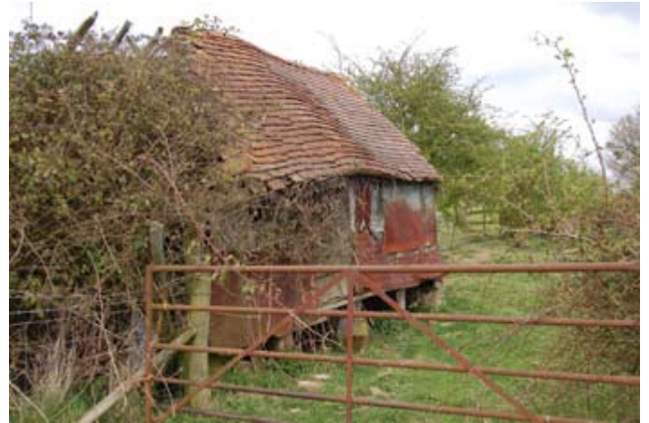
A fruit store at Crowle, raised above the ground to keep the crop dry. Photograph © Worcestershire County Council.
