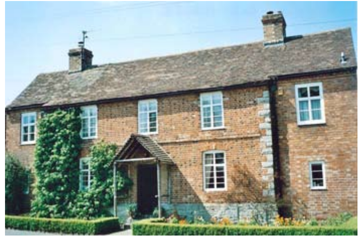
Early 18th century brick house with a stone plinth and quoins, and a tile roof. Photograph © Worcestershire County Council.
