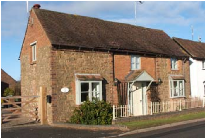
This former threshing barn in Martley, dates to around 1750 and is built of local red sandstone and brick, with a handmade tile roof. Photograph © Worcestershire County Council.
