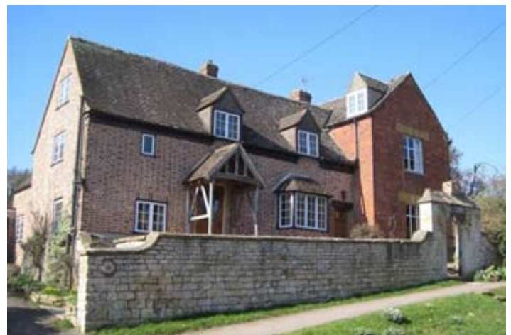
Mid 19th century red brick dwelling with later north wing addition. Tiled roofs with gable dormers. Formerly 'Charity Farm' which belonged to the Deacle charity school at Bengeworth, Evesham.
