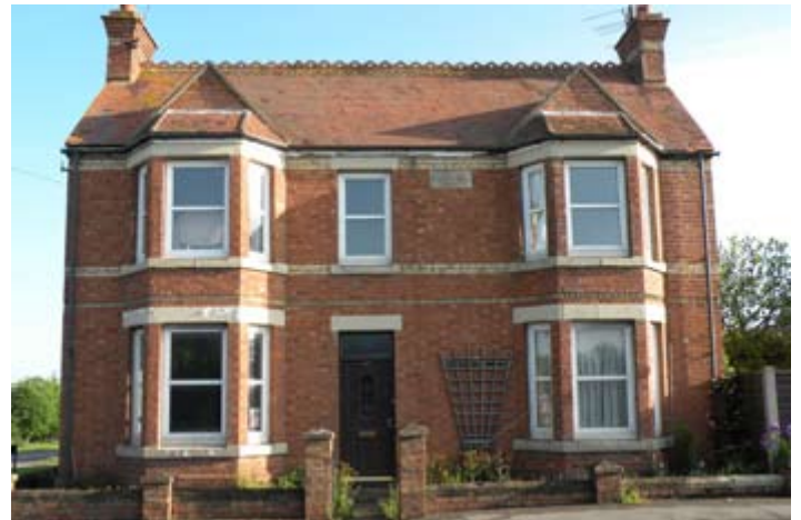
Late Victorian brick house. Photograph © Worcestershire County Council.
