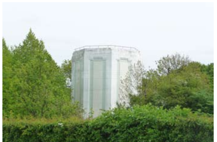
This 1933 octagonal, reinforced concrete water tower with its Deco panels, is an eye catching sight at Long Bank, Bewdley.
