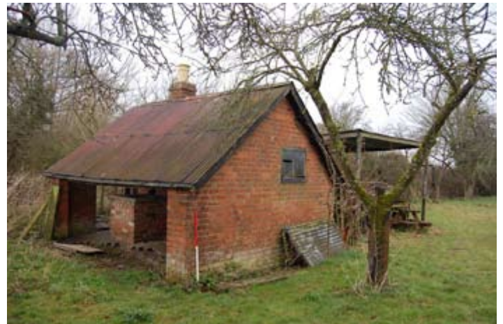
Old Ordnance Survey maps often record 'field barns' in areas of traditional orchard. This open-fronted late 19th century building at Birlingham has a chimneystack which serves a copper. This was probably used to heat and soften withies for making baskets, and in addition might have heated drink and food for orchard workers. Such modest structures are an integral and locally-important part of the county's historic landscape. Photograph © Worcestershire County Council.
