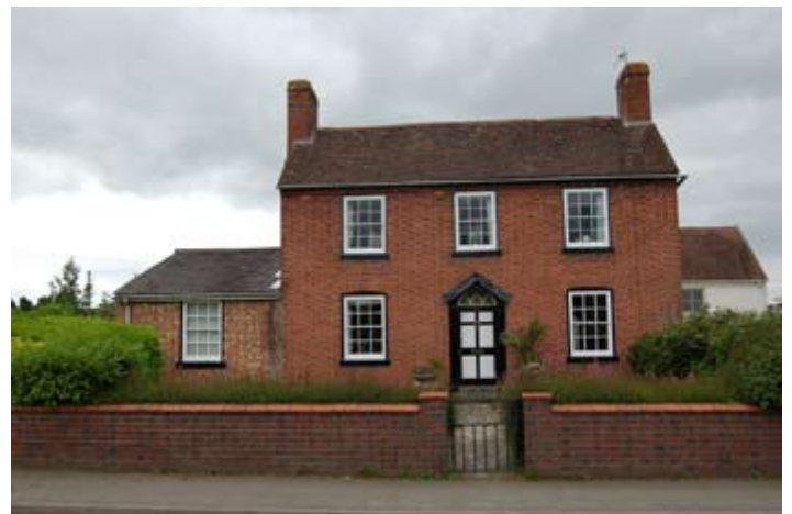
This early 19th century, two storey, red brick house has a symmetrical façade, sash windows and a classical door case with a contrasting Gothic fanlight. The house, which faces the road, looks into its own enclosed private garden.
