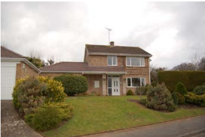
1960s housing is characterised by its simple style with large front picture windows, flush exterior doors and shallow pitched roofs. Photograph © Worcestershire County Council.
