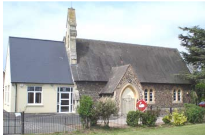
The original building at St Gabriel's School in Hanley Swan dates to 1862 and is constructed of irregular Malvern stone. The window's are situated within sandstone frames and the projecting gable porch a sandstone archway. The large stone structure on the southern gable end is a bellcote. Photograph © Worcestershire County Council.
