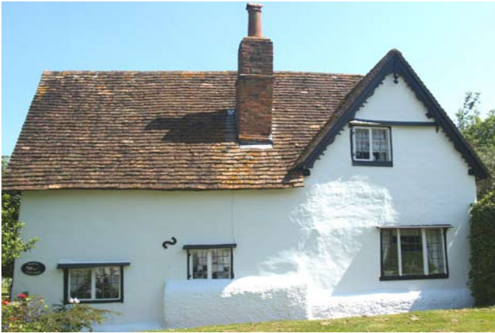
Concealed timber framing. Photograph © Worcestershire County Council.
