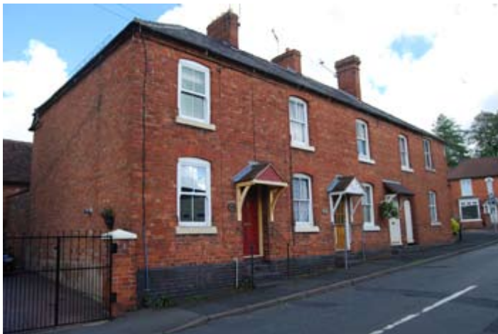
Mid Victorian red brick, double depth terraces. Each cottage has one bay and two storeys. Photograph © Worcestershire County Council.
