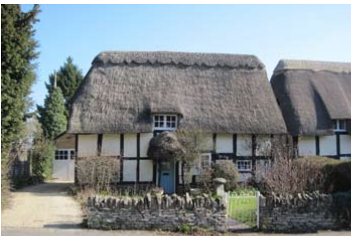
Square panelling with brick infill. Photograph © Worcestershire County Council.
