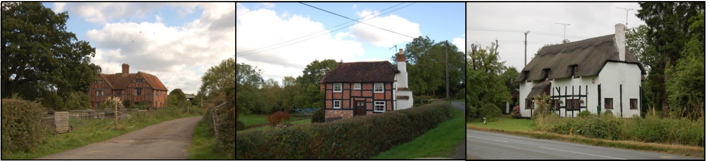
Photo 1: A prestigious late 16th or early 17th century timber-framed farmhouse in Hanbury. Like, many high-status rural and urban houses of this period, the house displays close studding on its main façade – facing the road – in a clear demonstration of wealth and status. Photo 2: A small scale, 17th century, cottage down Littlewood Lane. Smaller scale dwellings, dating to this period, are more prevalent in marginal landscapes, with small scale fields, woodland and heath. Photo 3: A small scale, 17th century, timber-framed cottage that has been raised to accommodate a second storey. Photographs © Worcestershire County Council.
