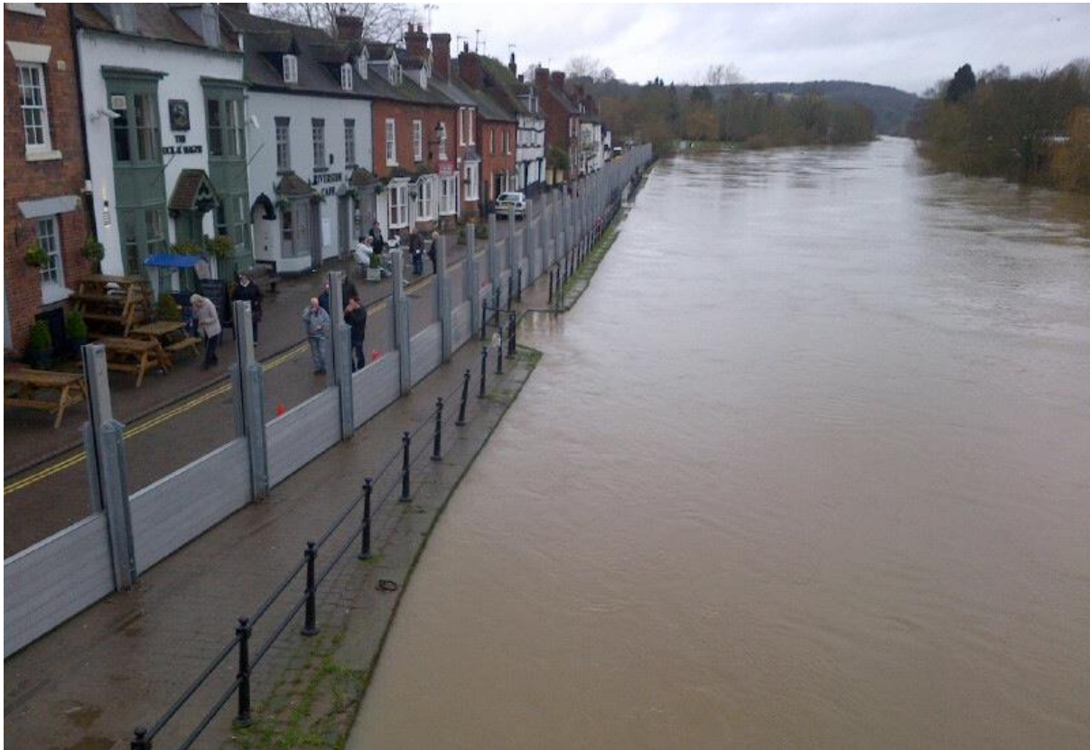
Figure 10: Environment Agency demountable defences in action at Bewdley. © Dave Throup
