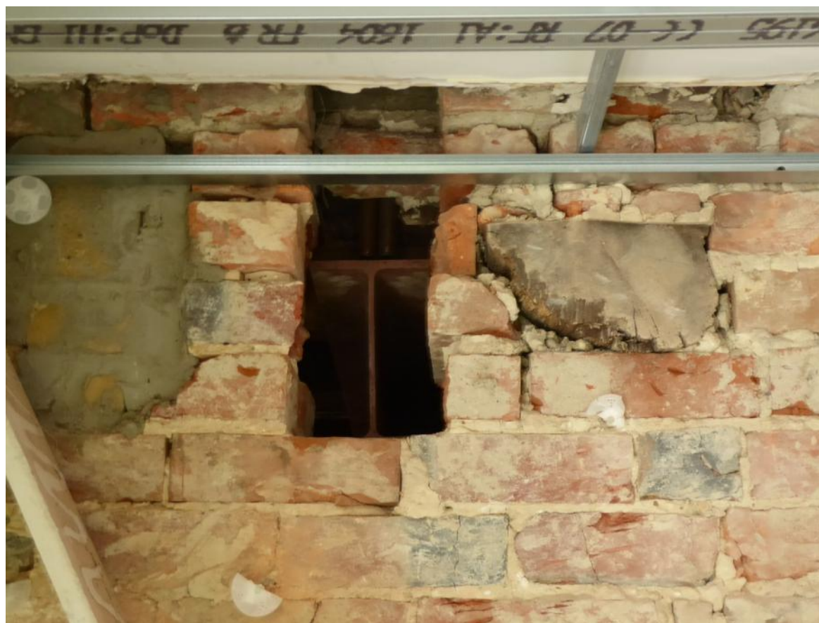
Fig 4.1.4; end of steel beam within north wall
