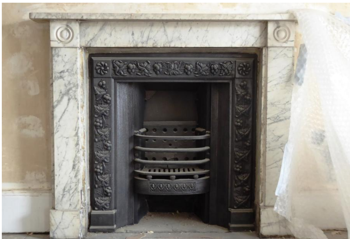
Fig 4.23.3; rebuilt marble fireplace
