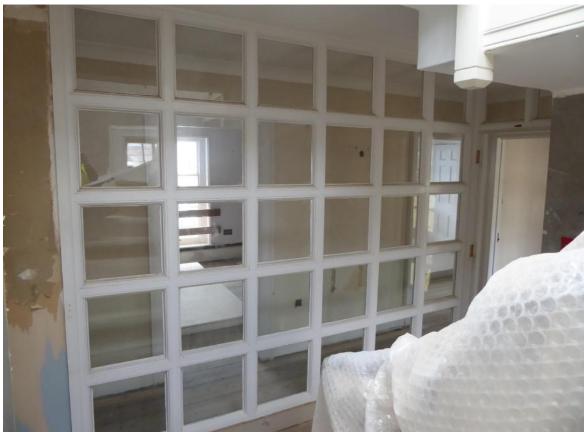
Fig 4.21.1; timber frame glazed screen
