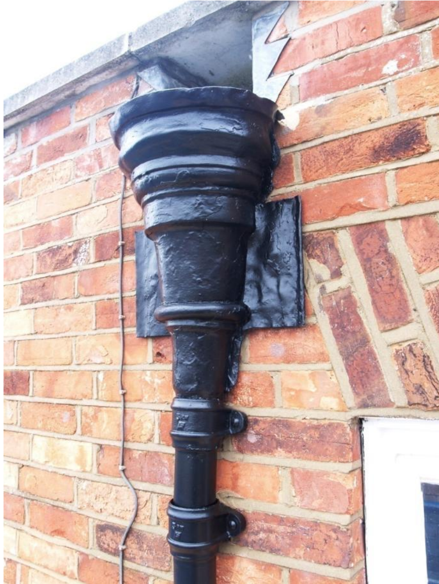
Fig 3.4.2; Hopper head to rear of building
