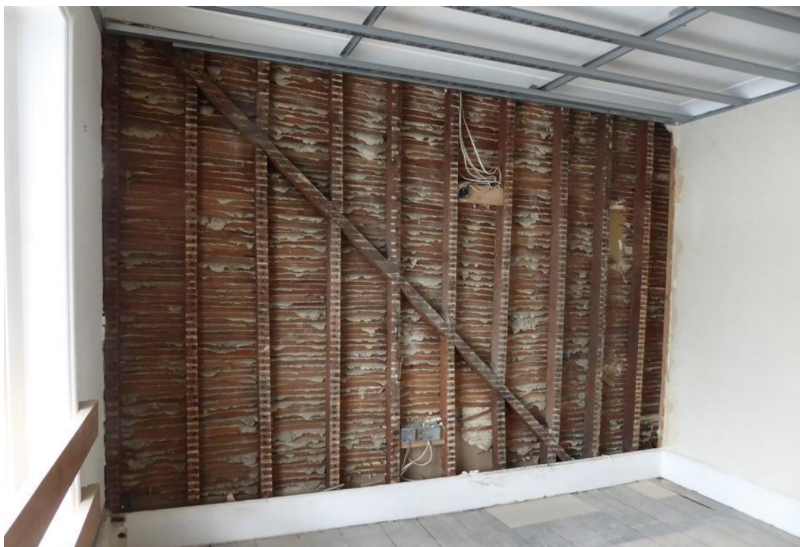
Fig 4.24.1; exposed lath and plaster walls
