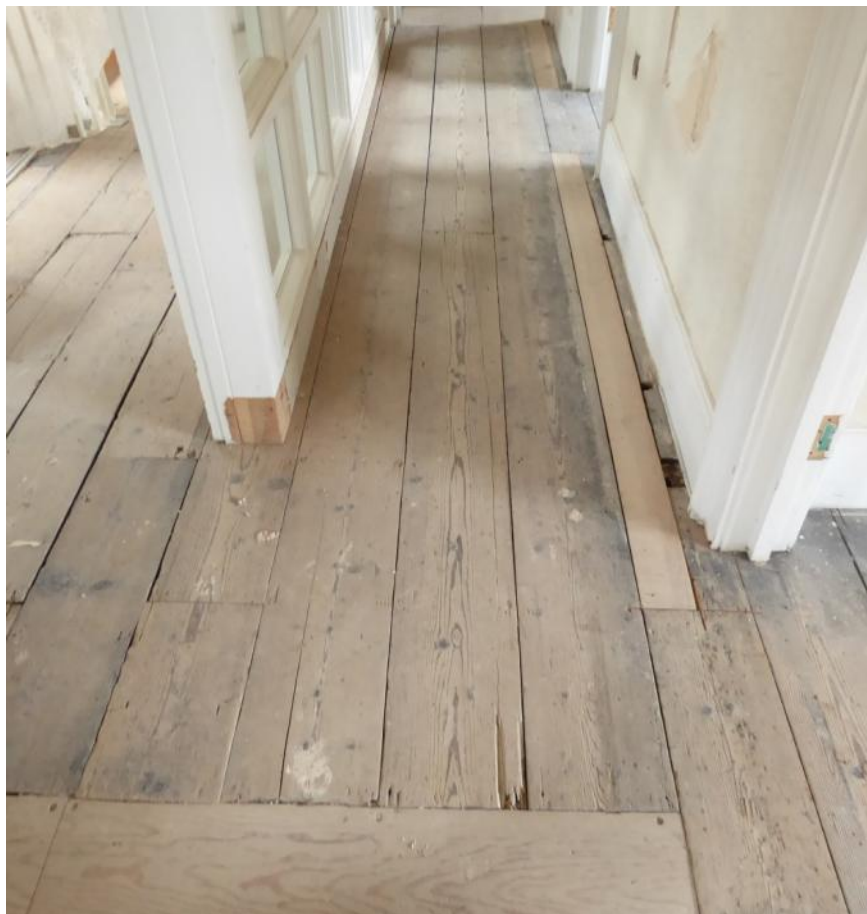
Fig 4.22; light floor boards showing where original wall would have been
