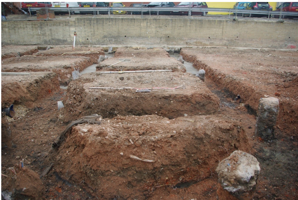
Fig 6. Northwest side of site showing maximum depth of excavation of ground beams.
