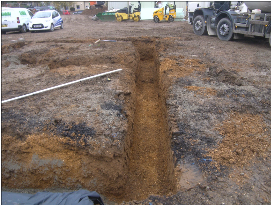
Plate 1: South-eastern foundations viewed from the east showing depth of disturbance
