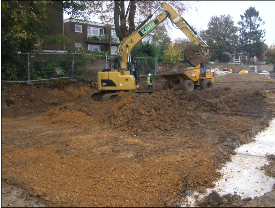
Plate 3: Stripping area in the north-eastern area of the Site showing River Terrace gravels
