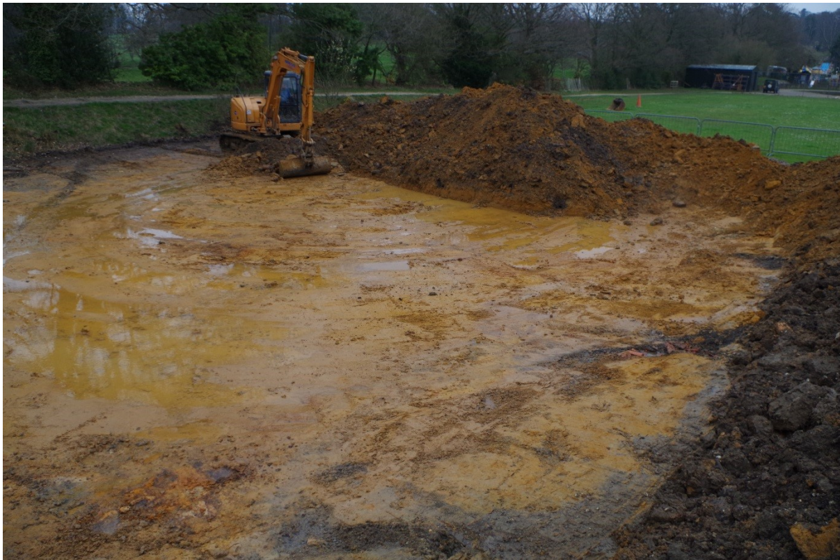
Figure 5. Excavation of the pond in progress, showing the London Clay.
