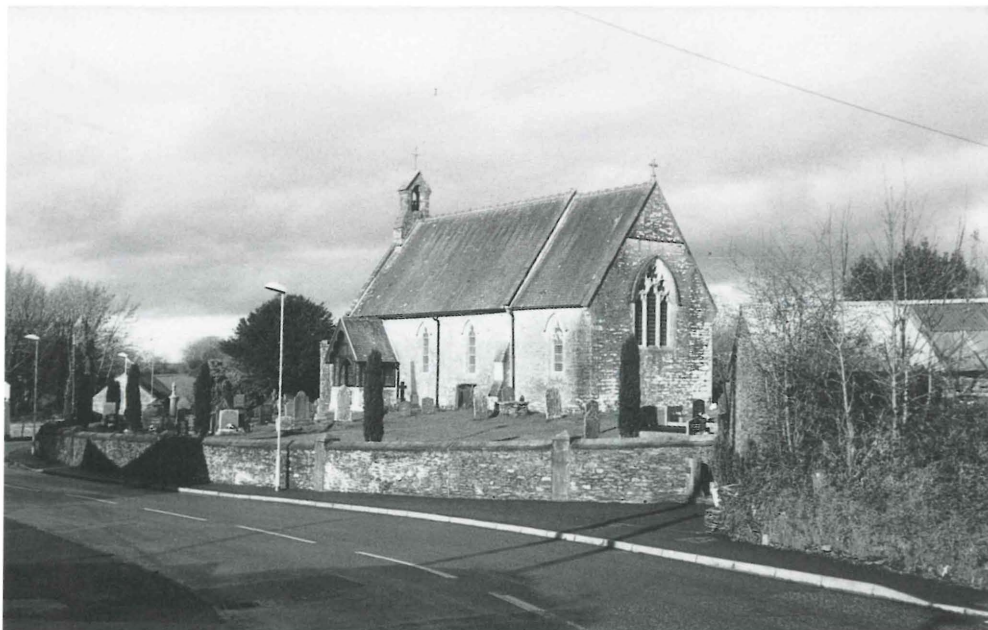
Fig. 14. The church of St Cristiolus, Eglwysrwr, from the south-east, after road-widening.
