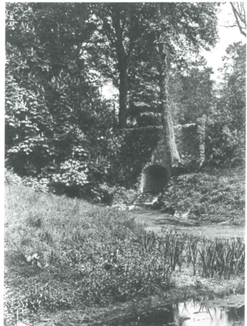
Plate 30. The Ham - Bridge on Drive. Edwin Miles photograph.
