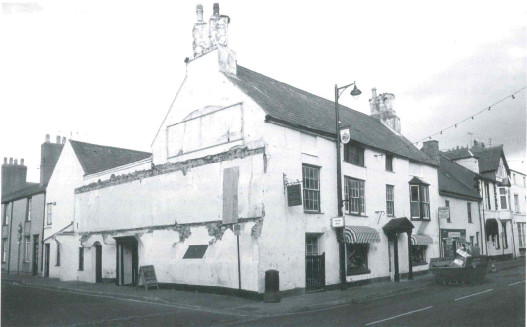
Fig. 7. No. 10 Castle Street, formerly a single house known as Ty Mawr, but converted into two premises by the early nineteenth century: a three-bay house facing Castle Street and a house with a single bay to Castle Street but the entrance in the return elevation to Rating Row. The corner premises was a tea rooms in the early twentieth century, when a balcony, taken down c. 2000, was added to the Rating Row elevation.
