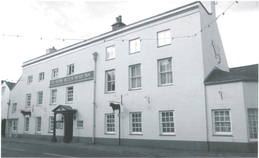
Fig. 3. The Old Bull's Head Inn. The oldest part of the present building is the left-hand section, which in its present form is dated 1766, although later heightened. The right-hand section was added in the early nineteenth century, as were the lean-to shops at either end.
