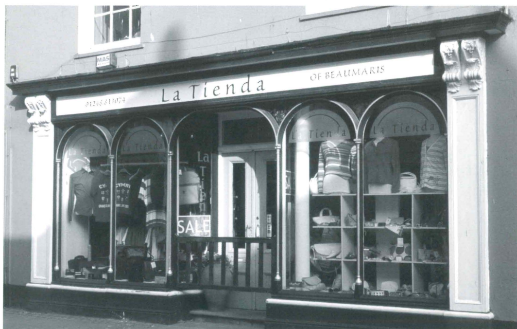
Fig. 15. Shop front to 33 Castle Street, originally Staples Grocers and Tea Dealers, of the early 1860s.
