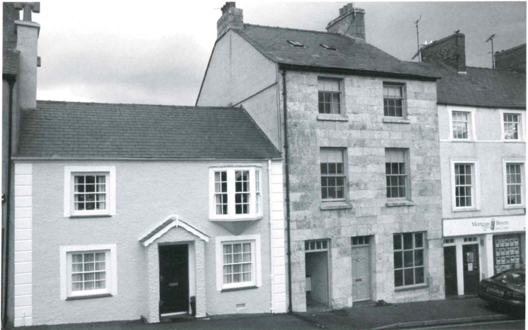
Fig. 8. Nos 24–26 Church Street. No. 26 on the left was the Prince of Wales public house by 1849. No. 24 on the right was built c. 1830 by Hansom and Welch, architects of York, and was one of the earliest houses in Beaumaris to incorporate a shop in the lower storey.
