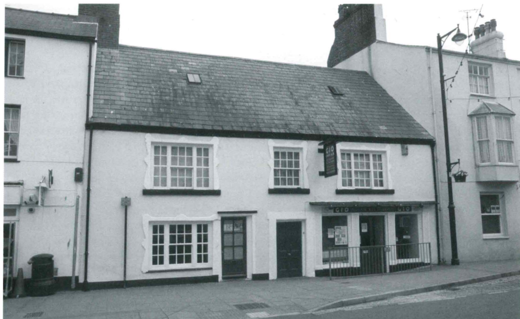
Fig. 5. No. 13 Castle Street, an eighteenth-century 3-bay house characterised by its steep roof and tripartite sash windows. The entrance left of centre, and the shop front to the right, were added in the late nineteenth century, dividing the house into two premises.
