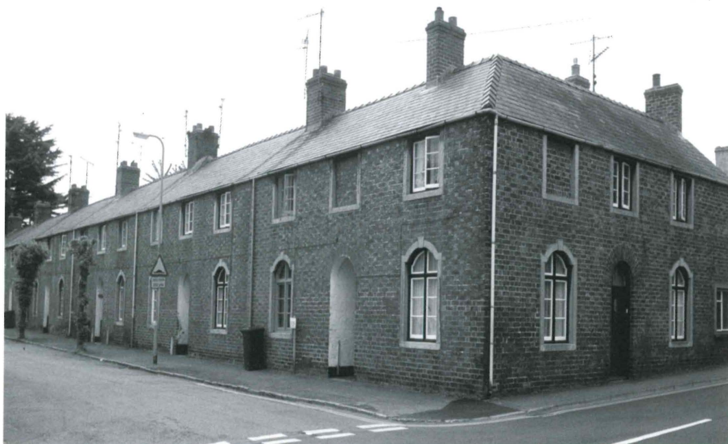
Fig. 18. Stanley Street, a Baron Hill estate terrace of the 1850s.
