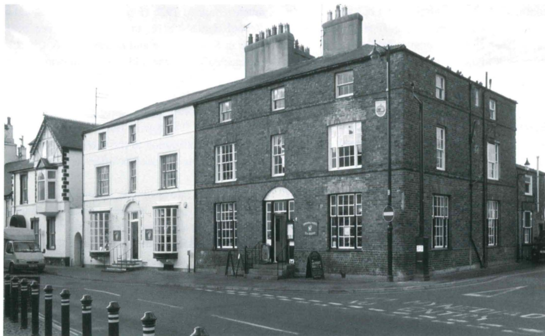
Fig. 6. Nos 2–4 Castle Street, both of which were houses converted for commercial use in the second half of the twentieth century.
