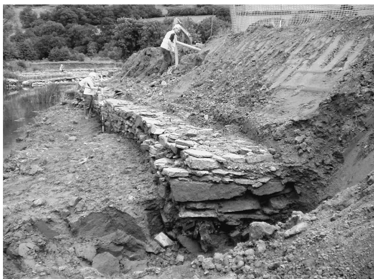
Fig. 5. View along wall 33, looking south-east.
