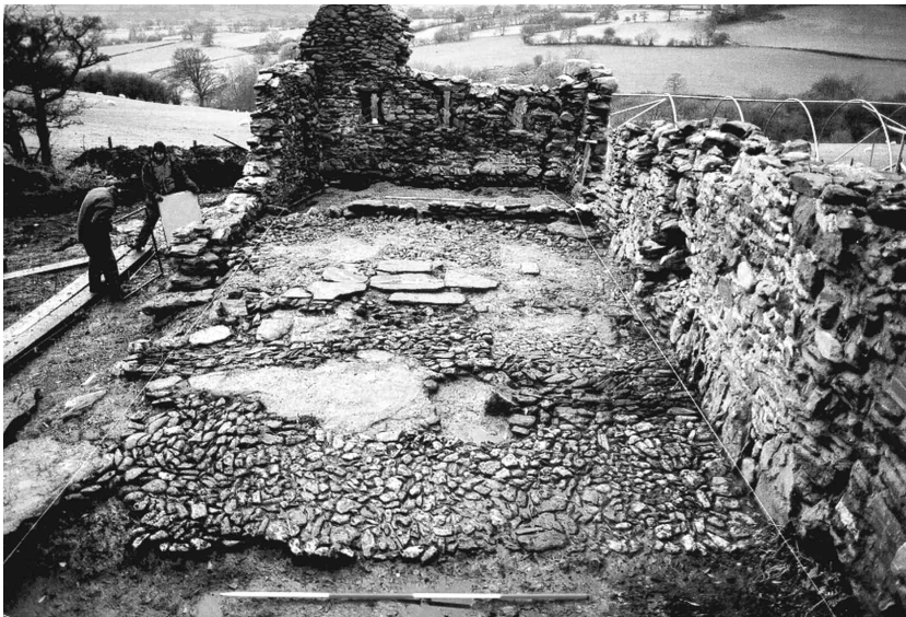
Fig. 14. Later cobbled and slab floors in Bays 2 and 3 (not shown on the published plans), concealing the foundations of the inserted chimney. The far sill wall divides Bay 4 from Bay 3 and is on the line of Truss B. The 2m ranging pole in the foreground is on the line of Truss D. Photograph CPAT 1319.2.
