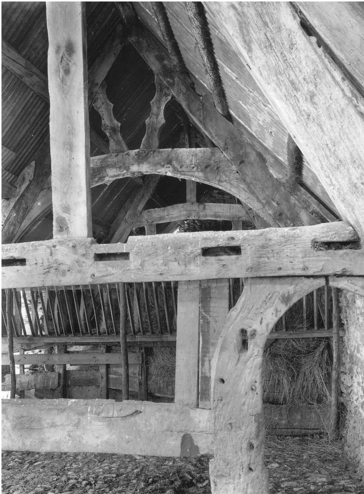
Fig. 7. Dais-end truss from the inner bay, looking south. View of part of the western end of the north face of Truss D, with the western doorway to the right and the mid-rail and tie-beam with mortise holes for the floor beams to the right, photographed in the 1950s. Part of the arch-braced central cruck-truss (Truss C) is visible beyond. © Crown Copyright: RCAHMW.
