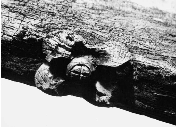
Fig. 9. Carved floral boss at the centre of the soffit of the central open truss. Photograph: CPAT CS02-013-024.
