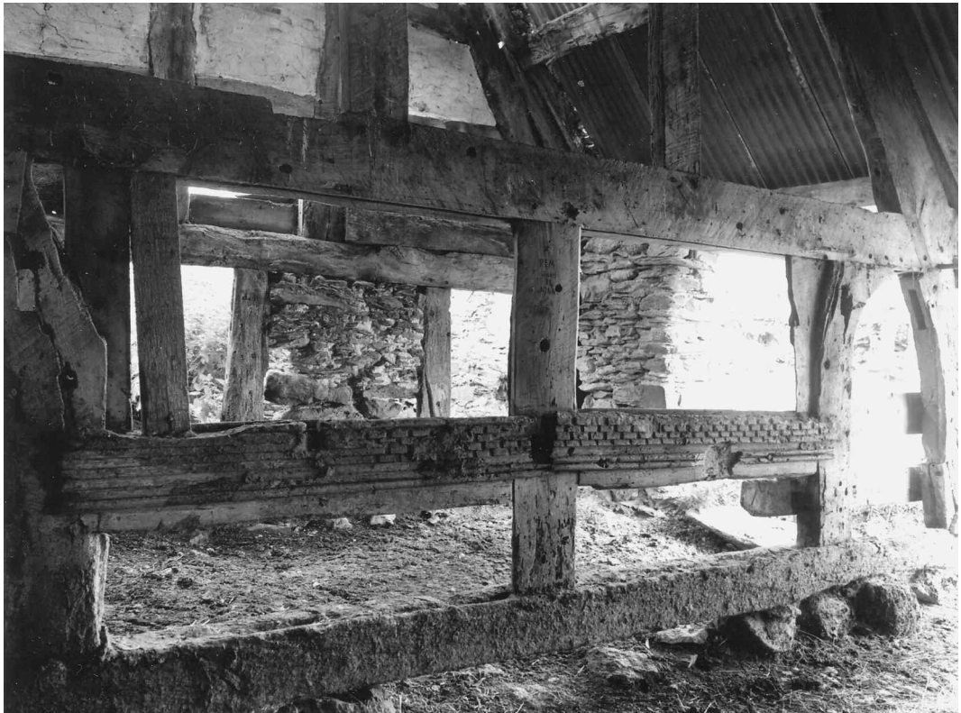
Fig. 8. Dais-end truss, looking north. The lower central portion of the south face of Truss D, photographed in 1952, showing the crenellated boards applied to the middle rail. © Crown Copyright: RCAHMW.
