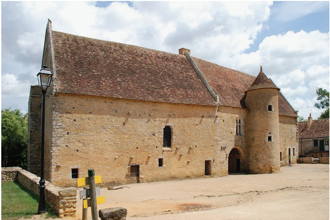
Fig. 15. Asnières-sur-Vègre (Sarthe). The southern façade of the great gatehouse, overlooking the courtyard. The row of corbels originally supported a gallery. Photograph: J. Mastrolorenzo.
