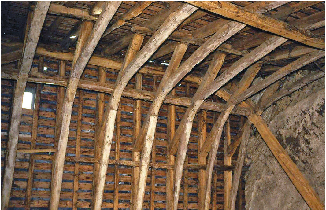
Fig. 35. Le Fretay, Pancé, Ille-et-Vilaine. The roof timbers of this chamber block have been dated by dendrochronology to 1440–42. Photograph: Archives départementales d'Ille-et-Vilaine: fonds Meirion-Jones.
