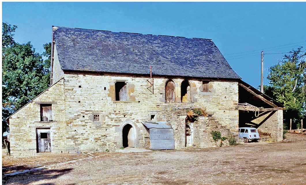
Fig. 34. Le Fretay, Pancé, Ille-et-Vilaine. A double chamber block at first-floor level approached by an external stairway over a ground-floor space destined either for stabling or for storage. Photograph: Archives départementales d'Ille-et-Vilaine: fonds Meirion-Jones.
