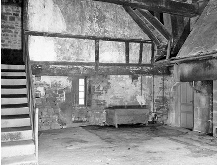
Fig. 11. Manoir de Lerre, Champcervon (Manche). A lateral gallery in the hall provides access to the chambers. Photograph: David Nicolas-Méry.
