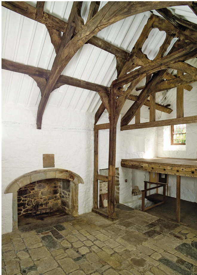
Fig. 23. Penarth Fawr, Llanarmon, Gwynedd. An important medieval hall with lateral fireplace. The spere truss is rare in Wales outside the north-east; it is an essentially English feature. © Crown Copyright: Royal Commission on the Ancient and Historical Monuments of Wales.
