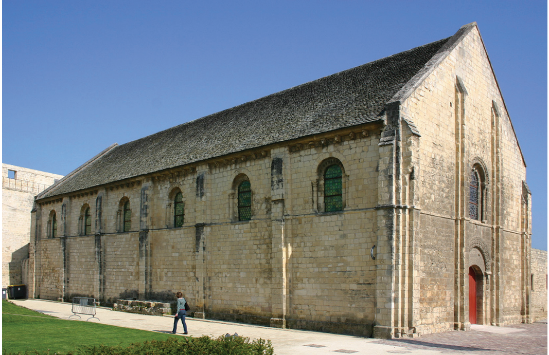
Fig. 13. Caen: L'Échiquier seen from the east, dominating the site of the palace of William the Conqueror. The ensemble, with the exception of the upper part of the three bays visible on the right is almost entirely original, though there are traces of subsequent modification during the Middle Ages, in particular the remains of a chimney inserted to serve a building attached to l'Échiquier during the fourteenth century. The 1960s building, visible on the left, masks a vaulted structure added in the twelfth century. Photograph: Edward Impey.
