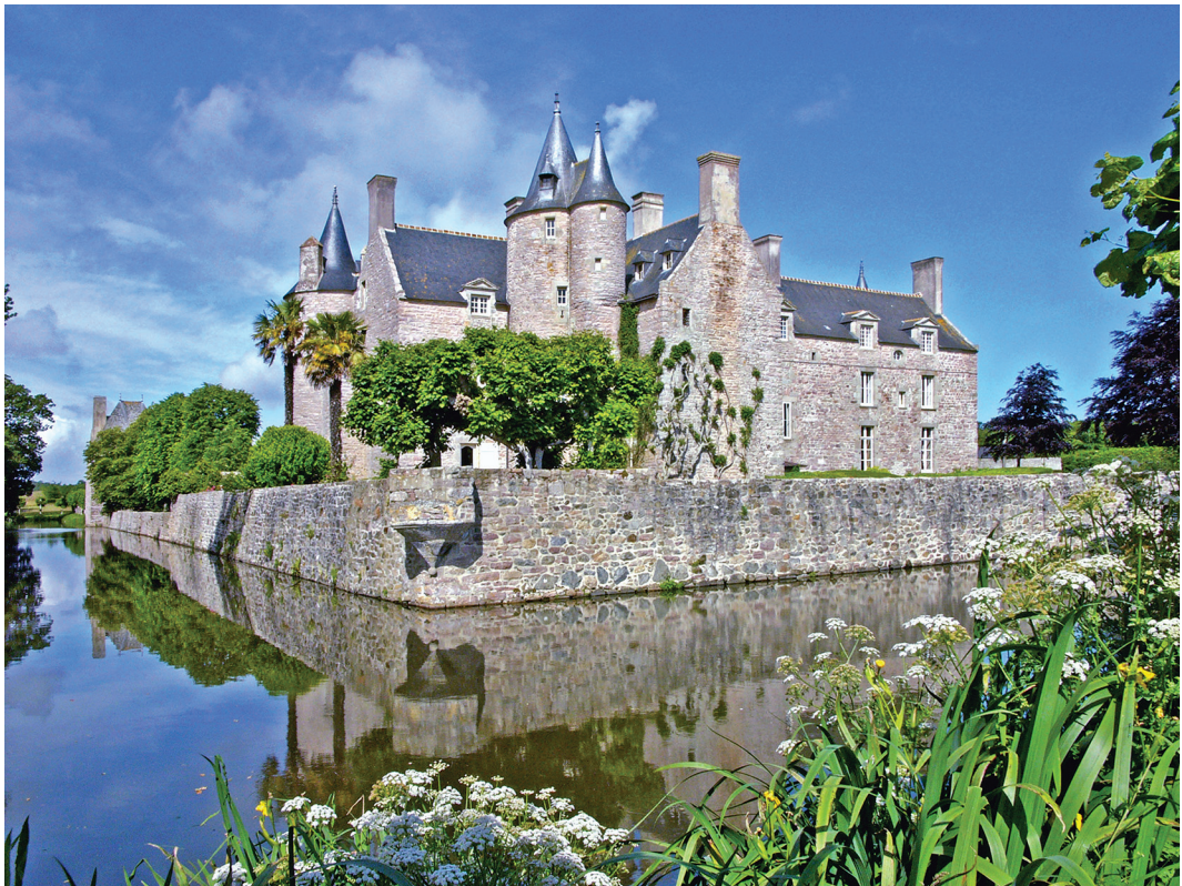
Fig. 33. Bienassis, Erquy, Côtes-d'Armor. An earlier manorial complex on this site was of timber construction, being replaced by this stone-built house between 1412 and 1434. Photograph: Gwyn Meirion-Jones.
