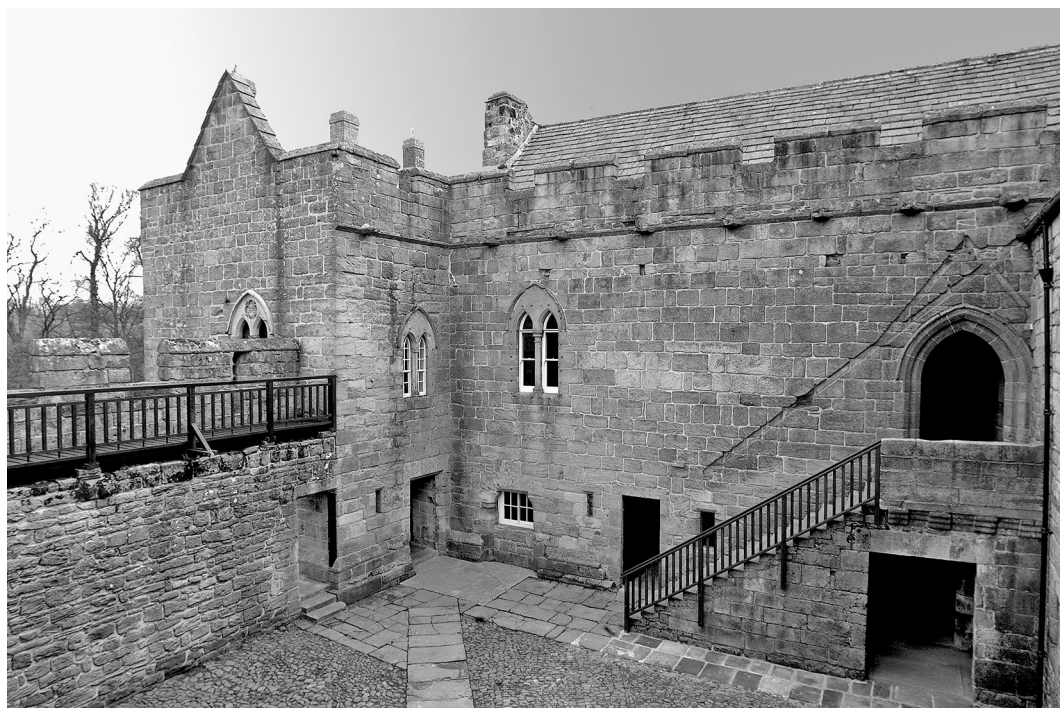
Fig. 2. Aydon Hall, Northumberland. On the left is a two-storey chamber block, the crenulation of which is probably original ( circa 1290). To the right the first-floor hall, circa 1300, replaces a timber ground-floor hall, with nave and aisles, of thirteenth-century date. The crenulations was added after 1305. Photograph: Philip Dixon.
