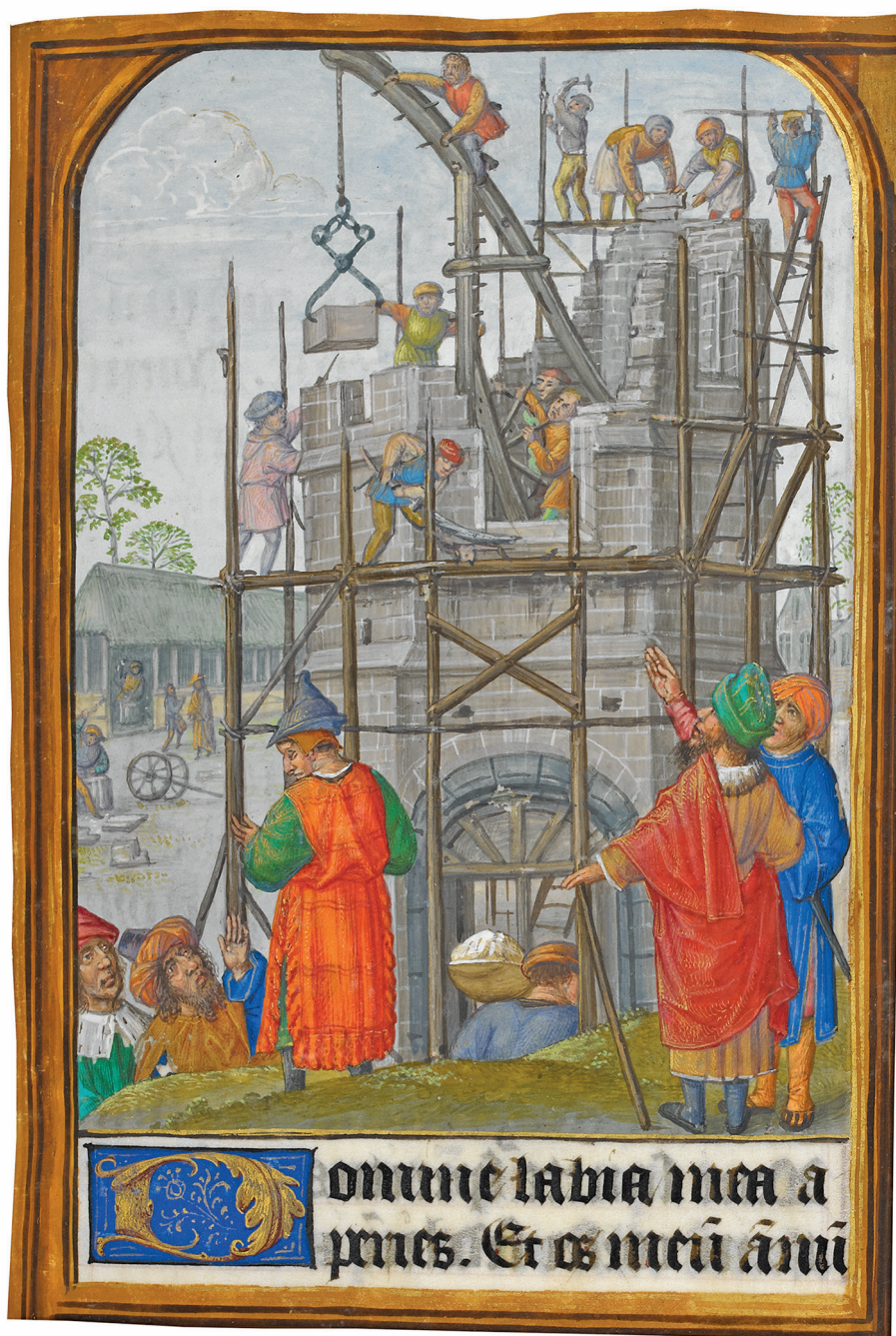
Fig. 3. Building a tower about 1500. The master mason and his patron are standing bottom right, and the labourers are carrying mortar, erecting scaffolding and lifting stones with a crane. Walling masons are laying blocks on the tower and banker masons are dressing stones outside and in their lodge at the rear left. © British Library Board, (ADD MS 35313, fo. 34').
