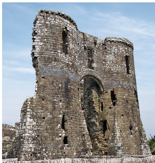
Fig. 6. Top Gatehouse to Carmarthen Castle. © Crown copyright (2017) Welsh Government. Bottom Gatehouse of Llawhaden Castle, Pembrokeshire. Photograph: Rick Turner.
