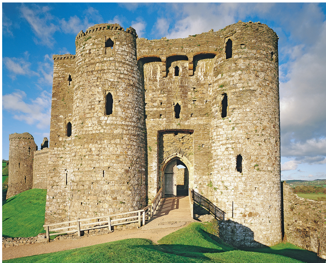
Fig. 4. Front elevation of the great gatehouse at Kidwelly Castle. © Crown copyright (2017) Welsh Government.
