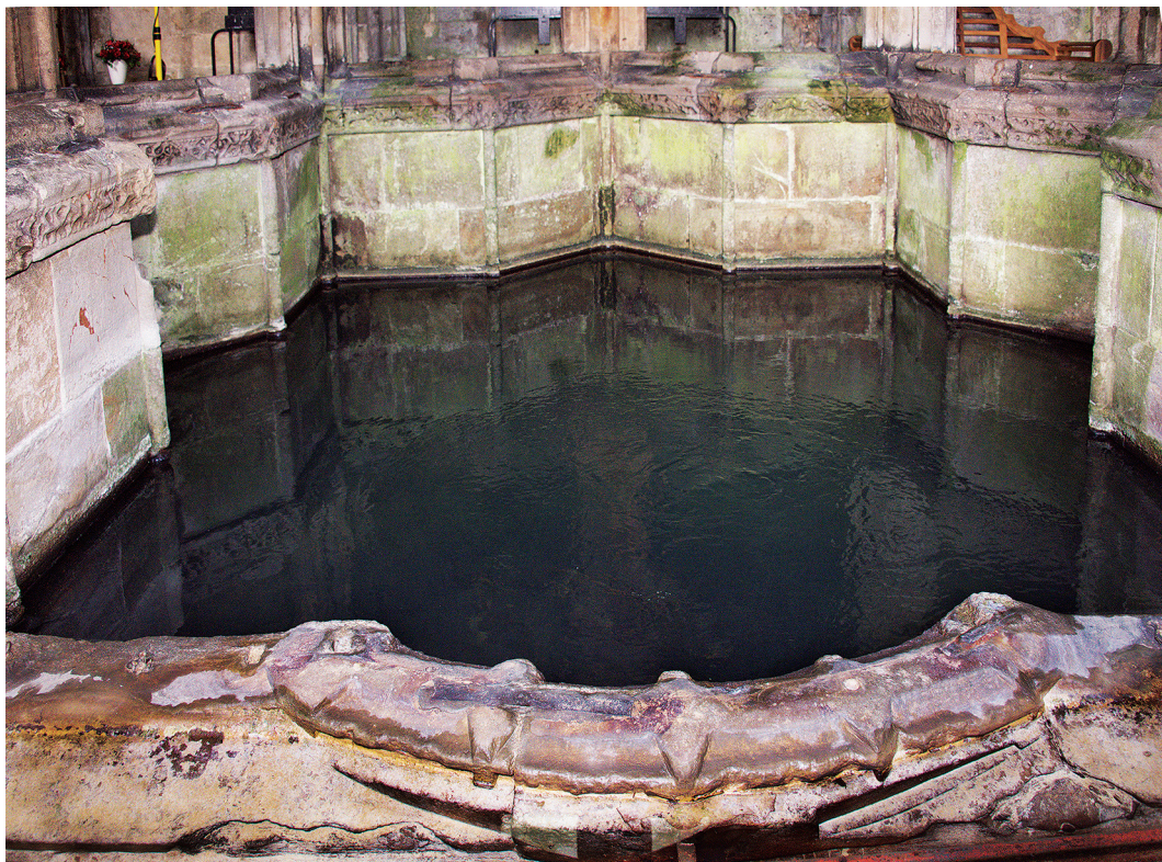
Fig. 13. The star-shaped well basin and base of the mullioned window in the Well Chapel. Photograph: Lee Wilkinson.
