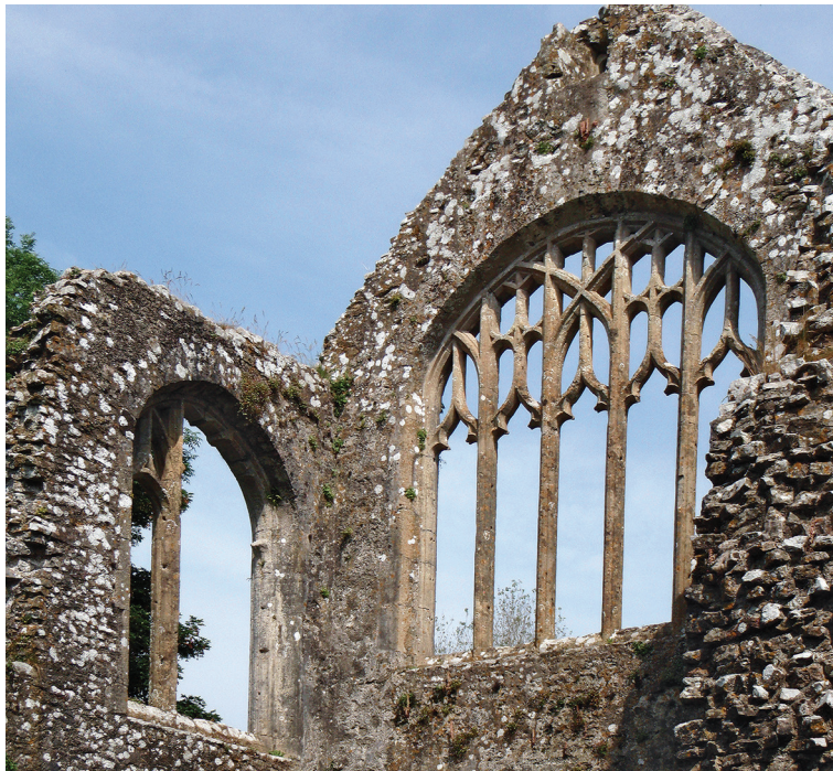
Fig. 21. The east window of Bishop Vaughan's chapel, Lamphey Bishops' Palace, Pembrokeshire. Photograph: Rick Turner.
