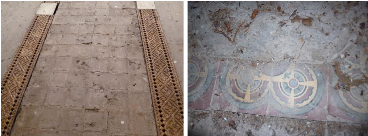
Fig.10: central aisle with heating grilles (left) and tiling around removed pulpit, in nave (right)
