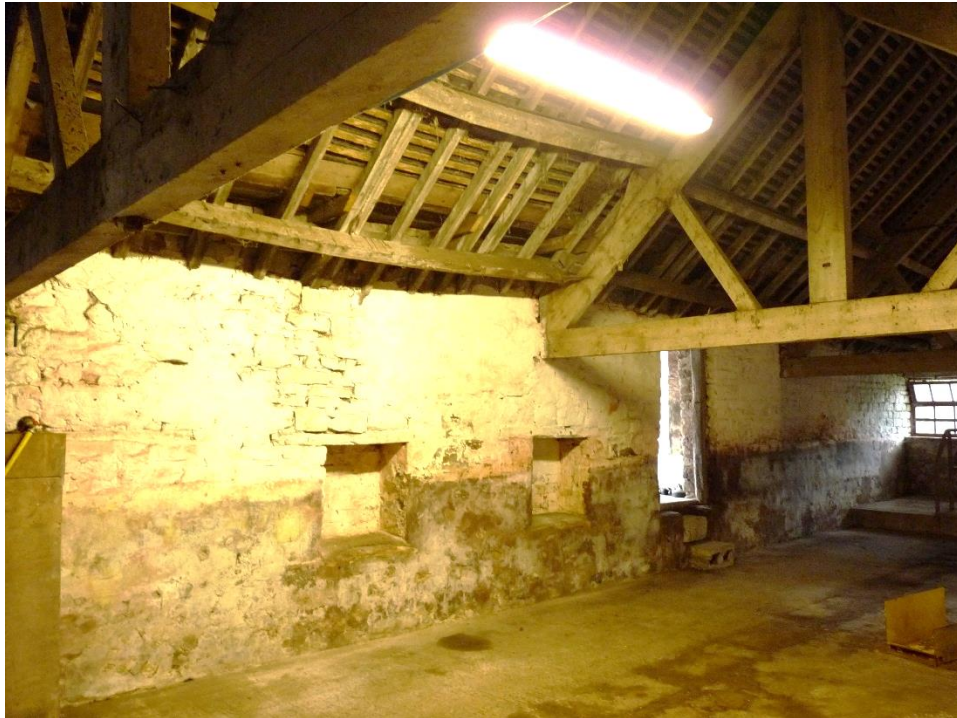
Fig.11: blocked feed-holes and doorway on the south wall of Building 2, from the south-east
