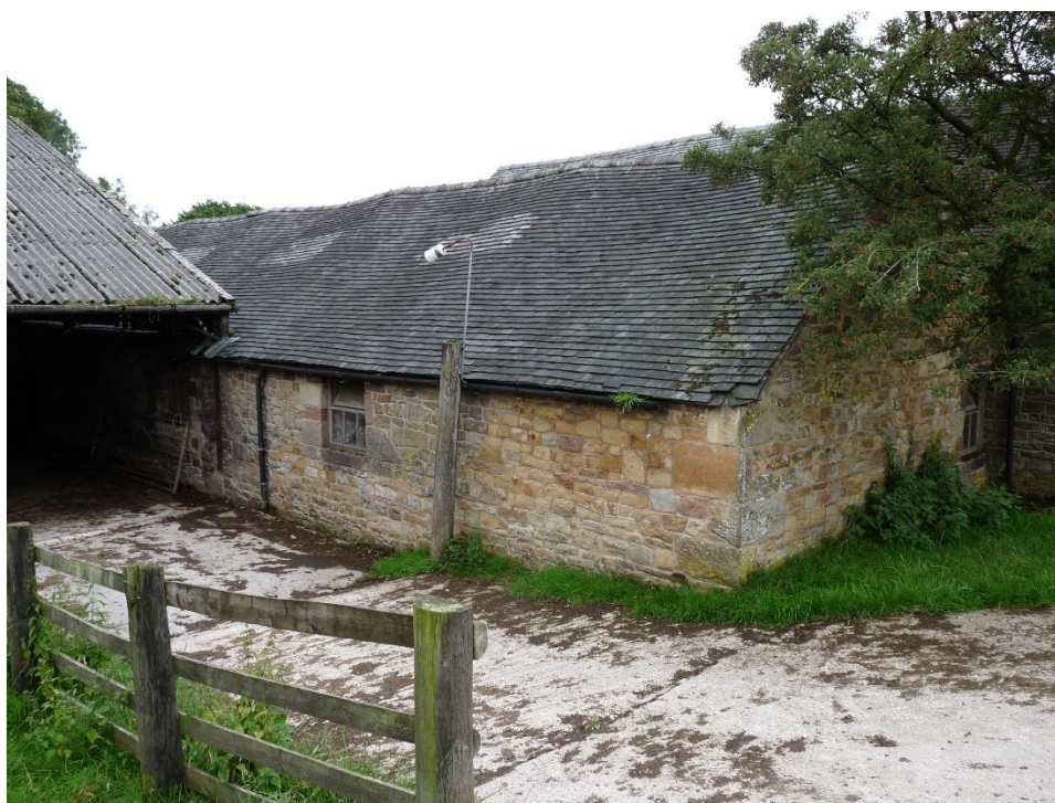
Fig.9: Building 2 from the north-west
