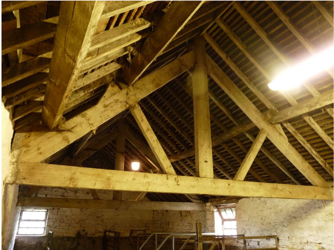
Plate 17: roof truss in Building 2 from the east
