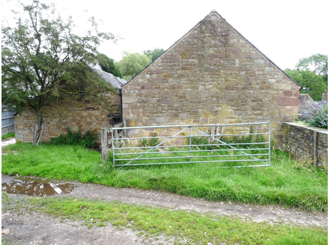
Plate 3: west gable-ends of the farm buildings, from the west
