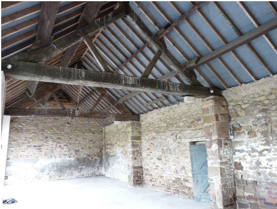
Fig.8: interior of Building 1 from the east
