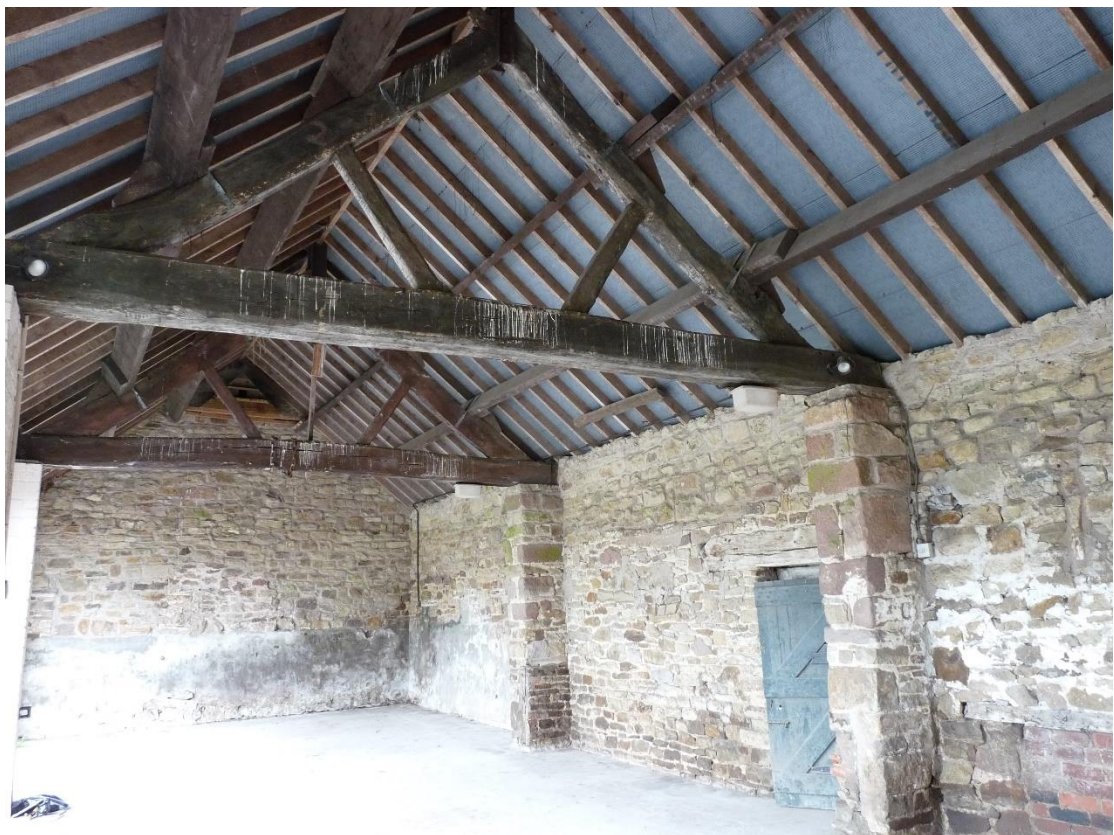
Plate 10: Interior of Building 1 from the east
