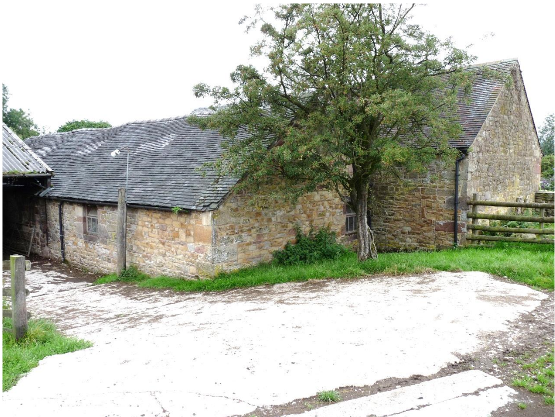
Plate 4: Building 2 (left) and the west end of Building 1 (right), from the north-west
