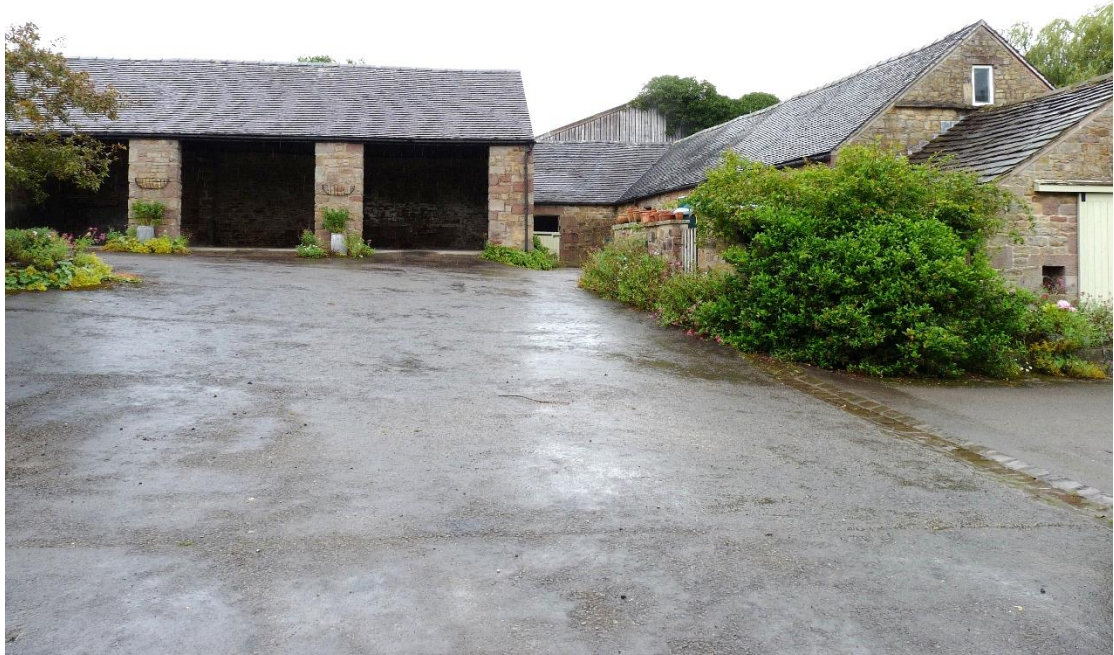
Fig.9: Building 1 and the east range of the farmstead from the south
