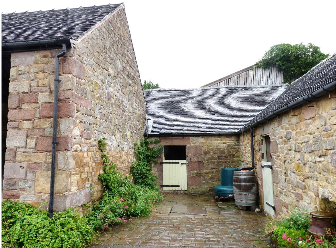
Plate 8: gable end of Building 1 and south elevation of Building 2 from the south-east
