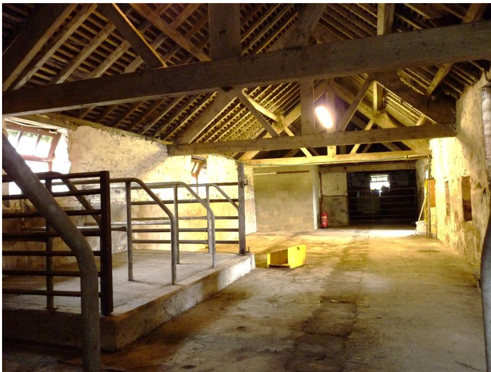
Fig.10: interior of Building 2 from the west
