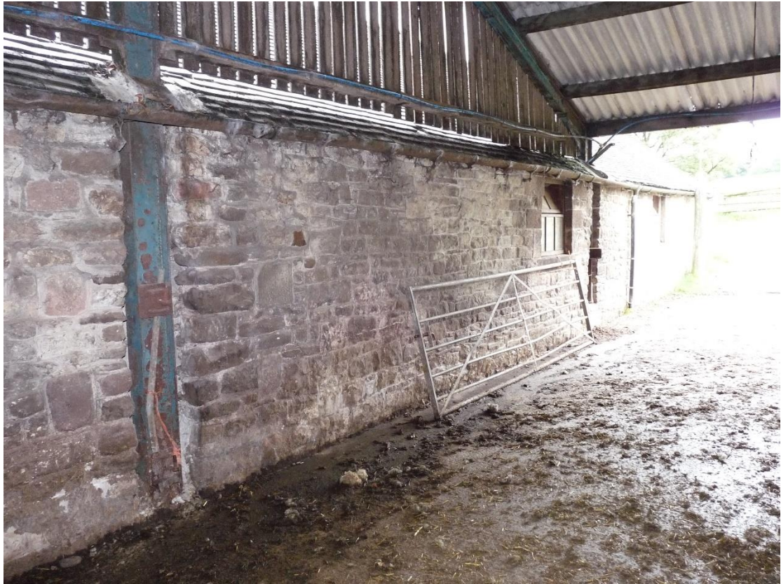
Plate 7: Building 2 from within the portal frame shed, from the north-east
