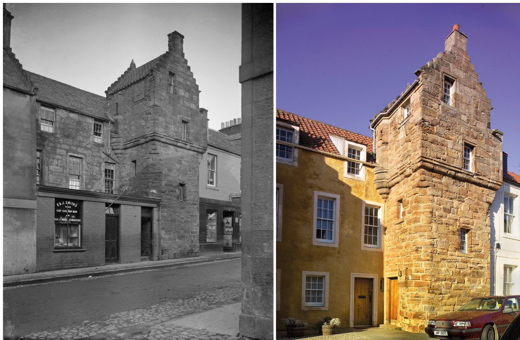
ILLUS 1 Kellie Lodging before and after restoration. (Canmore ID 34283 © Courtesy of HES)
