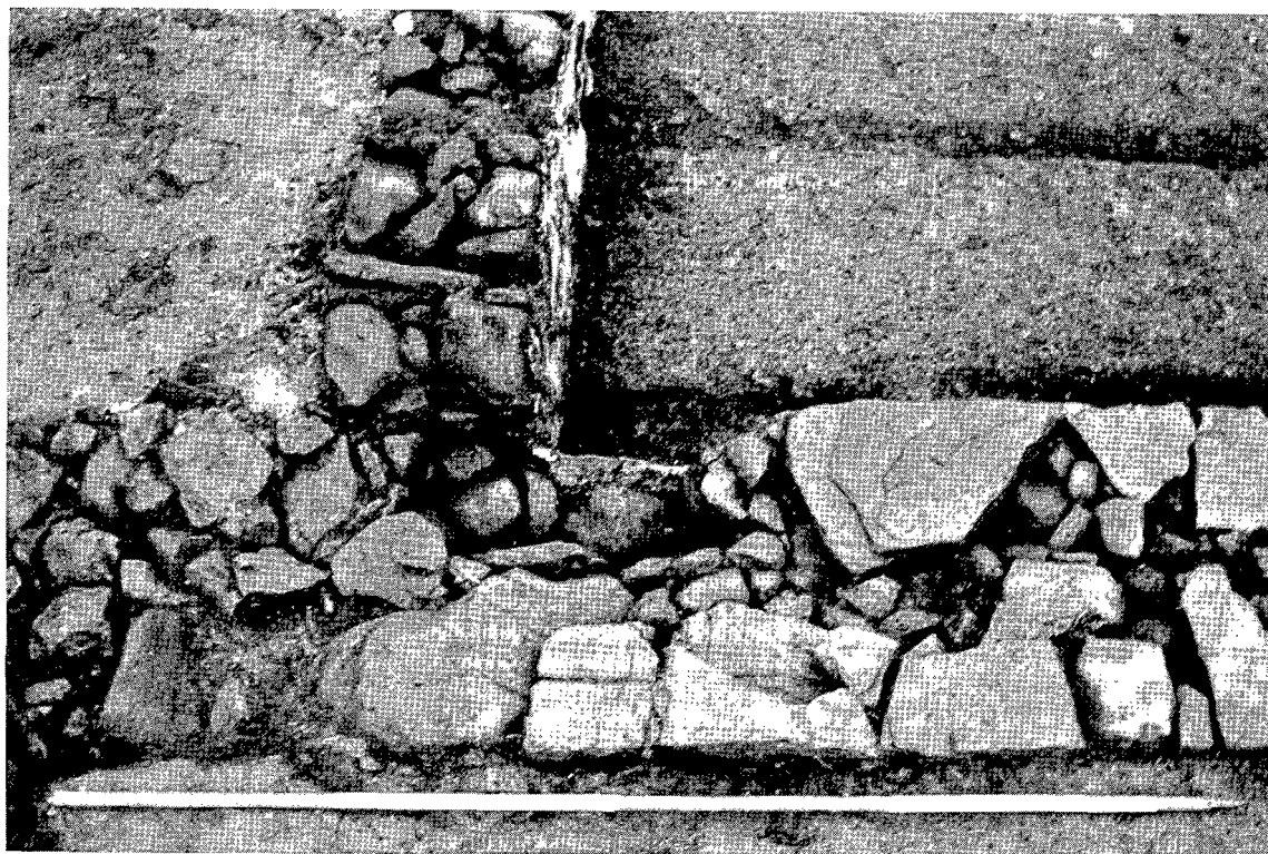
ILL 37 : Linlithgow. Detail of SE corner of chapter house constructed during Period 3, Phase 10. The S ends of two joist slots, mortar facing on the inner surfaces of the walls and a possible recess (6616) in the E wall are visible. Looking W
