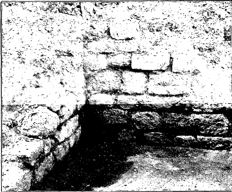
Fig. 17. Masonry of south-west corner of room No. 5.
