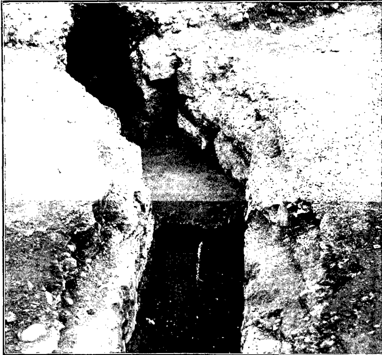
Fig. 14. View of the Flue passing from room No. 2 to room No. 3.
