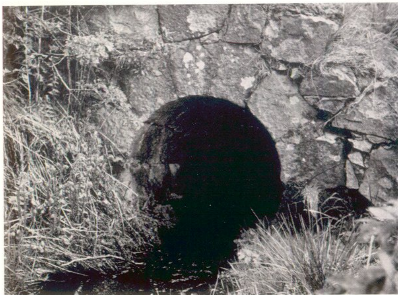
b St Fergus Canal, Inverquinzie branch: culvert on Cuttie Burn
