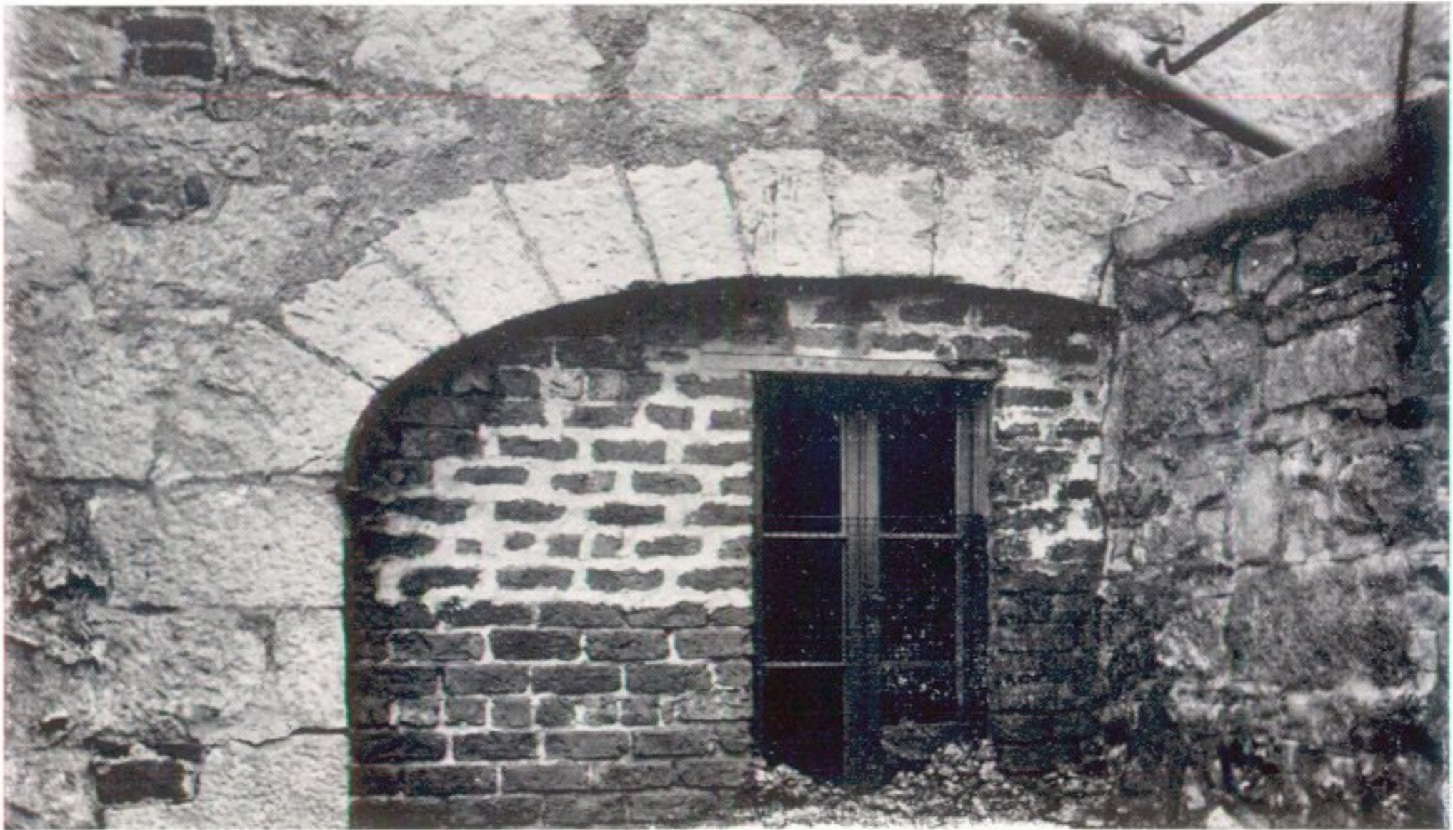
b Archway in former grain-store on Aberdeenshire Navigation Canal at Port Elphinstone
