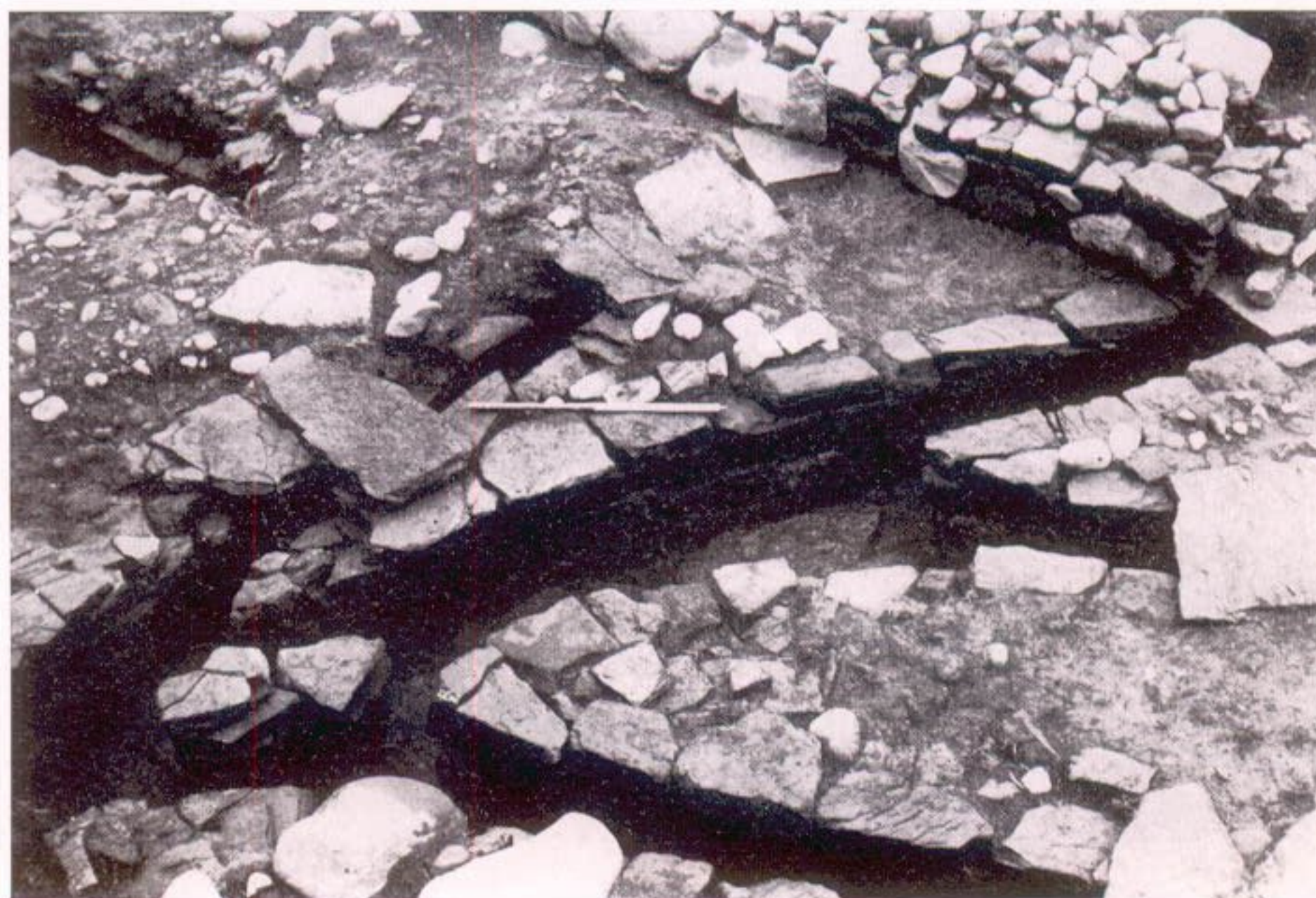
b Kemper Avenue: flues of E hypocaust system, from the SE, showing central plinth and unused duct (N4)
