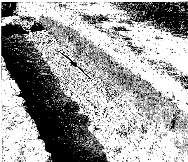
ILLUS 30 Road metalling of the via praetoria inside the east gate, from north-east (Trench A2)
