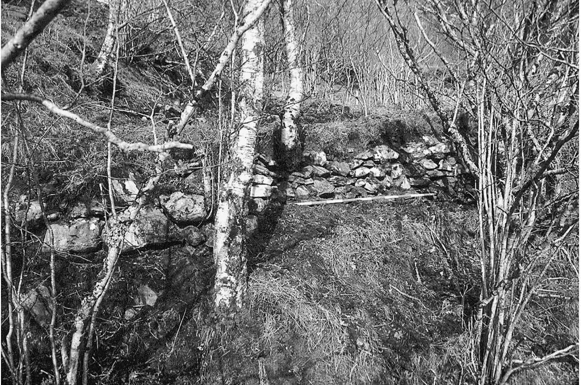
ILLUS 4 Retaining wall (g), from the south (scale rod divisions at 0.2 m intervals)
