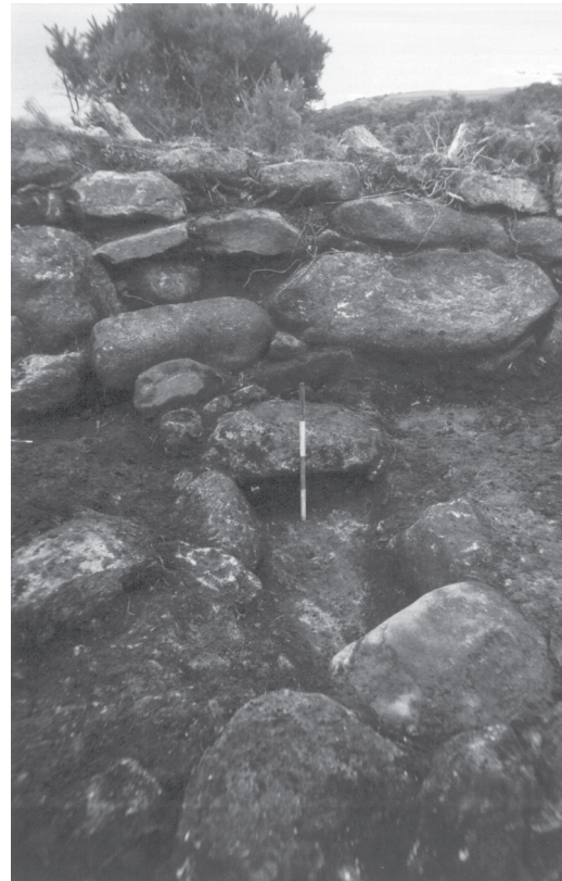
ILLUS 7 View of lintel over internal drain [123] as it exits the roundhouse under wall [106]
