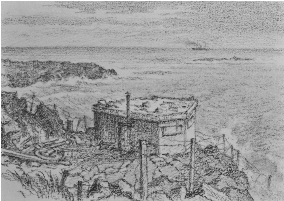
ILLUS 15 Blockhouse No. 5 (according to the 1918 numbering) at the south-east corner of Inchkeith, as sketched by 2nd Lt A Ross during the war. Note the stove pipe (courtesy of Mrs Fiona Buchanan)
