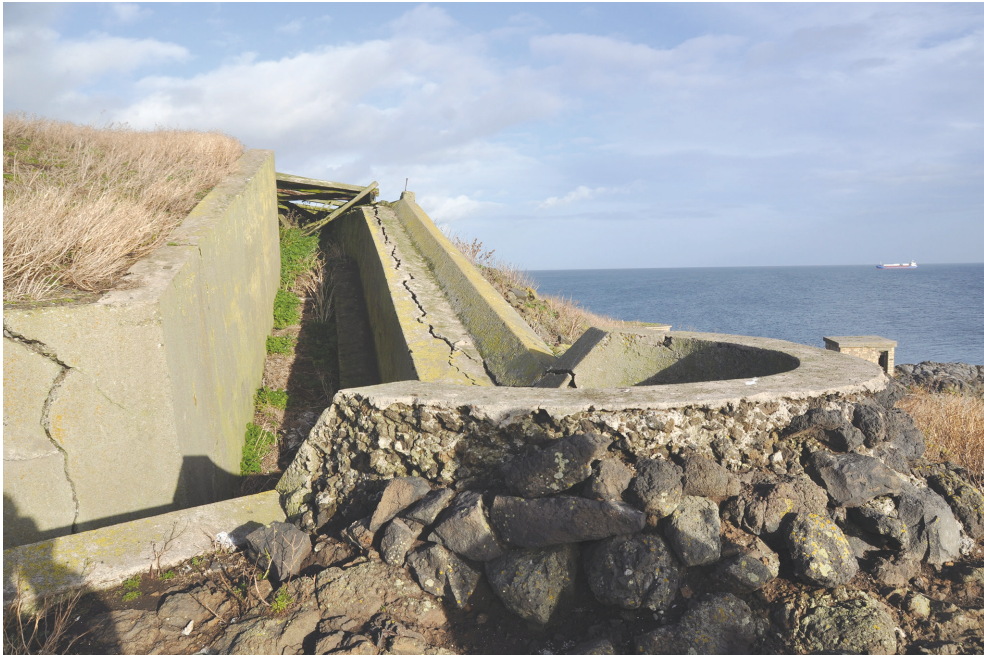
ILLUS 13 The concrete-lined, timber-roofed firing trench built across the south front of the South Fort on Inchkeith by the time of the 1911 map (Authors)
