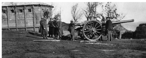
ILLUS 6 Photograph by Major F R Burnet, of the Spiershill Fort, showing the blockhouse and one of the two 4.5-inch guns on field mountings. The 4.5-inch gun was the same as used, on a different mounting, in coast batteries (Inverclyde Museums)
