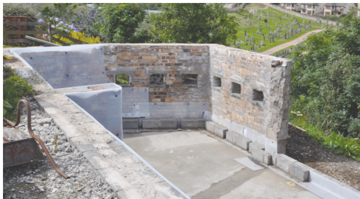
ILLUS 10 The surviving blockhouse at Kinghorn/Pettycur, partially demolished and being incorporated into a modern building, 2016 (Authors)
