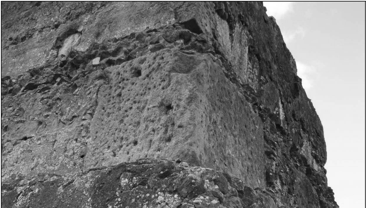
Plate 4: piece of re-used masonry built into engine platform - note the hole on the left hand face of the stone near the top; this may be for a fitting of some form or could be an indentation left by the brace used to lift and transport the block (112)
