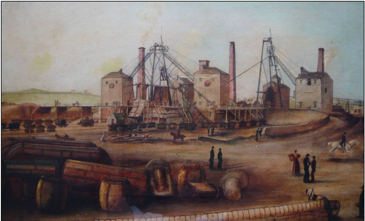
Plate 1: a painting of Crowtrees colliery by the artist J. Wood (c. 1840) held in the Beamish Museum collection. This painting clearly illustrates the high standard of the mine buildings, stone from which may have been used in the construction of the Phase III winding-engine house.
