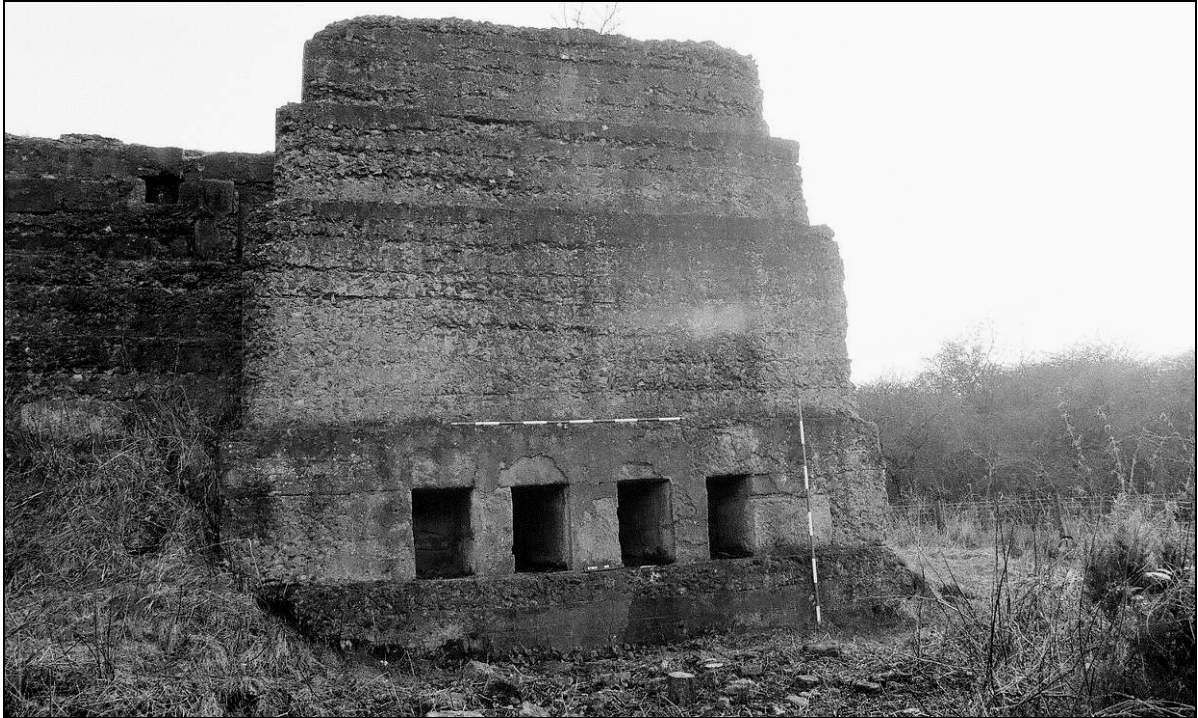
Plate 9: North facing elevation (130) of winding-engine base showing bolt access apertures (131) in the cement stack (160)
