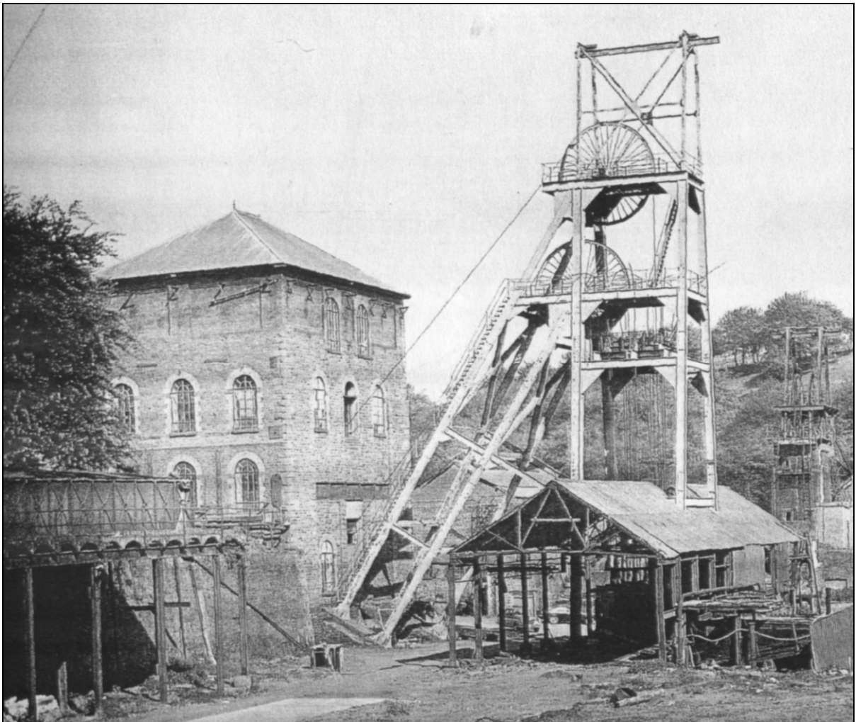
Plate 13: 19th century winding-engine house and headframe at Tirpentwys in Wales. The engine here was a vertical winder, so the building is taller than Crowtrees would have been but it does show the relationship of the various elements of the pit head.
