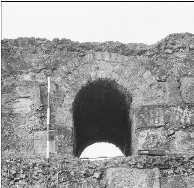
Plates 6 & 7: brick headed arch (111). The second photographs shows the detail of the slot on the arch soffit which links with the bolt holes at the top of the engine platform
