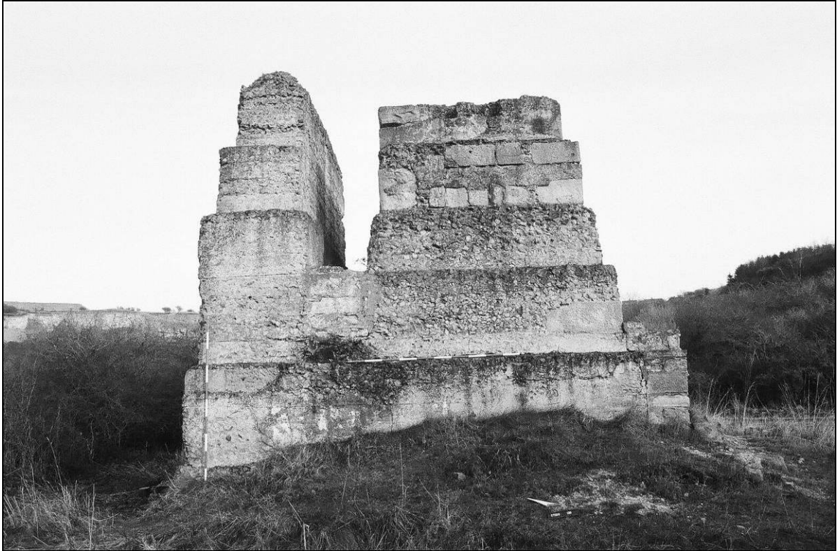
Plate 8: West facing elevation of winding-engine base showing engine platform (150) to the right, crank arm slot (170) and stack (160) to right.
