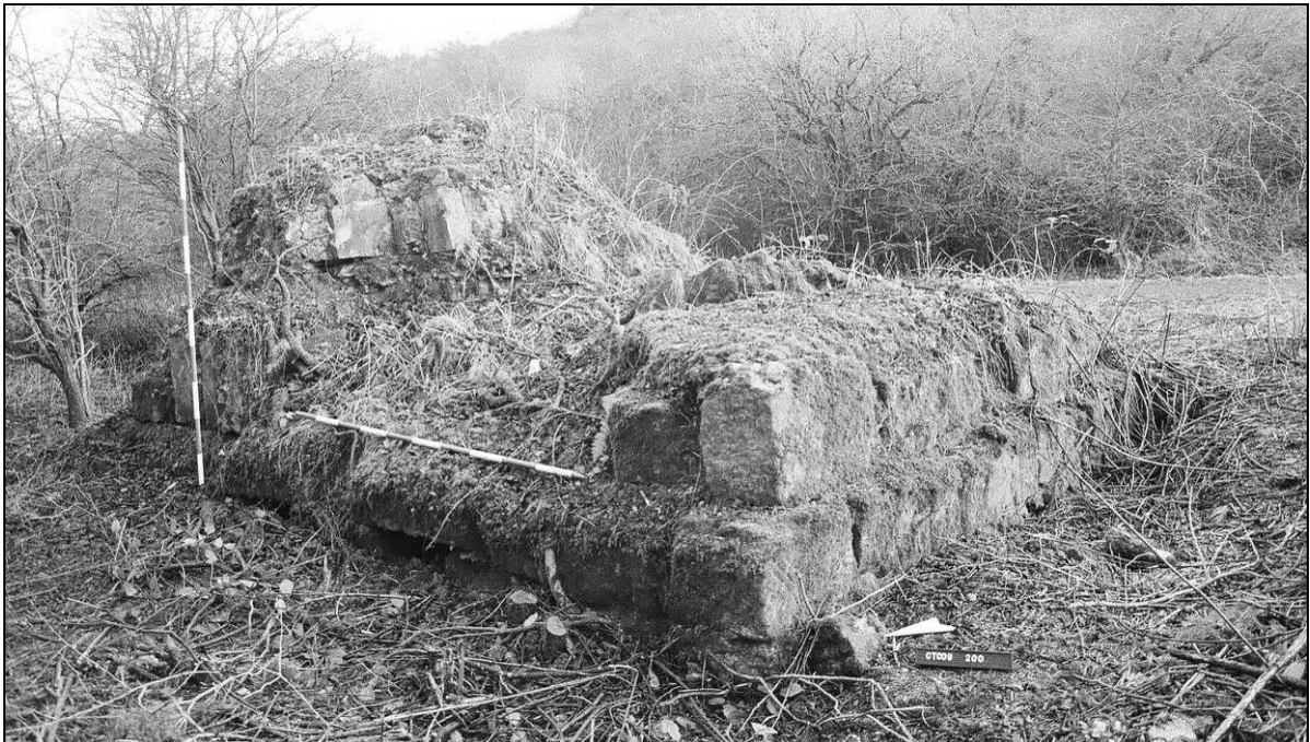
Plate 12: East platform (200) showing north face (110) with bolt access apertures (211) just visible
