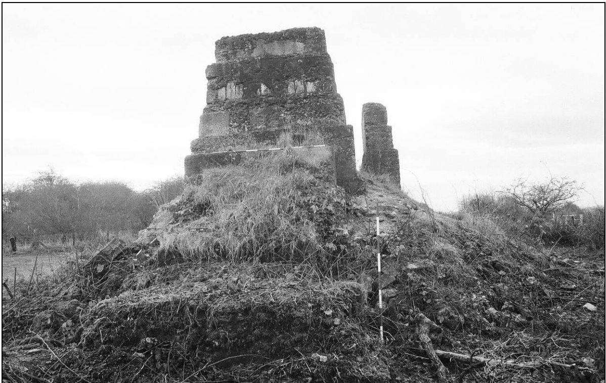
Plate 11: East facing elevation (140) of winding-engine base showing structure (180), probably the base support of the headframe
