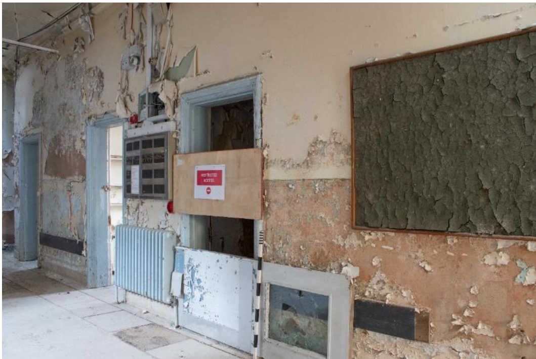
Photo 148: west side of north block corridor, facing west (1796_148.TIF)
