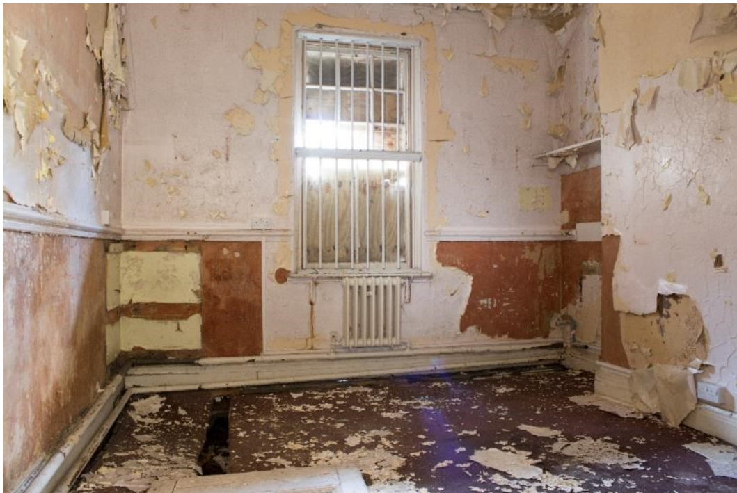
Photo 138: Room 3, facing north (1796_138.TIF)
