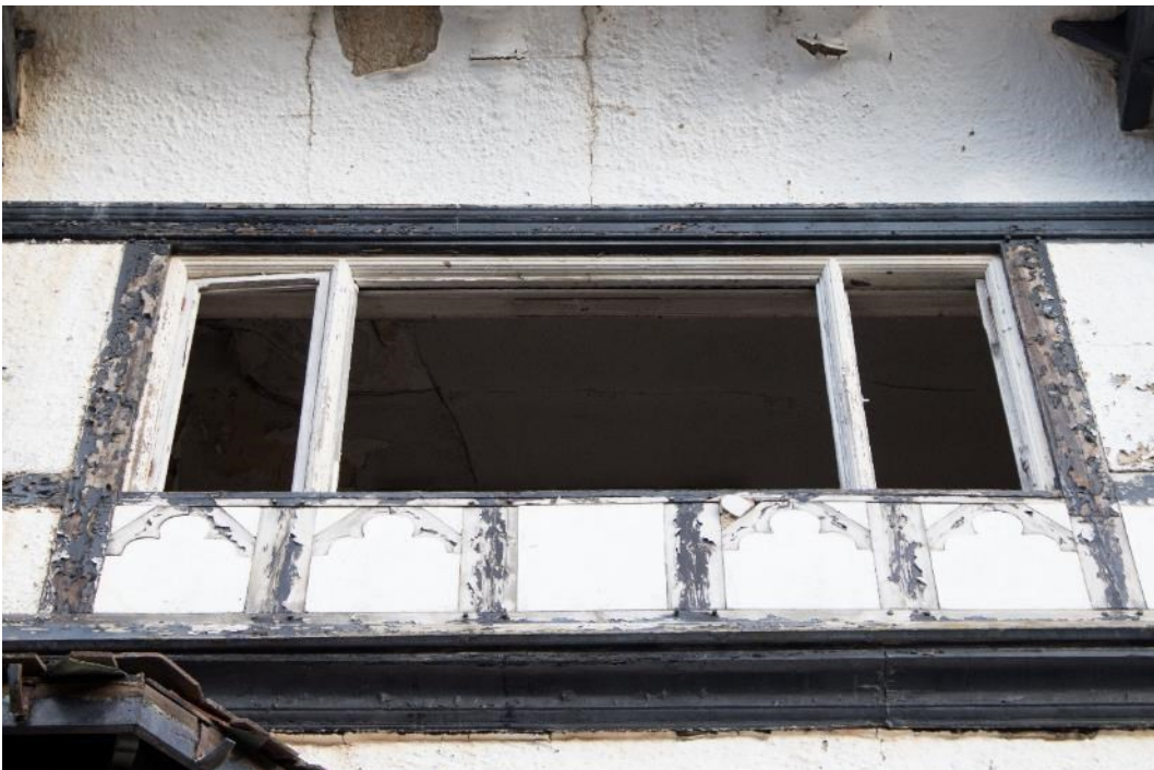
Photo 32: Window to second floor, facing north-east (1796_032.TIF)
