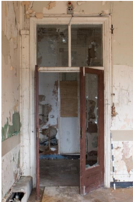
Photo 252: Door to west dayroo, facing north-east (1796_252.TIF)
