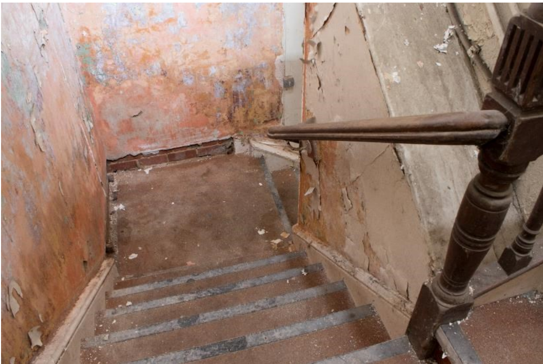
Photo 316: Stairs from ground to first floor, facing south-west (1796_316.TIF)
