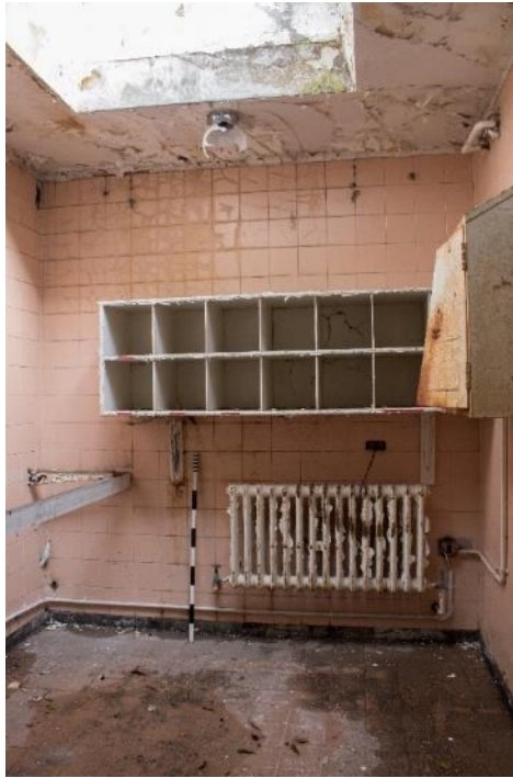
Photo 209: Room 35 facing east (1796_209.TIF)
