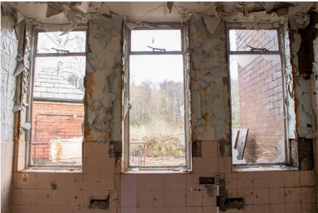
Photo 218: Windows to room 31, facing east (1796_218.TIF)
