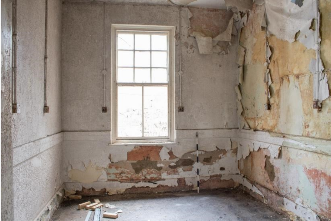
Photo 133: Room 6, facing north-east (1796_132.TIF)
