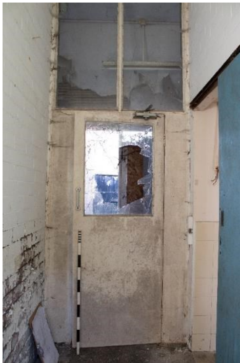
Photo 174: Entrance passage to service range, facing north-east (1796_173.TIF)
