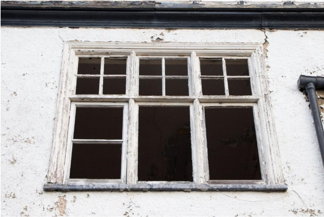
Photo 23: Window to first floor south-west room (45), facing north-east (1796_023.TIF)
