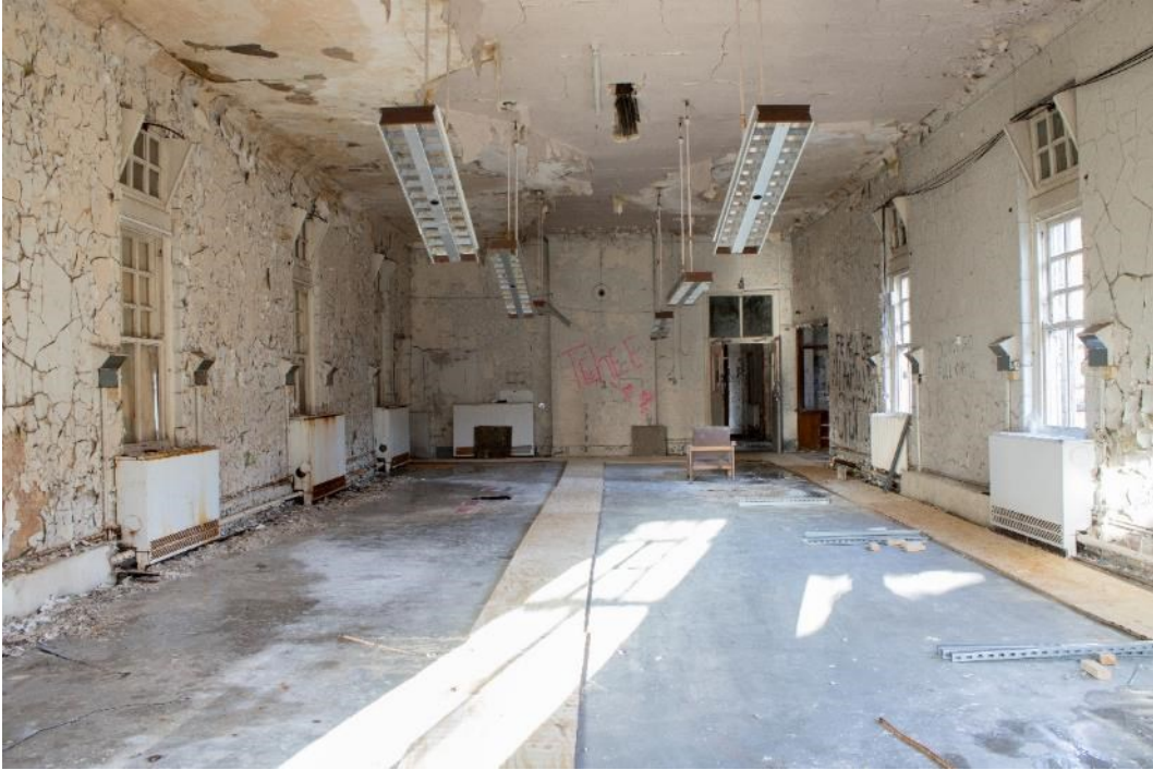
Photo 271: East ward, facing north (1796_271.TIF)
