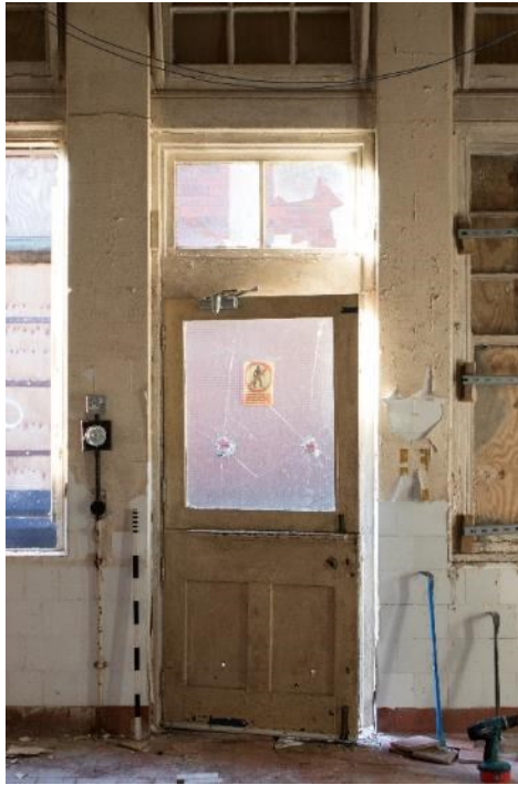
Photo 157: Kitchen doorway, facing south-west (1796_157.TIF)
