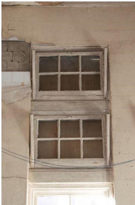
Photo 158: Kitchen top-lights, facing south-west (1796_158.TIF)
