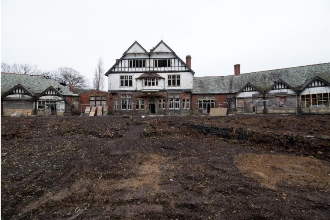
Photo 1: South elevation (1796_001.TIF)
