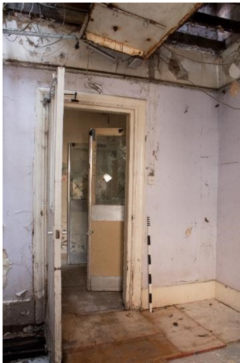
Photo 204: Room 12, facing south-west (1796_204.TIF)
