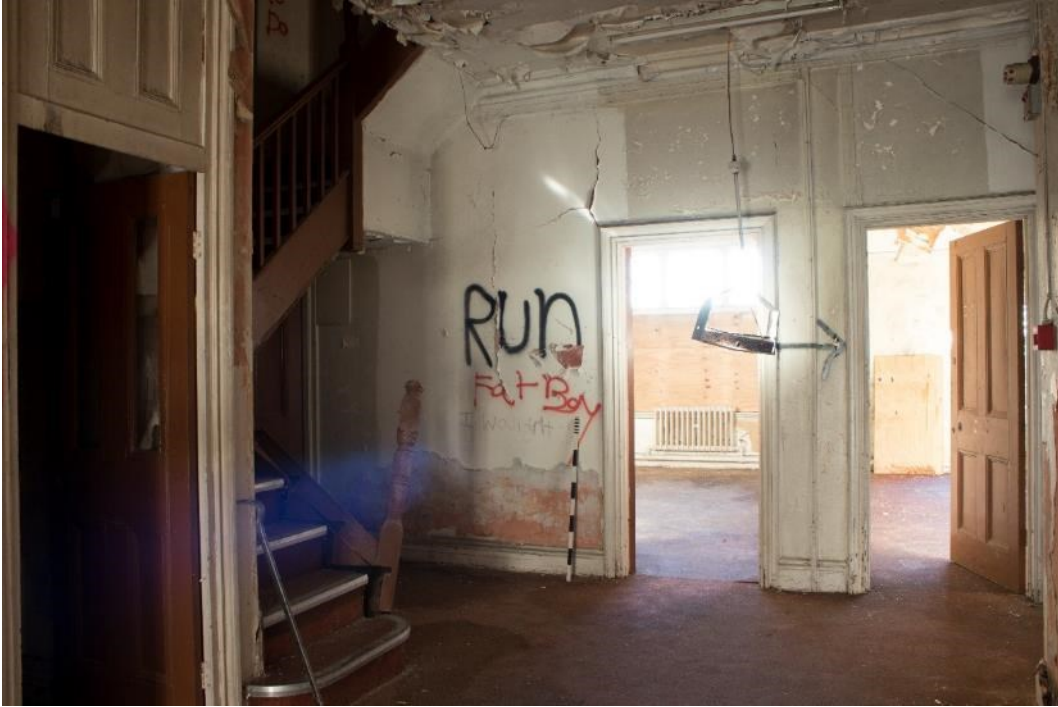
Photo 293: First floor hallway, facing south-west (1796_293.TIF)
