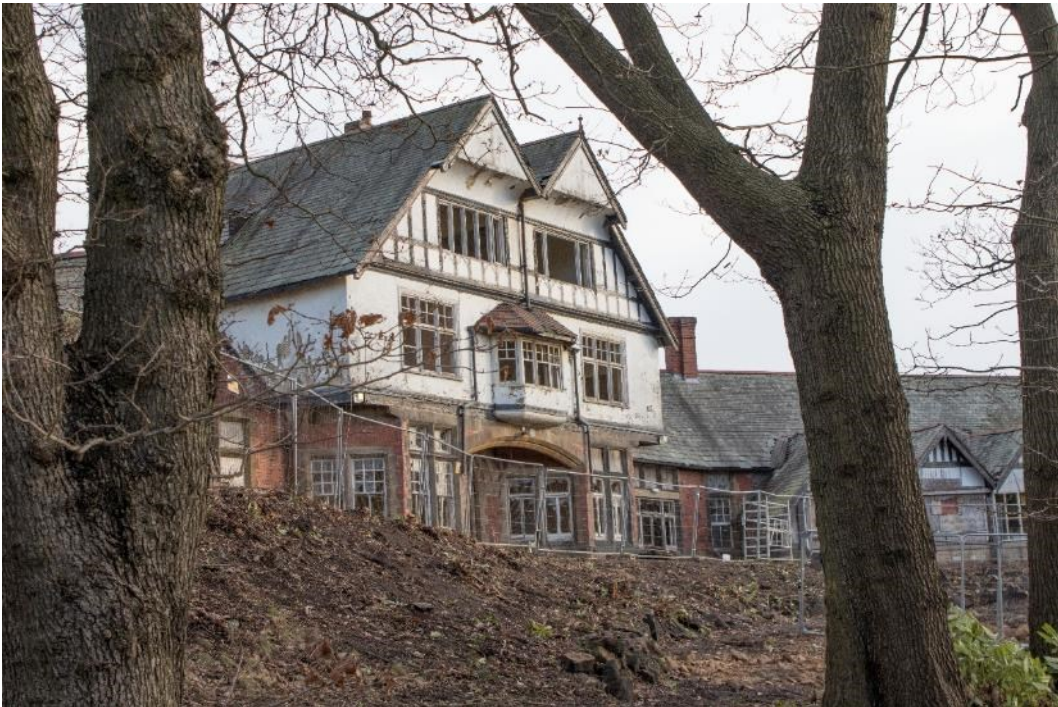
Photo 48: Distant view of central block, facing east (1796_048.TIF)
