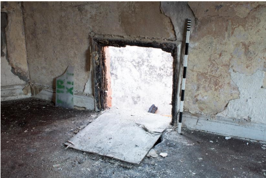
Photo 310: Roof access hatch in room 46, facing west (1796_310.TIF)
