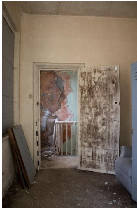
Photo 200: Room 54, facing south-west (1796_200.TIF)
