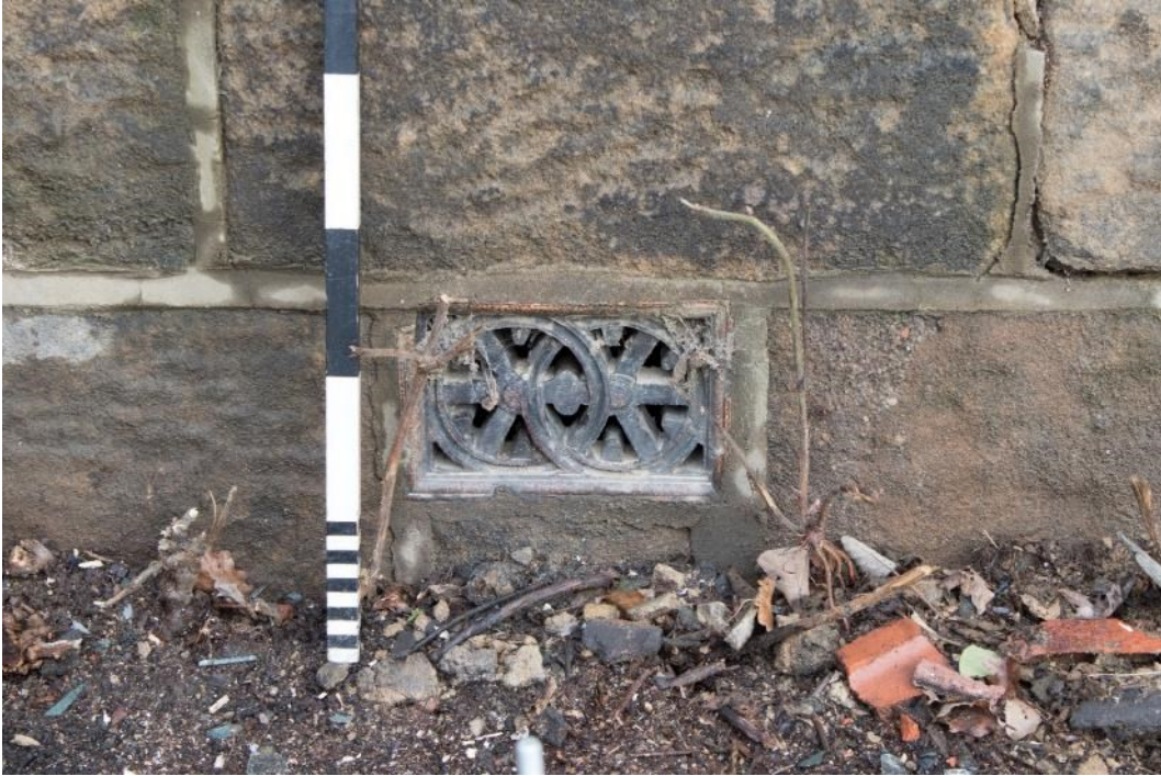
Photo 21: Detail of ventilation grill, facing north-east (1796_021.TIF)
