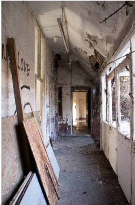
Photo 179: Service range corrdior/enclosed veranda, facing north-west (1796_179.TIF)
