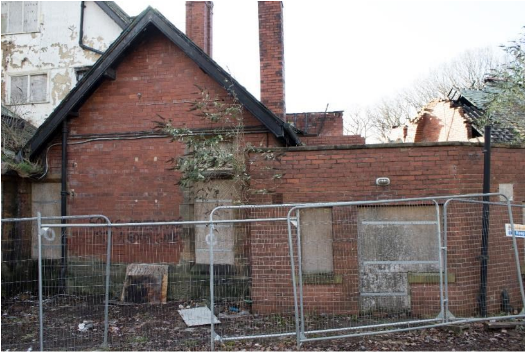
Photo 57: North elevation of west wing and wash block, facing south-west (1796_057.TIF)
