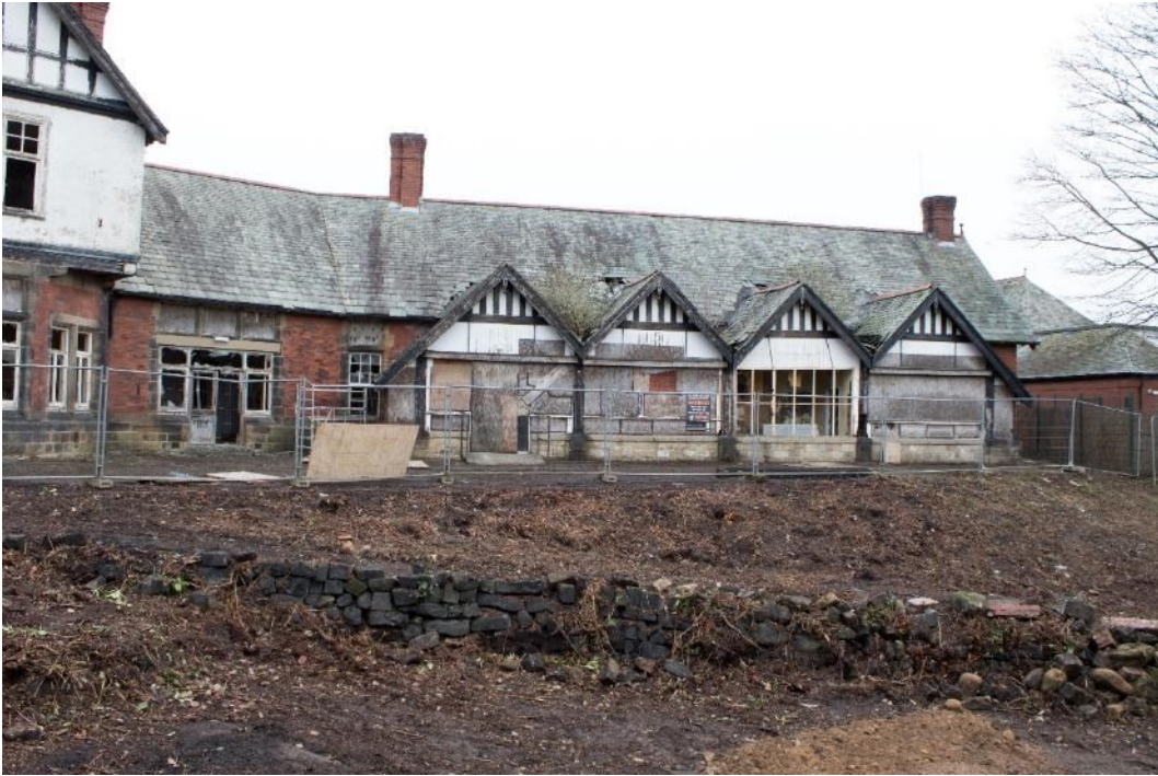
Photo 5: East wing, south elevation (1796_005.TIF)
