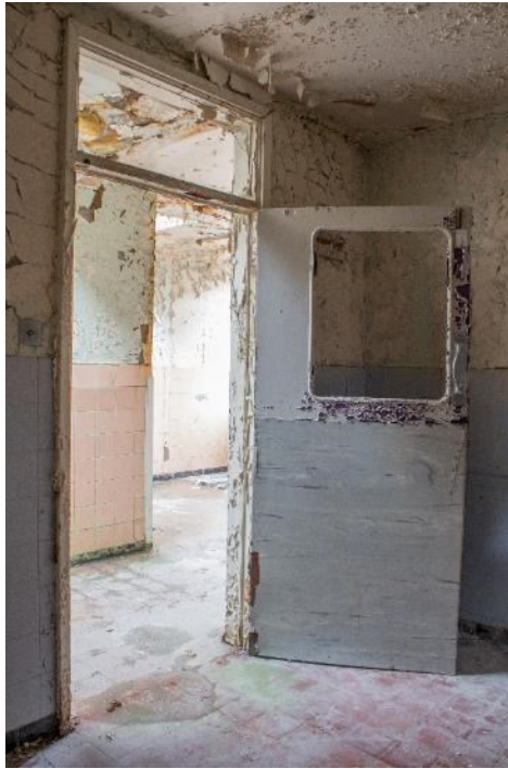
Photo 229: Door to room 28, facing north-east (1796_229.TIF)
