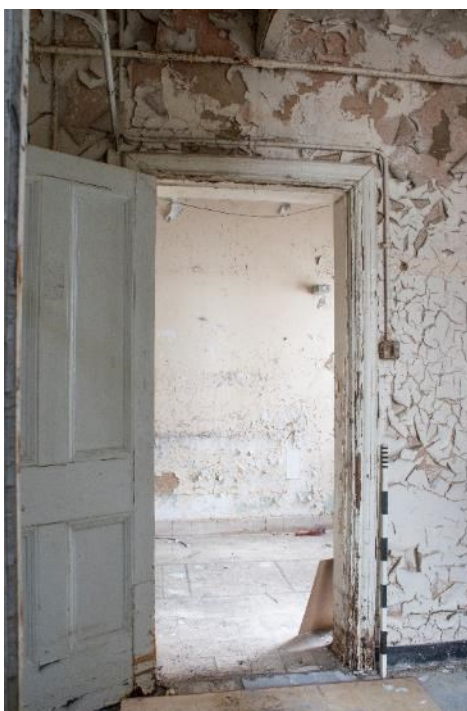
Photo 130: Room 11, facing south-west (1796_130.TIF)
