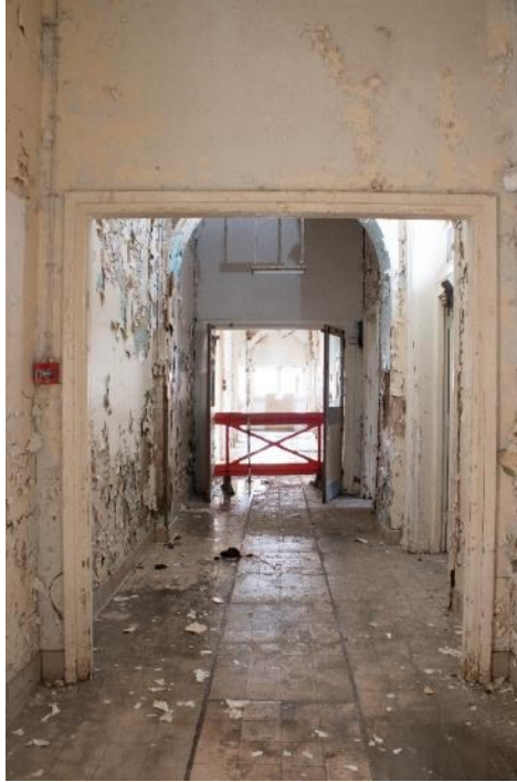
Photo 259: East-west corridor, facing north-west (1796_259.TIF)
