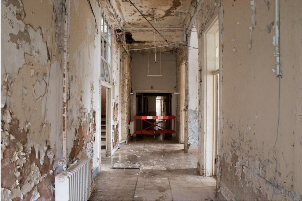
Photo 241: Main east-west corridor, facing south-east (1796_241.TIF)
