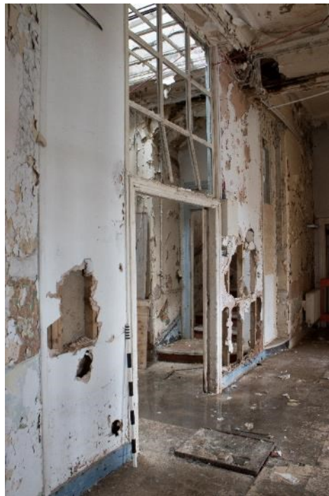
Photo 242: Inserted partition between north and central block corridors, facing east (1796_242.TIF)
