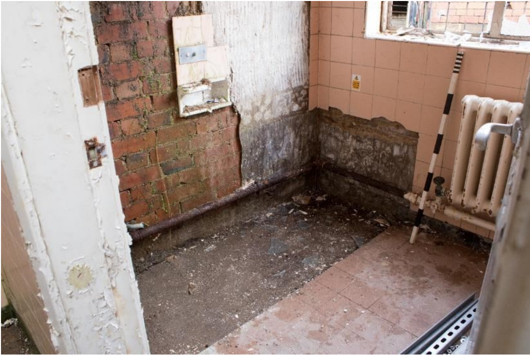
Photo 221: Location of bath, room 32, facing north-east (1796_221.TIF)
