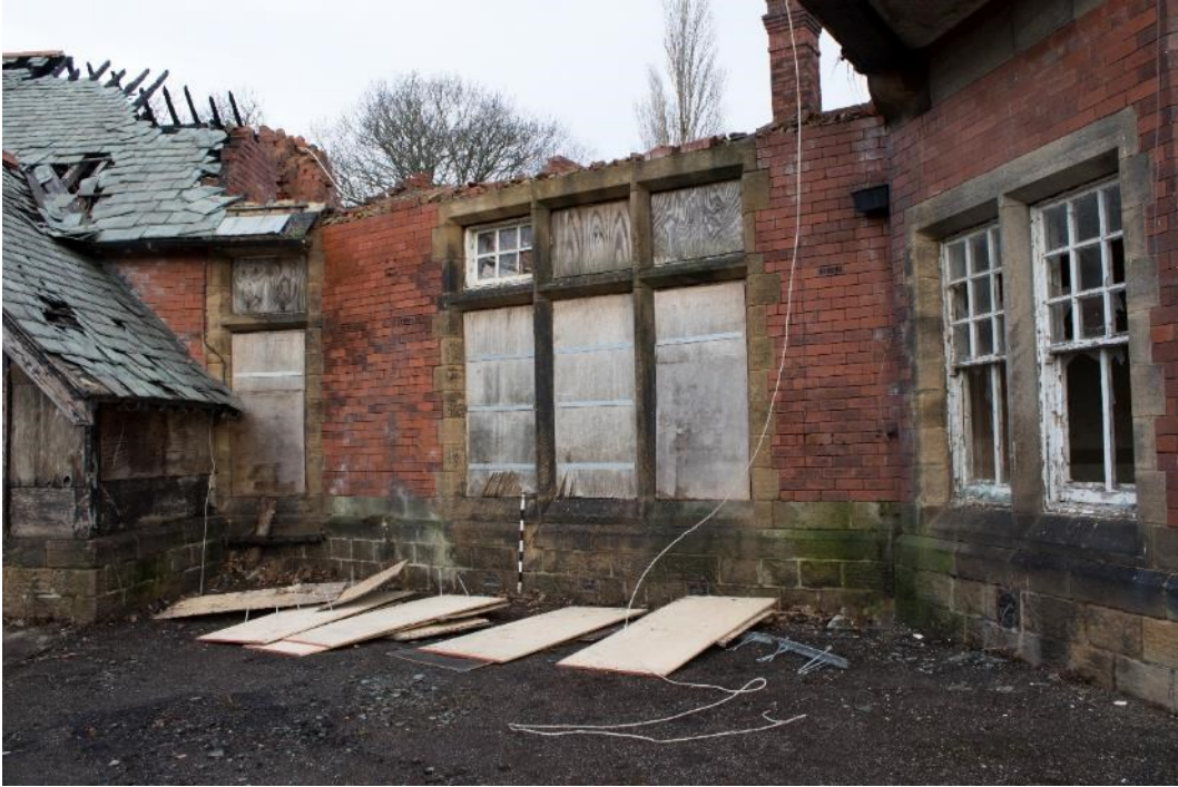
Photo 19: Exterior of room 55, central block, facing north (1796_019.TIF)
