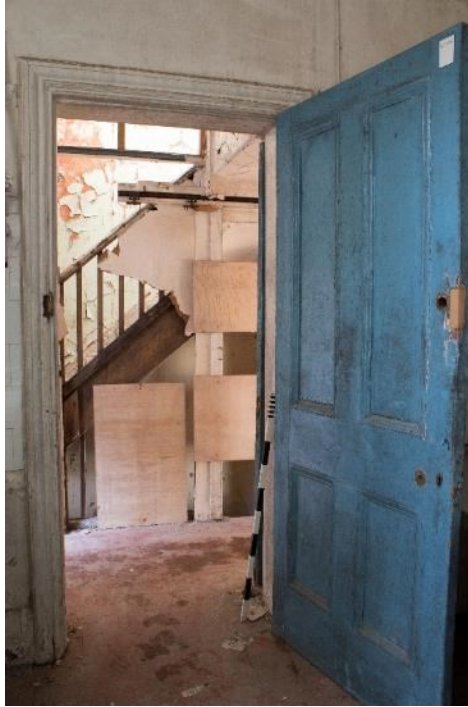
Photo 195: Door to room 20, facing south-east (1796_195.TIF)
