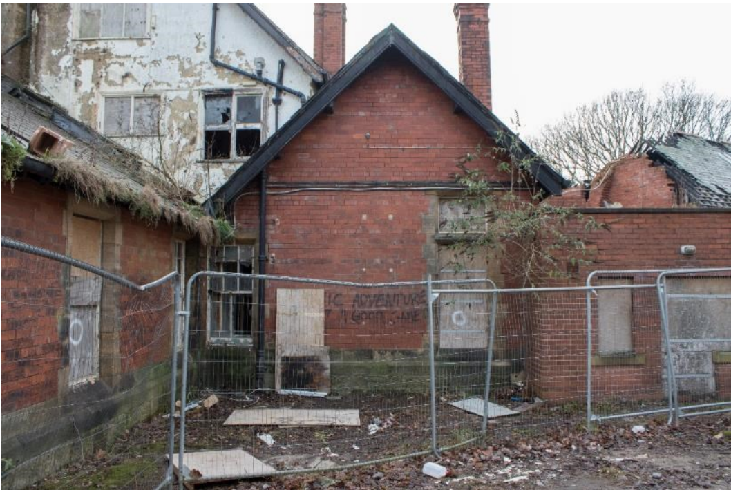
Photo 96: North elevation of central block (56) (1796_096.TIF)
