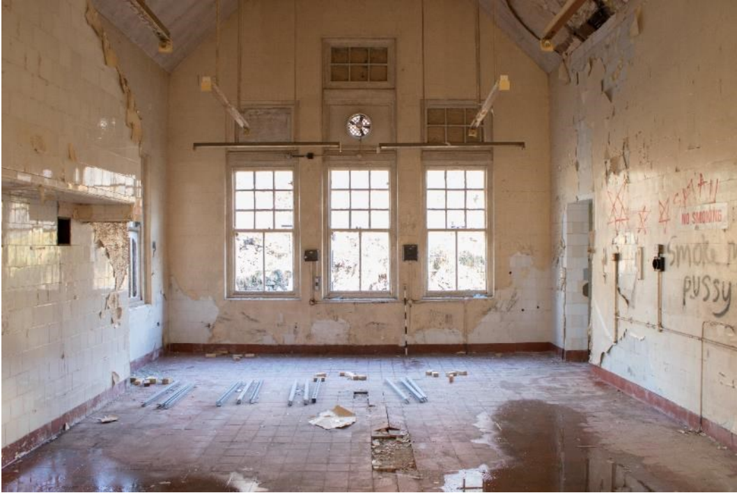
Photo 153: Kitchen, facing, north-east (1796_153.TIF)
