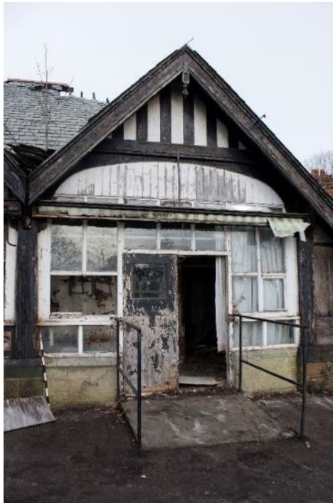
Photo 16: West veranda bay with doorway, facing north (1796_016.TIF)
