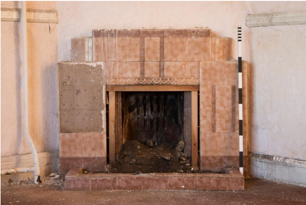
Photo 304: Fireplace to room 45, facing north (1796_304.TIF)
