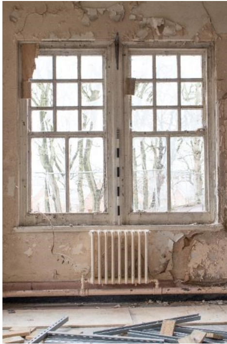
Photo 233: East dayroom windows, facing west (1796_233.TIF)
