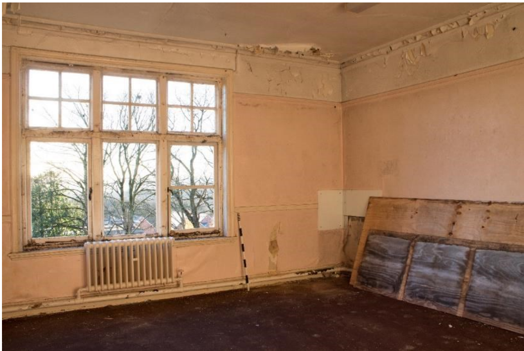
Photo 300: Room 45, facing south-west (1796_300.TIF)
