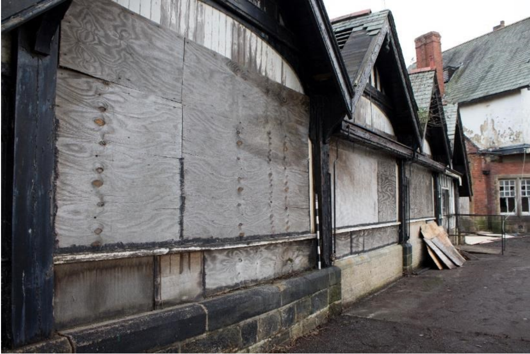
Photo 13: West veranda, facing north-east (1796_013.TIF)
