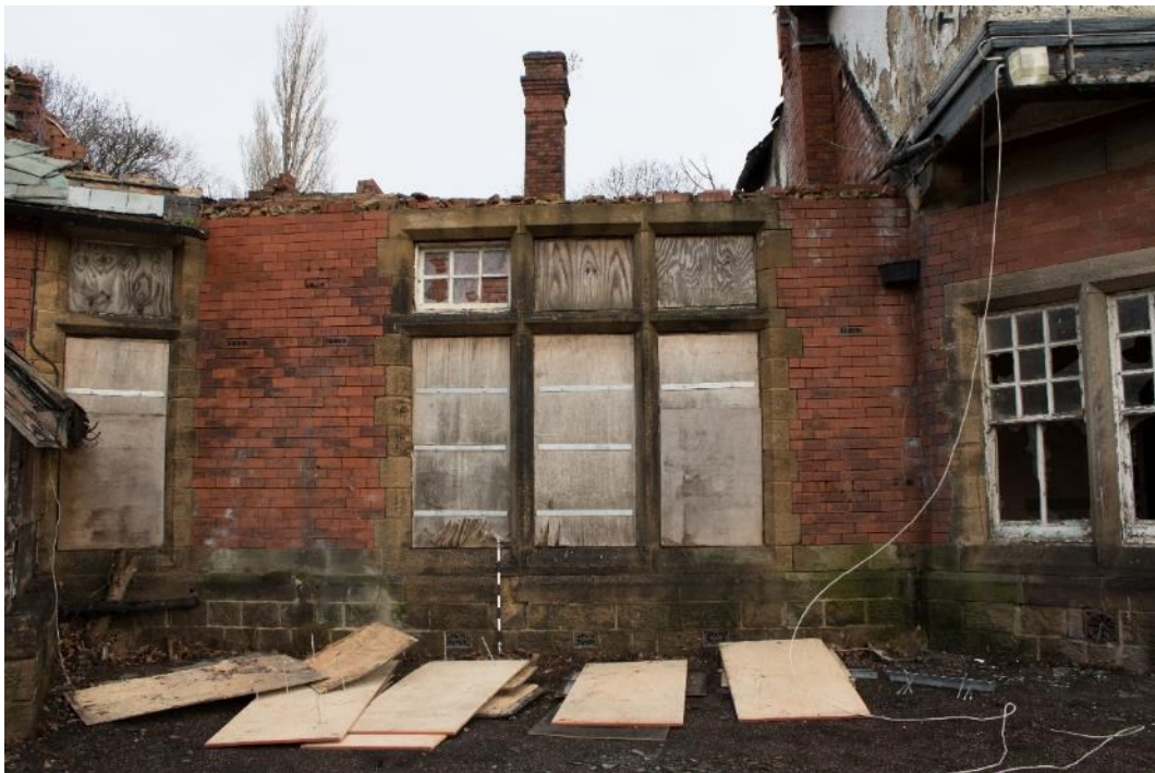
Photo 18: Exterior of room 55, central block, facing north-east (1796_018.TIF)
