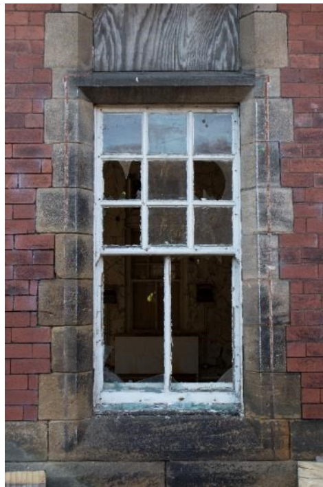
Photo 114: Typical east wing sash window, facing west (1796_114.TIF)
