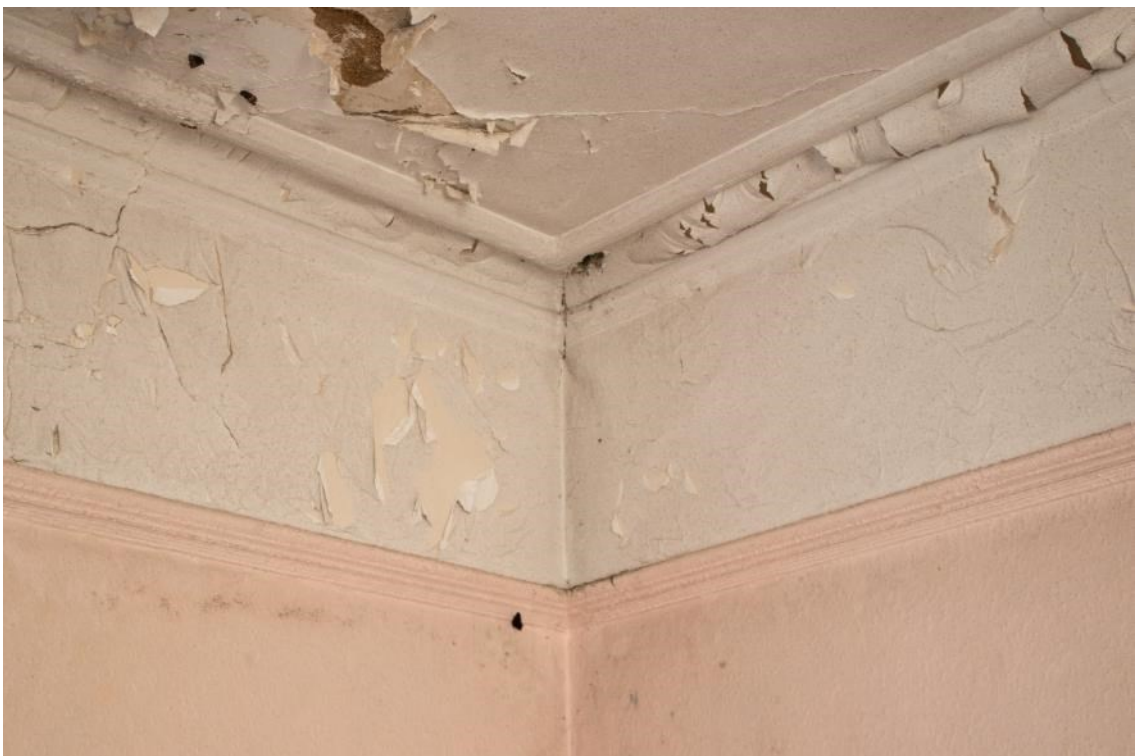
Photo 306: Picture rail and cornice in room 45, facing west (1796_306.TIF)
