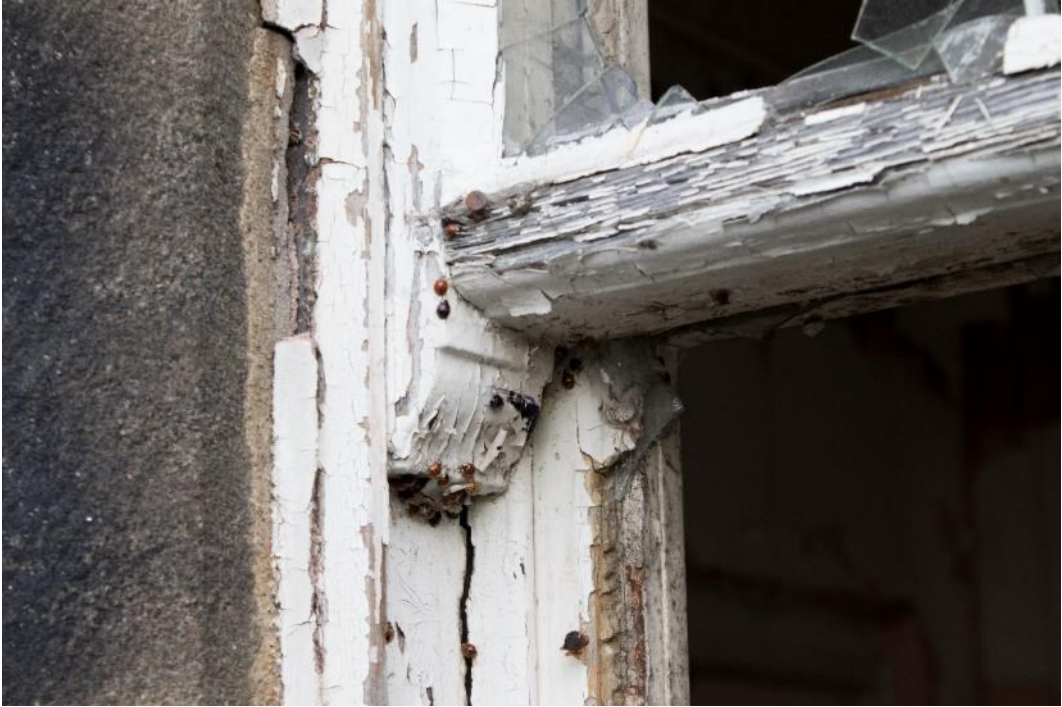
Photo 25: Sash window horn, facing north-east (1796_025.TIF)
