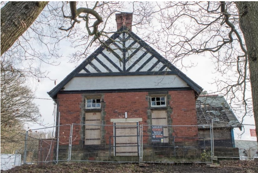
Photo 50: West elevation of west wing, facing east (1796_050.TIF)
