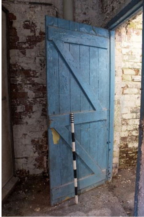
Photo 183: Door to room 24, facing south-east (1796_183.TIF)
