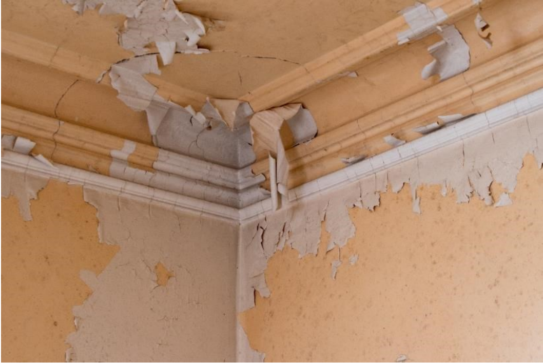
Photo 119: Room 2 cornice, facing west (1796_119.TIF)
