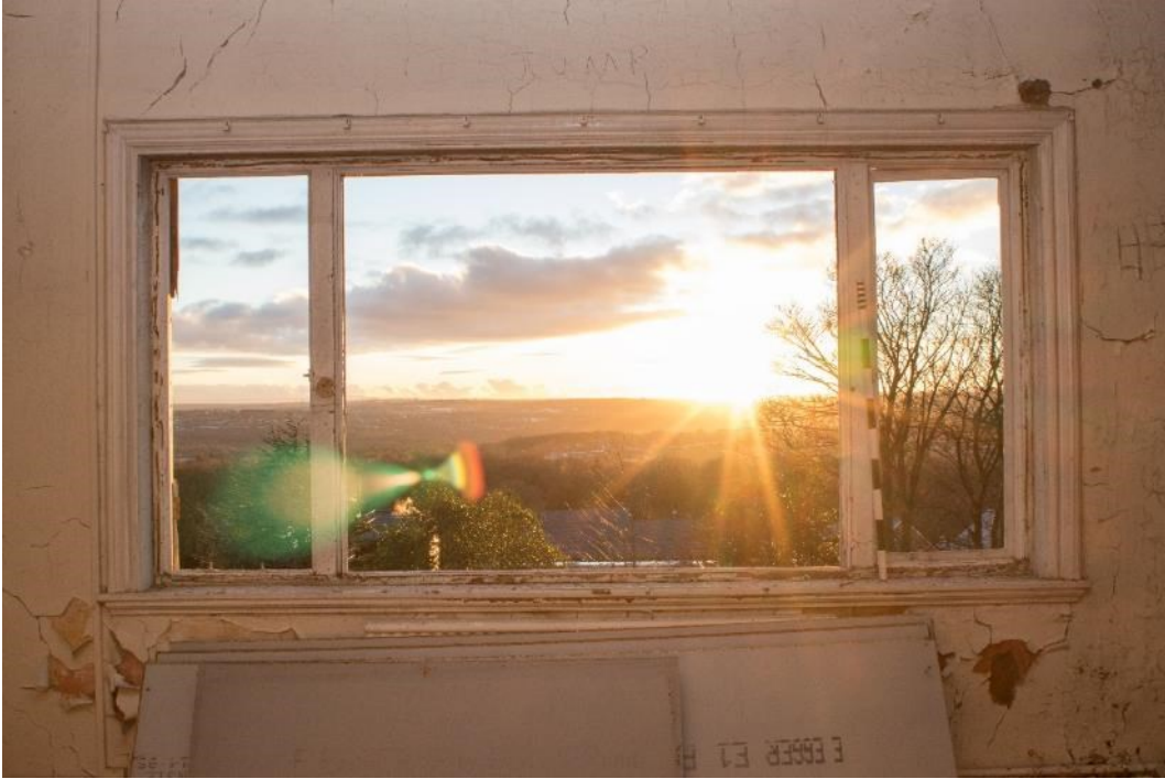
Photo 321: East window to room 47, facing south-east (1796_321.TIF)
