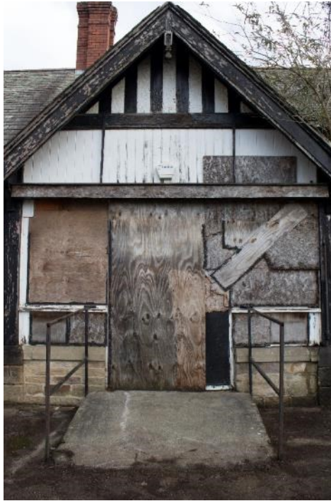
Photo 37: Entrance bay to east veranda, facing north-east (1796_037.TIF)
