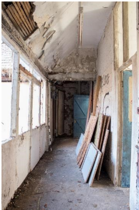
Photo 178: Service range corridor/enclosed veranda, facing south-east (1796_178.TIF)
