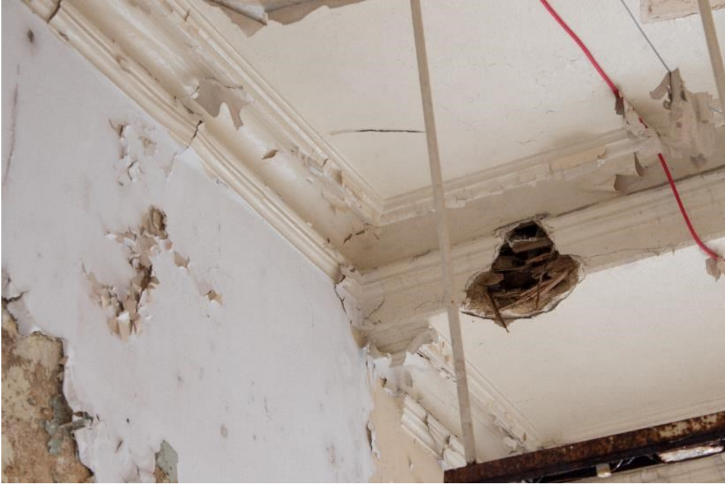
Photo 237: Cornicing in south entrance corridor, facing south (1796_237.TIF)
