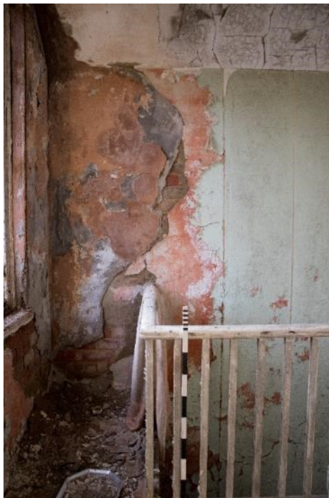
Photo 196: Room 53, facing south-west (1796_190.TIF)
