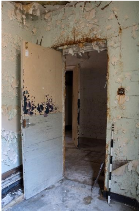
Photo 207: Room 36, facing west (1796_207.TIF)
