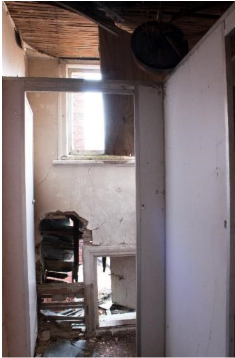
Photo 329: Second floor W.C. (50), facing north-west (1796_329.TIF)
