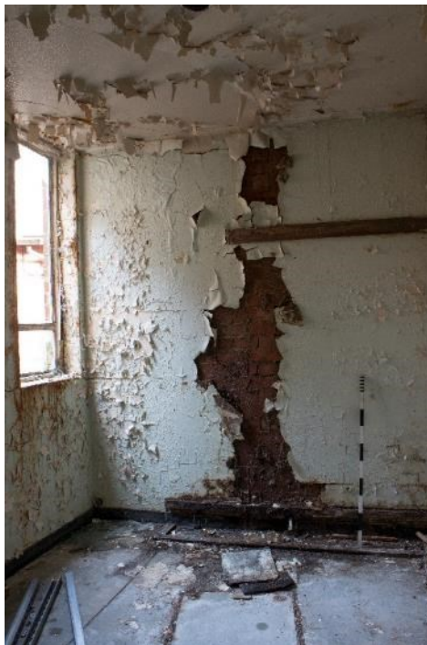
Photo 206: Room 36, facing east (1796_206.TIF)
