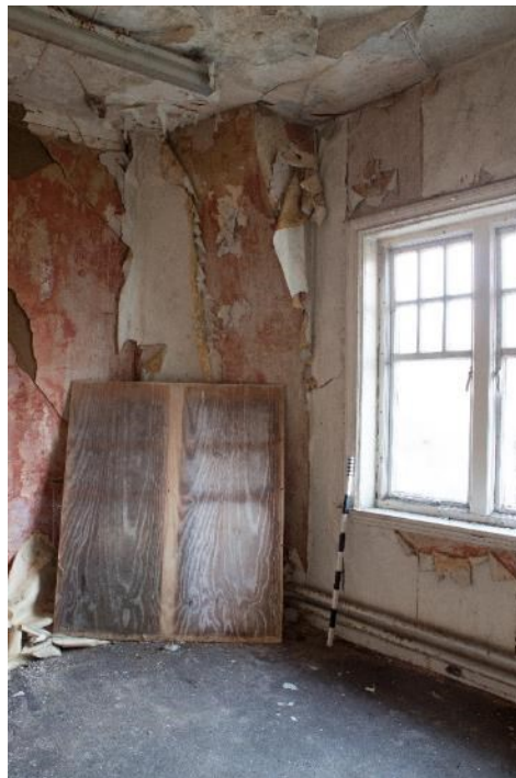
Photo 324: Room 48, facing north (1796_324.TIF)
