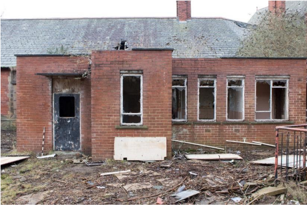
Photo 107: East wing wash block, north elevation (1796_107.TIF)
