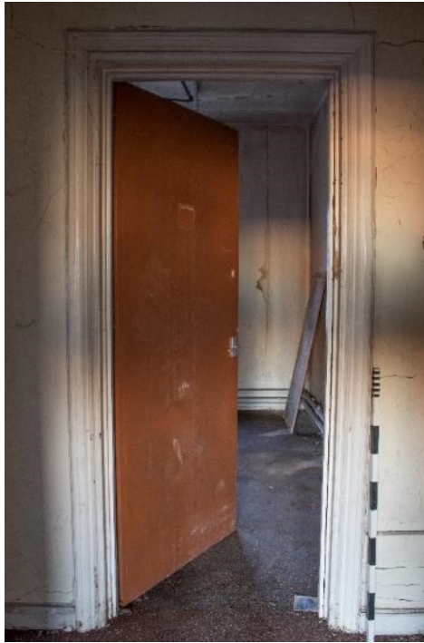
Photo 331: Doorway to room 48, facing north-east (1796_331.TIF)
