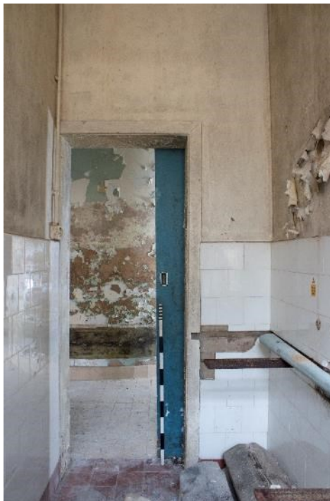
Photo 132: Room 5 facing south-west (1796_132.TIF)
