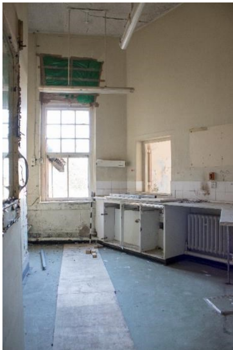
Photo 268: Room 26, facing west (1796_268.TIF)
