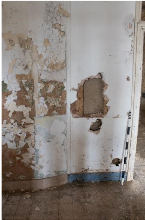
Photo 243: Inserted partition between north and central block corridors, facing north-east (1796_243.TIF)
