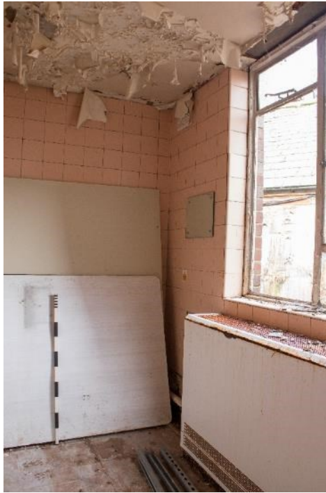
Photo 219: Room 33, facing north, (1796_219.TIF)
