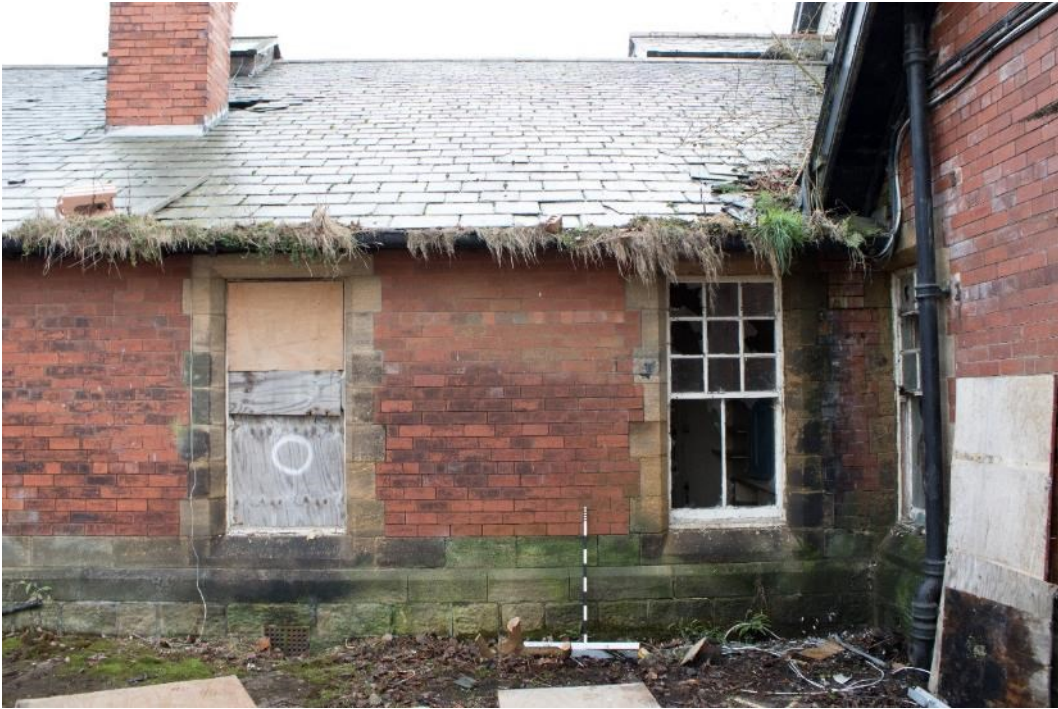
Photo 97: West elevation of north block (1796_097.TIF)
