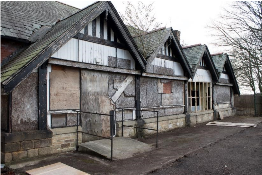
Photo 36: East veranda, facing east (1796_036.TIF)
