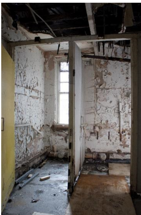
Photo 129: Room 11, facing north-east (1796_129.TIF)
