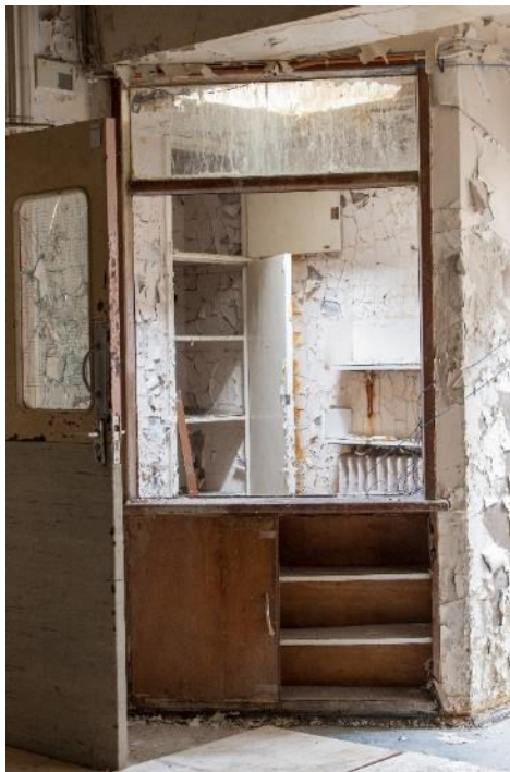
Photo 212: Room 34 as viewed from the east ward, facing north (1796_212.TIF)
