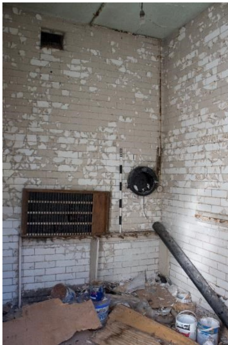
Photo 176: Mortuary (51), facing north-east (1796_176.TIF)
