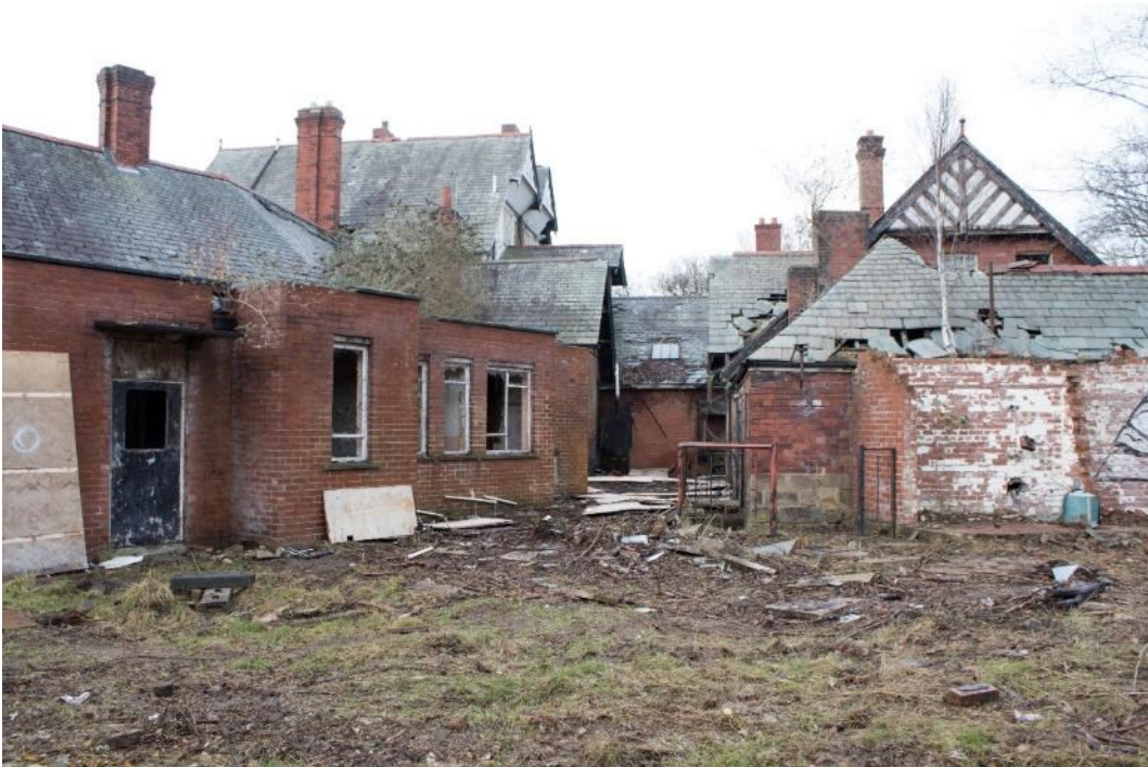
Photo 86: East side of the hospital, facing north-west (1796_086.TIF)
