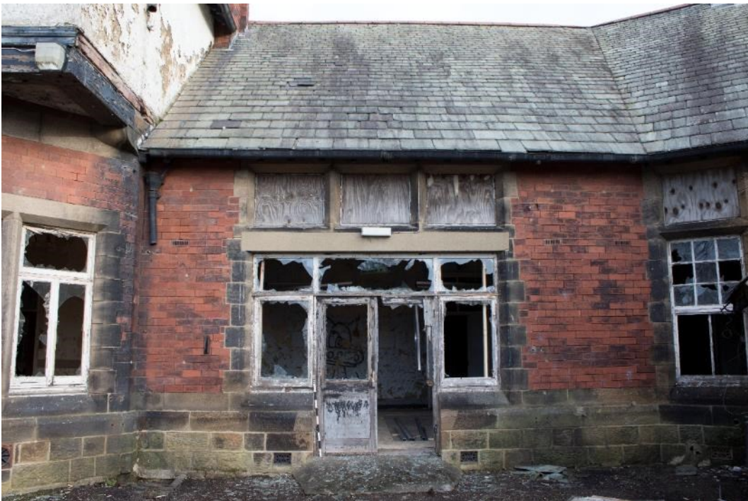
Photo 34: Exterior of room 38, facing north east (1796_034.TIF)
