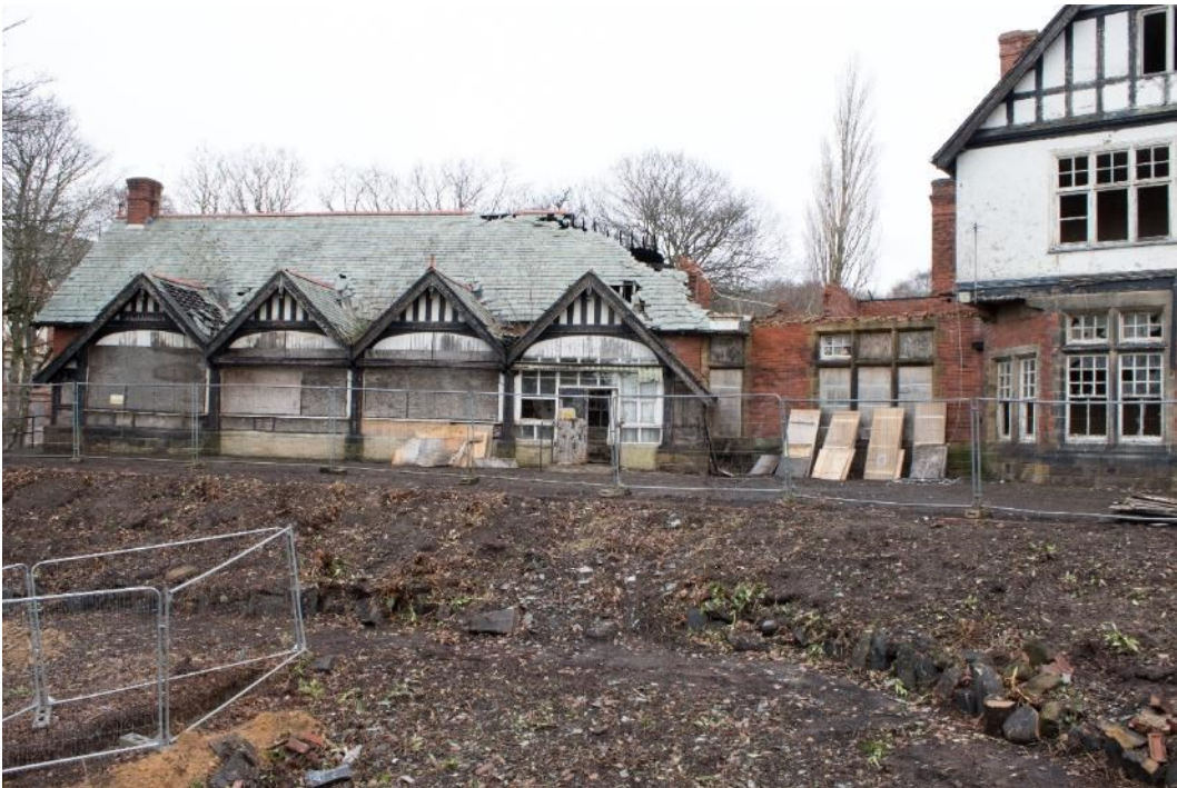
Photo 6: West wing, south elevation (1796_006.TIF)
