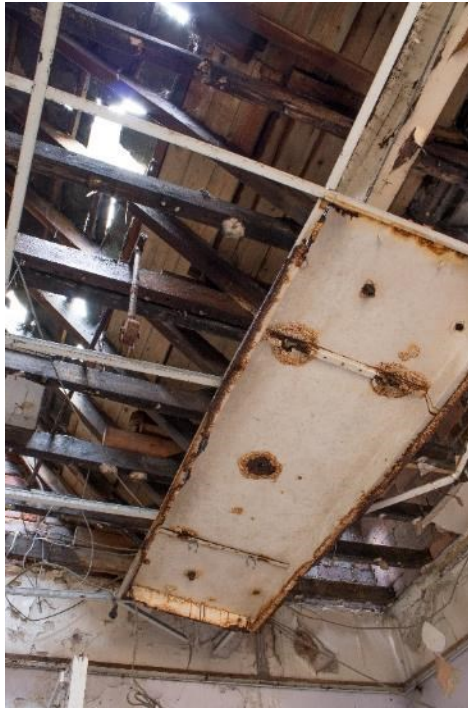
Photo 205: Ceiling above room 12, facing south-west (1796_205.TIF)
