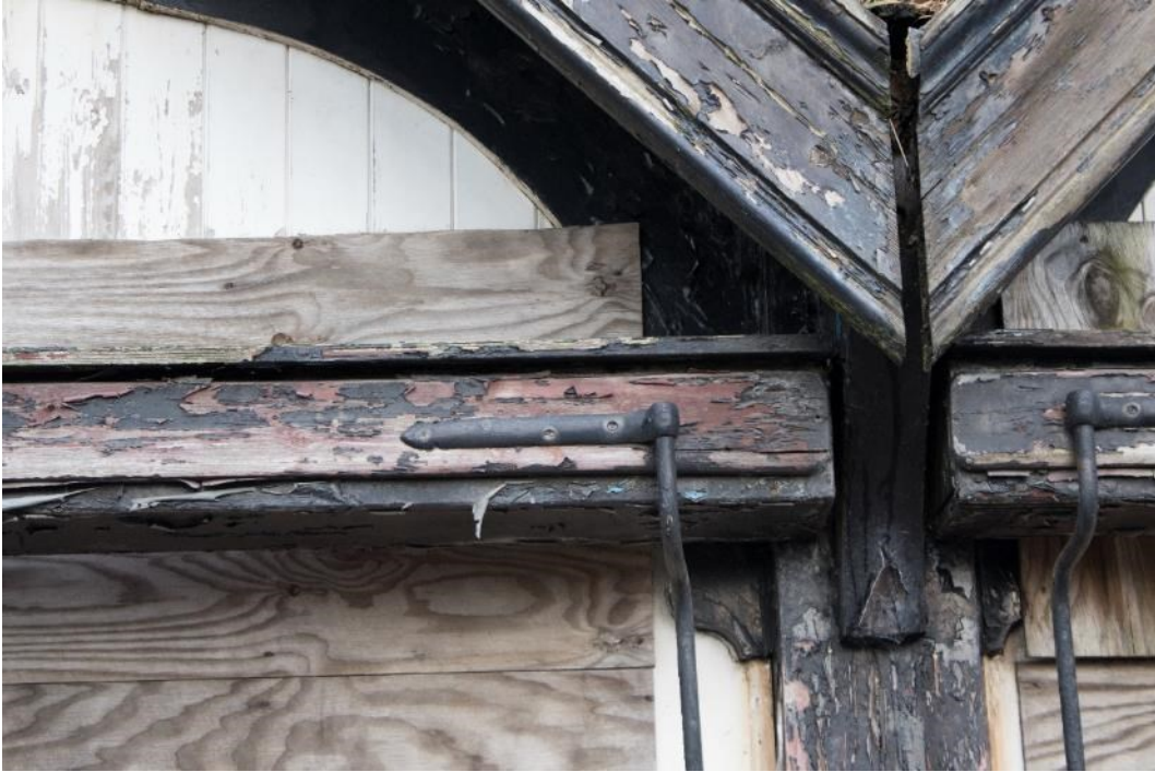
Photo 15: West veranda, awning obscuring arch brace, facing north (1796_015.TIF)
