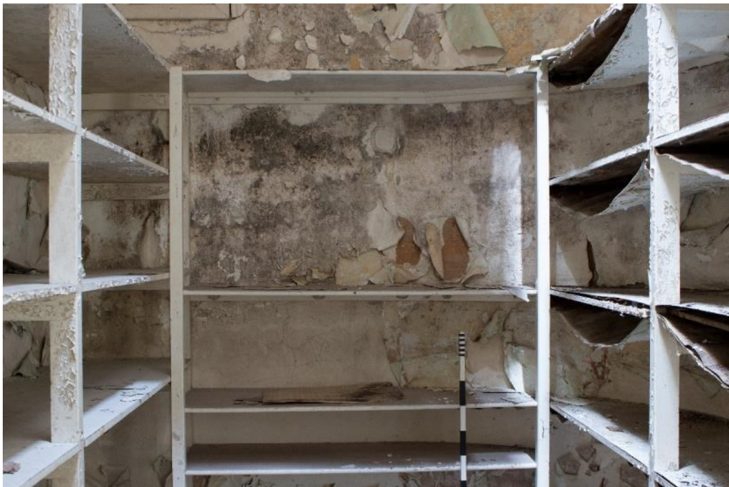
Photo 136: Room 7, facing north-west (1796_136.TIF)
