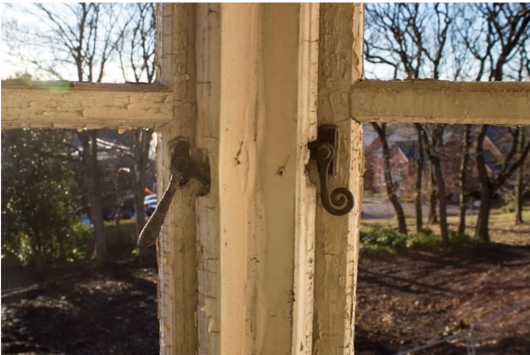
Photo 290: Details of window fittings in room 44, facing south-west (1796_290.TIF)
