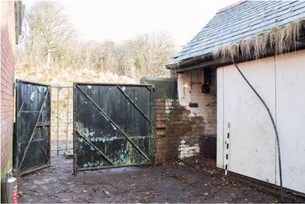
Photo 187: Kitchen courtyard, facing north-east (1796_187.TIF)
