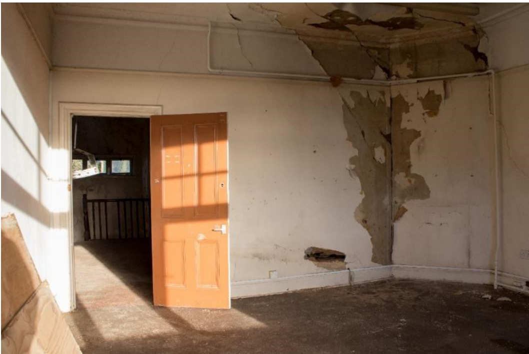
Photo 282: Room 43, facing north-east (1796_282.TIF)
