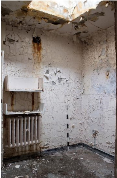
Photo 211: Room 34, facing east (1796_211.TIF)
