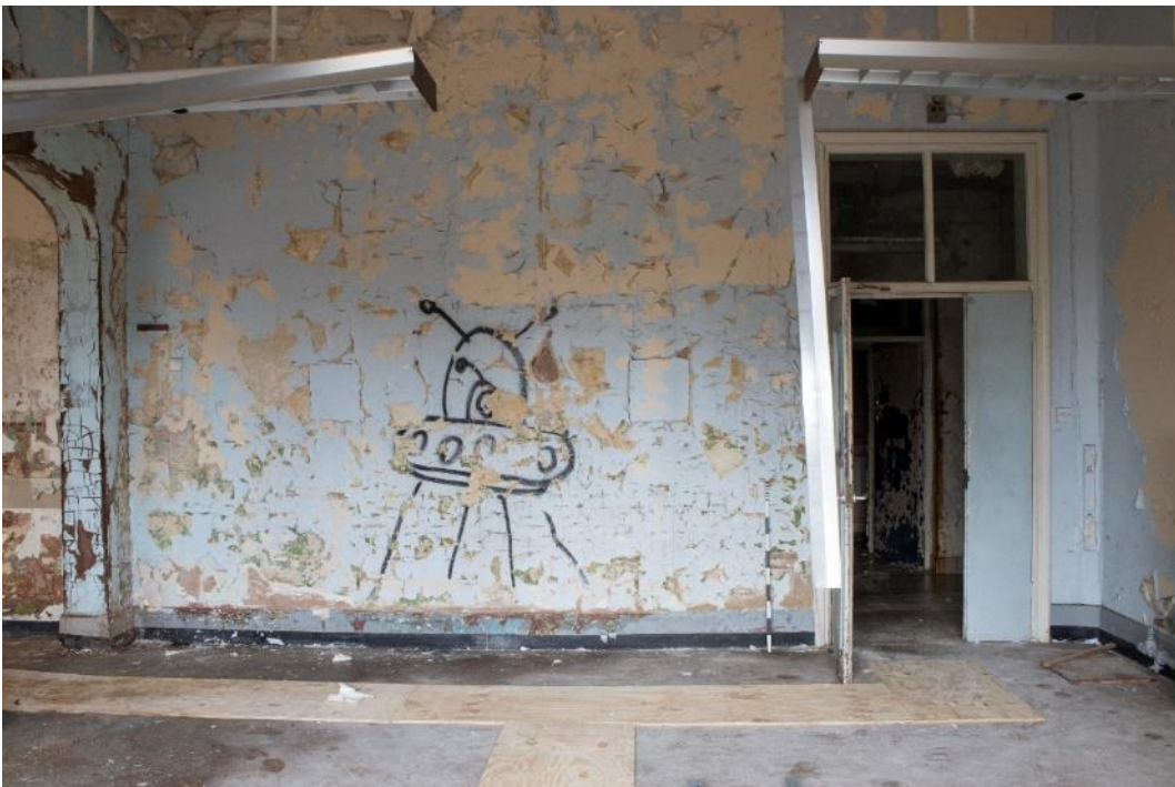
Photo 254: Room 38, facing north-east (1796_254.TIF)
