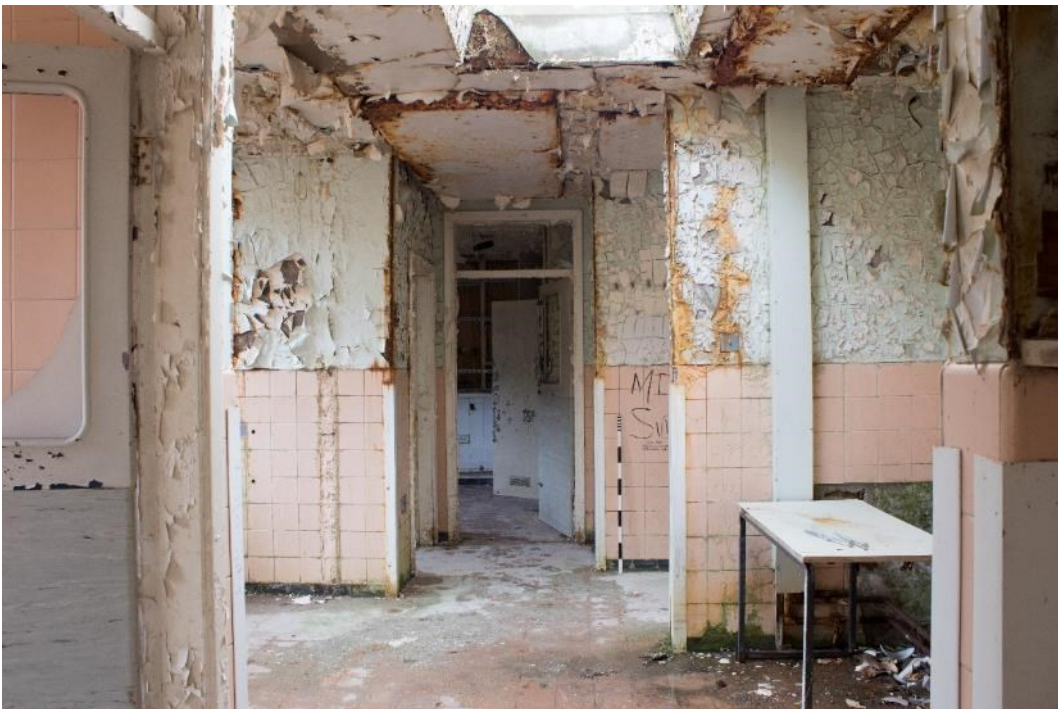
Photo 216: East wing wash block (31), facing south (1796_216.TIF)
