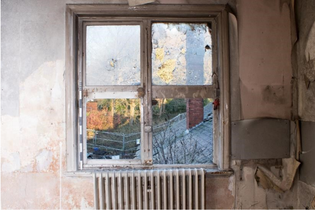
Photo 309: Window to room 46, facing north-east (1796_309.TIF)
