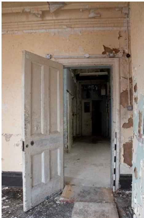
Photo 118: Room 2 door, facing south-east (1796_118.TIF)
