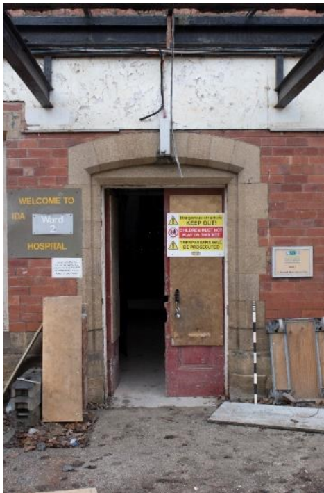
Photo 72: Entrance to north block, facing south-west (1796_072.TIF)
