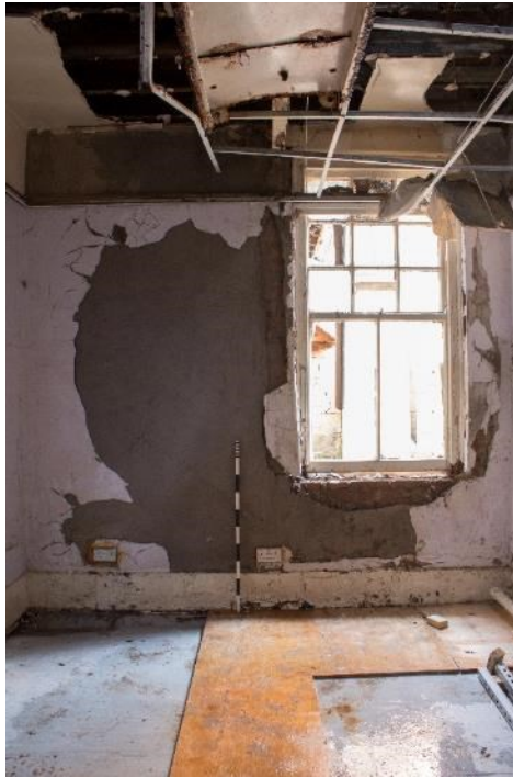
Photo 203: Room 12, facing north-east (1796_203.TIF)
