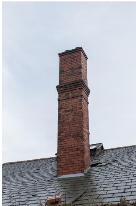
Photo 98: Chimneystack above north block, facing south-west (1796_098.TIF)
