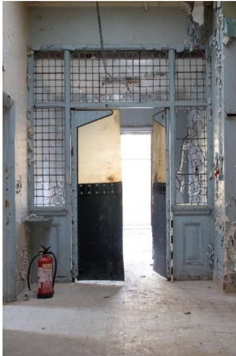
Photo 145: North entrance to north block, facing north-east (1796_148.TIF)
