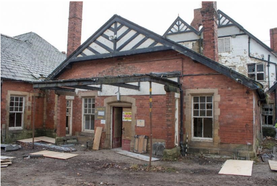
Photo 70: North elevation of north block (1796_070.TIF)
