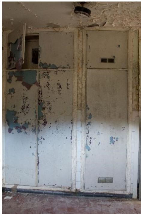
Photo 226: Cupboards in room 29, facing west (1796_226.TIF)
