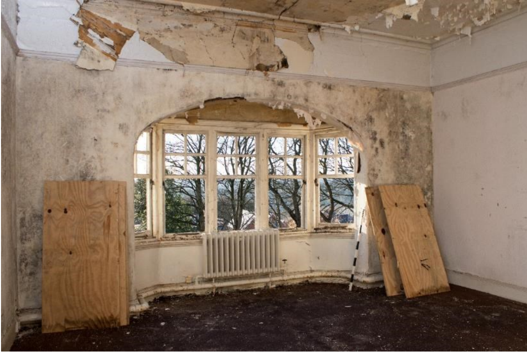
Photo 285: Room 44, facing west (1796_285.TIF)
