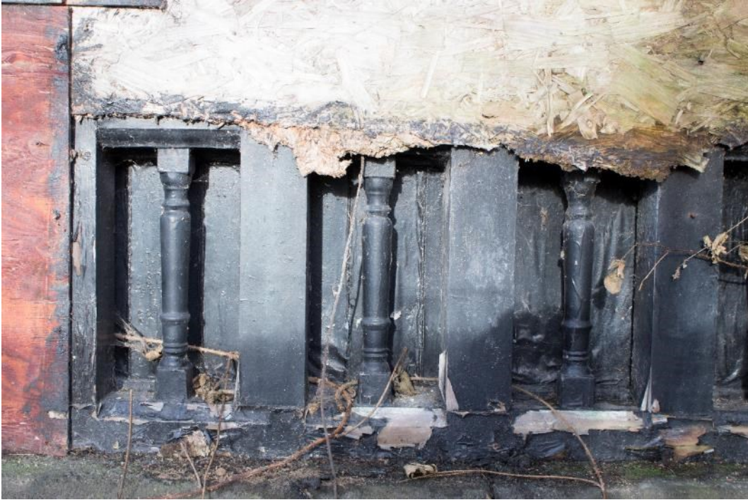
Photo 43: Detail of east veranda return elevation, facing north (1796_043.TIF)
