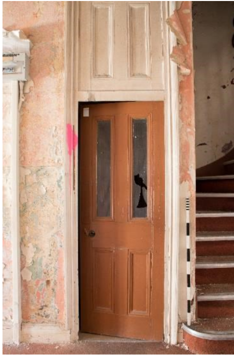
Photo 295: Door to room 41, facing south-east (1796_295.TIF)
