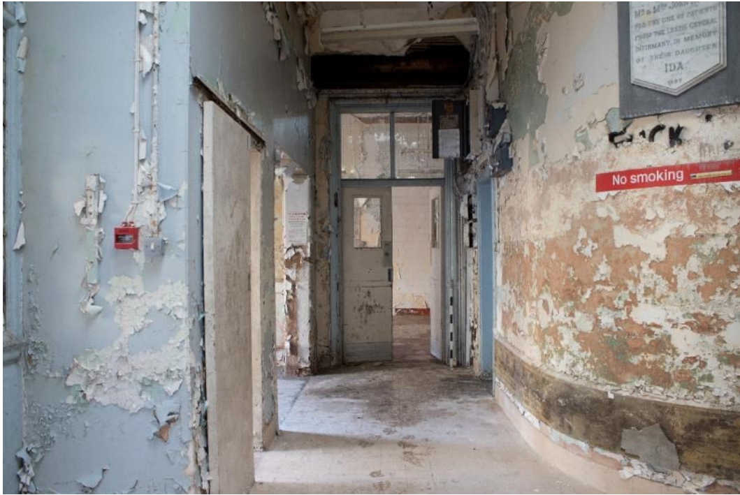
Photo 141: Kitchen corridor, facing south-east (1796_141.TIF)
