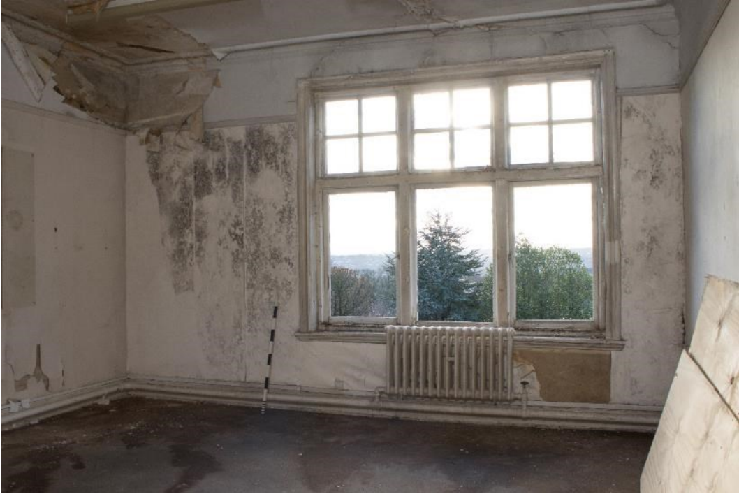
Photo 281: Room 43, facing south west (1796_281.TIF)
