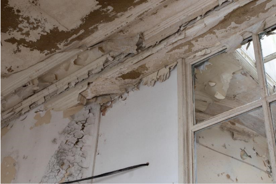
Photo 245: Inserted partition between north and central block corridors, facing north (1796_245.TIF)
