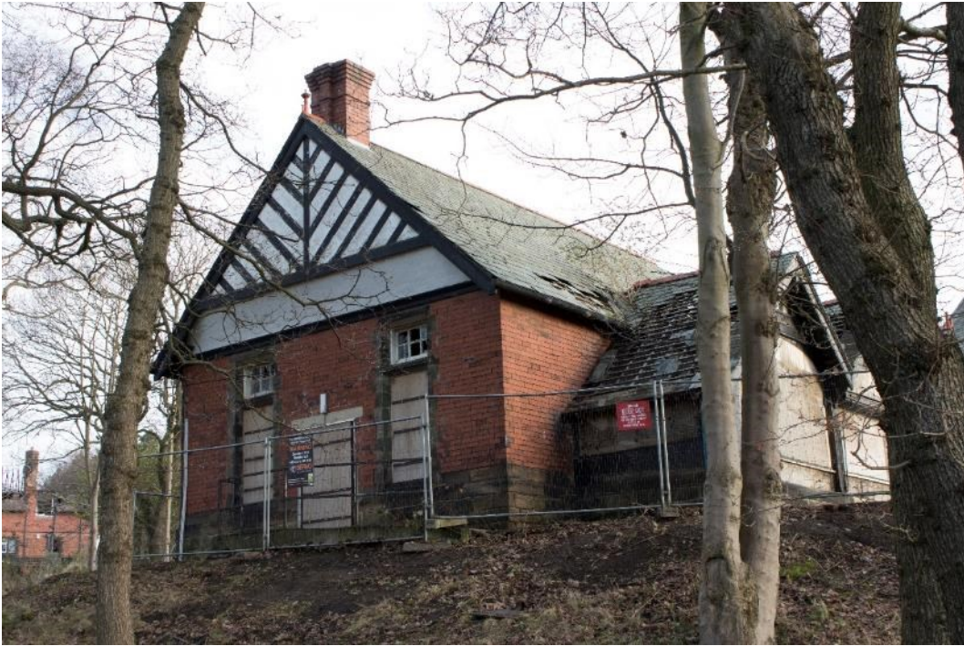
Photo 49: West elevation of west wing, facing east (1796_049.TIF)
