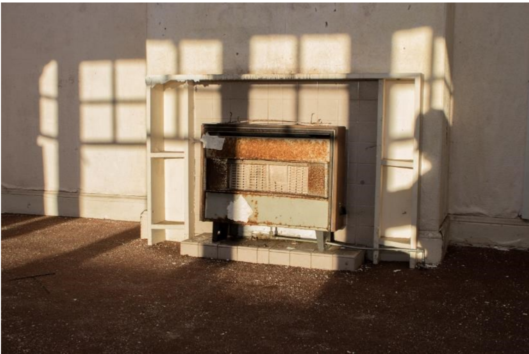
Photo 288: Fireplace to room 44, facing north-east (1796_288.TIF)
