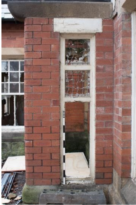
Photo 73: Glazed stub-wall to north of north block, facing south-east (1796_073.TIF)
