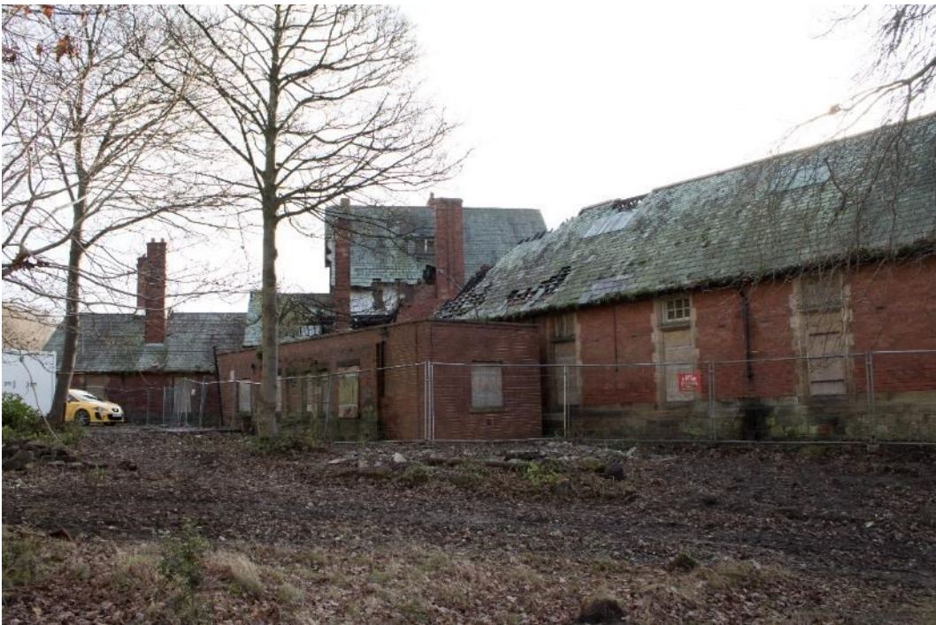
Photo 52: General view of the rear of the hospital, facing south-east (1796_052.TIF)
