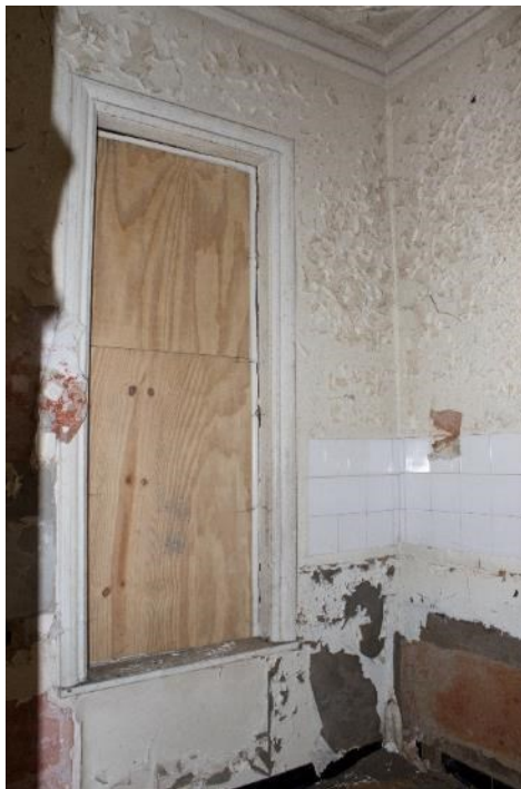
Photo 314: Room 41, facing east (1796_314.TIF)
