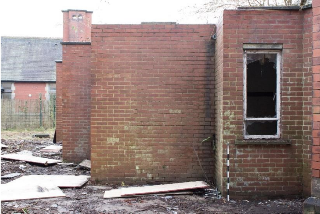
Photo 103: West elevation of east wing was block (1796_103.TIF)
