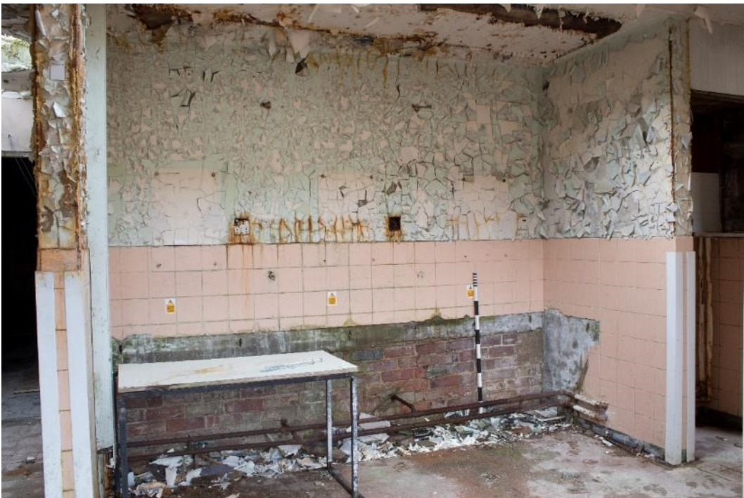
Photo 222: Location of wash basins in room 31, facing west (1796_222.TIF)
