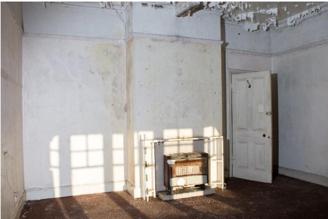
Photo 286: Room 44, facing north-east (1796_286.TIF)
