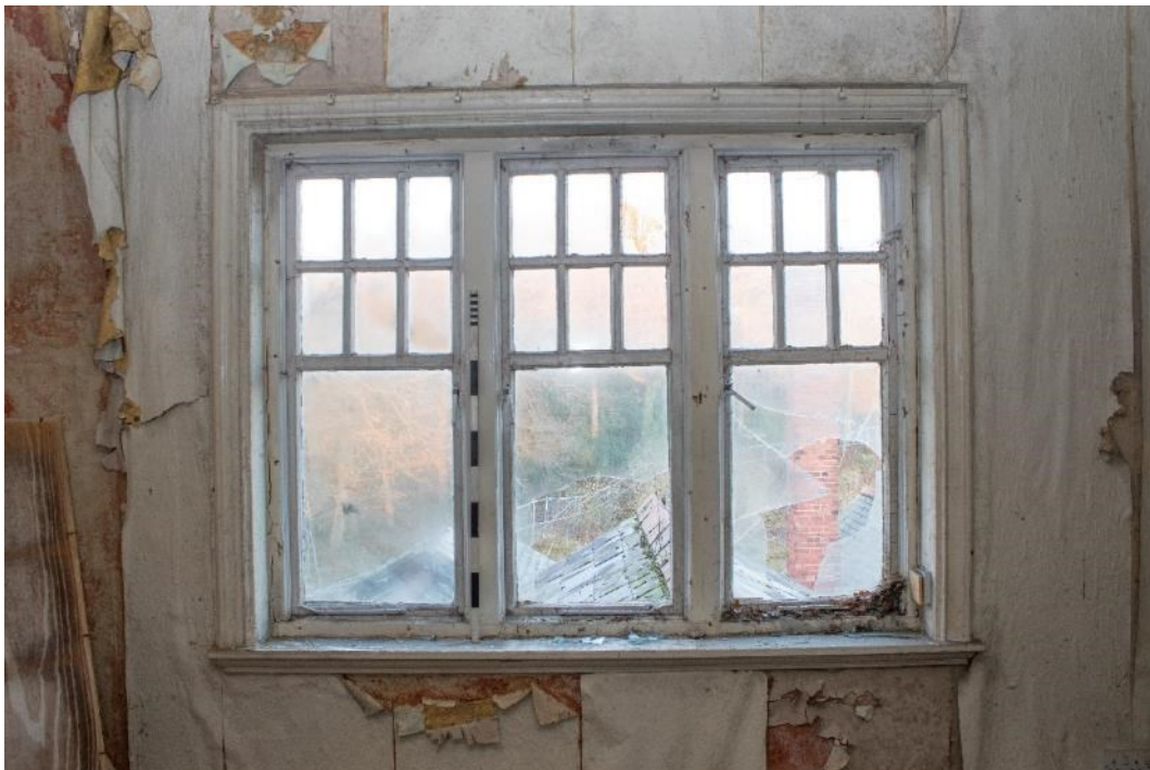
Photo 326: Window to room 48, facing north-east (1796_326.TIF)
