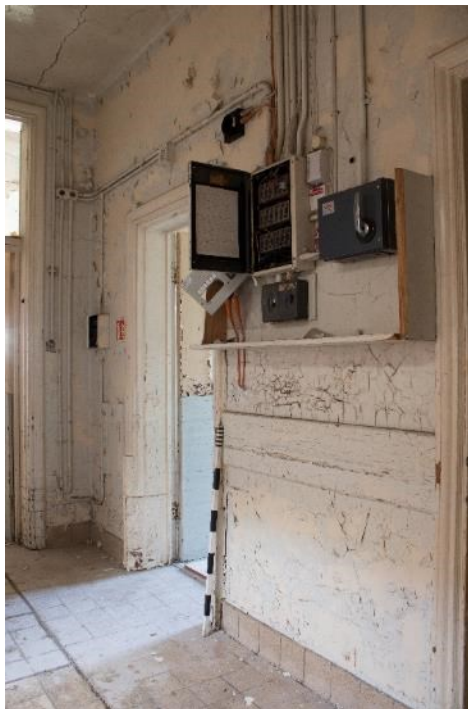
Photo 266: South side of east end of east-west corridor, facing south (1796_266.TIF)
