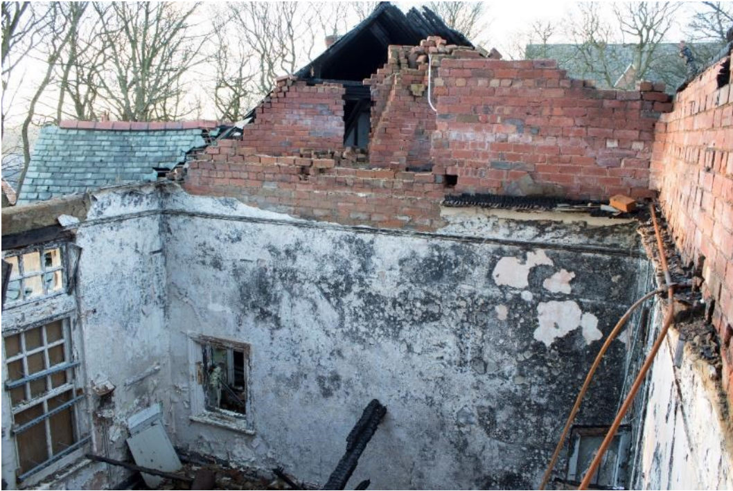
Photo 311: Room 55 viewed from roof access hatch in room 46, facing west (1796_311.TIF)
