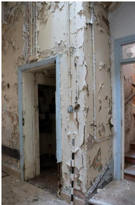
Photo 152: Entrance to cupboard under stairs, facing east (1796_152.TIF)
