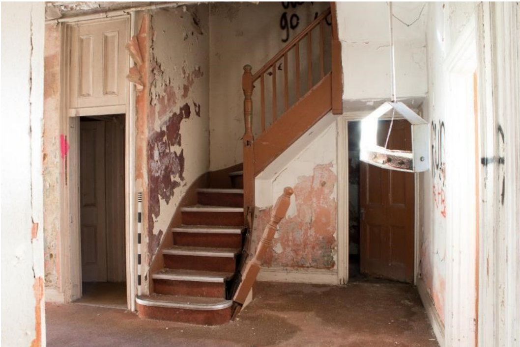
Photo 294: Stairs to second floor, facing south-east (1796_294.TIF)
