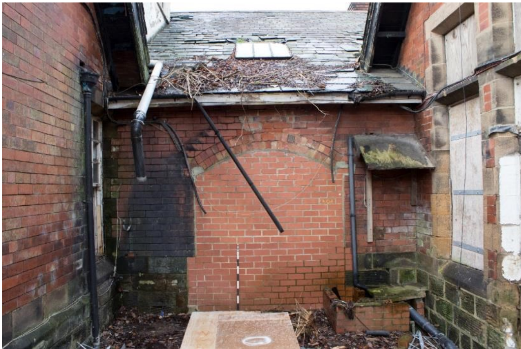
Photo 100: Blocked entrance to east elevation of north block, facing north-east (1796_100.TIF)
