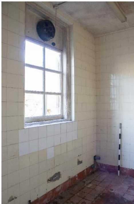
Photo 164: Room 18, facing east (1796_164.TIF)
