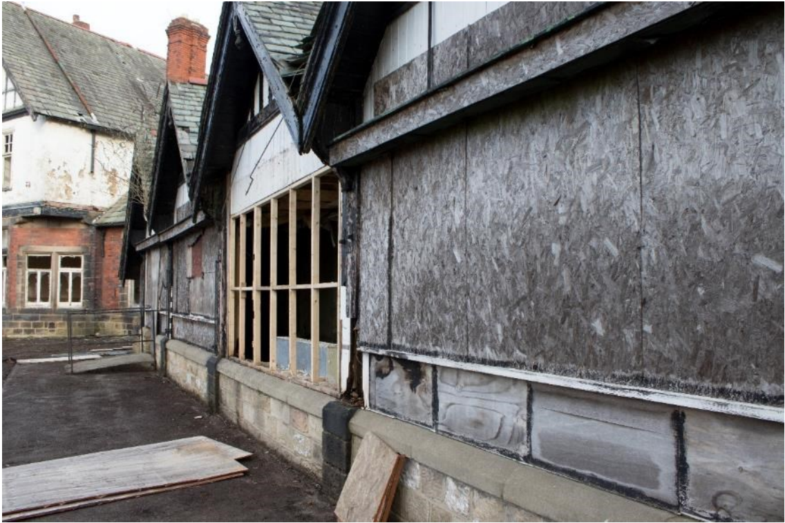
Photo 39: East veranda, facing north (1796_039.TIF)
