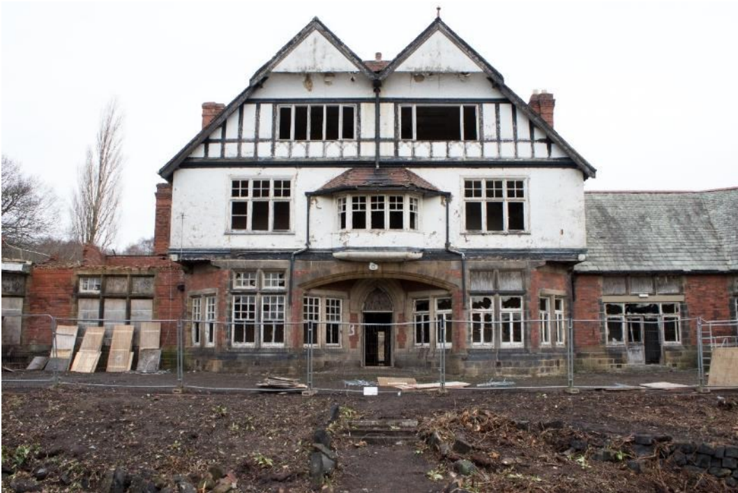
Photo 4 Central block, south elevation (1796_004.TIF)
