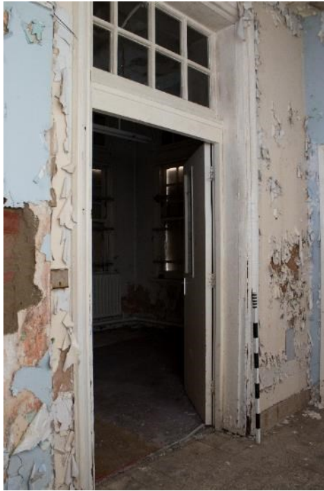
Photo 261: Door to room 13, facing east (1796_261.TIF)
