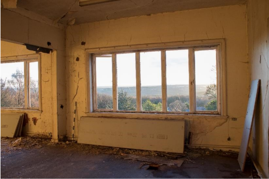
Photo 317: West half of room 47, facing south (1796_317.TIF)
