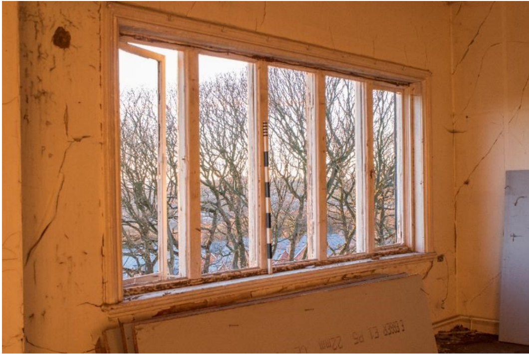
Photo 323: West window to room 47, facing west (1796_323.TIF)
