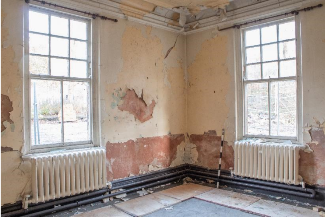
Photo 115: Interior of room 1, facing north (1796_115.TIF)
