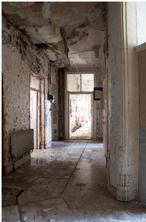
Photo 262: East end of east-west corridor, facing south (1796_262.TIF)
