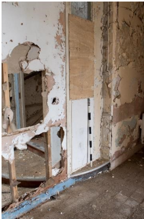
Photo 244: Inserted partition between north and central block corridors, facing east (1796_244.TIF)
