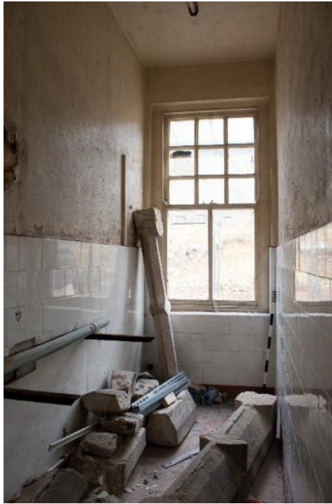
Photo 131: Room 5, facing north-east(1796_131.TIF)
