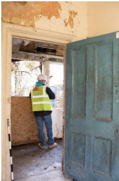
Photo 172: Door to room 21, facing north-east (1796_172.TIF)
