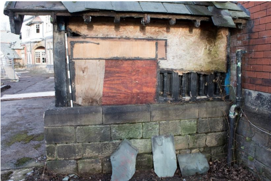
Photo 42: Return elevation of east veranda, facing north (1796_042.TIF)
