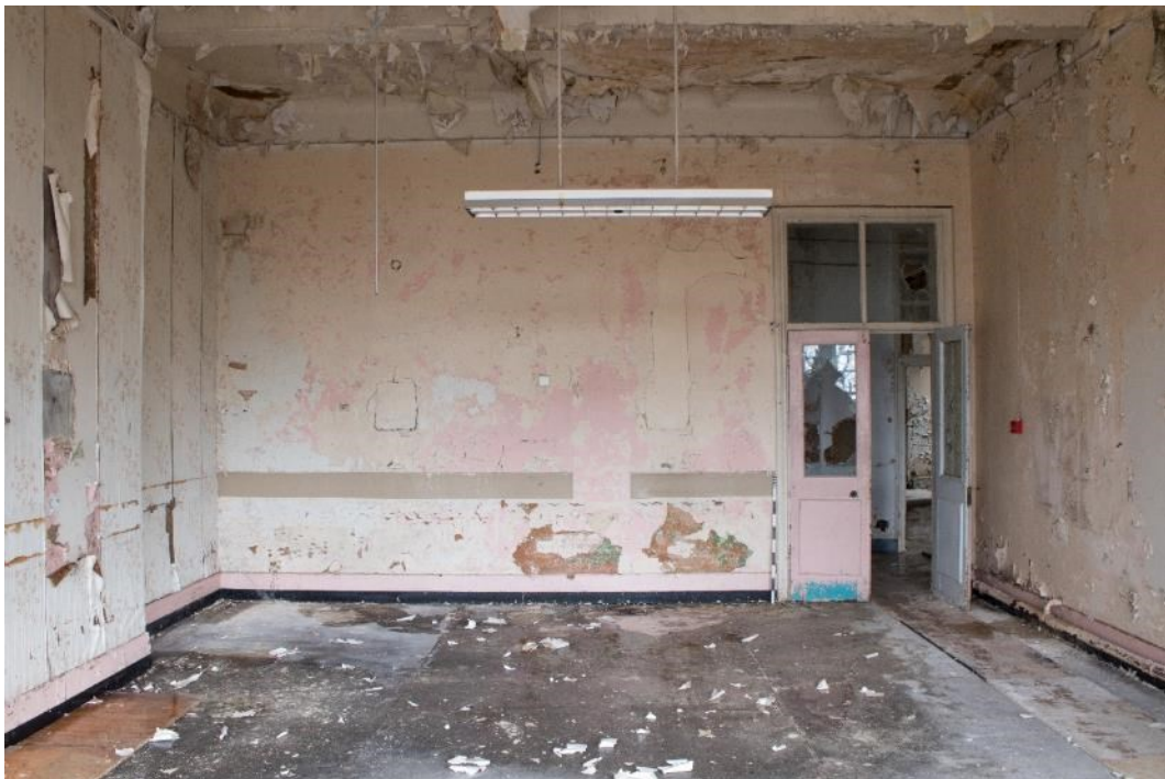
Photo 230: East dayroom (15), facing north-east (1796_2.TIF)
