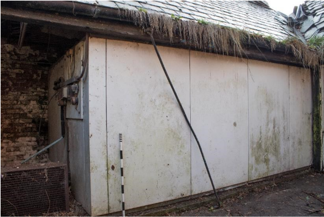
Photo 189: Large refridgerator in kitchen courtyard, facing south-east (1796_189.TIF)
