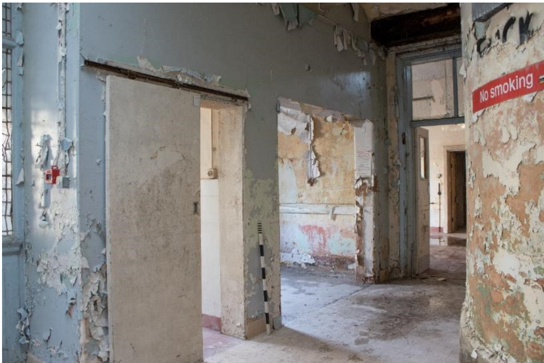
Photo 146: Kitchen corridor, facing east (1796_146.TIF)
