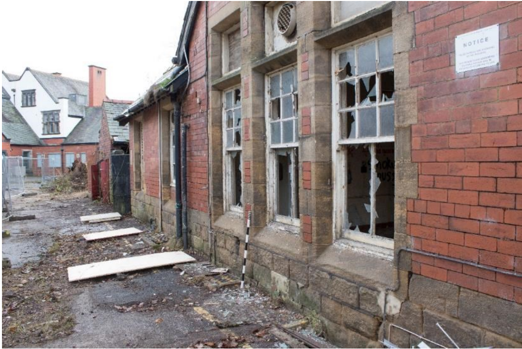
Photo 75: Oblique view of service range north elevation, facing south-east (1796_075.TIF)
