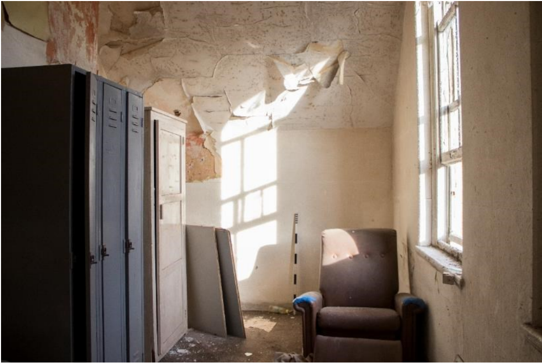
Photo 199: Room 54, facing north-east (1796_199.TIF)
