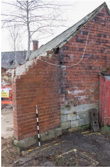
Photo 83: Partially demolished extension to east of service range, facing south-west (1796_083.TIF)
