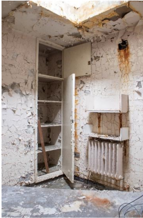
Photo 213: Room 34, facing north (1796_213.TIF)
