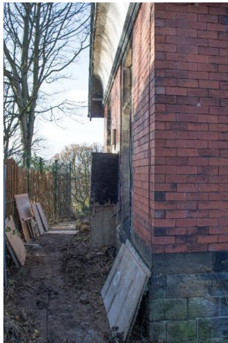
Photo 110: Very oblique view of east wing east elevation, facing south-west (1796_110.TIF)
