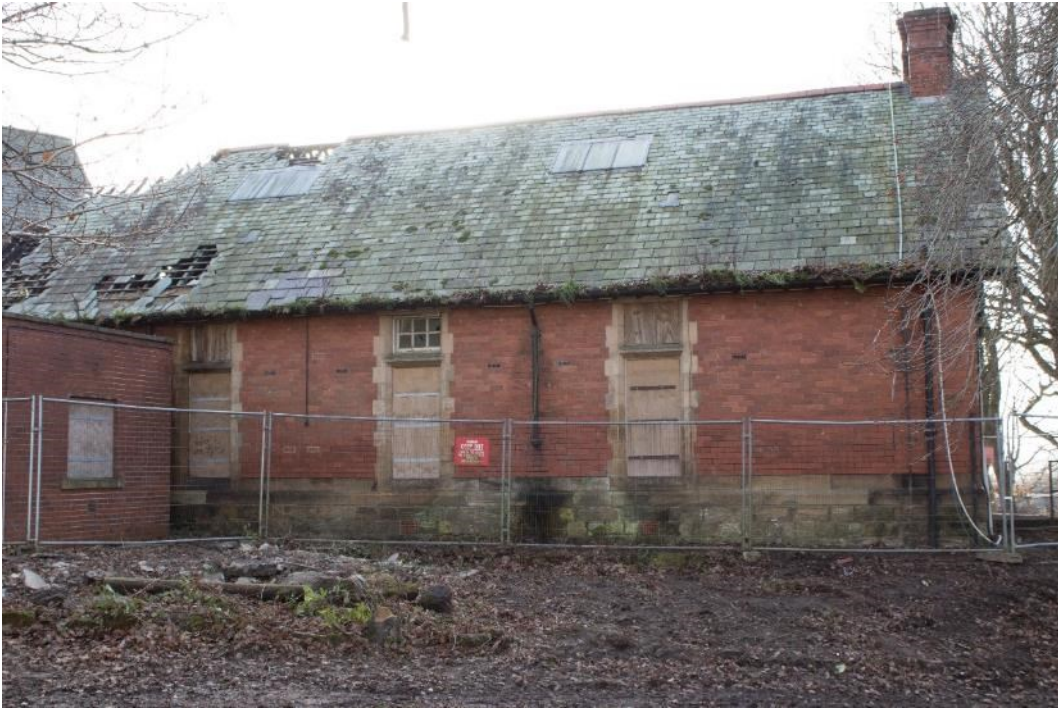
Photo 53: North elevation of west wing (1796_053.TIF)
