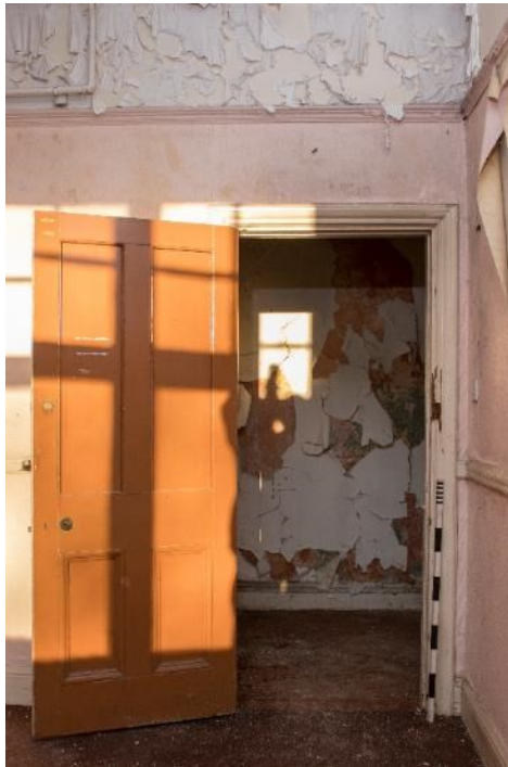
Photo 302: Door to room 45, facing north-east (1796_302.TIF)
