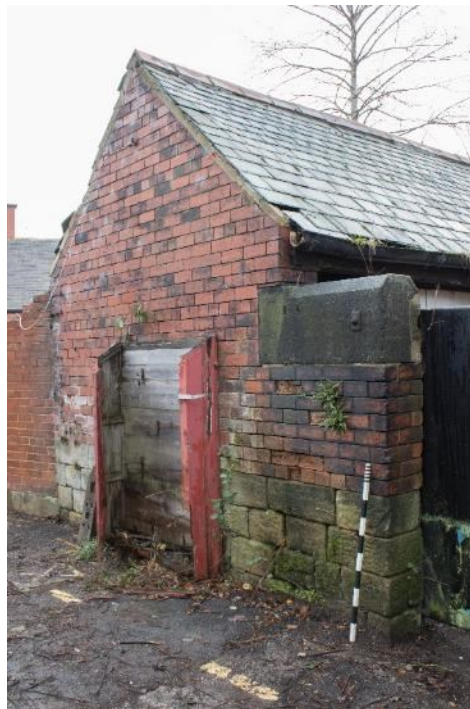
Photo 82: North elevation of service range (1796_082.TIF)
