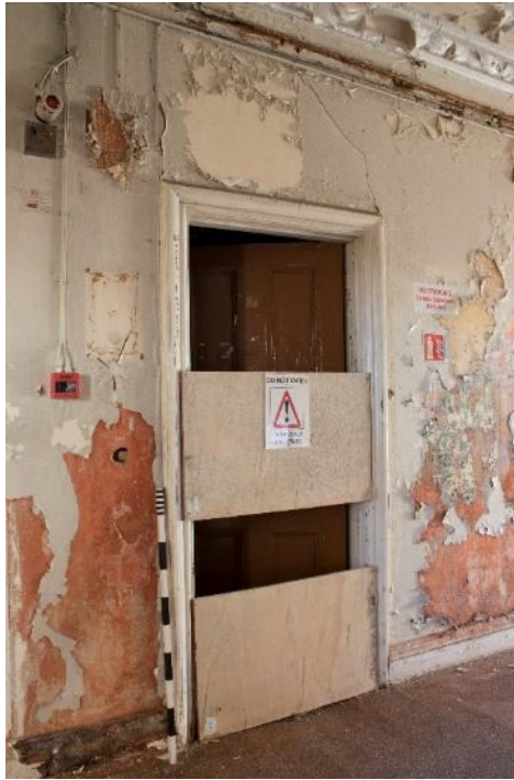
Photo 297: Door to room 65, facing north (1796_297.TIF)
