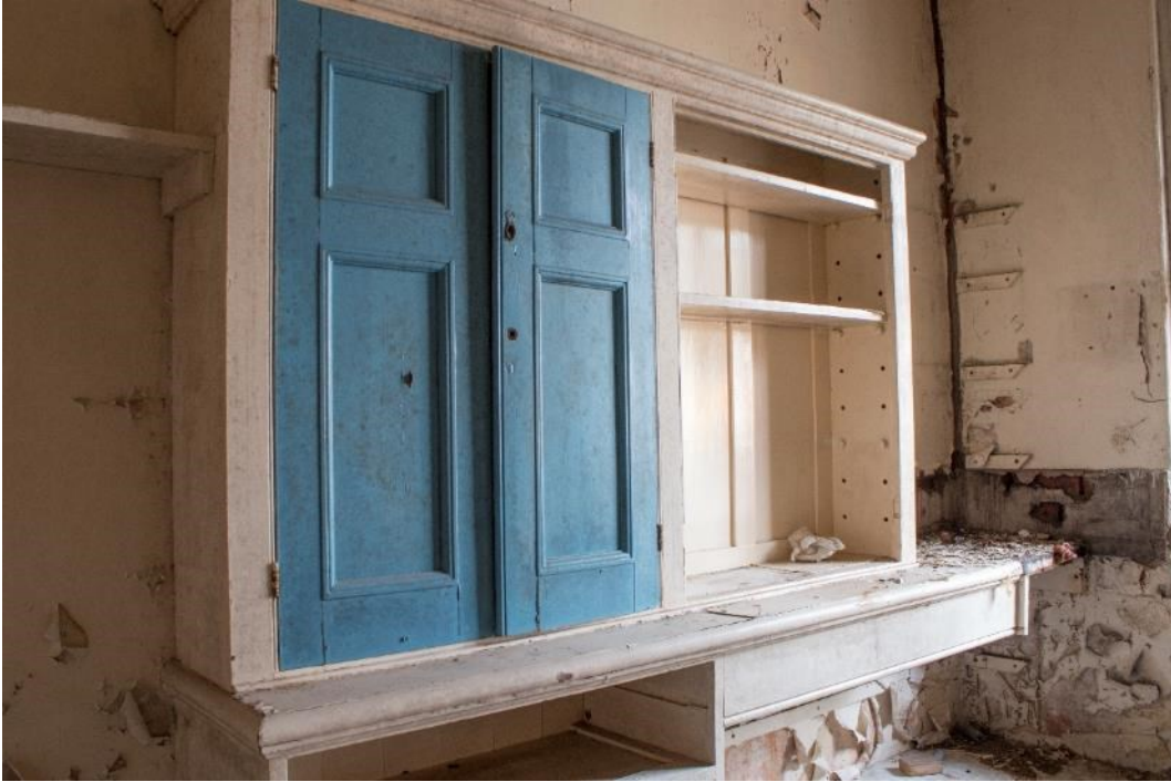
Photo 123: Room 4 cupboard, facing west (1796_123.TIF)
