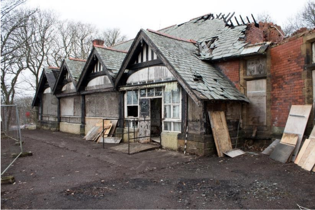
Photo 7: West veranda, facing west (1796_007.TIF)
