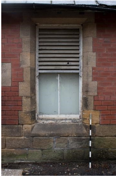
Photo 79: Window to service range fridge (52), facing south-west (1796_079.TIF)
