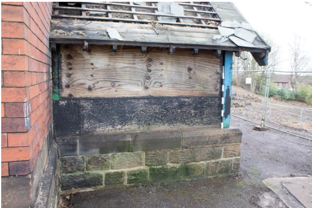
Photo 10: Side elevation of west veranda, facing east (1796_010.TIF)
