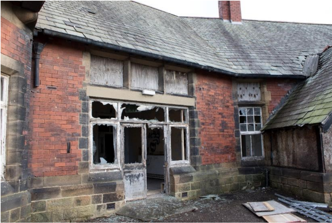
Photo 35: Exterior of room 38, facing east (1796_035.TIF)
