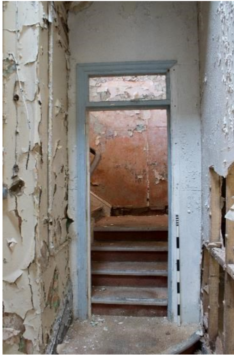
Photo 151: Stairs to first floor, facing south-east (1796_151.TIF)
