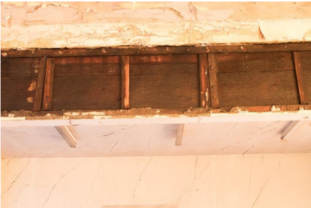
Photo 322: Beam above room 47, facing south-west (1796_322.TIF)
