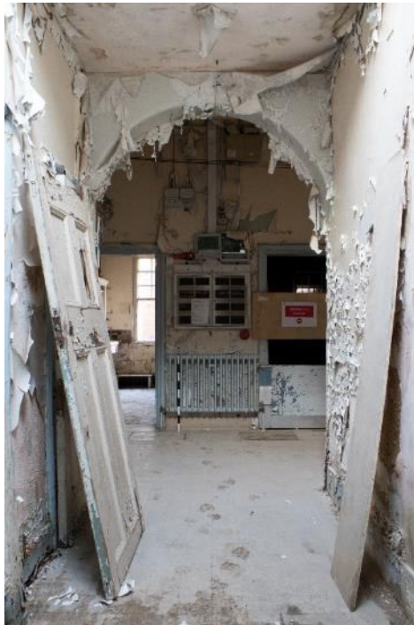
Photo 144: North block corridor to Arthington Hospital, facing north-west (1796_144.TIF)
