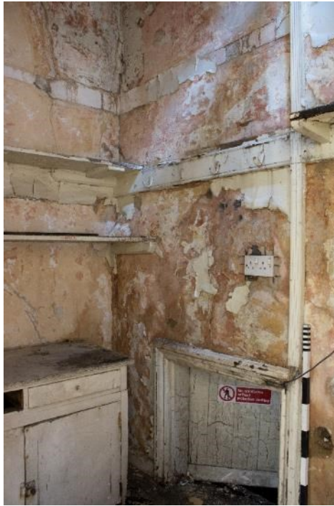
Photo 313: Room 42, facing east (1796_313.TIF)
