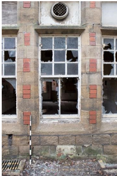
Photo 76: Kitchen windows, facing south-west (1796_076.TIF)
