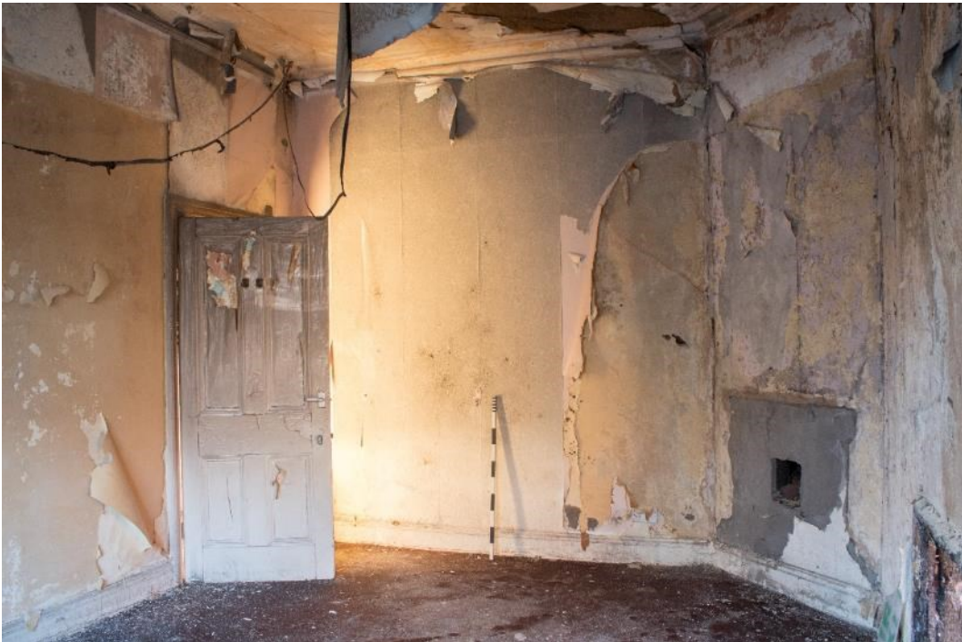
Photo 308: Room 46, facing south-west (1796_308.TIF)
