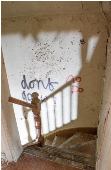
Photo 330: Stairs from first to second floor, facing south-east (1796_330.TIF)
