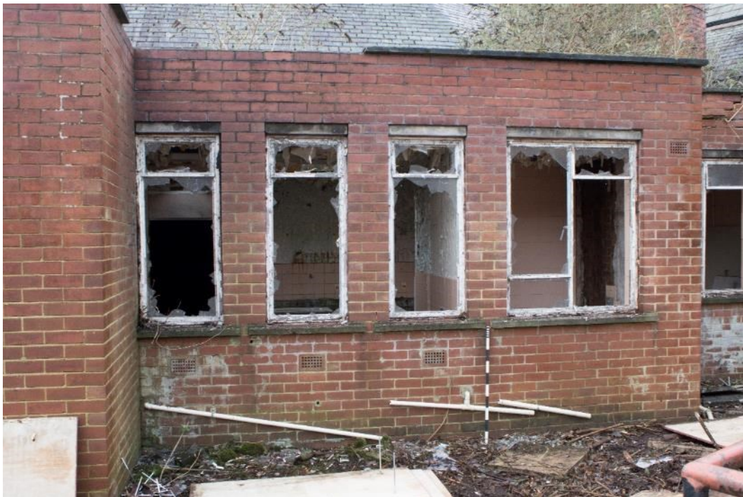
Photo 106: Windows to east wing wash block, facing west (1796_106.TIF)
