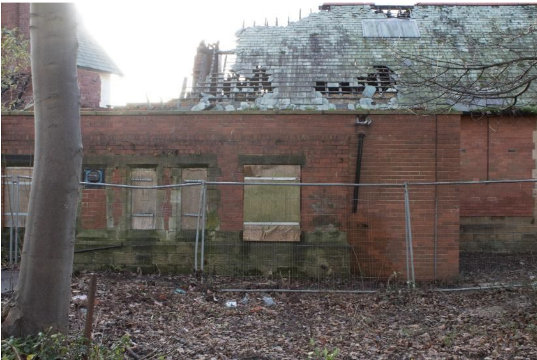
Photo 54: North elevation of west wing wash block (1796_054.TIF)
