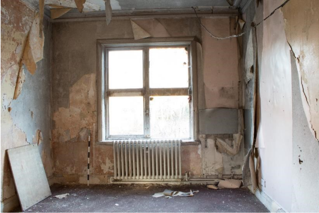
Photo 307: Room 46, facing north-east (1796_307.TIF)
