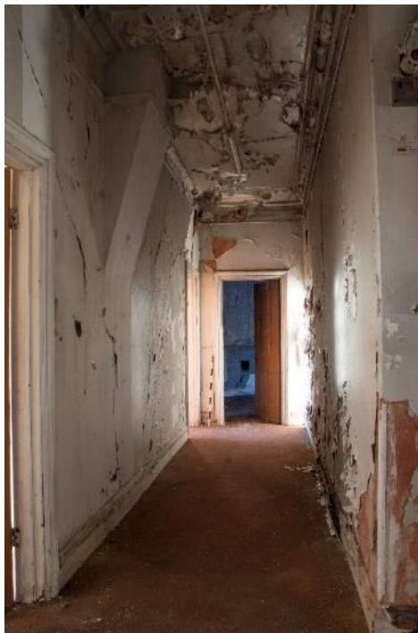
Photo 296: First floor hallway, facing north-west (1796_296.TIF)
