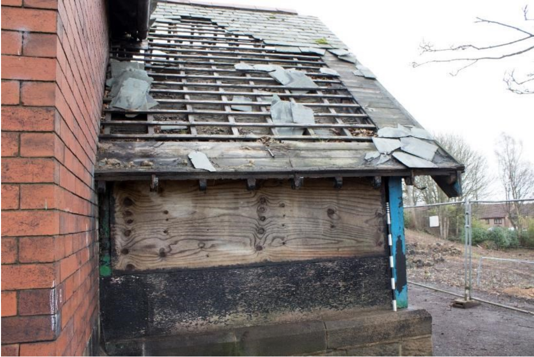
Photo 11: Side elevation of west veranda, facing east (1796_011.TIF)
