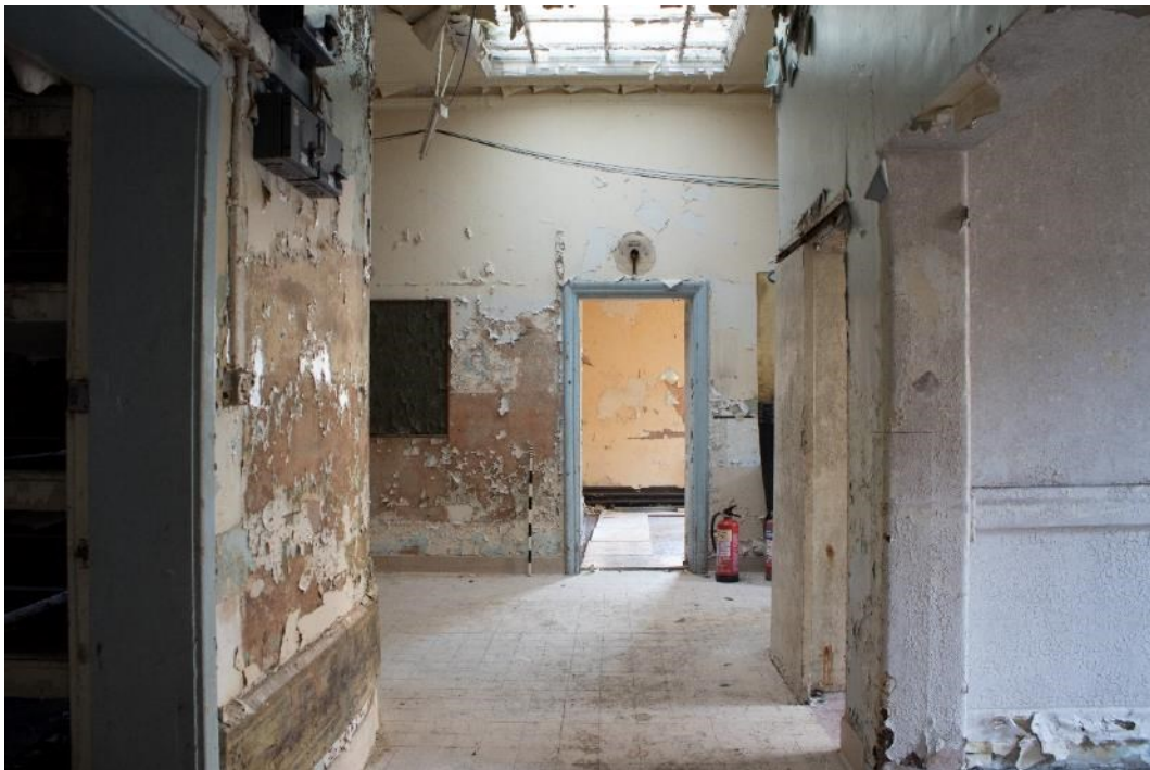
Photo 142: Kitchen corridor, facing north-west (1796_142.TIF)
