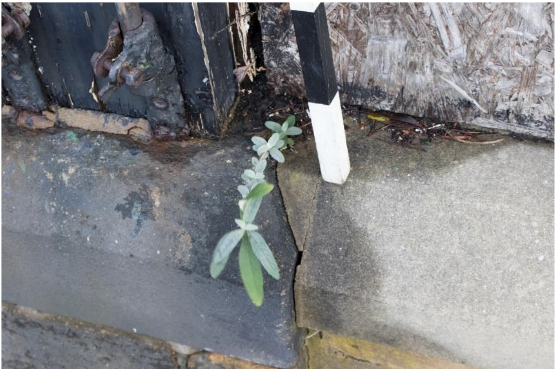
Photo 40: Detail of join on veranda plinth stonework, facing north-east (1796_040.TIF)
