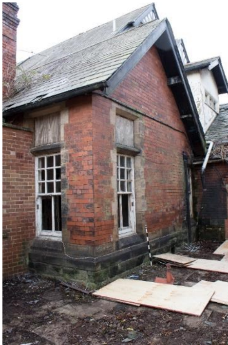
Photo 102: Exterior of room 13, facing west (1796_102.TIF)
