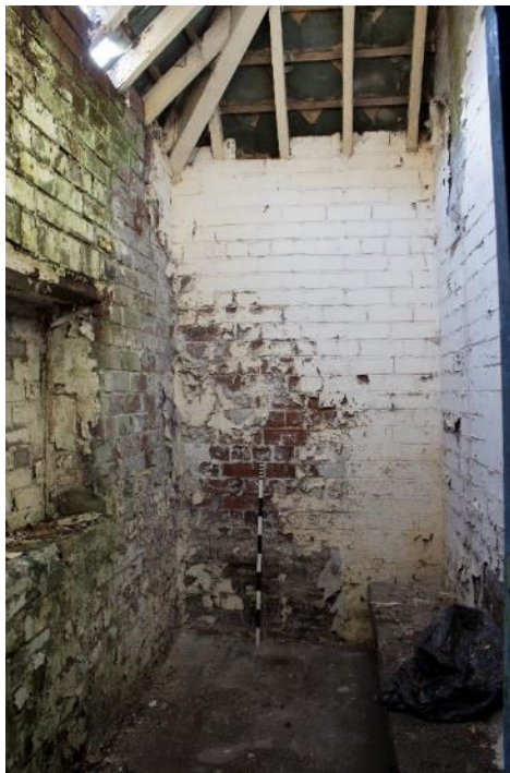
Photo 180: Room 24. Facing south-west (1796_180.TIF)
