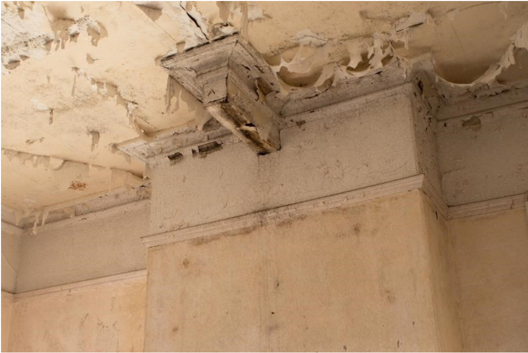
Photo 289: Projecting beam above fireplace in room 44, facing north-east (1796_289.TIF)
