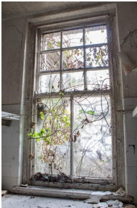
Photo 194: Room 20 window, facing south-east (1796_194.TIF)
