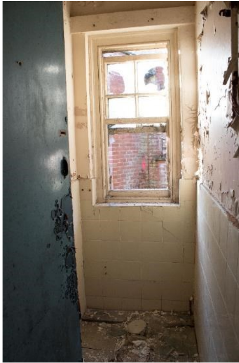
Photo 175: Service range W.C (22) facing south-west (1796_175.TIF)
