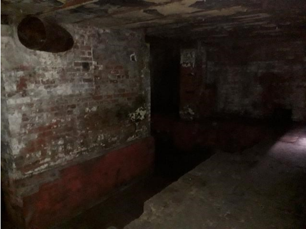
Photo 333: East room in basement (64) facing east (1796_333.TIF)
