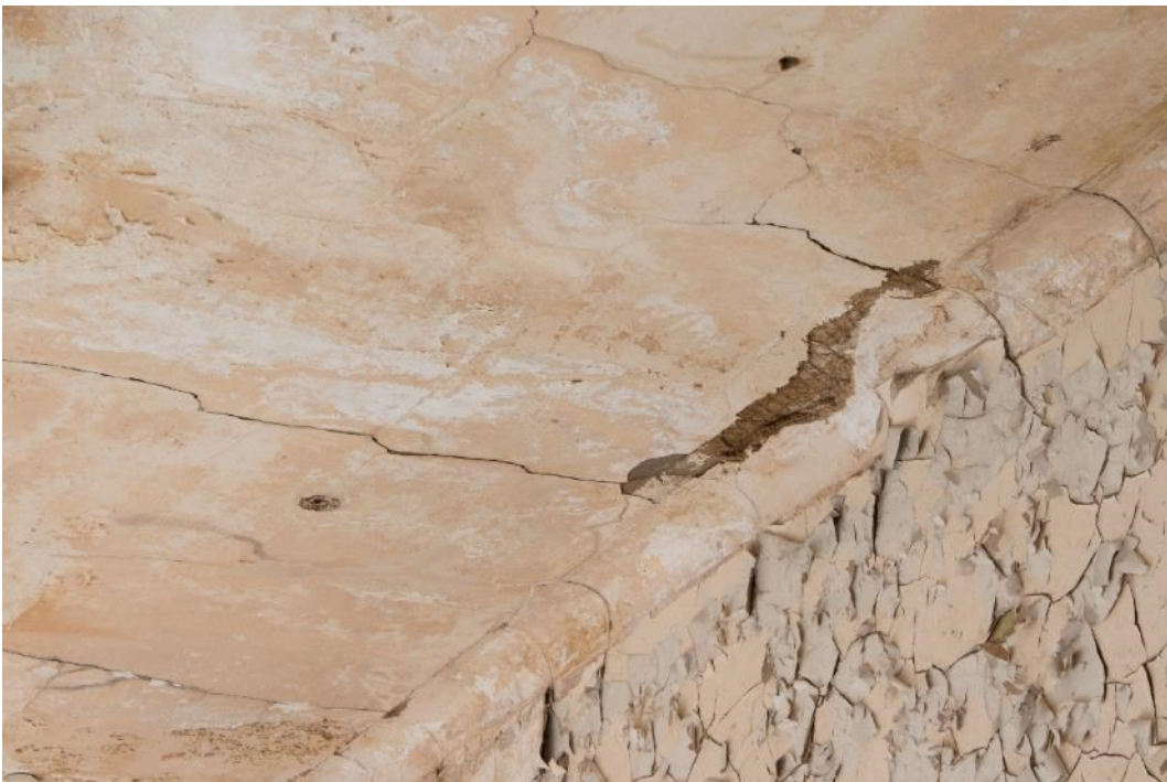
Photo 278: Coving to west ward ceiling, facing south-west (1796_278.TIF)
