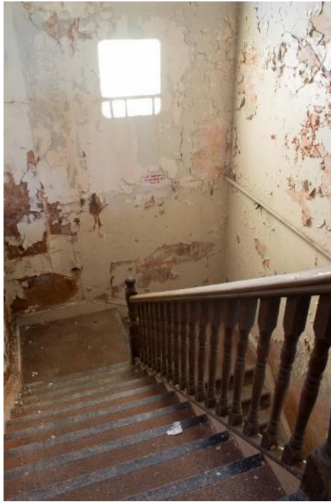
Photo 299: Stairs from ground to first floor, facing north-east (1796_299.TIF)
