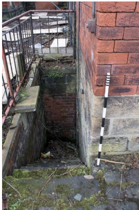
Photo 88: External stairs to basement, facing north-west (1796_088.TIF)
