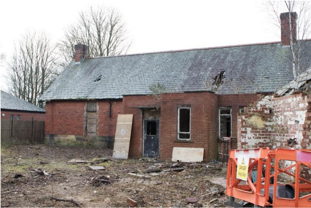
Photo 85: North elevation of east wing and wash block (1796_085.TIF)
