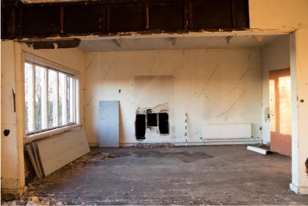
Photo 319: Room 47, facing north-west (1796_319.TIF)
