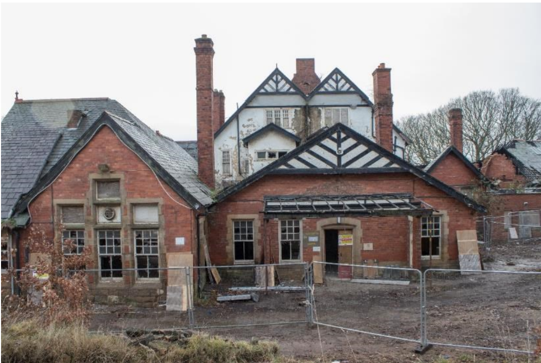
Photo 68: North elevation of kitchen, north block and central block (1796_068.TIF)
