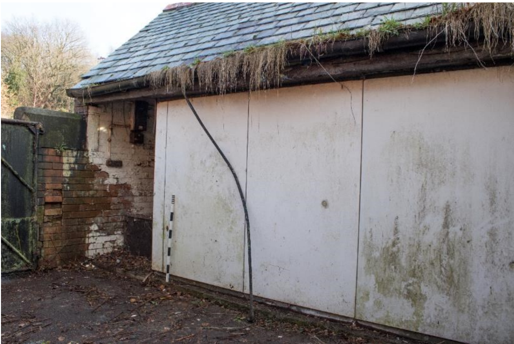
Photo 188: Kitchen courtyard, facing east (1796_188.TIF)
