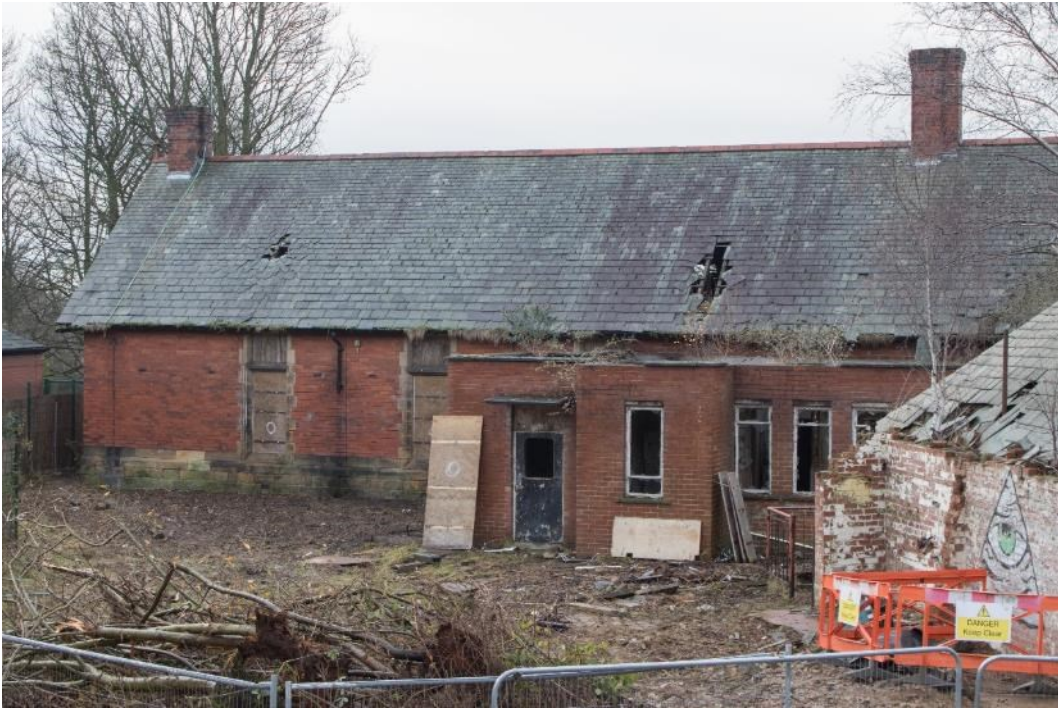
Photo 63: North elevation of east wing and wash block (1796_063.TIF)
