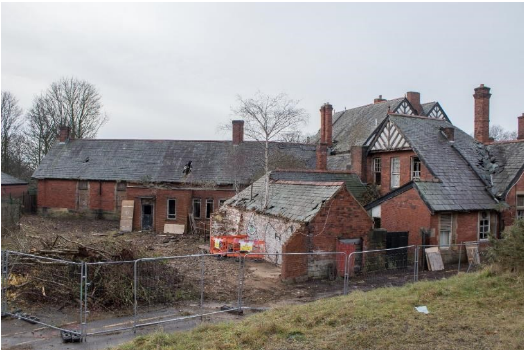
Photo 62: Rear of east wing and service range, facing south-west (1796_062.TIF)
