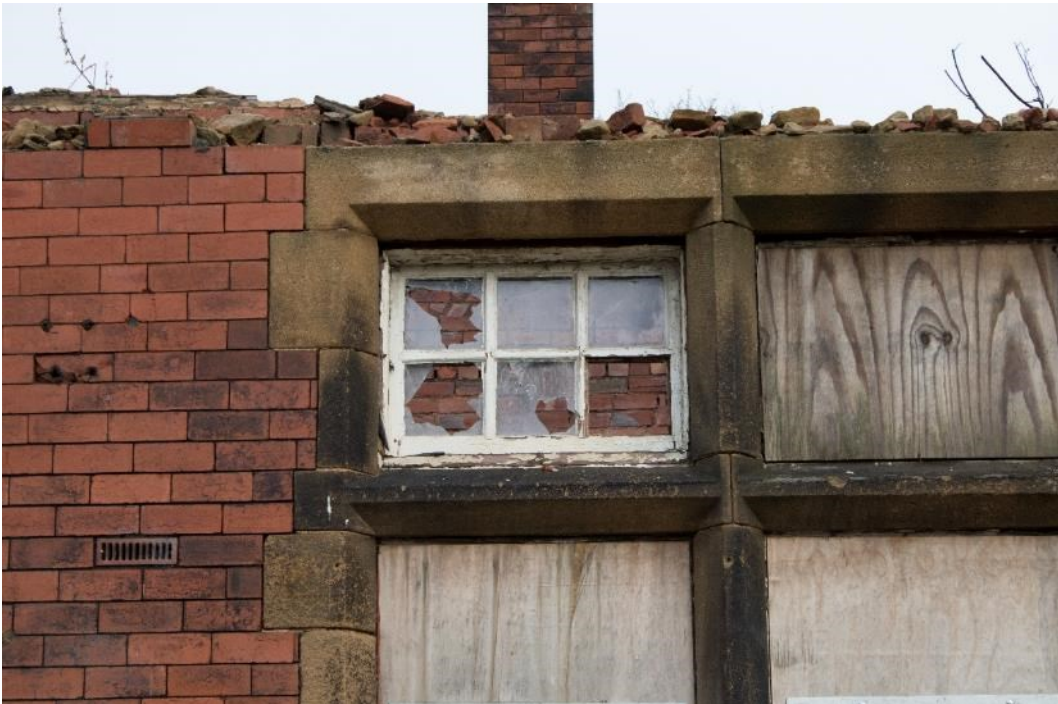
Photo 20: Detail of top-light, facing north-east (1796_020.TIF)
