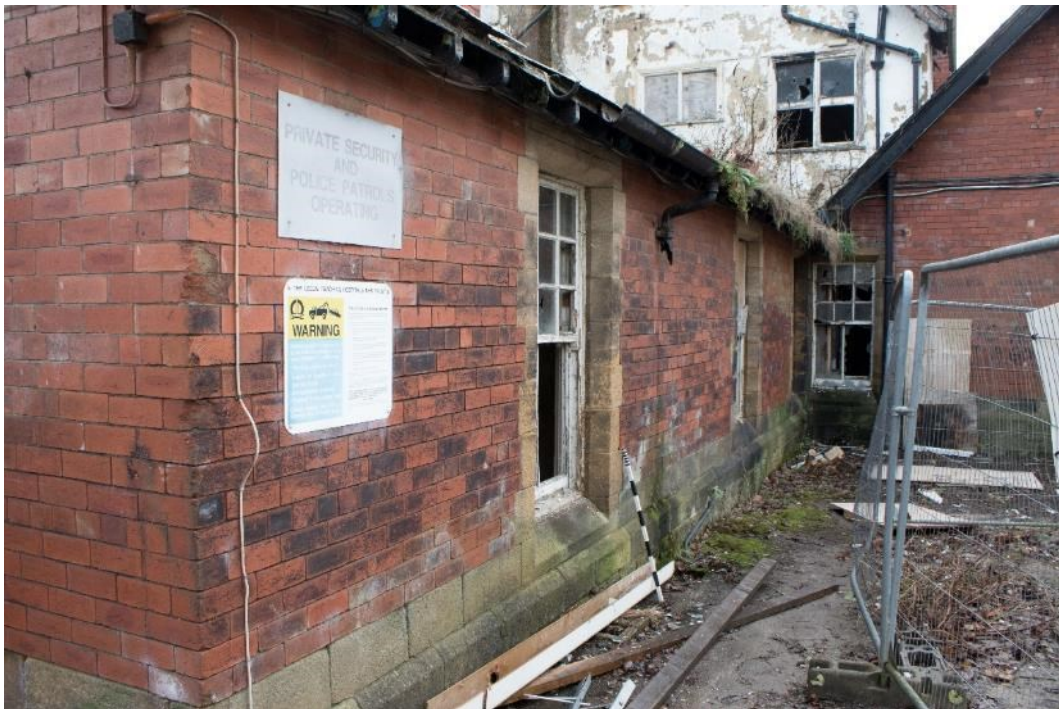
Photo 94: North elevation of central block (12 & 13), facing west (1796_094.TIF)
