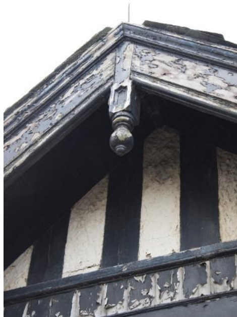
Photo 12: Gable of west veranda (1796_012.TIF)
