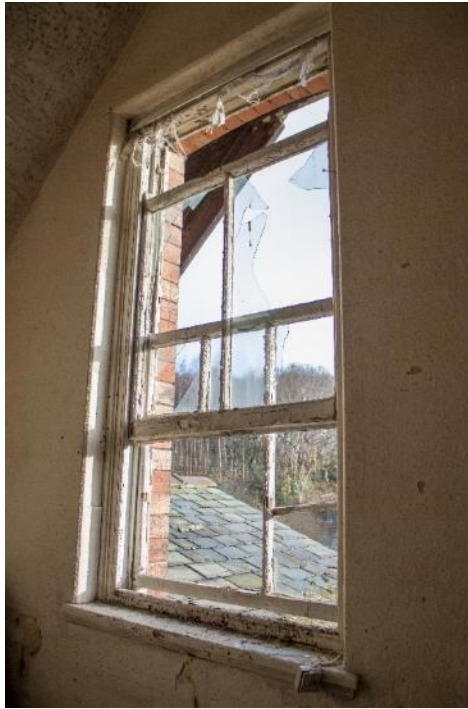
Photo 201: Room 54 window, facing east (1796_201.TIF)
