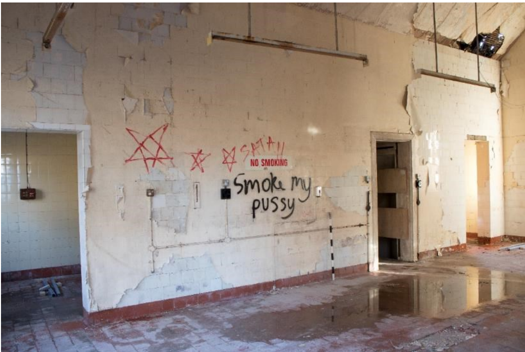
Photo 156: Kitchen east wall, facing south (1796_156.TIF)
