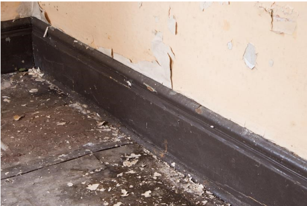
Photo 120: Room 2 skirting board, facing west (1796_120.TIF)
