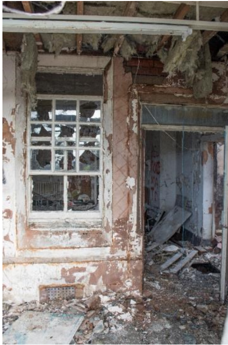
Photo 17: Interior of west veranda, facing north (1796_017.TIF)
