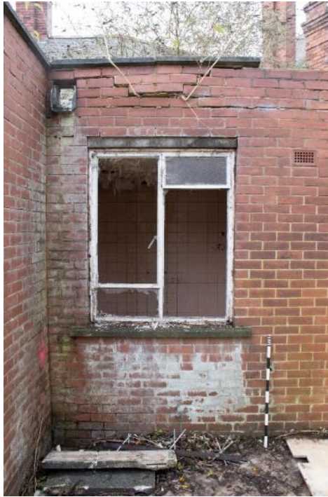
Photo 105: Window to east wing wash block, facing west (1796_105.TIF)
