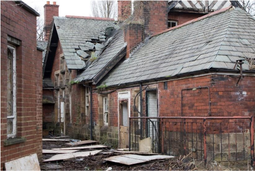
Photo 87: South elevation of the service range, facing north (1796_087.TIF)
