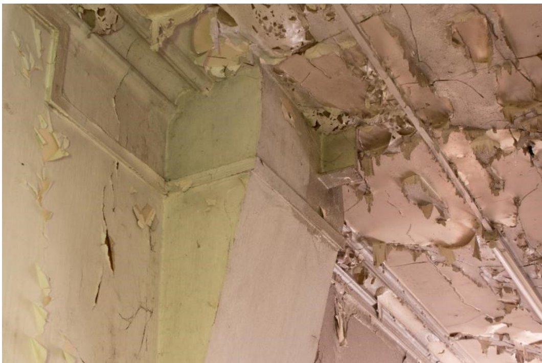
Photo 298: Projecting wall feature in first floor hallway, facing west (1796_298.TIF)
