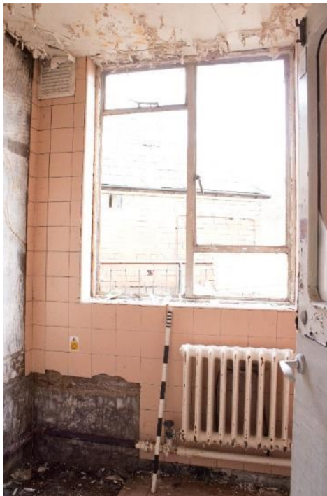
Photo 220: Room 33, facing east (1796_220.TIF)
