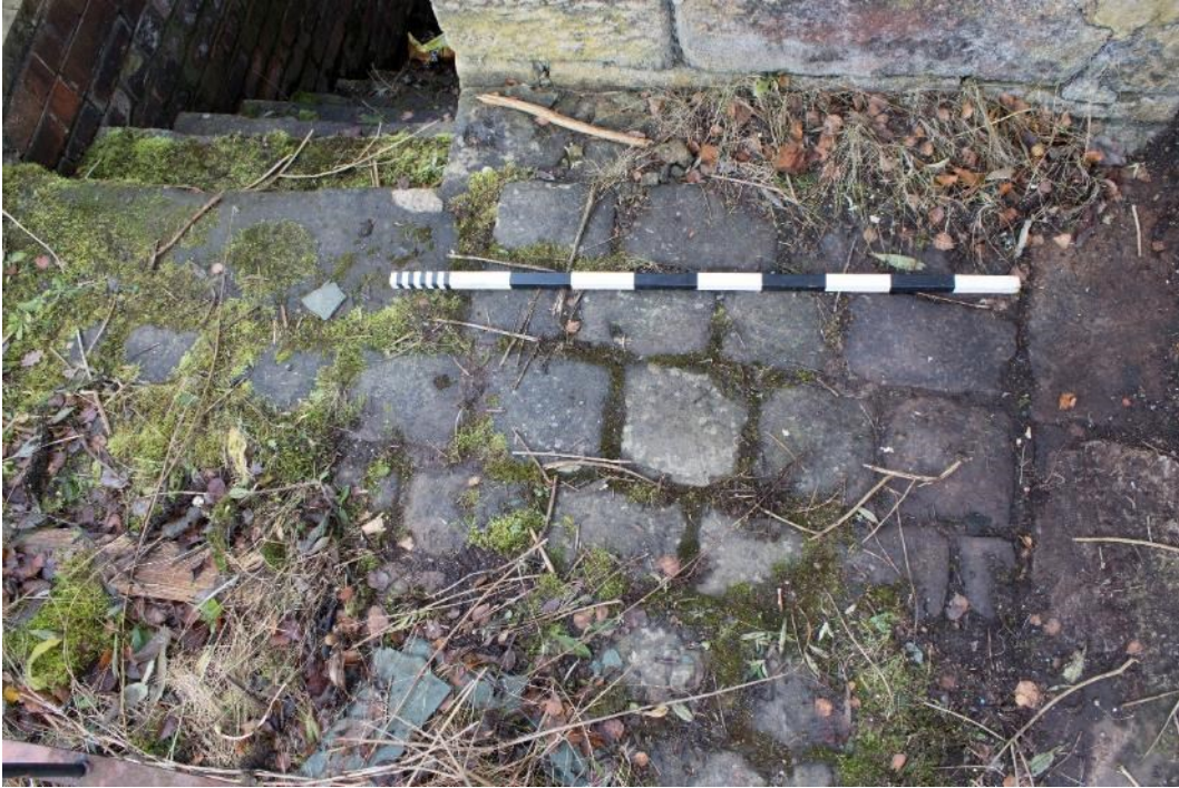
Photo 89: Paving sets to the east of the service range, facing north-west (1796_089.TIF)
