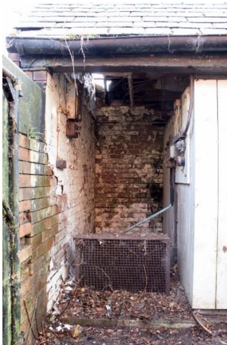
Photo 190: Space behind refridgerator, facing south-east (1796_190.TIF)
