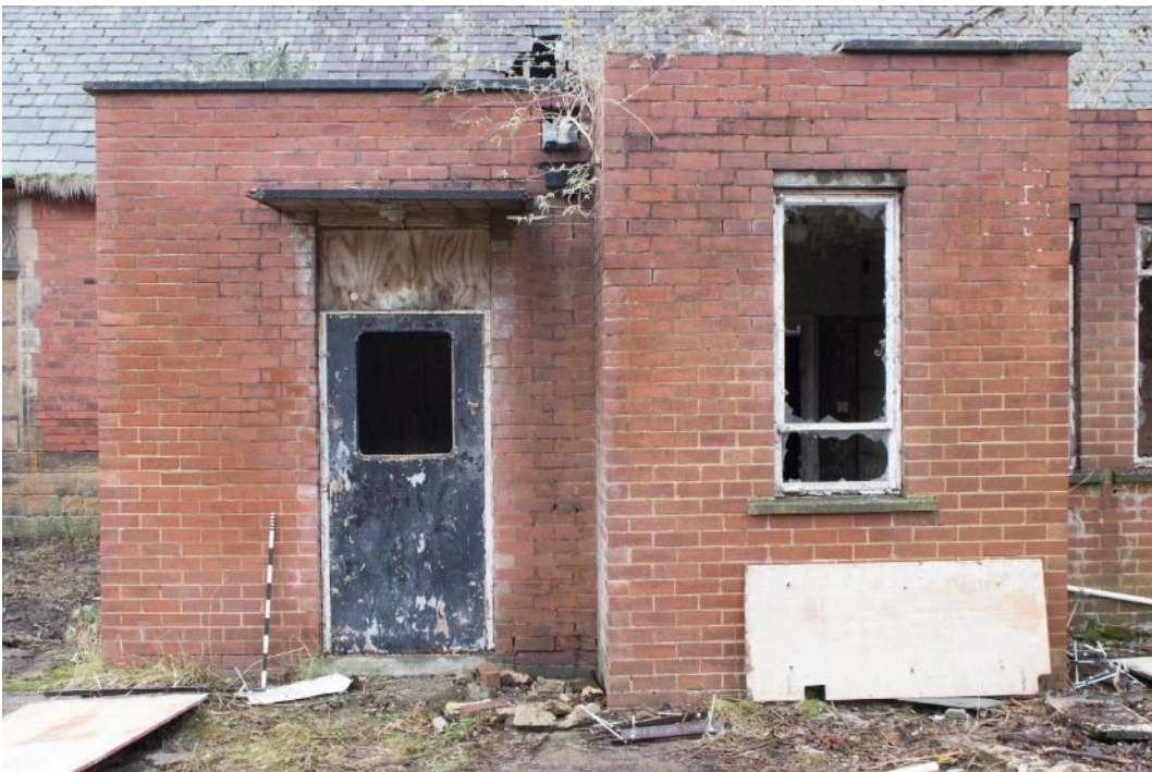
Photo 108: Entrance and window to east wing was block, facing west (1796_108.TIF)
