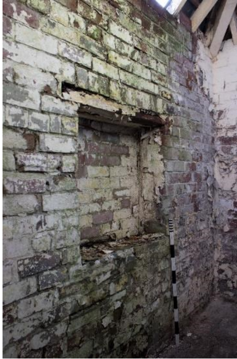
Photo 181: Blocked window in room 24, facing south (1796_181.TIF)
