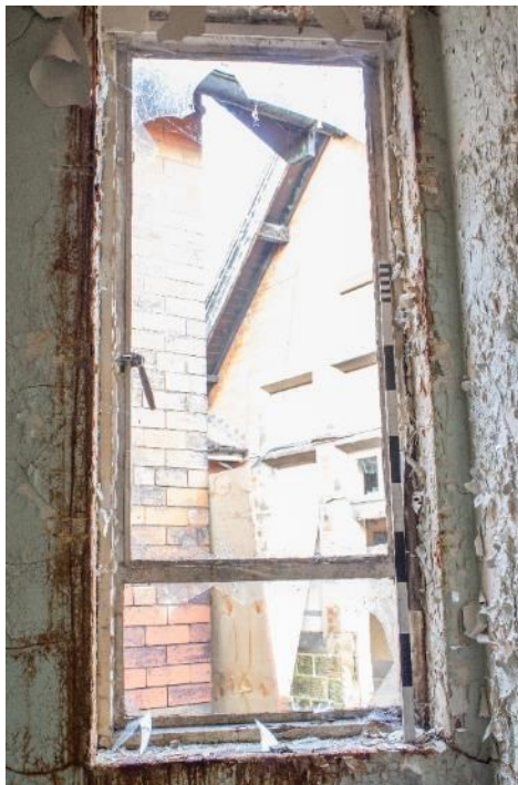
Photo 208: Window to room 36, facing north (1796_208.TIF)
