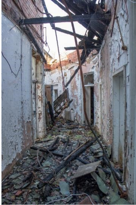
Photo 279: West end of east-west corridor, facing north-west (1796_279.TIF)
