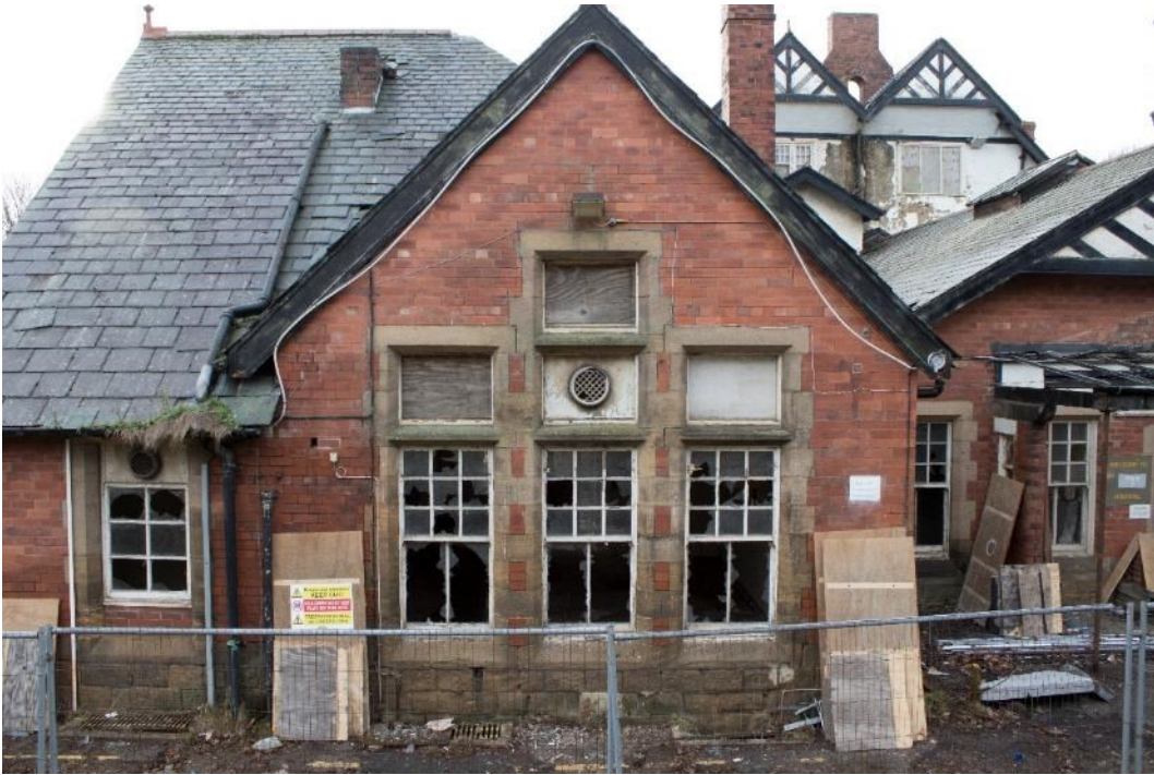
Photo 67: North elevation of kitchen (1796_067.TIF)
