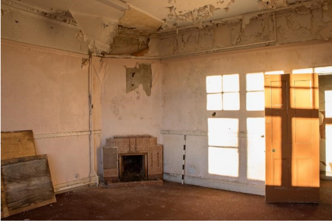
Photo 301: Room 45, facing north (1796_301.TIF)
