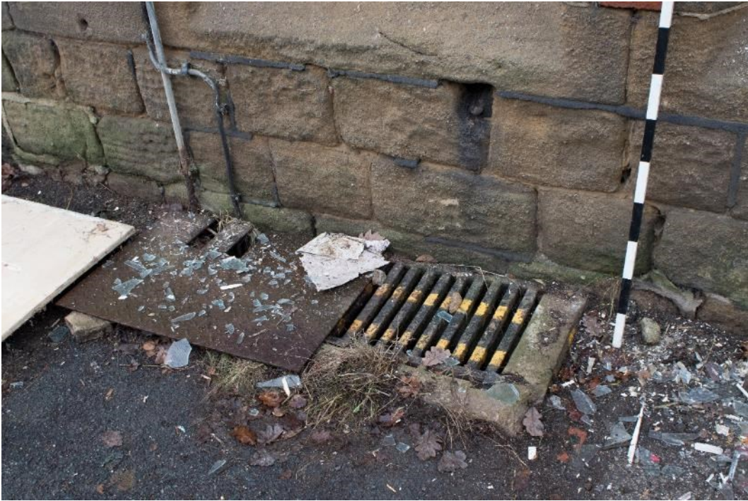
Photo 77: Light/ventilation well to basement, facing south-west (1796_077.TIF)
