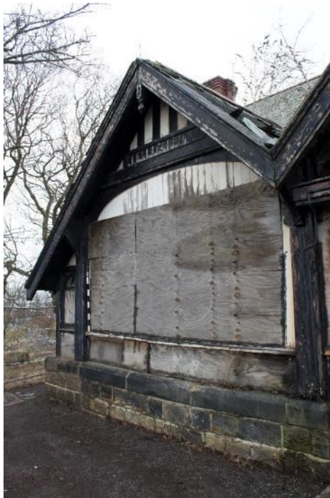
Photo 8: West veranda, facing west (1796_008.TIF)
