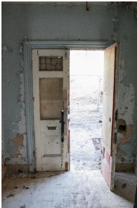
Photo 280: Main door to north block, facing north-east (1796_280.TIF)
