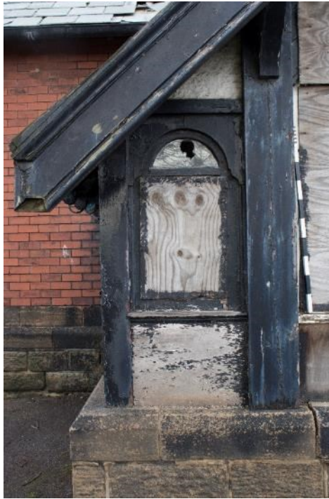
Photo 9: Detail of west veranda, facing north (1796_009.TIF)
