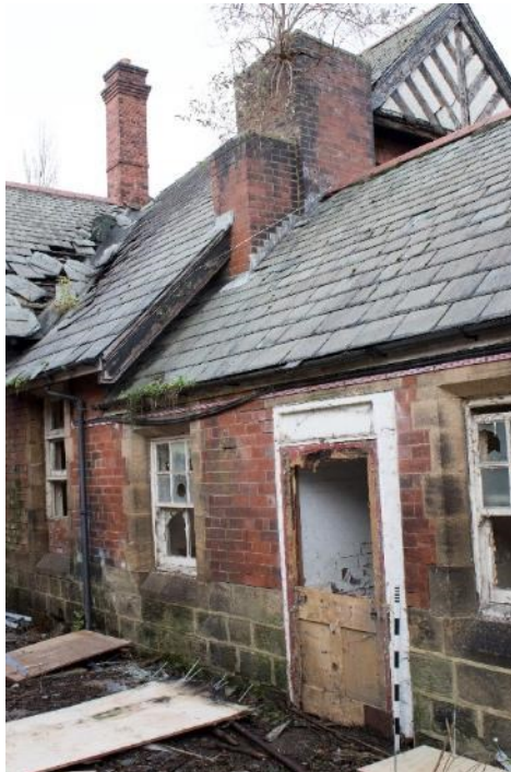
Photo 90: South elevation of the service range (1796_090.TIF)
