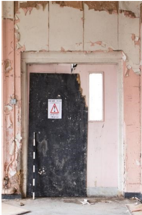
Photo 232: Door to east dayroom (15) from room 55, facing north-west (1796_232.TIF)
