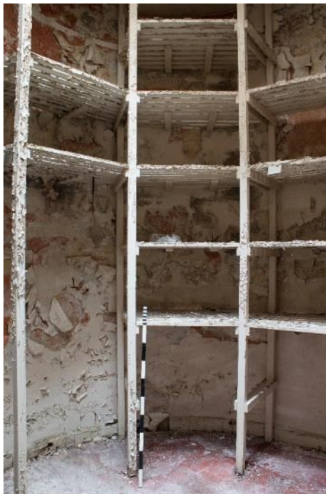
Photo 126: Room 10, facing south-west (1796_126.TIF)
