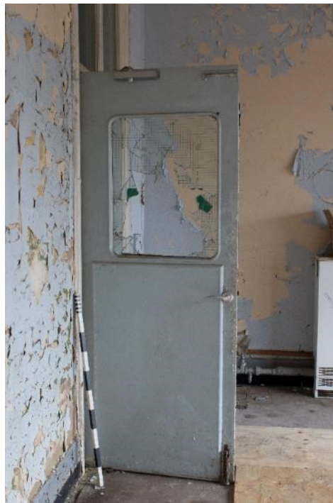
Photo 258: Door to room 38, facing south-east (1796_257.TIF)
