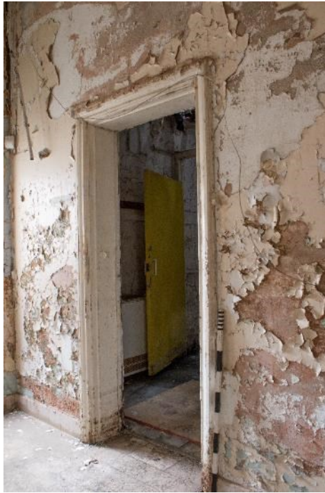
Photo 247: Door to room 11, facing north (1796_247.TIF)
