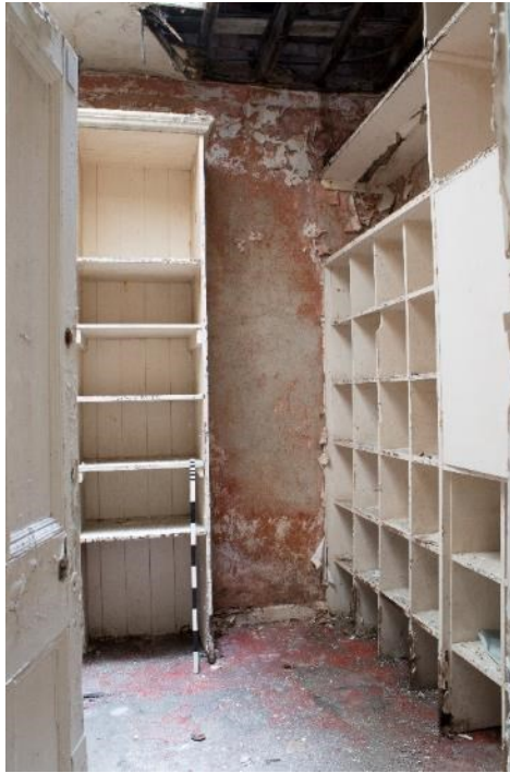
Photo 125: Room 10, facing north-west (1796_125.TIF)
