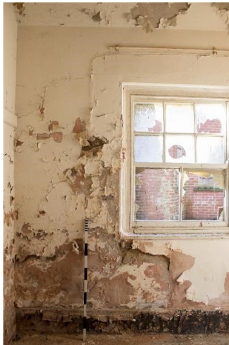
Photo 170: Room 21, facing south-west (1796_170.TIF)
