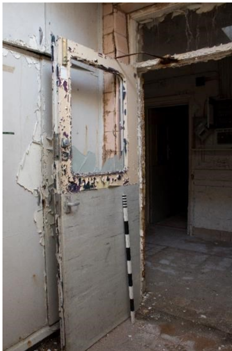
Photo 210: Door to room 35, facing south-west (1796_210.TIF)
