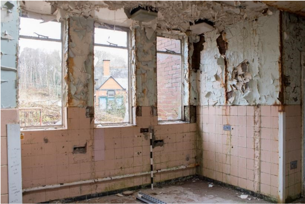
Photo 217: Location of former toilet stalls in room 31, facing south-east (1796_2107TIF)
