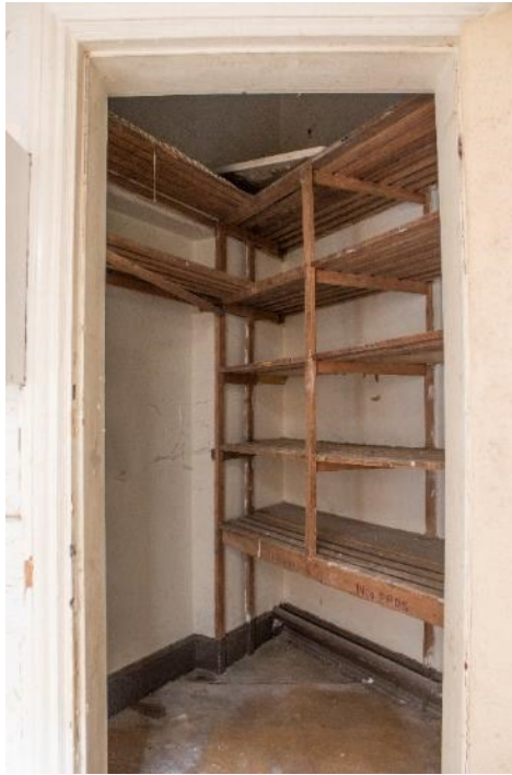
Photo 265: Room 25, facing west (1796_265.TIF)
