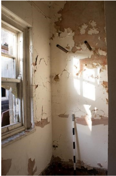
Photo 171: Room 21, facing west (1796_171.TIF)
