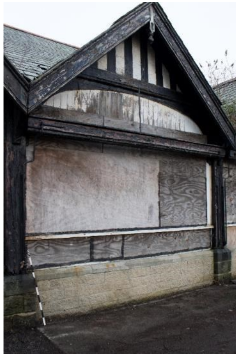
Photo 14: Bay of west veranda, facing north (1796_014.TIF)
