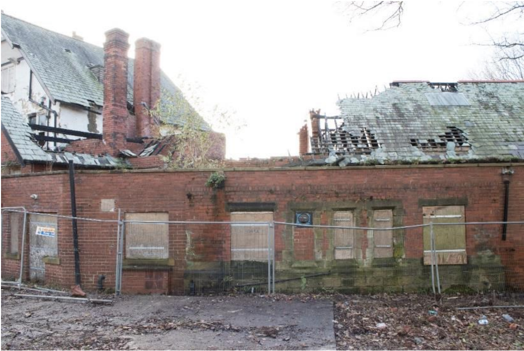
Photo 55: North elevation of west wing wash block (1796_055.TIF)
