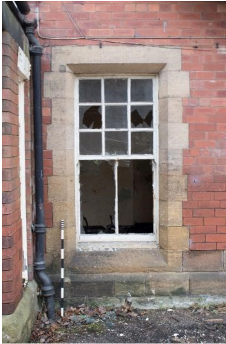
Photo 71: Typical 9x2 sash window, facing south-west (1796_071.TIF)
