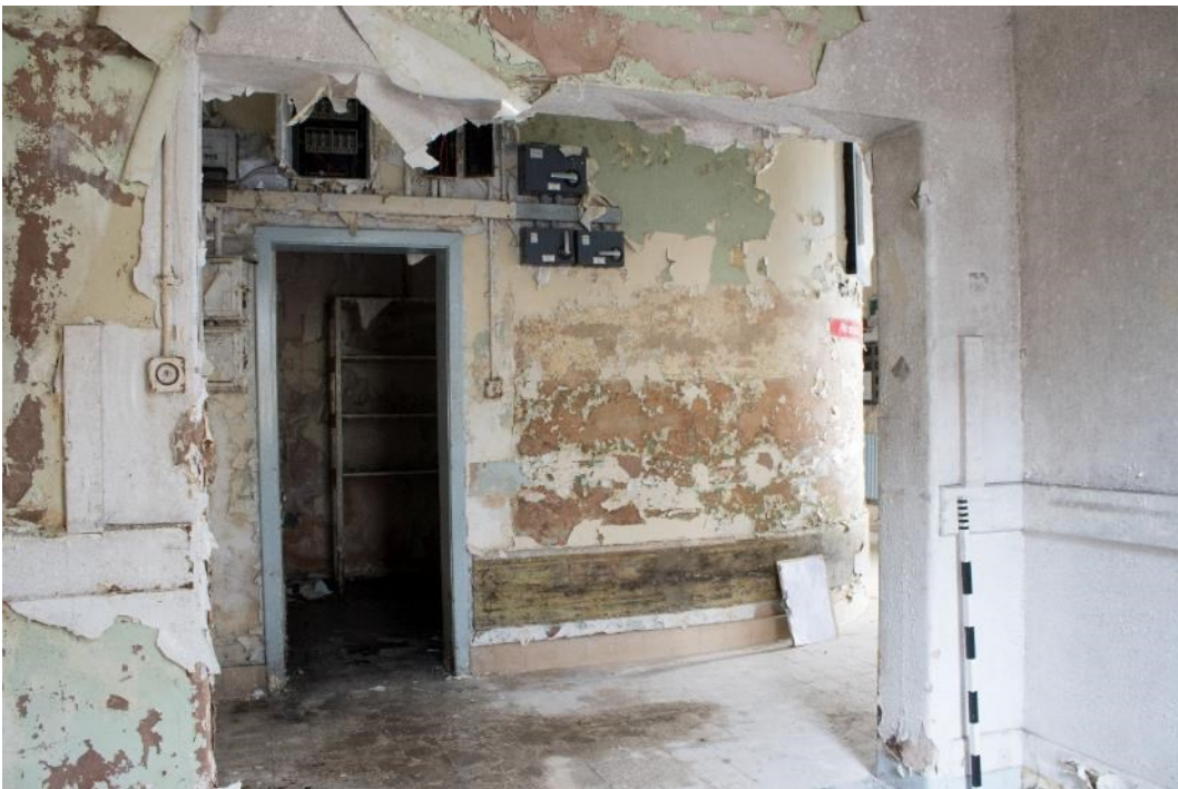
Photo 134: Room 6, facing south-west (1796_13740.TIF)
