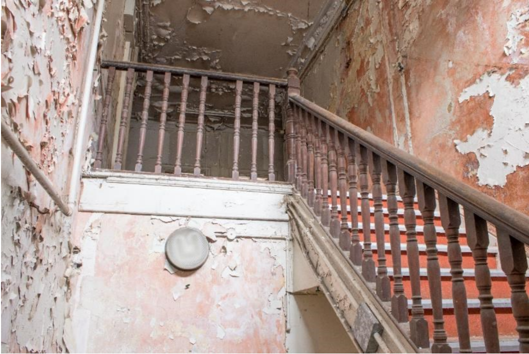
Photo 315: Stairs from ground to first floor, facing south-west (1796_315.TIF)
