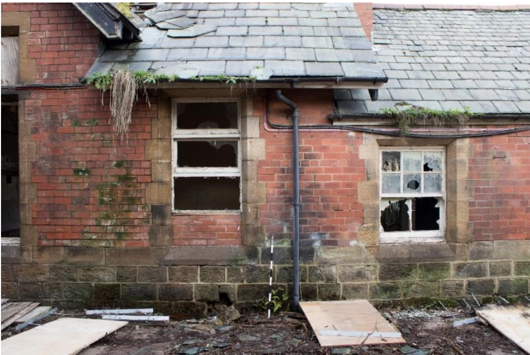
Photo 92: South elevation of the service range (1796_092.TIF)
