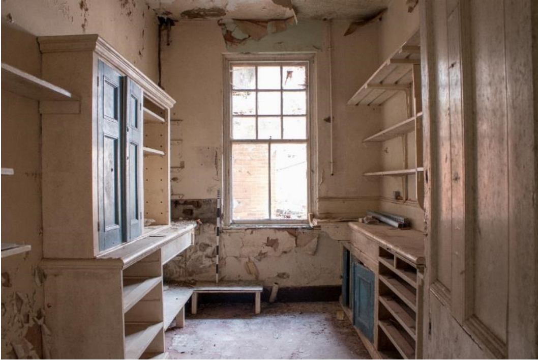
Photo 121: Room 4, facing north-west (1796_121.TIF)
