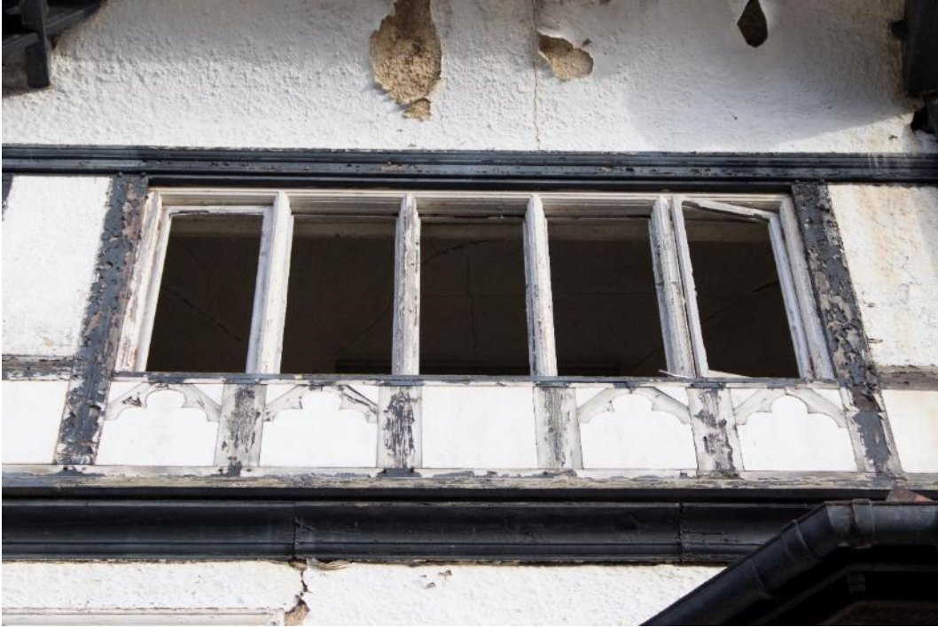
Photo 33: Window to second floor, facing north-east (1796_033.TIF)
