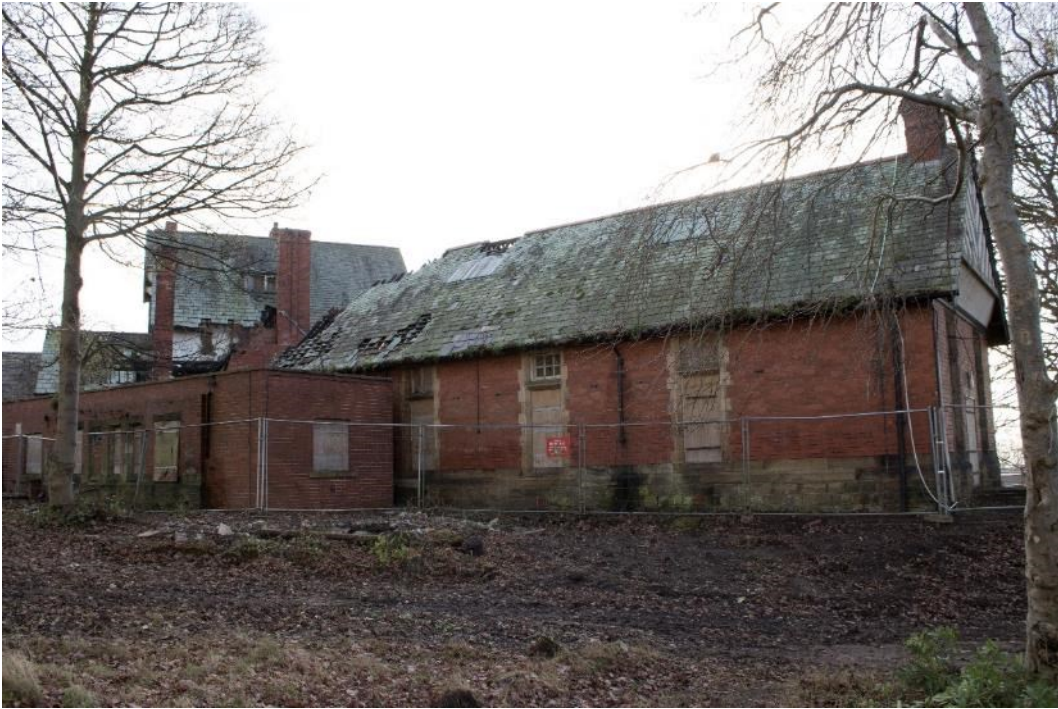
Photo 51: North elevation of west wing, facing south (1796_051.TIF)
