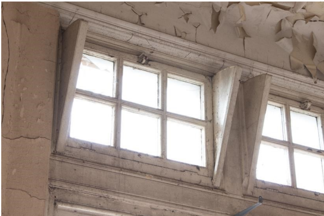
Photo 234: East dayroom toplights, facing west (1796_234.TIF)
