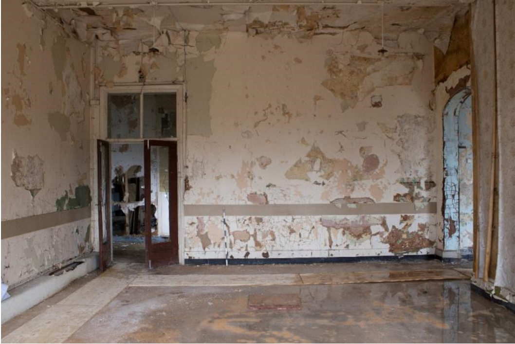
Photo 249: West dayroom, facing north-east (1796_249.TIF)
