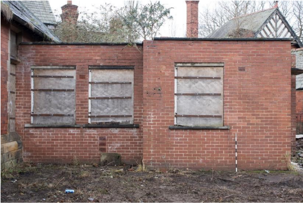
Photo 109: East elevation of east wing wash block (1796_109.TIF)
