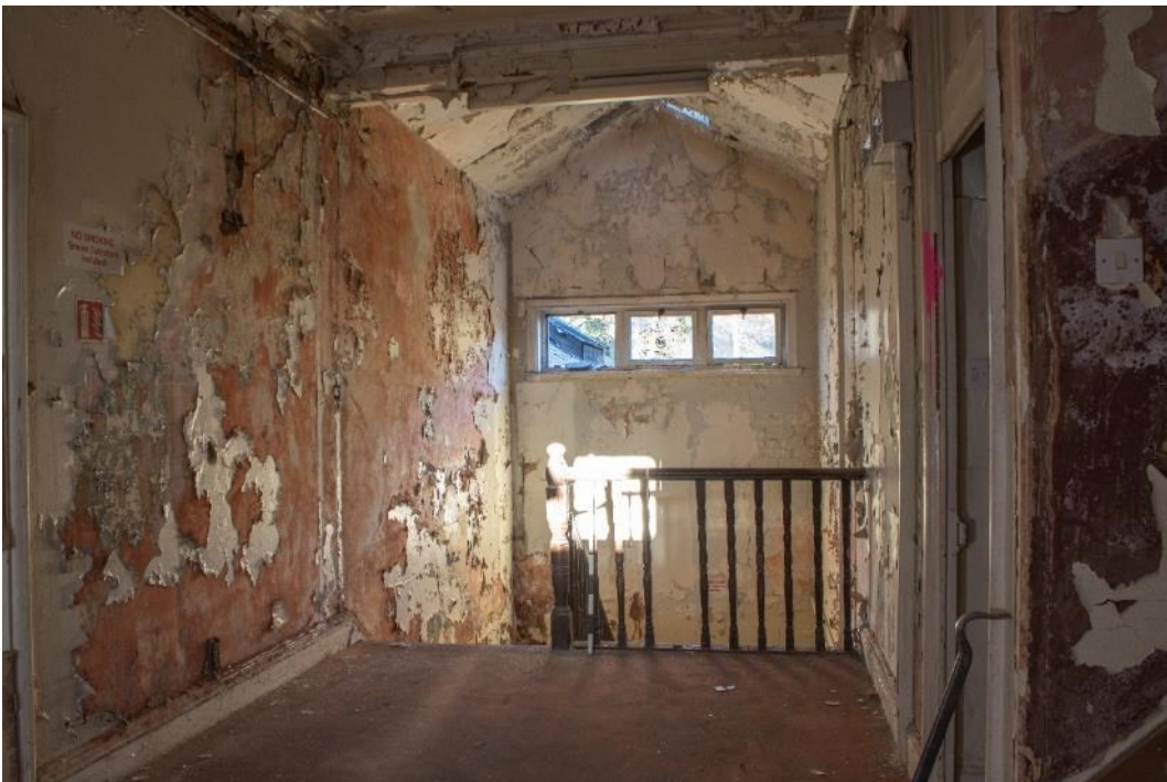
Photo 292: First floor stair landing, facing north-east (1796_292.TIF)
