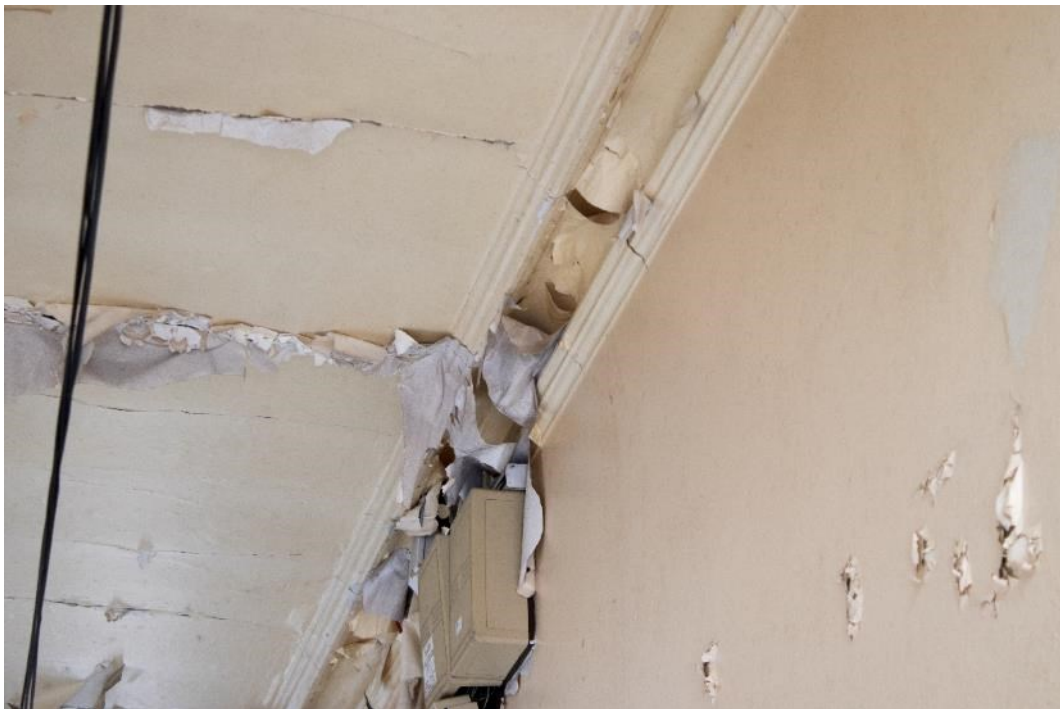
Photo 150: North block corridor cornice, facing west (1796_150.TIF)
