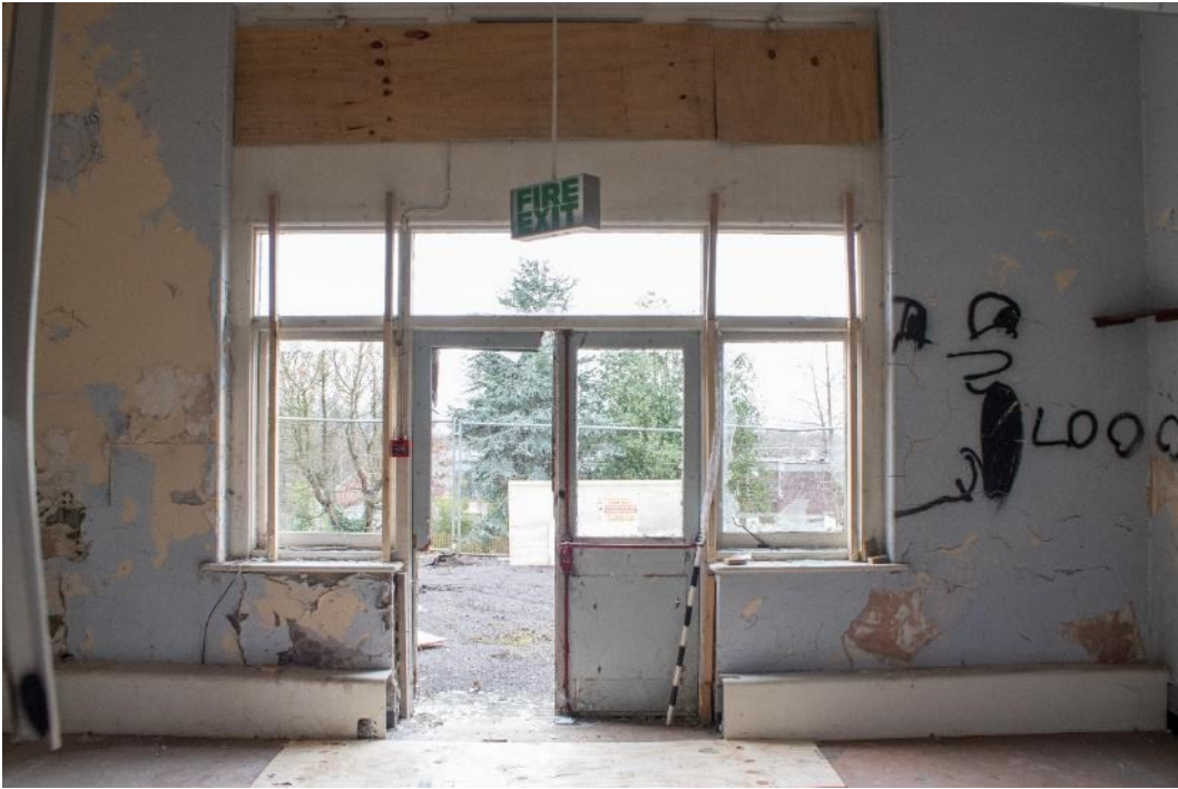
Photo 257: Windows and doors to room 38, facing south-west (1796_257.TIF)
