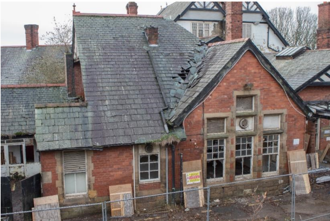
Photo 66: North elevation of kitchen (1796_066.TIF)
