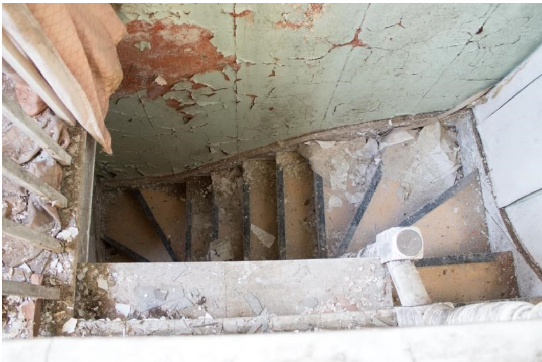
Photo 198: Stairs to first floor of service range, facing south-west (1796_198.TIF)
