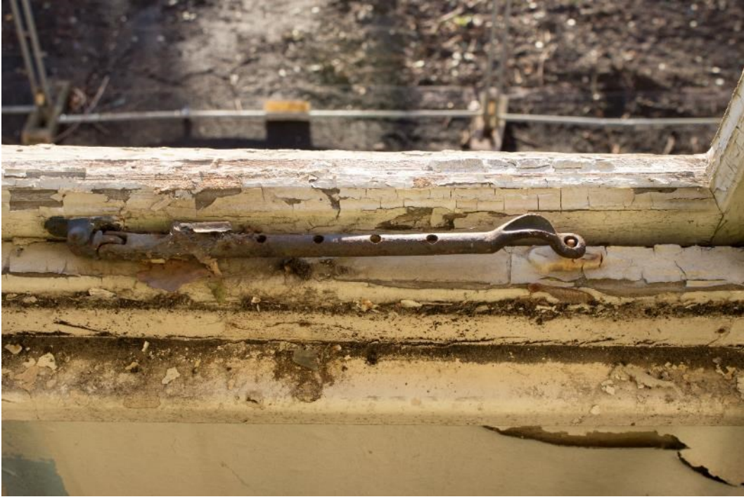
Photo 291: Window stay in room 44, facing south-west (1796_291.TIF)
