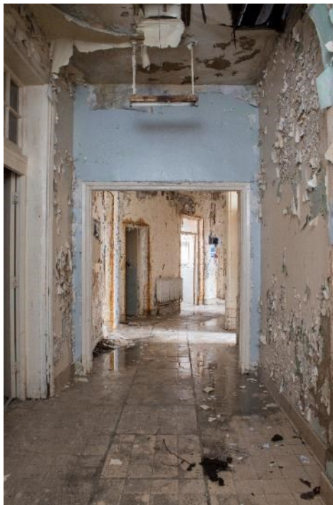
Photo 260: East-west corridor, facing south-east (1796_260.TIF)
