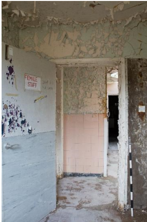
Photo 224: Room 30, facing west (1796_224.TIF)
