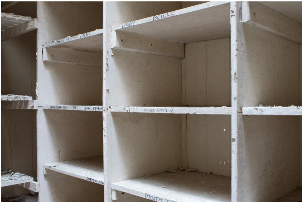
Photo 128: Room 10 shelving, facing west (1796_128.TIF)
