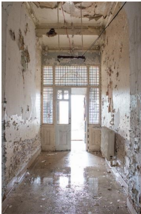
Photo 236: South entrance corridor, facing south-west (1796_236.TIF)
