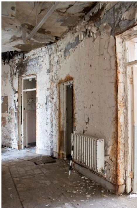
Photo 264: North side of east end of eas-west corridor, facing north (1796_264.TIF)
