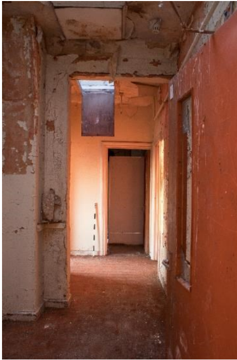
Photo 327: Second floor hallway, facing north-west (1796_327.TIF)
