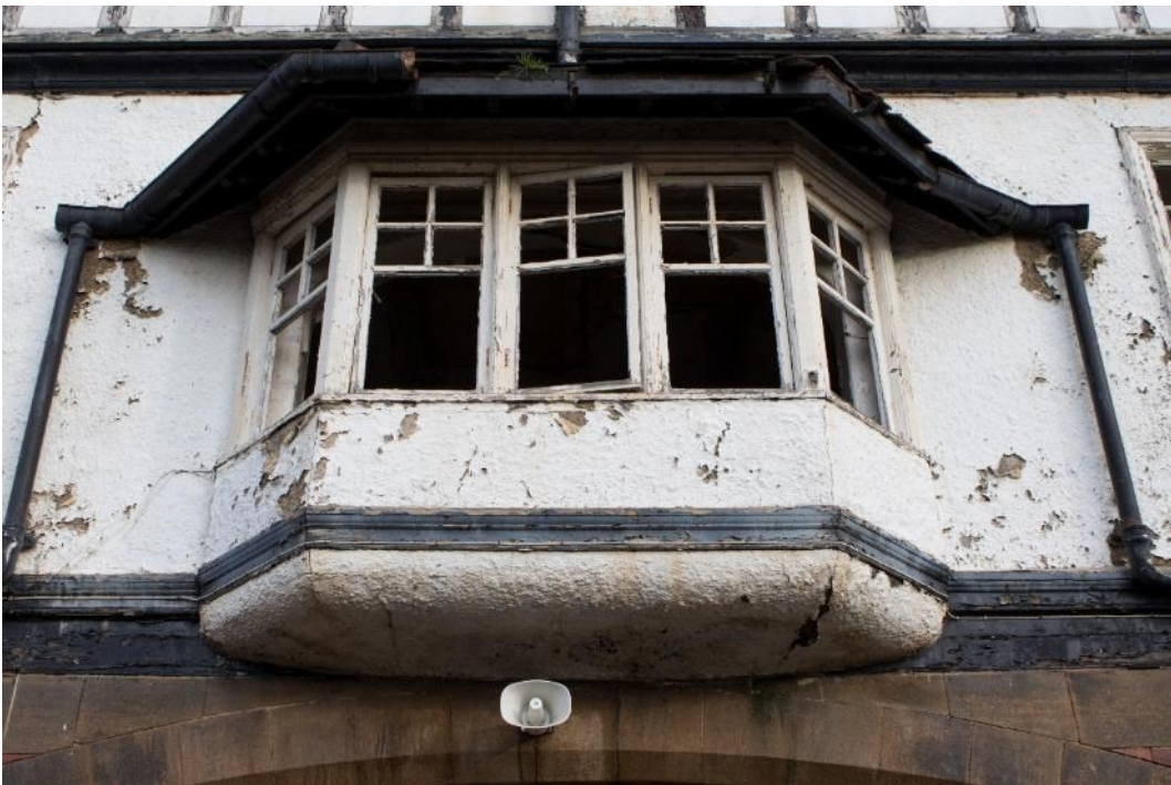
Photo 28: Oriel window to first floor central block, facing north-east (1796_028.TIF)
