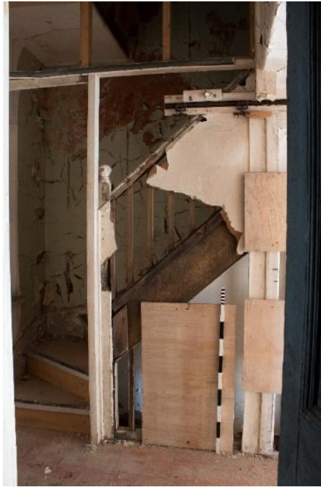
Photo 169: Stairs to first floor of service range, facing south-west (1796_169.TIF)
