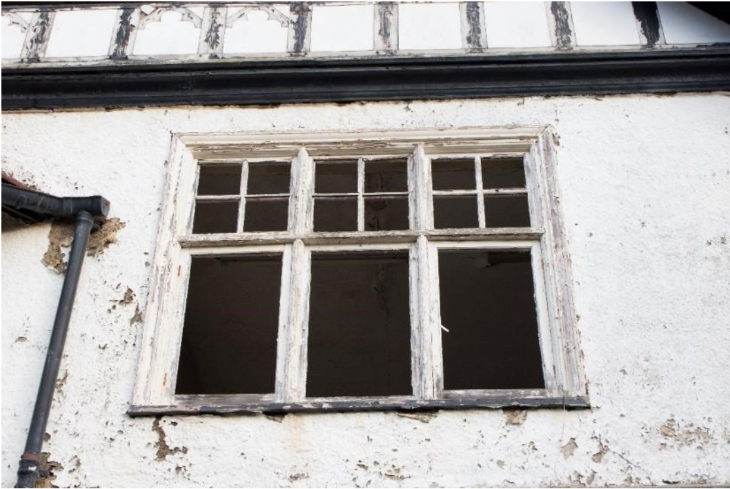
Photo 31: Window to south-east first floor room (43), facing north-east (1796_031.TIF)
