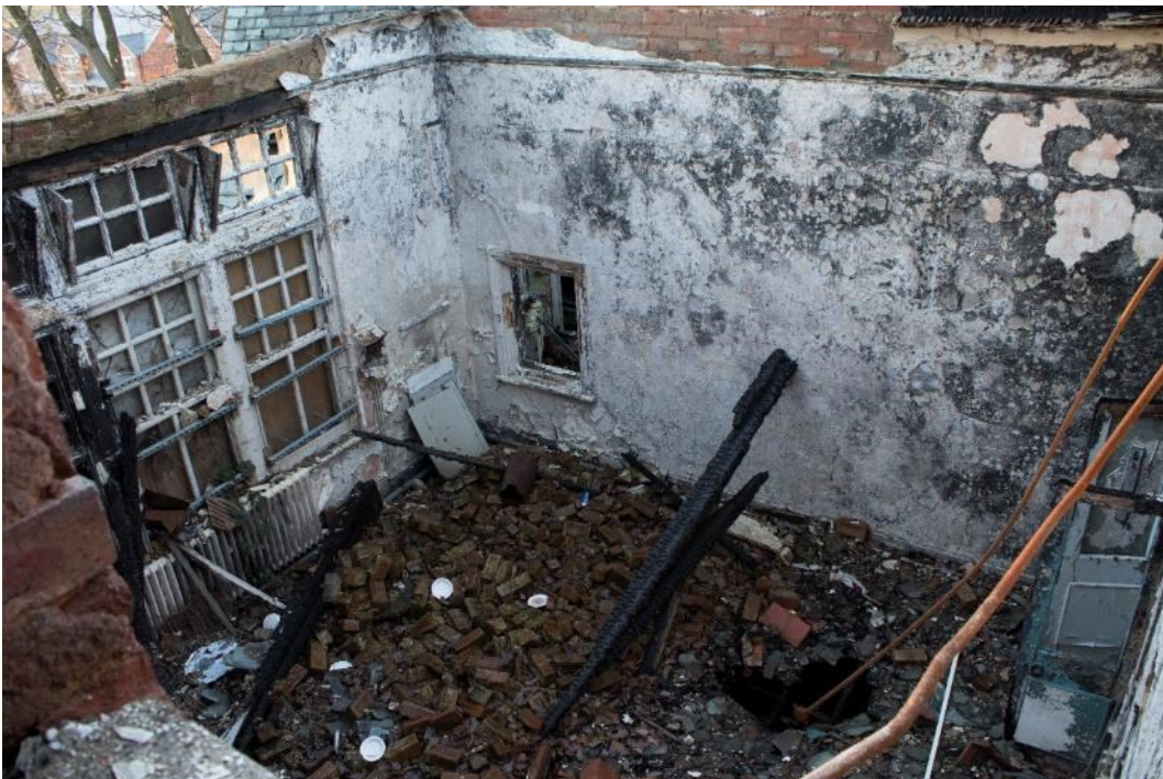
Photo 312: Room 55 viewed from roof access hatch in room 46, facing west (1796_312.TIF)
