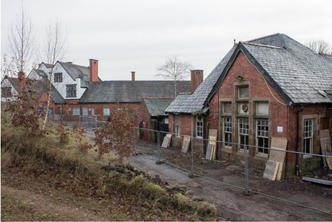
Photo 69: Service range and Robert Arthington Hospital, facing south (1796_069.TIF)
