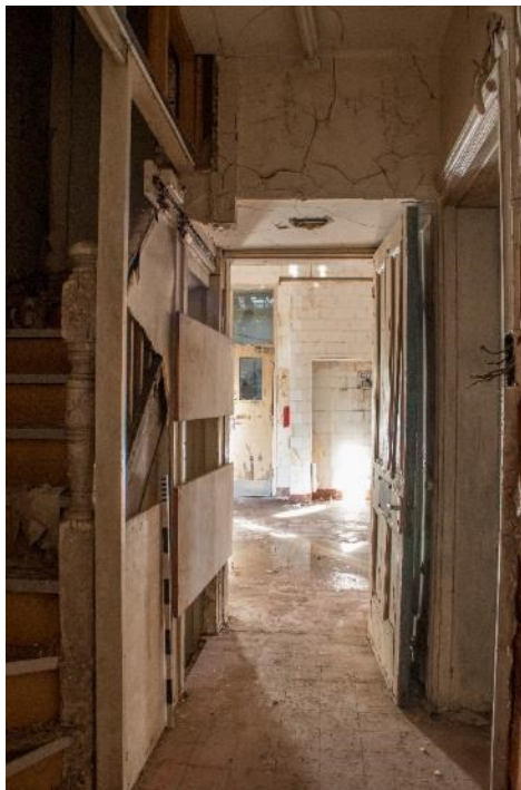
Photo 168: Corrdior from service range to kitchen, facing north-west (1796_168.TIF)
