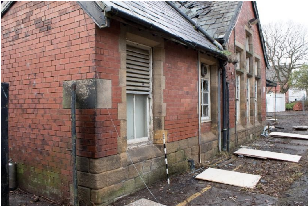
Photo 80: Oblique view of kitchen range, facing west (1796_080.TIF)
