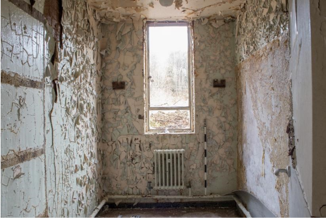
Photo 223: Room 30, facing east (1796_223.TIF)
