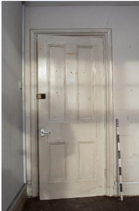
Photo 284: door to room 43, facing north-east (1796_284.TIF)
