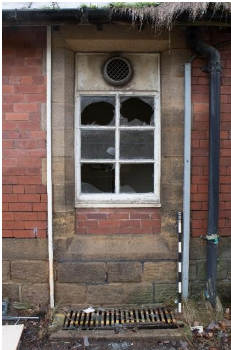
Photo 78: Modified window to kitchen wash room (18) facing south-west (1796_078.TIF)
