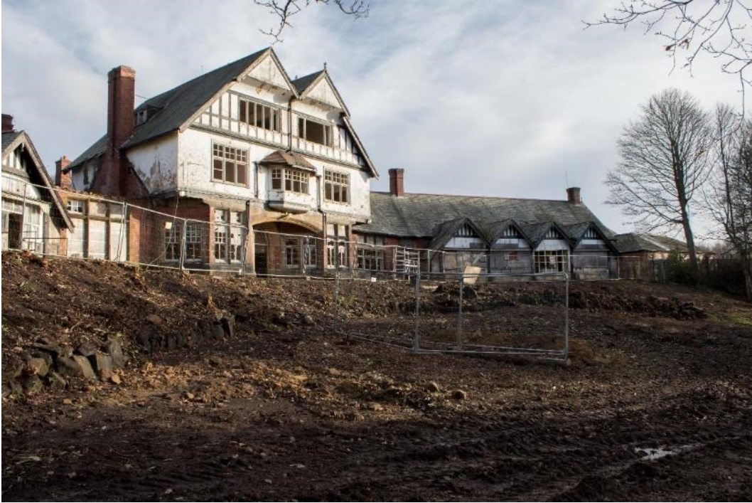
Photo 47: Oblique view of south elevation, facing east (1796_047.TIF)
