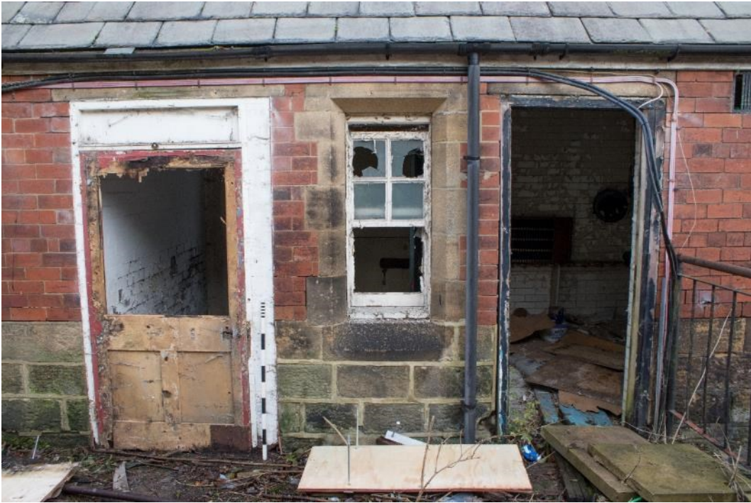
Photo 91: Entrance to service range and mortuary (1796_091.TIF)
