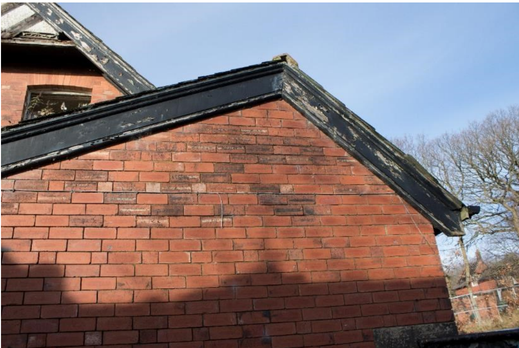
Photo 192: Gable of courtyard elevation of service range, facing north-west (1796_1902.TIF)
