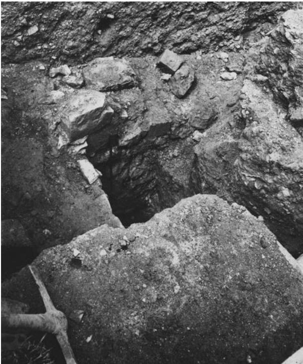
Fig 4.30 South-west corner of nave, looking north west (1926 photograph: © Glastonbury Abbey)
