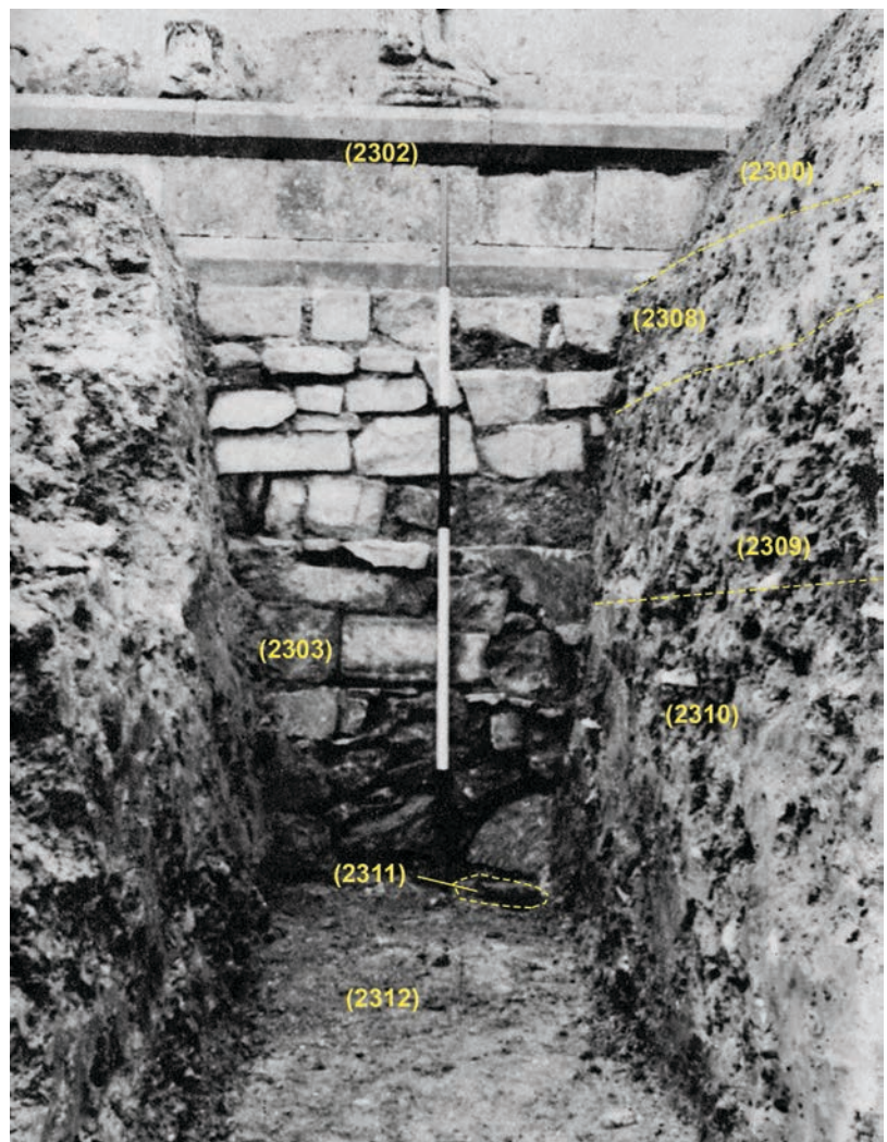
Fig 4.31 Nave and south aisle foundations (possibly two phases), looking south (1955 photograph: © EHA)
