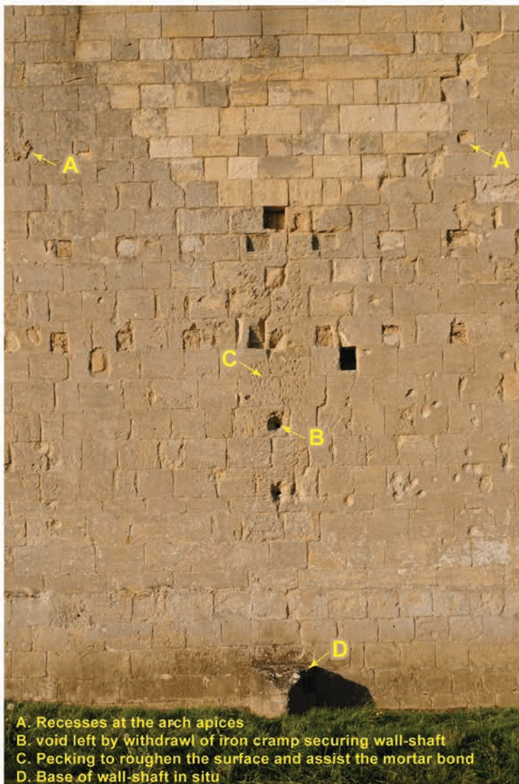
Fig 9.12 Carved stones: (61) '2 inch roll' type mouldings with roof boss (far left), all probably deriving from the vaulting of Abbot Chinnock's cloisters (?after 1407); (62) scars left on the south elevation of the south nave aisle wall from the erection of the fifteenth-century cloister (left). The rectangular recesses in two regular registers belong to the first post-fire cloister. An analogous campaign in Wells Cathedral's west cloister (from the third quarter of the fifteenth century) also pinned the new wall-shafts to the thirteenth-century wall using lead-grouted iron dog-cramps which have subsequently spalled the stone surface exposing their ends (right) (photos: Jerry Sampson)
