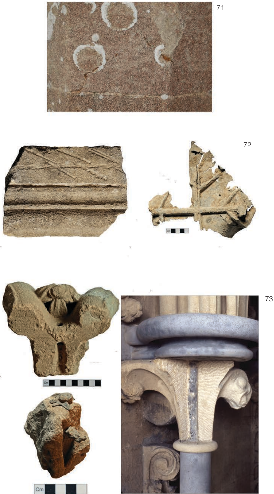
Fig 9.15 Carved stones: (71) irregular break in an ashlar block in bay 2 of the south choir aisle refixed with a brown mastic; (72) S987a (left) with incisions of the bed joint to assist the mortar bond, and L14 (right), a lead pour from a more deeply incised bed joint grouted with lead; (73) S1067 (top left) showing the empty lead grout channel in the soffit and the pouring hole below the floret; S209 (left) a fragment from a pinnacle reinforced across the joint; (right) an internal armature of poured lead connecting two stones (photos: Jerry Sampson)
