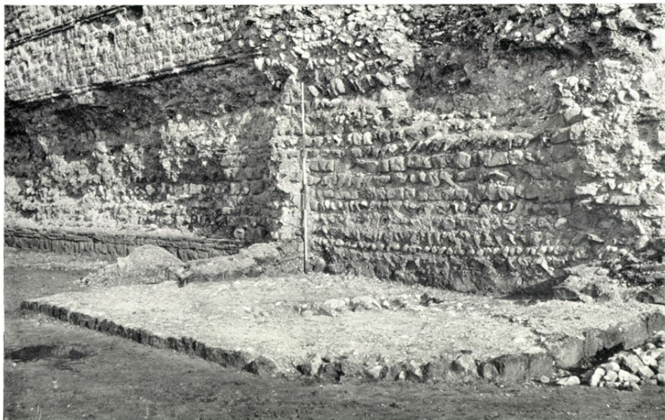
a. Turret, showing remains of its side walls bonded into the fort wall
