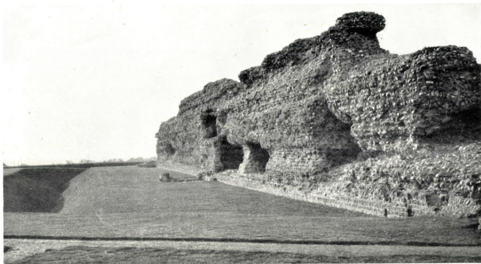
a. Wall, south side, showing berm and ditch at original Roman level
