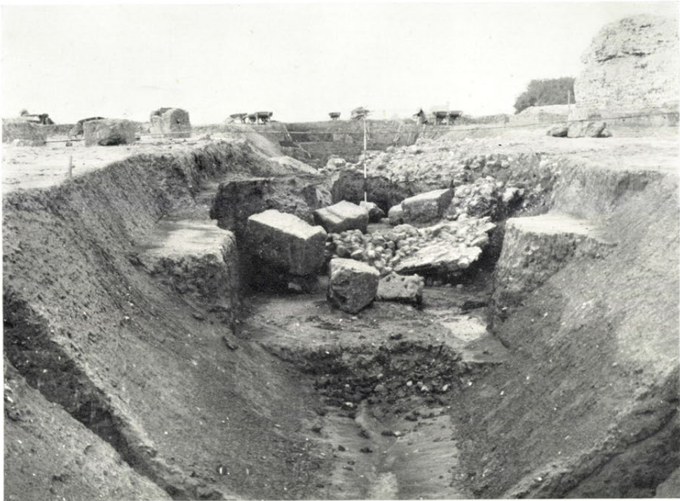
b. Fallen masonry in inner ditch opposite West Gate, p. 68
