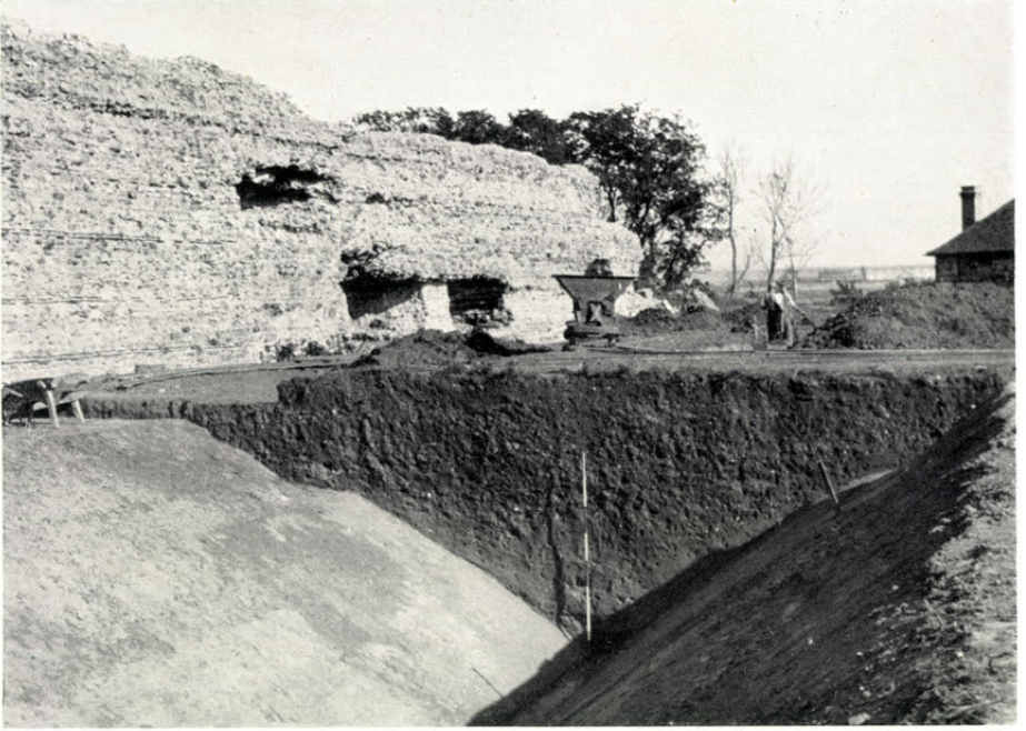
a. Inner ditch, south side, showing the marked difference between the undisturbed soil and the ditch filling
