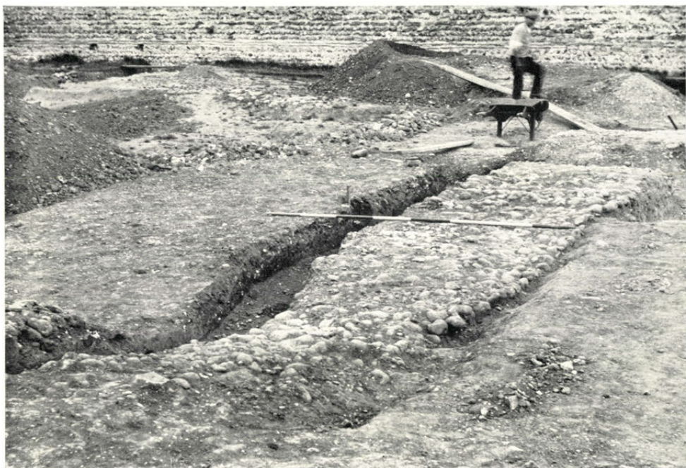
b. Area XI. Metalled causeway across the filled-in outer ditch of the third-century earth fort, p. 62
