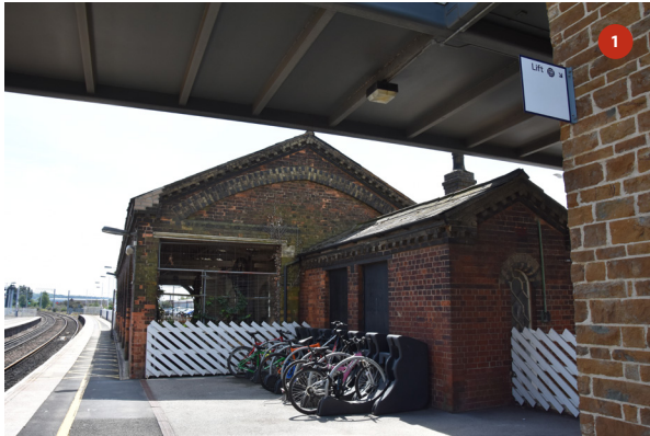
General view of north elevation as viewed from Platform 1
