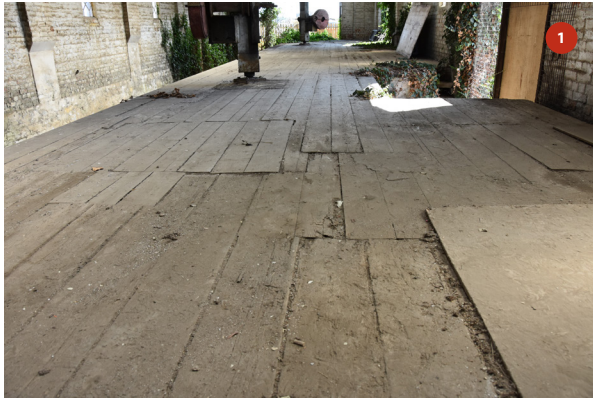
General view of timber boarding of loading platform
