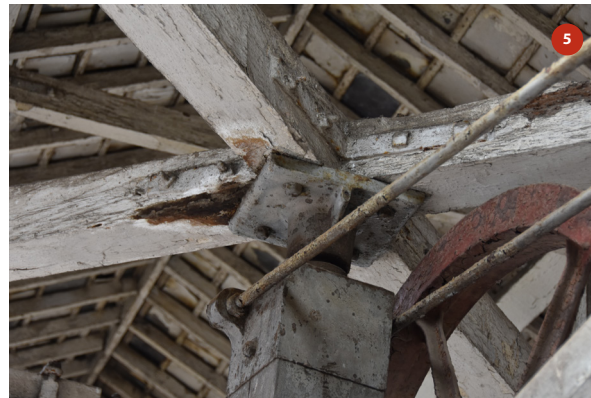
Detail showing connection of jib crane to timber roof structure
