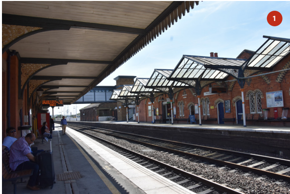
North and east elevations in context of canopies and passenger bridge as viewed from northern end of Platform 2
