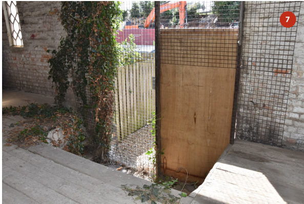
Detail of Bay 5 showing lowered floor around opening
