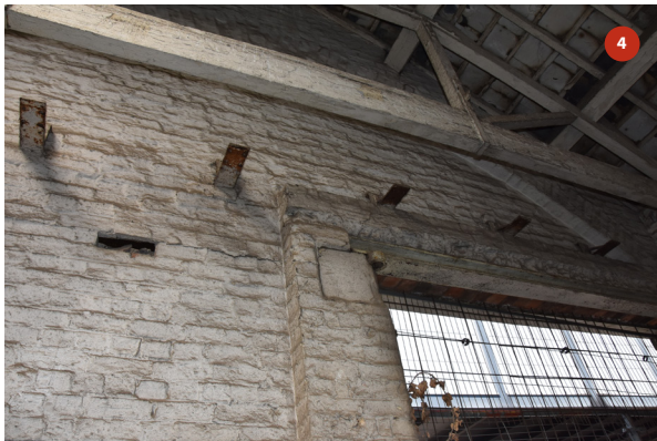
Detail showing wagon entry opening
