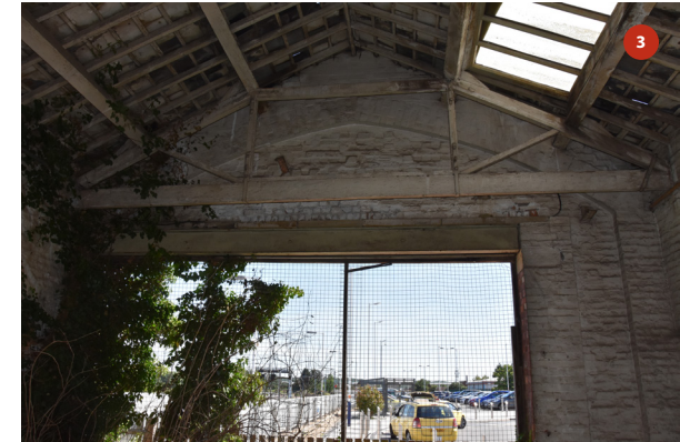
Detail showing the enlarged wagon entry opening
