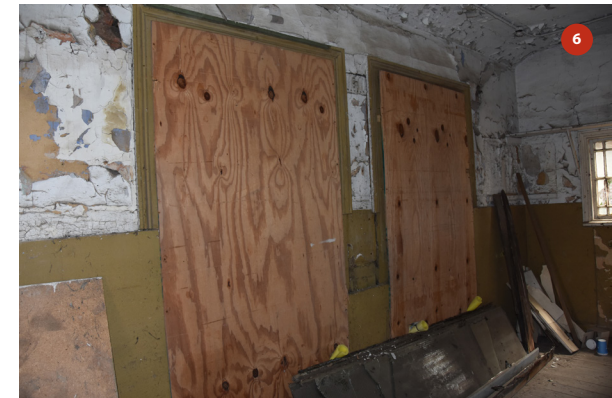
East elevation showing boarded up windows onto Platform 1
