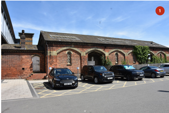
West elevation of goods office and goods shed as viewed from the car park
