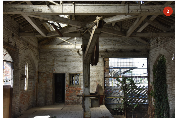
North elevation and jib crane
