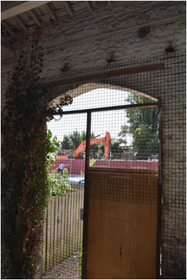
Bay 5 - north opening
