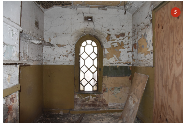
Detail of north elevation showing round headed window
