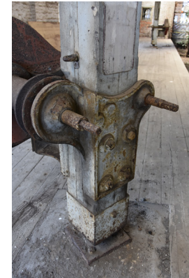
Detail showing base
