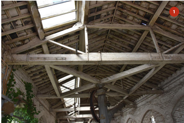
General view of roof structure from southern end
