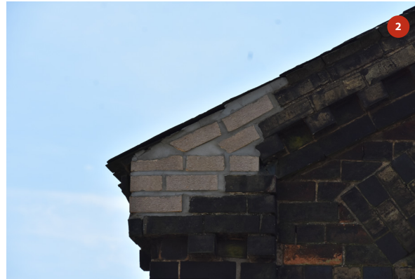
Detail of north elevation showing existing repair to brickwork
