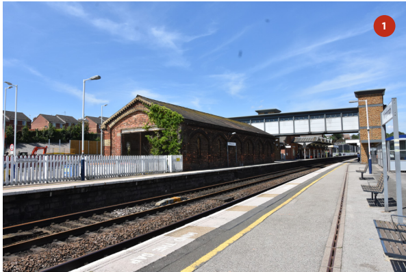
South and east elevations as viewed from southern end of Platform 2
