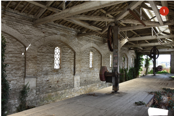
General view of the interior from the north west corner
