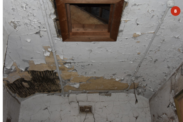
Detail showing the ceiling access hatch in the centre of the room
