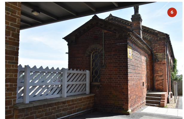
North and west elevations of goods office and good shed beyond
