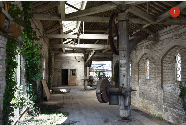
General view of interior looking north
