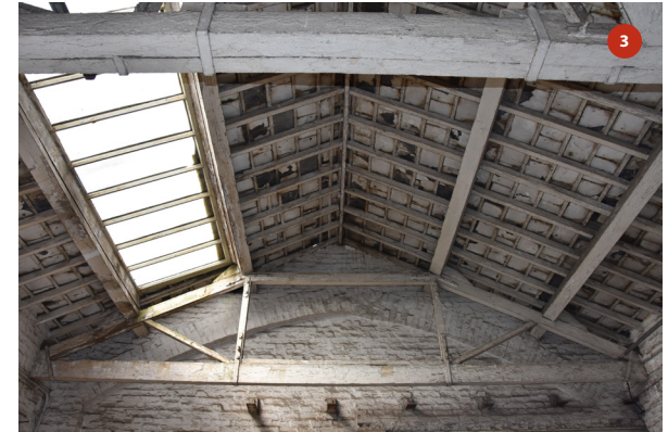
View of timber truss by north elevation
