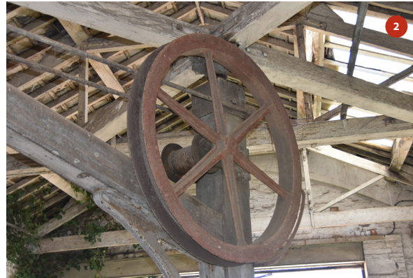
Detail showing part of winding mechanism
