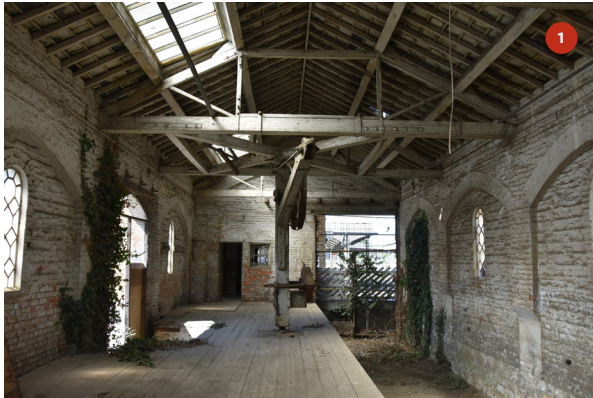
General view of interior looking north
