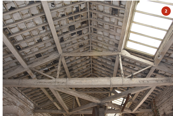
View of timber truss by central skylight
