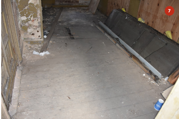
Detail showing the timber flooring
