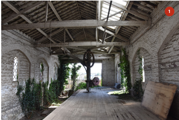
General view of interior looking south
