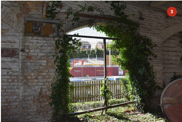
Bay 2 - south opening
