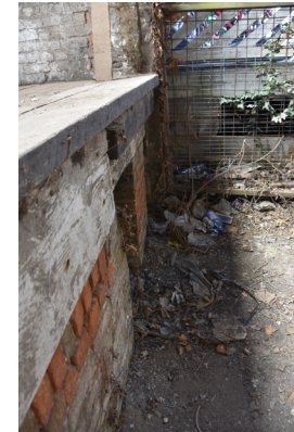
Detail of edge of loading platform looking north
