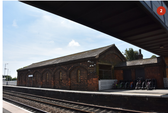
North and east elevations as viewed from Platform 2
