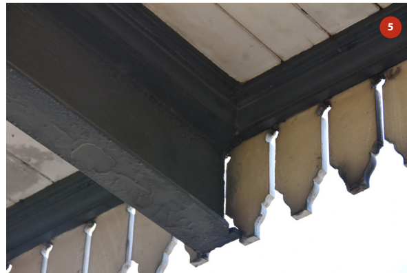
Detail of steel beam and wooden valances
