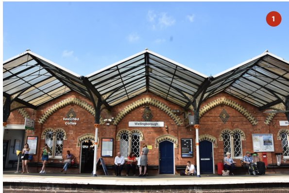
Elevation of bay 4 taken from Platform 2
