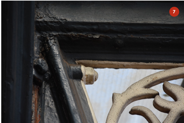
Detail of bolt joining brackets together around central column
