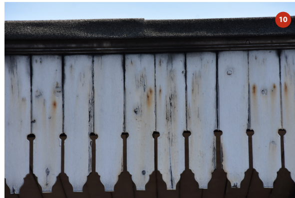
Detail of timber valances taken from Platform 1
