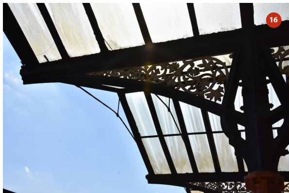
Southern elevation of bay 5
