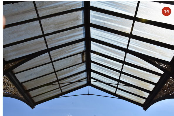
Roof of bay 4
