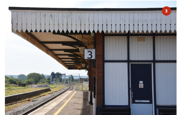
North elevation of canopy over Platform 3
