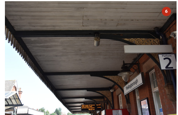
General view of underside of canopy
