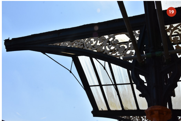
Southern elevation of bay 6
