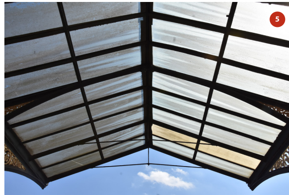
Roof of bay 1
