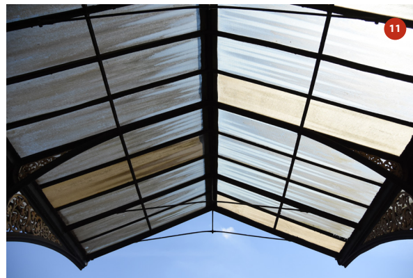
Roof of bay 3
