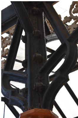
Detail of bolts joining brackets together around central column
