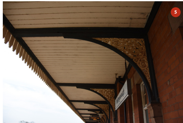
General view of underside of canopy
