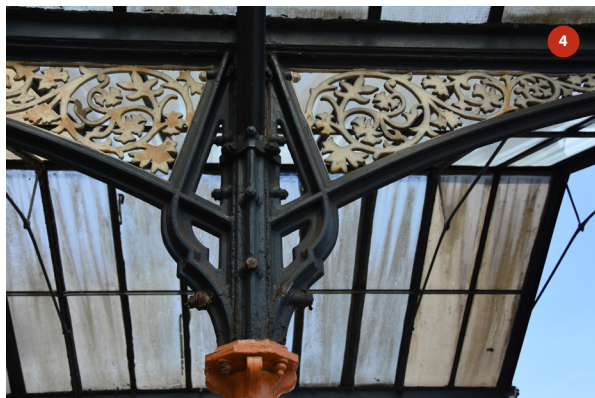
Detail of bolts and strapping joining brackets together around central column
