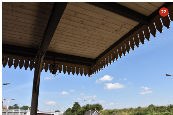
Timber canopy northern corner internal view
