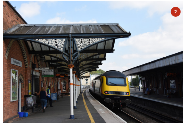
View from south of Platform 1 showing southern 1883 canopy
