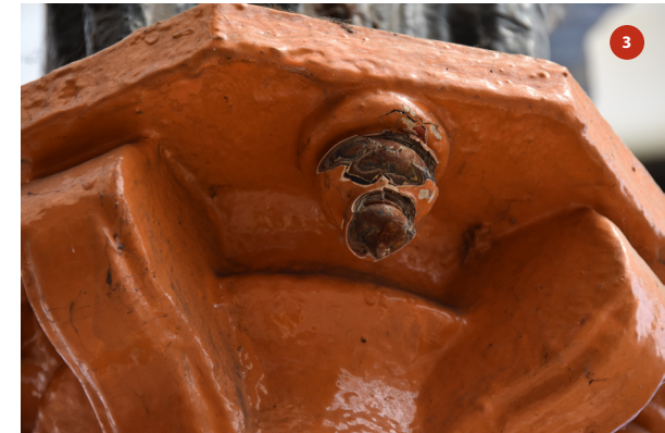
Detail of where brackets meet column (close up of photo 2)
