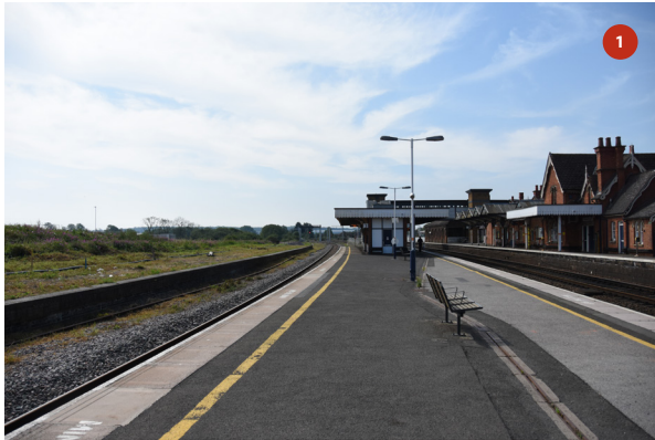
General view from north end of Platforms 2 & 3
