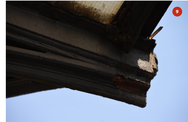
Detail of bracket and gutter beam end
