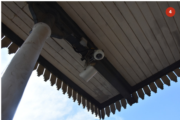
Southern corner internal view
