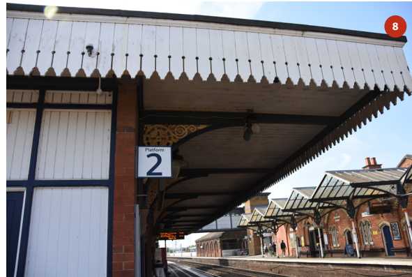
North elevation of canopy
