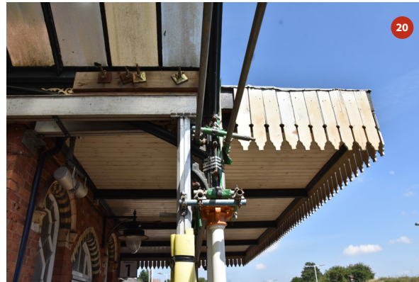
Location of spandrel removed for trial dismantling
