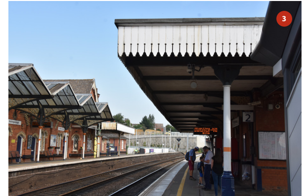
South elevation of canopy
