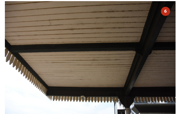
Southern corner internal view
