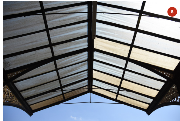
Roof of bay 2
