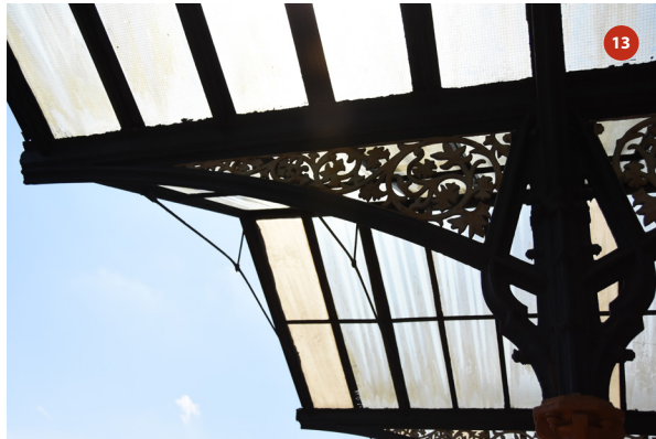
Southern elevation of bay 4
