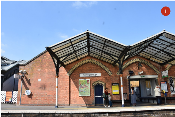
Elevation of bay 1 taken from Platform 2
