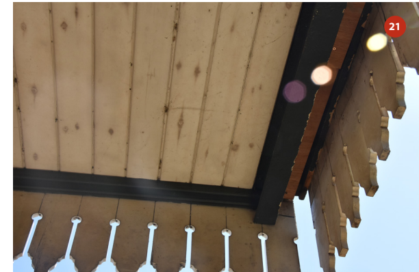
Timber canopy southern corner internal view
