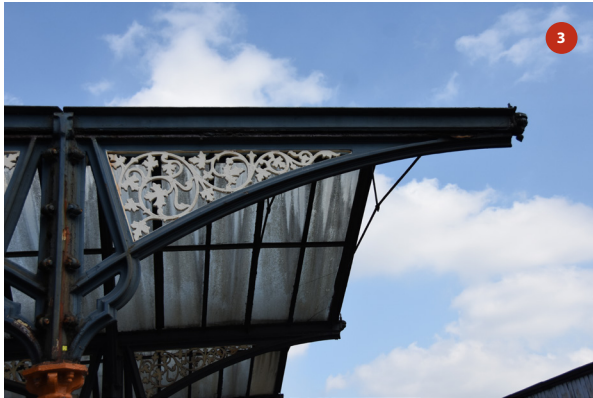
Southern end of Platform 1 canopy
