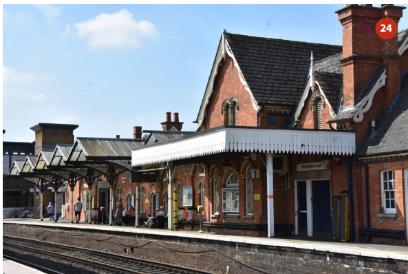
View of Platform 1 timber canopy from Platform 2
