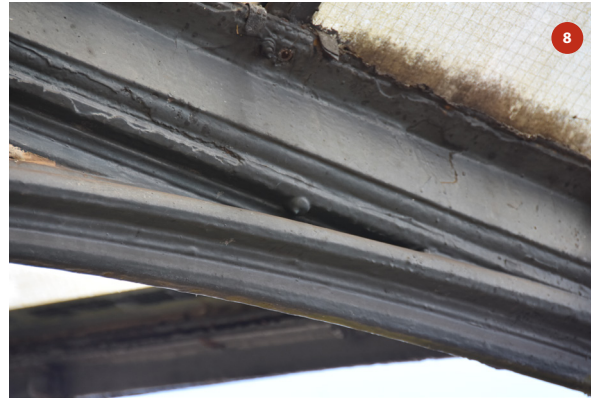
Detail of bracket connection with gutter beam
