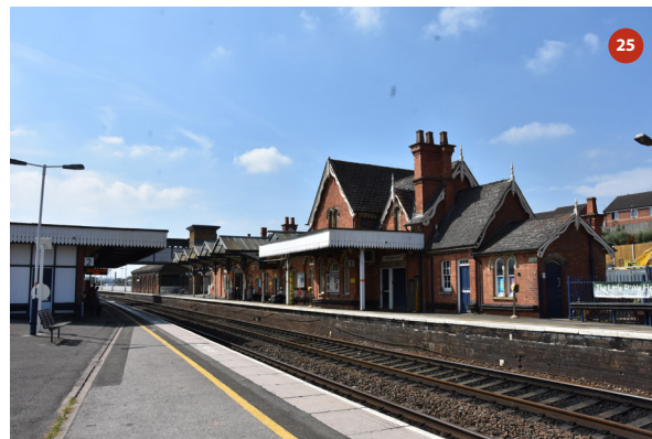
View of Platform 1 from northern end of Platform 2
