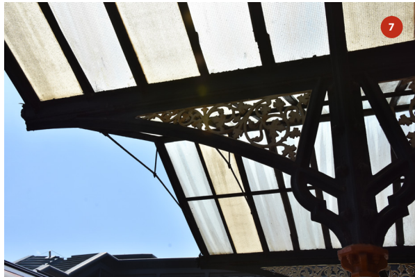
Southern elevation of bay 2
