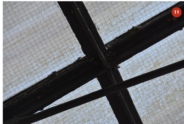
Detail of purlin connection to tied rafter
