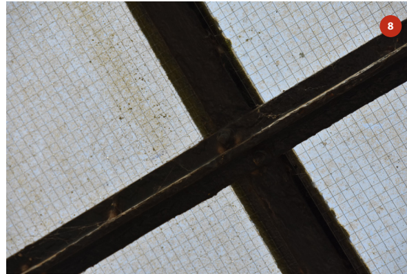
Detail of purlin connection to secondary rafter
