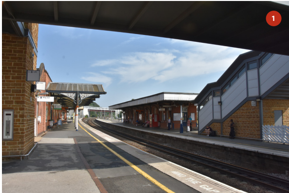
General view from south end of Platform 1
