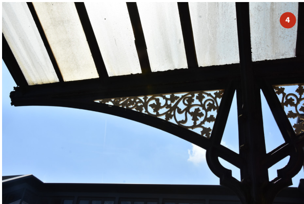
Southern elevation of bay 1
