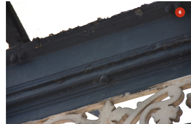
Detail of bracket connection with gutter beam
