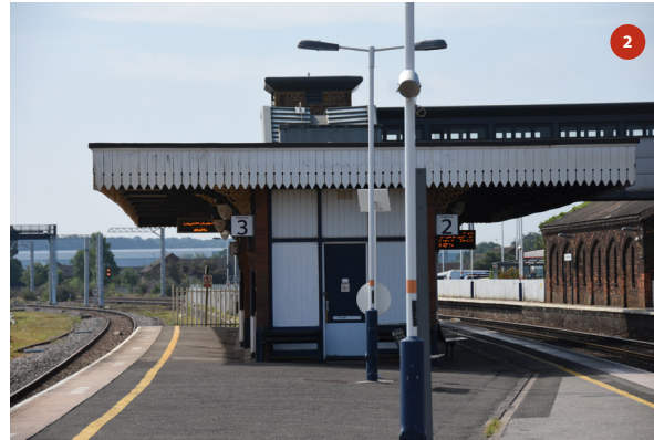
North elevation of canopy over Platforms 2 & 3
