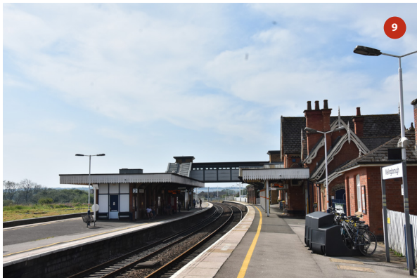
General view from north end of Platform 1
