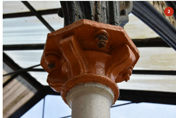
Detail of where brackets meet column
