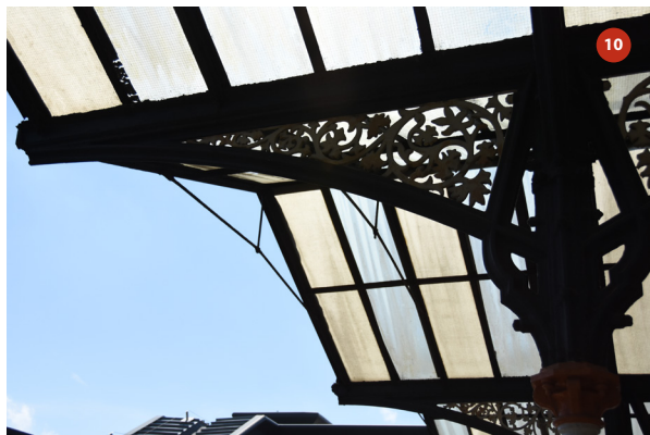
Southern elevation of bay 3
