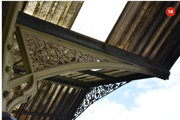
Southern elevation of bay 5
