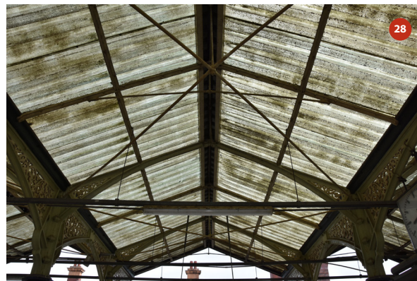
Roof of bay 8
