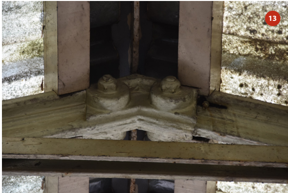
Detail of connection between two rafters (close up of photo 12)
