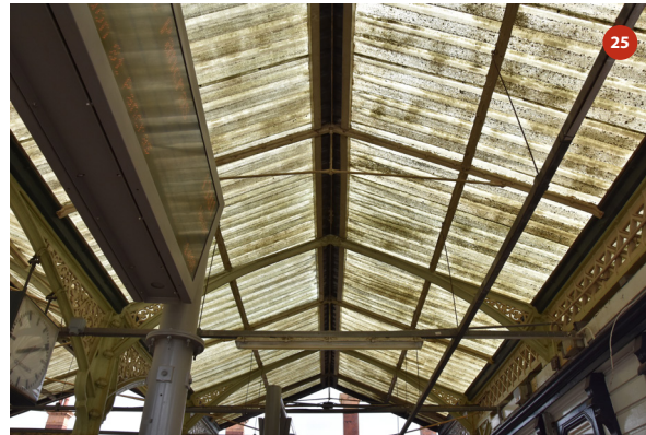
Roof of bay 7
