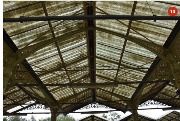
Roof of bay 5
