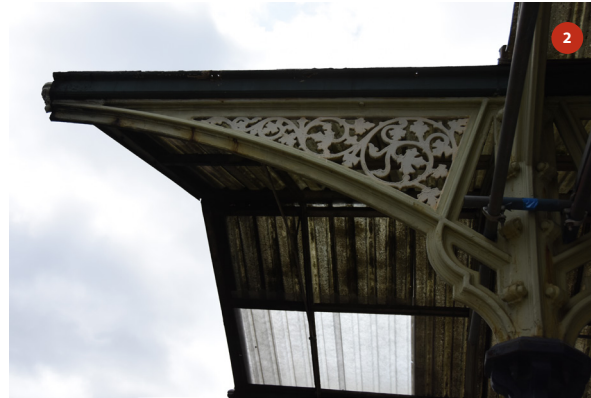
Southern elevation of bay 1
