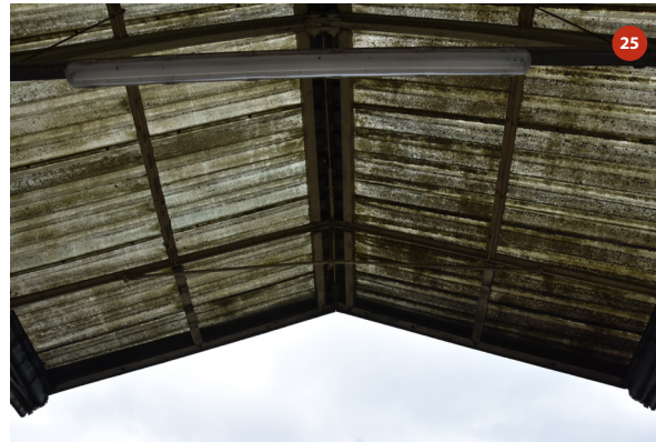
Roof of bay 9
