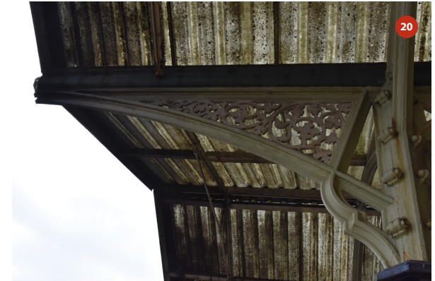
Southern elevation of bay 7
