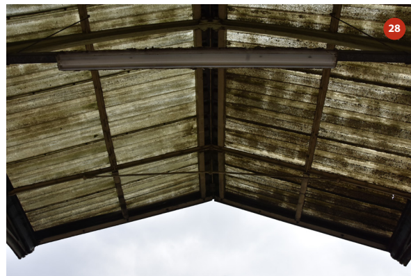
Roof of bay 10
