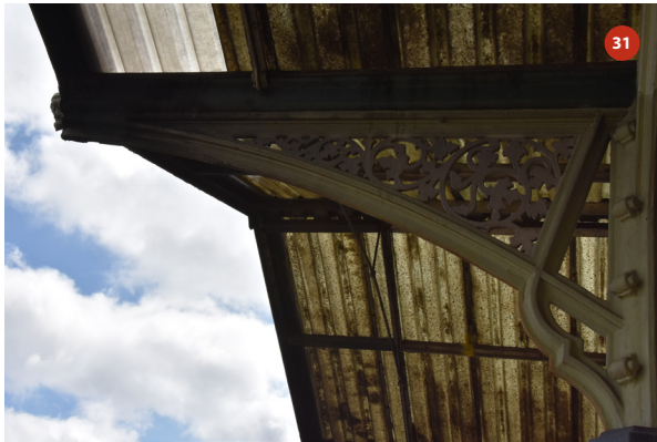
Southern elevation of bay 10
