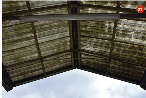
Roof of bay 11
