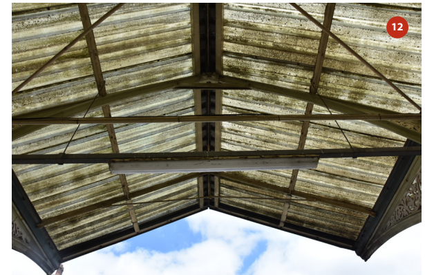
Connection of two rafters at apex of bay roof
