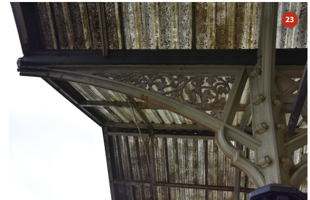
Southern elevation of bay 8
