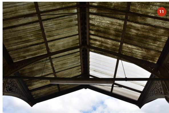
Roof of bay 3
