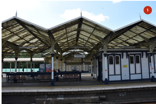
Elevation of bay 4, platform 2 as seen from the middle of platform 1
