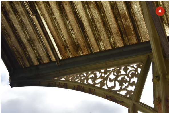
Southern elevation of bay 1
