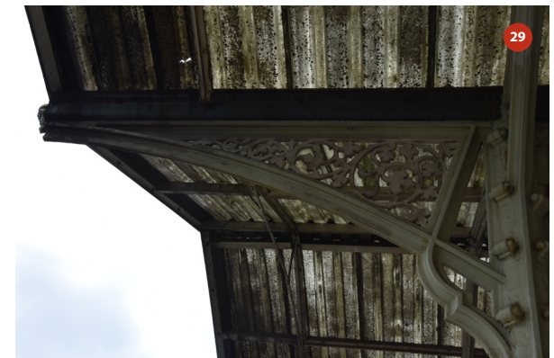
Southern elevation of bay 10
