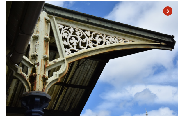
Southern end of platform 4 canopy
