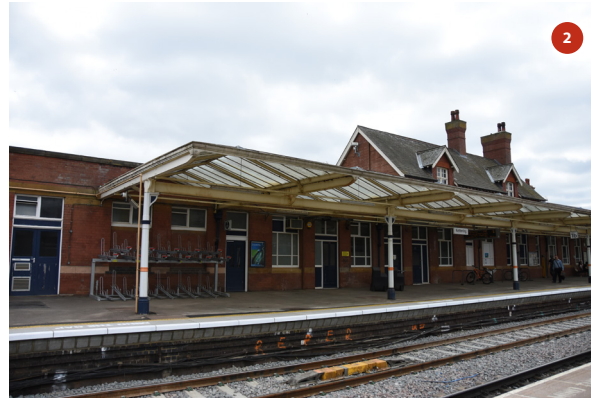
Northern end of platform 1 canopy looking east from platform 2
