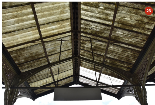
Roof of bay 7
