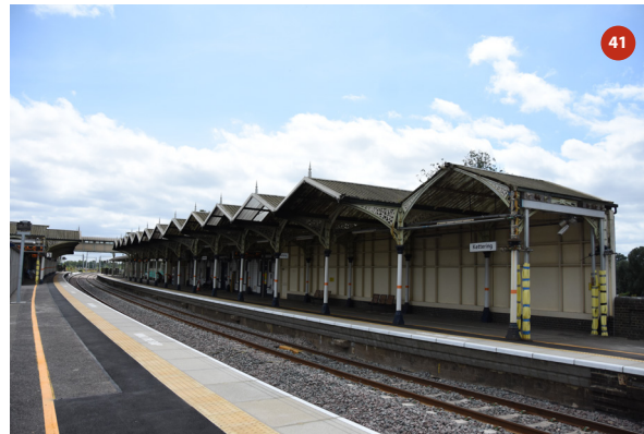
Platform 4 canopy seen from northern end of platforms 2/3
