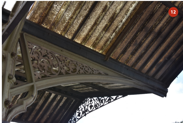
Southern elevation of bay 3
