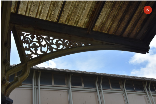
Southern elevation of bay 1
