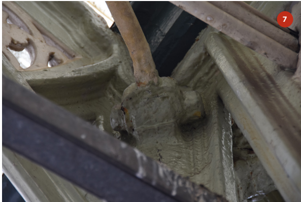
Detail of cross-bracing connection to bracket bolt (close up of photo 6)
