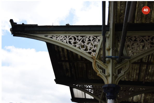
Southern elevation of bay 13
