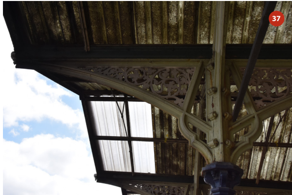
Southern elevation of bay 12
