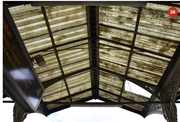
Roof of bay 8
