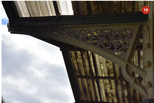
Southern elevation of bay 6
