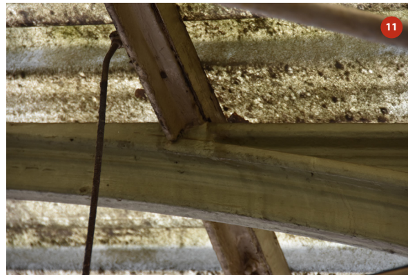
Detail of rafter connection with purlin
