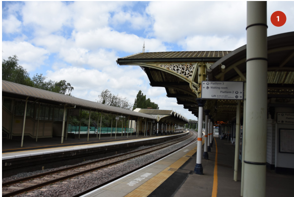
Platform 4 canopy seen from southern end of platform 3
