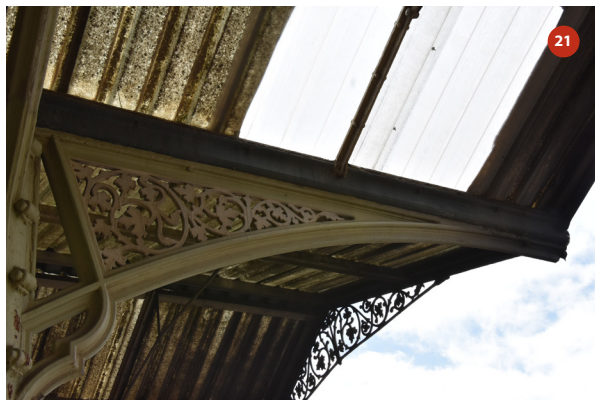
Southern elevation of bay 6
