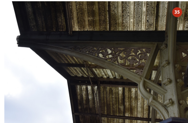
Southern elevation of bay 12
