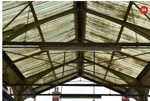
Roof of bay 10
