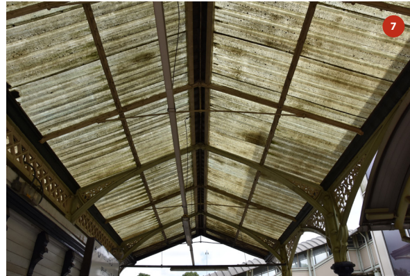
Roof of bay 1
