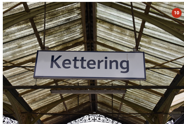
Roof of bay 4
