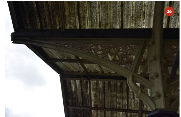
Southern elevation of bay 9
