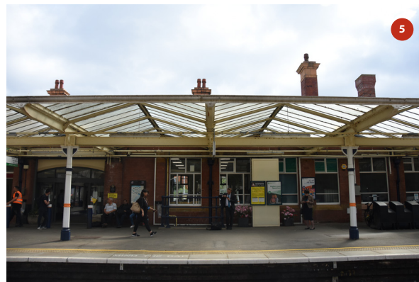
Elevation of platform 1 canopy, seen from middle of platform 2
