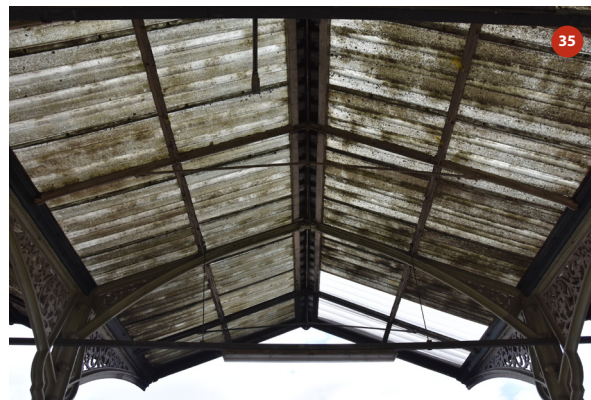
Roof of bay 11
