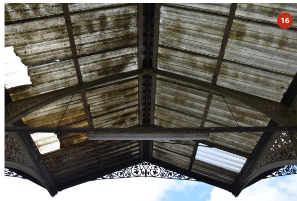
Roof of bay 4
