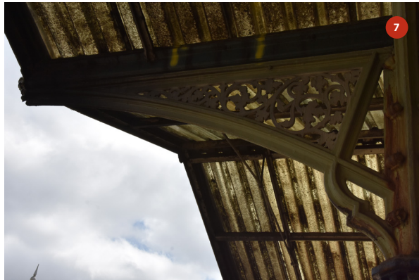
Southern elevation of bay 2
