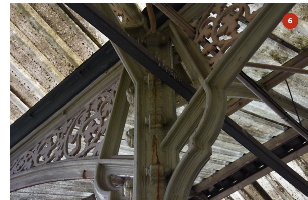
Detail of cross-bracing connection to bracket bolt
