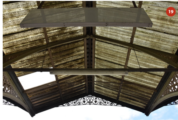
Roof of bay 5
