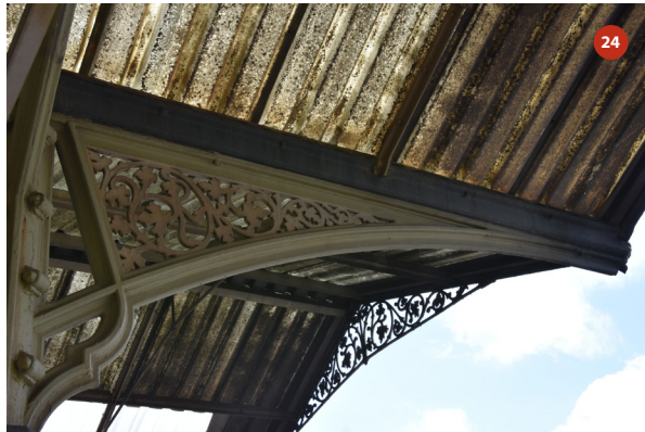
Southern elevation of bay 7
