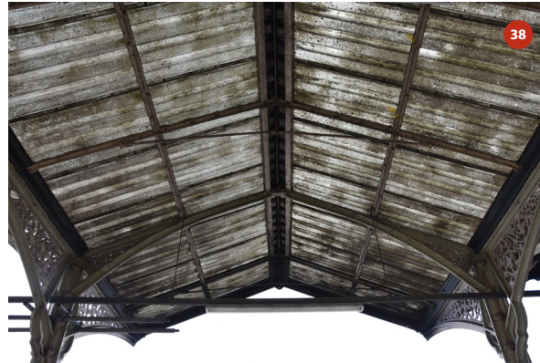
Roof of bay 12
