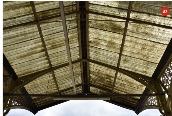
Roof of bay 13
