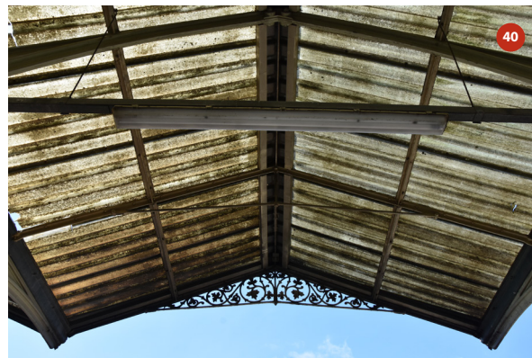
Roof of bay 12
