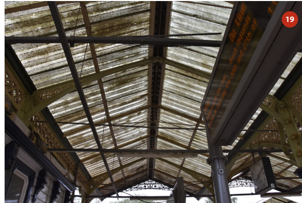
Roof of bay 7
