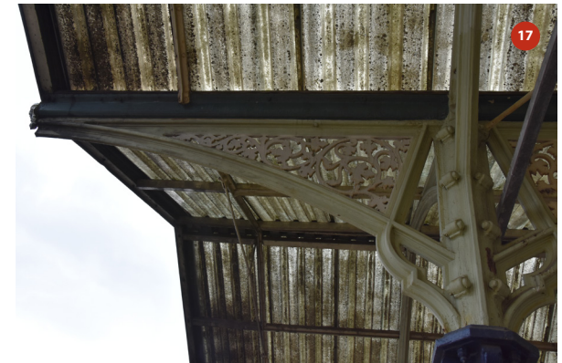
Southern elevation of bay 6
