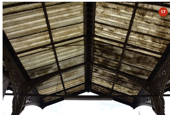
Roof of bay 5
