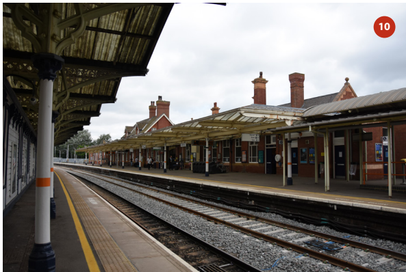
Platform 1 canopy, looking north-east from the southern end of platform 2
