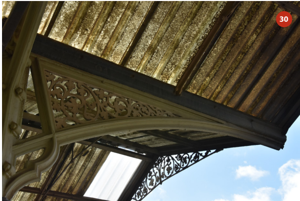
Southern elevation of bay 9
