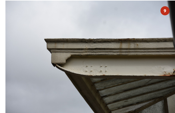
Detail of southern end of platform 1 canopy
