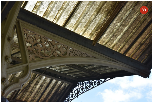
Southern elevation of bay 10
