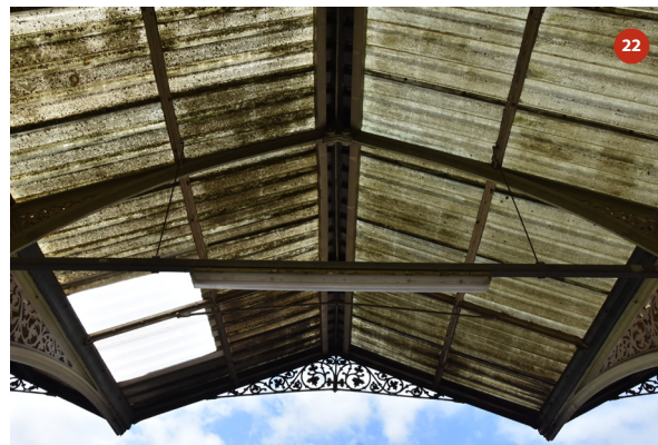
Roof of bay 6
