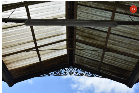
Roof of bay 11
