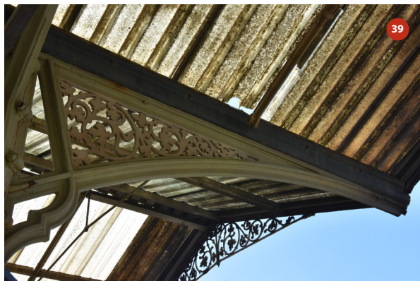
Southern elevation of bay 12
