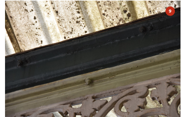
Detail of bracket connection with gutter beam (close up of photo 8)
