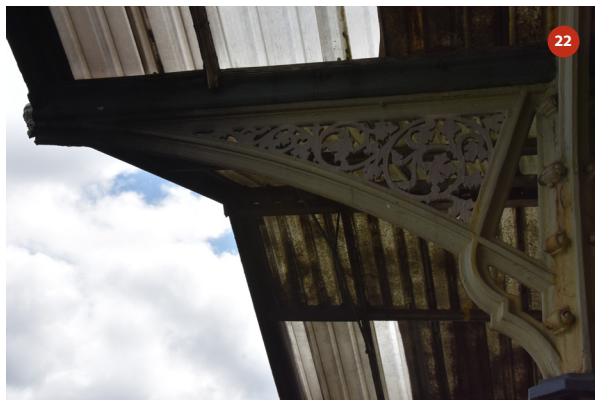
Southern elevation of bay 7
