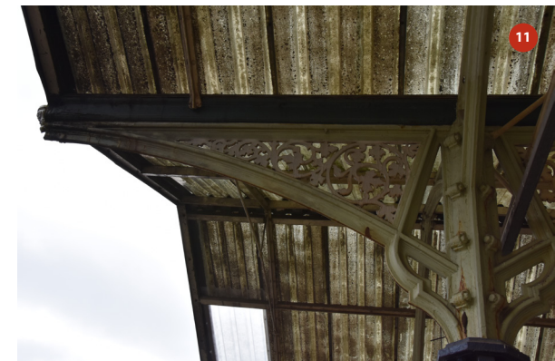
Southern elevation of bay 4
