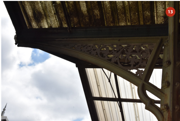
Southern elevation of bay 4
