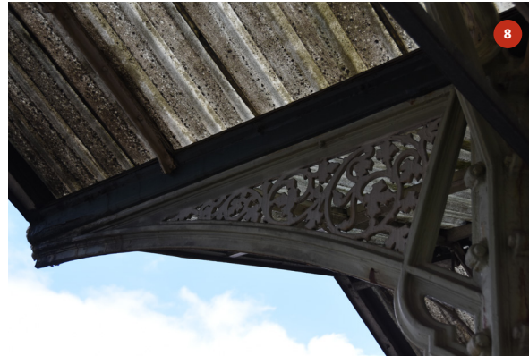
Bracket connection with gutter beam
