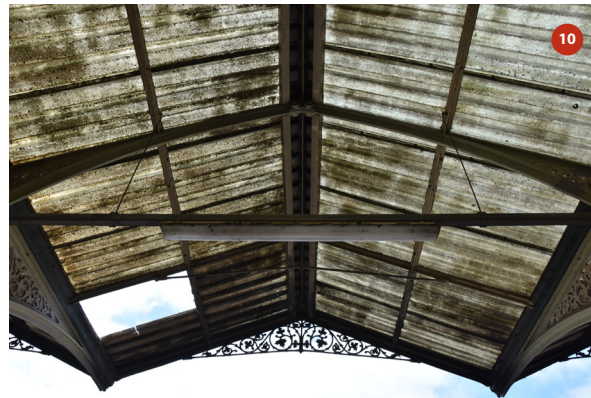
Roof of bay 2
