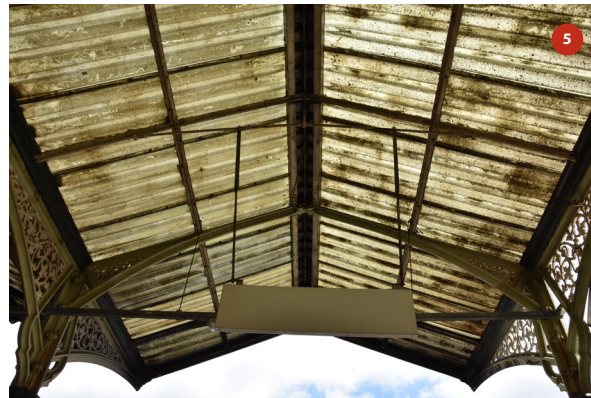
Roof of bay 1
