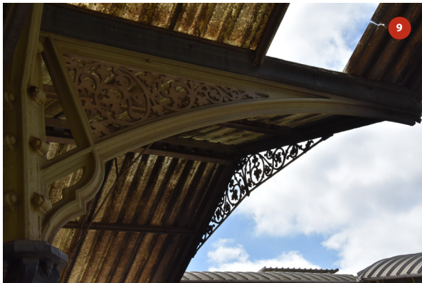
Southern elevation of bay 2
