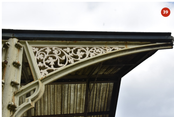
Southern end of platform 2 canopy
