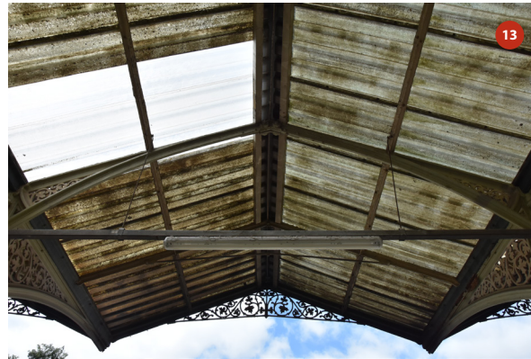
Roof of bay 3
