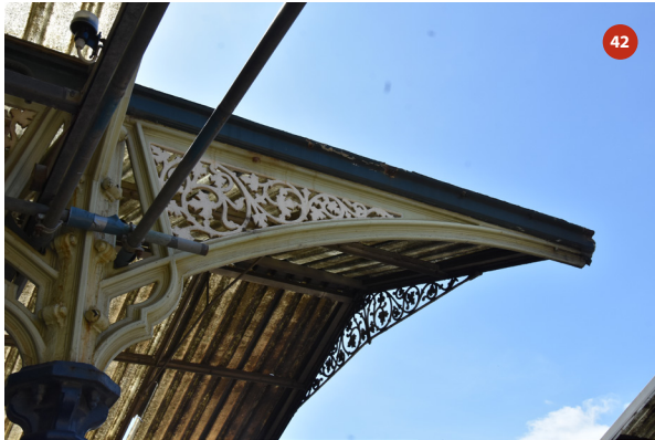
Southern elevation of bay 13
