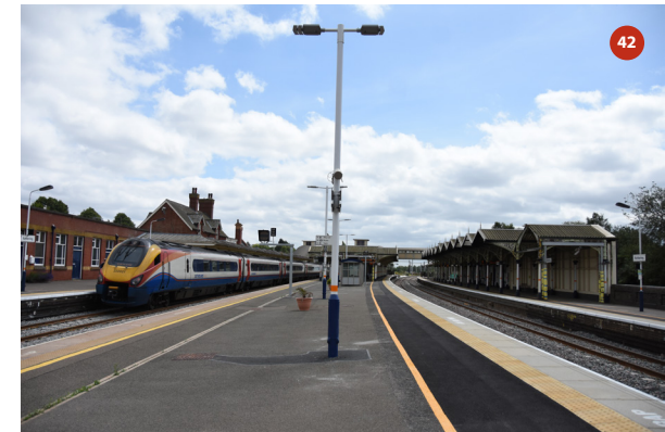
Platform 4 canopy seen from extreme northern end of platforms 2/3
