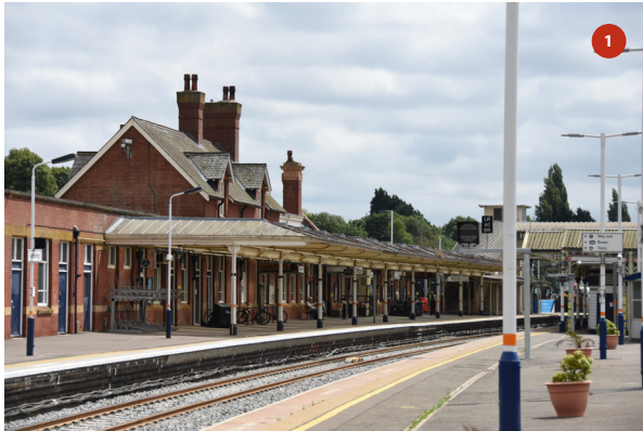
Platform 1 canopy looking south-east from the northern end of platform 2
