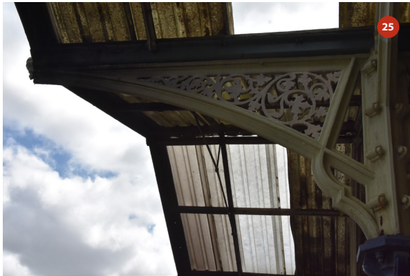
Southern elevation of bay 8
