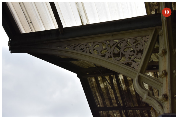
Southern elevation of bay 3
