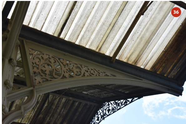
Southern elevation of bay 11
