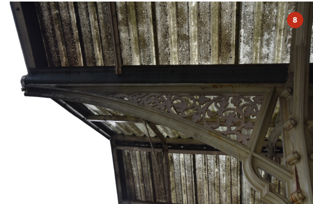
Southern elevation of bay 3
