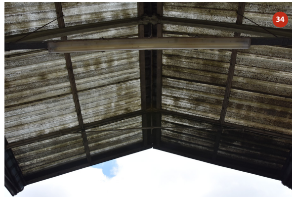
Roof of bay 12
