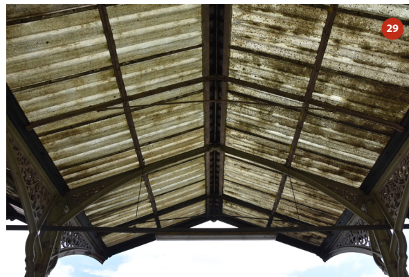
Roof of bay 9
