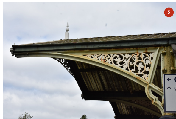
Southern end of platform 3 canopy
