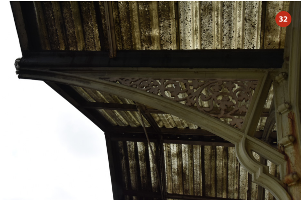
Southern elevation of bay 11
