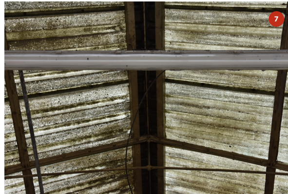
Roof of bay 3
