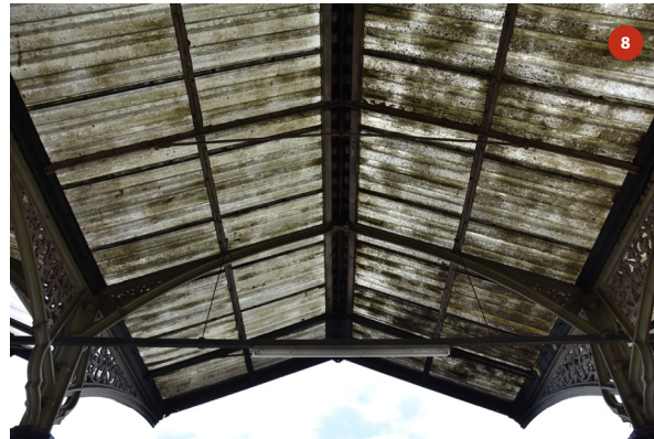
Roof of bay 2
