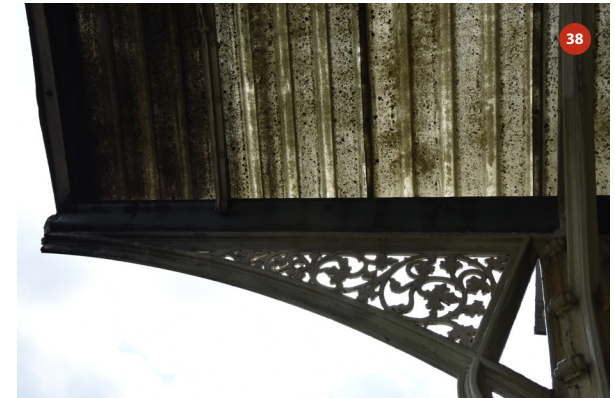
Southern elevation of bay 13
