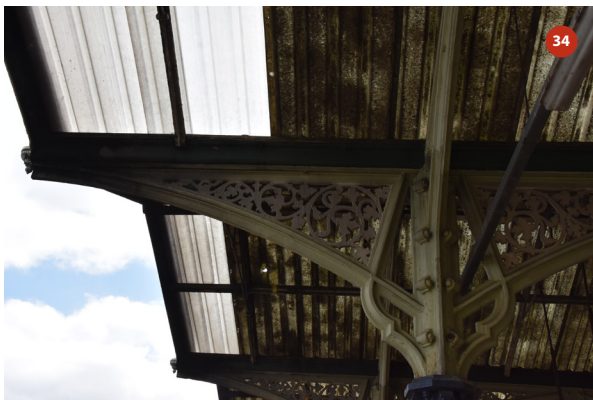
Southern elevation of bay 11
