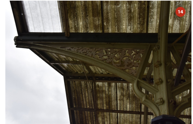
Southern elevation of bay 5
