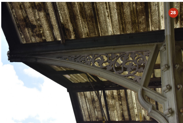
Southern elevation of bay 9
