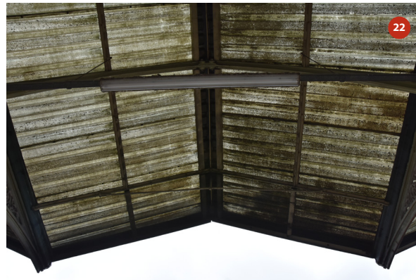
Roof of bay 8
