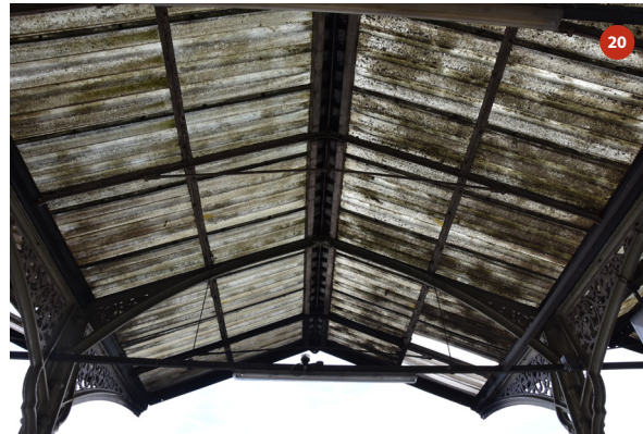
Roof of bay 6
