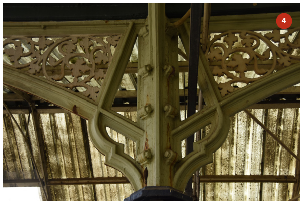
Detail of bolts joining brackets together around central column
