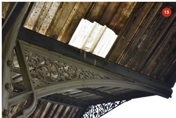
Southern elevation of bay 4
