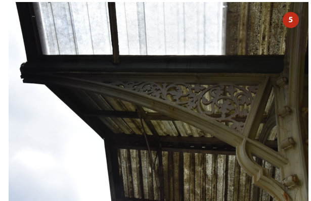
Southern elevation of bay 2
