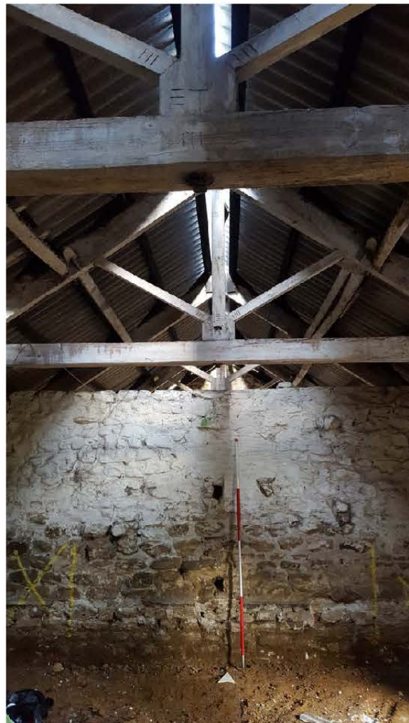
119-200_roof detail_carpenters marks III 200 both trusses and 201
