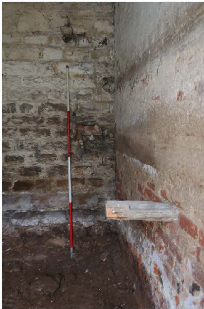
082_2000_2240-2103_trough W wall
