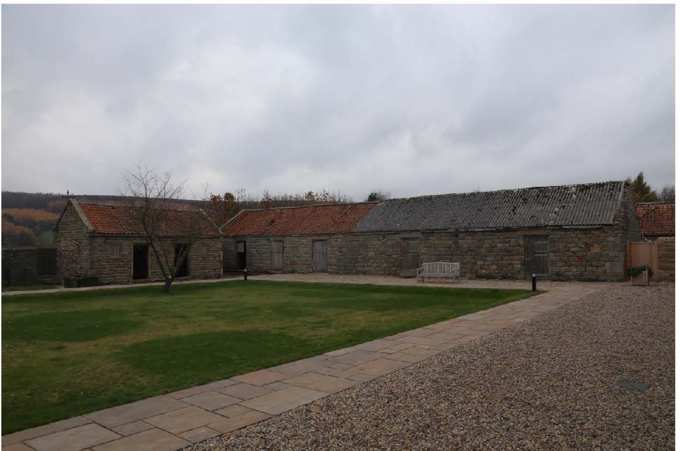
089_Gen_view of stable and byre ll. SW
