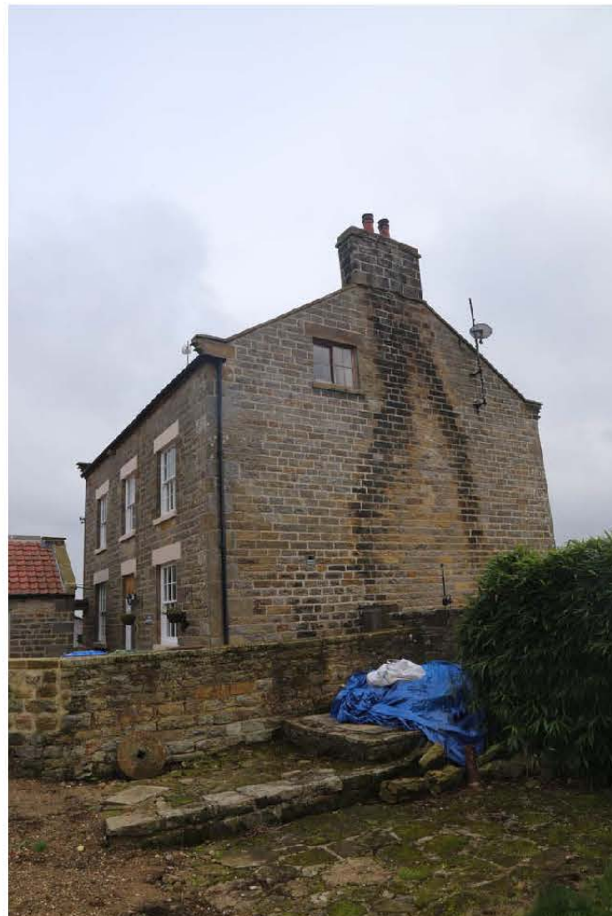
091_Gen_view of W gable of house lk SW
