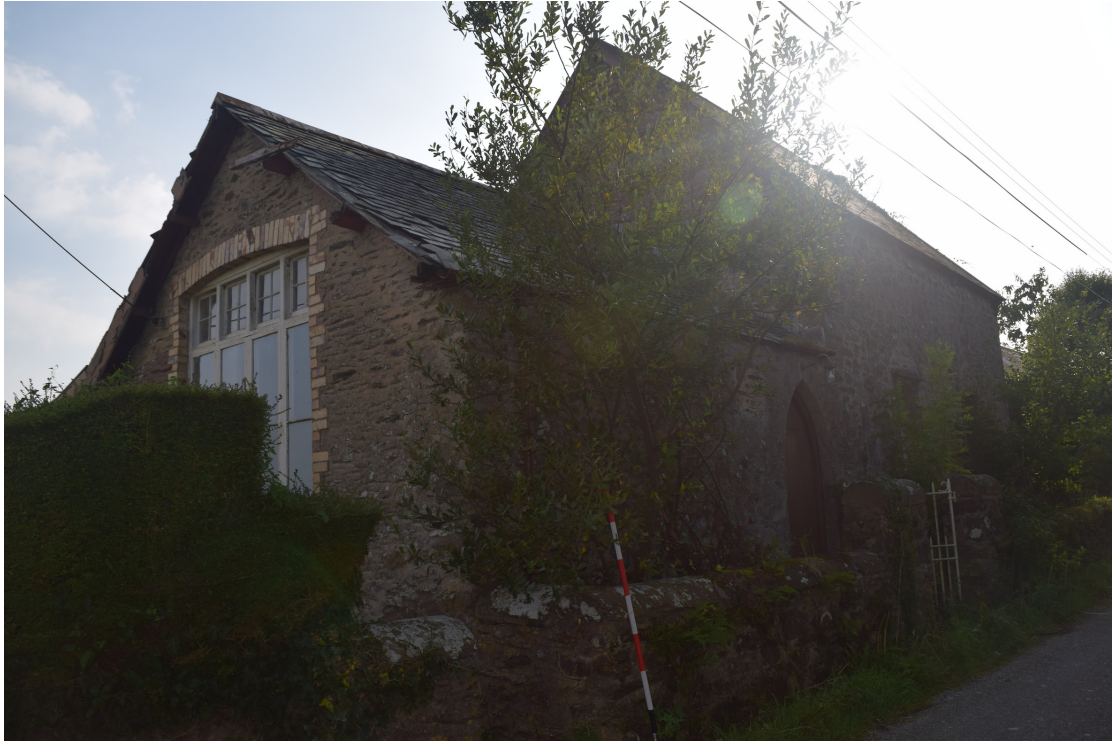
Figure 17 – View of the chapel from the road
