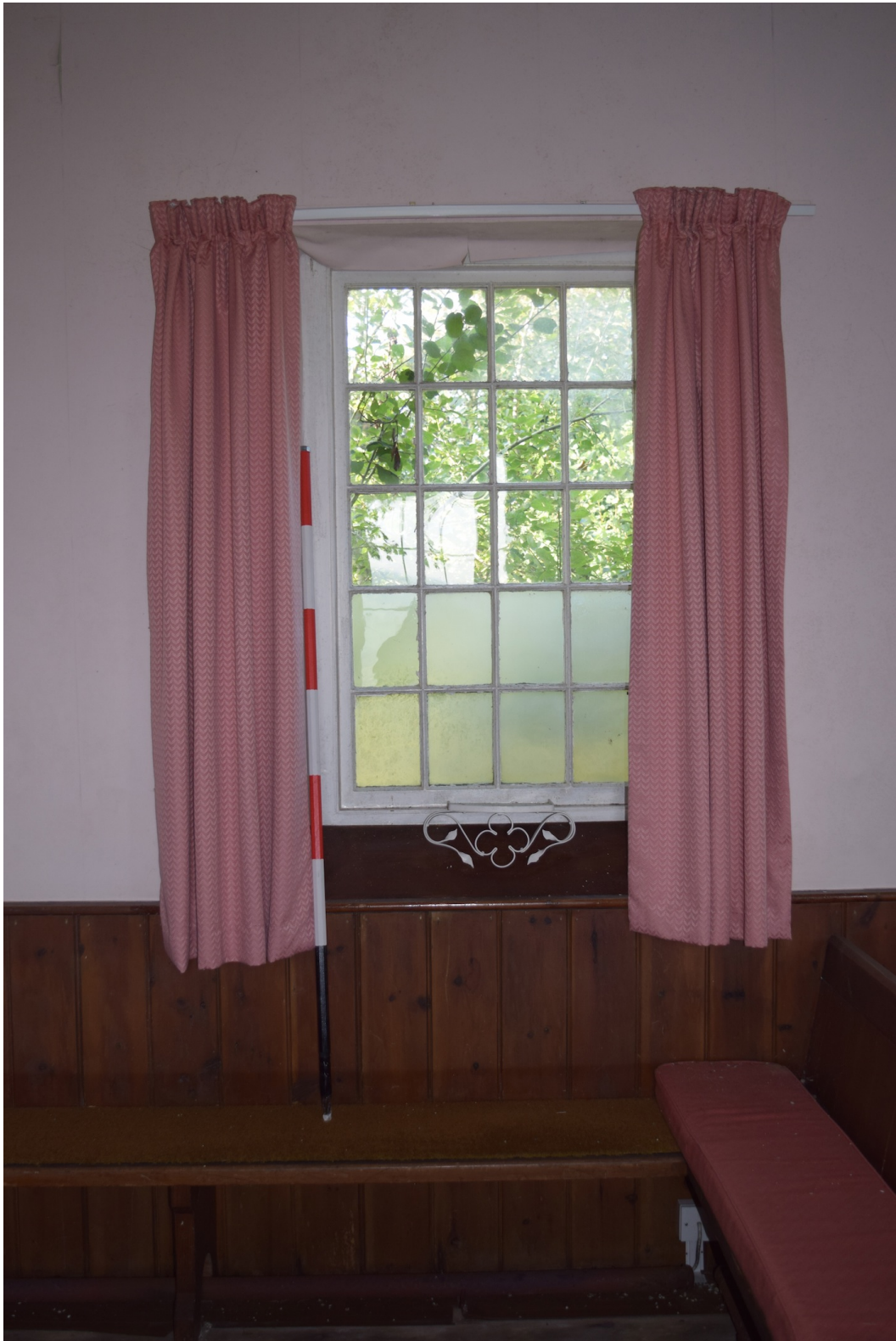
Figure 12 – one of the windows in the original section of the hall
