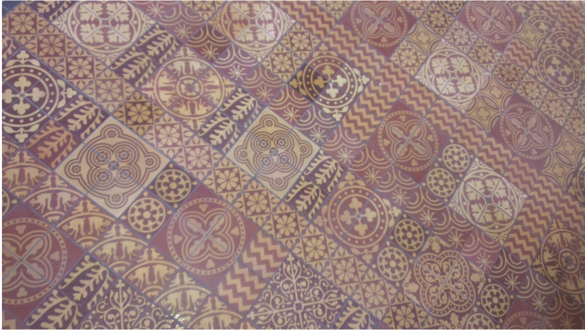
Figure 11: Encaustic tiles used to decorate the floor of the local Chapel in Lugwardine. © CHAC
