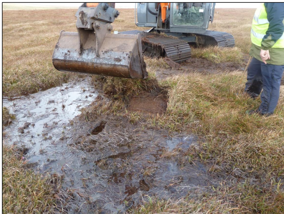
Plate 1 Peat being extracted for use in block construction.
