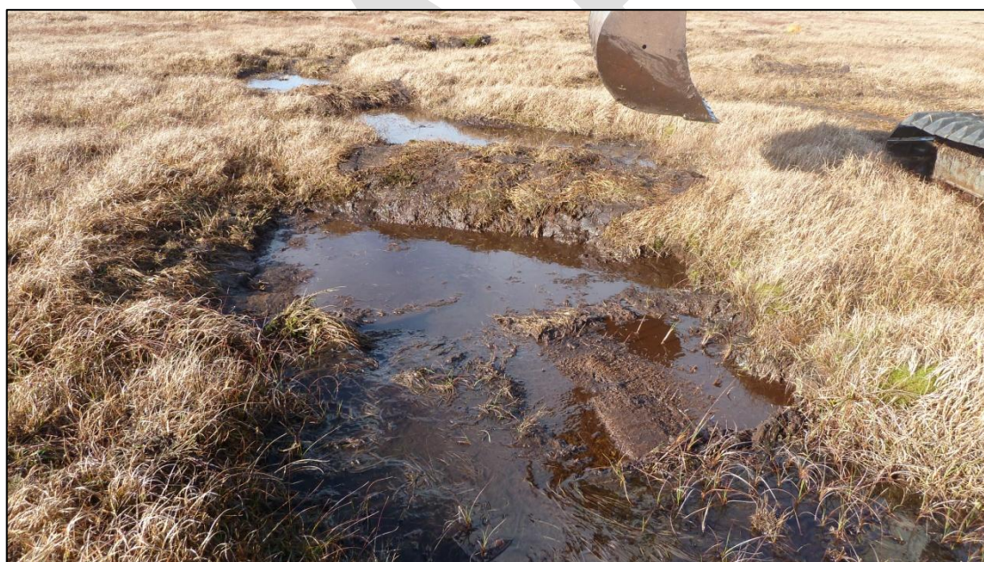
Plate 6 Erosion gully after block construction.
