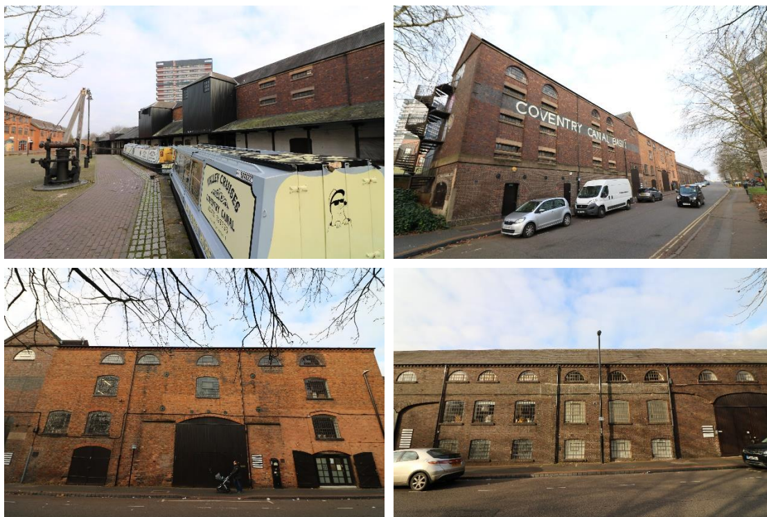
Fig 27: Coventry Canal Basin, with the Grand Union wharf and warehouses. Photographs by authors
