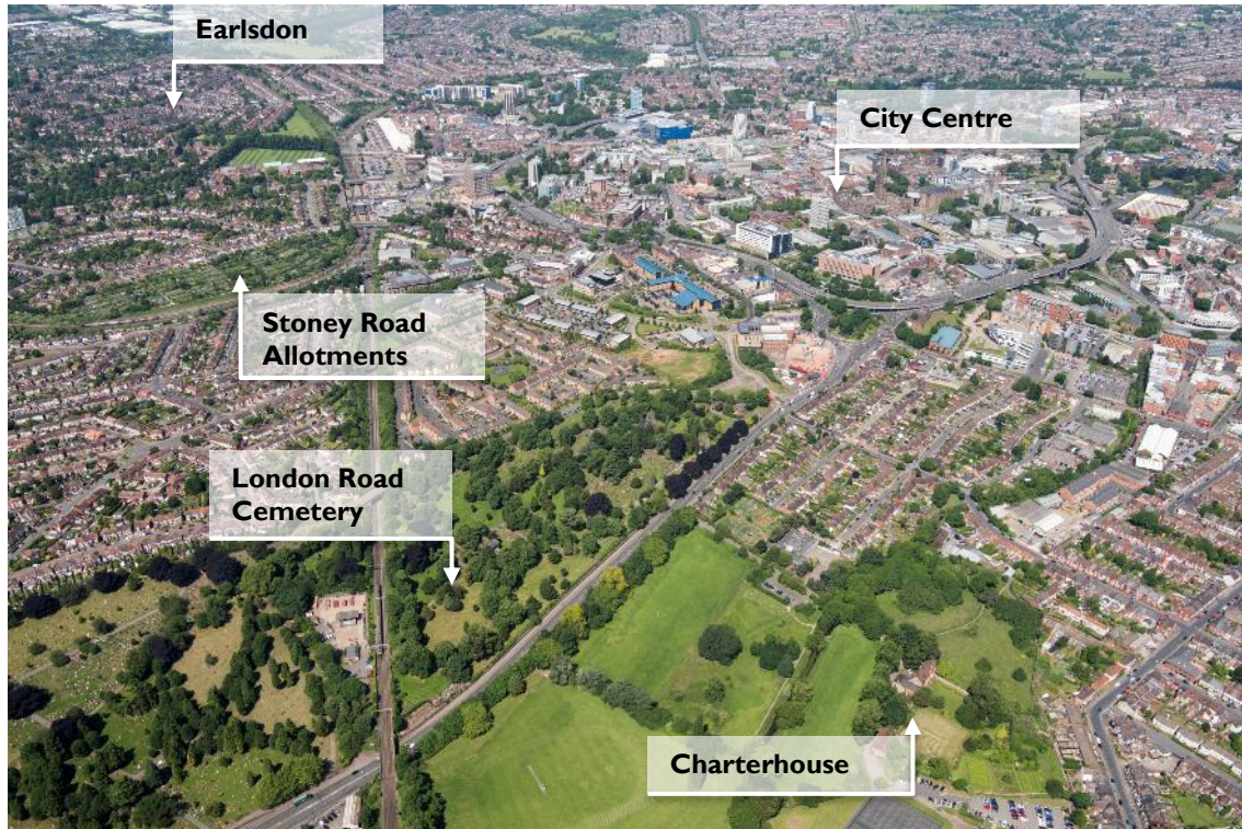
Fig 80: Aerial view looking towards the city centre from the southeast. Labelled places of historic significance that, whilst peripheral to the centre, have held close historical connections, both physically and cognitively. The ring road can be seen to have created a clear boundary between the centre and this environ. Historic England (33181_027)
