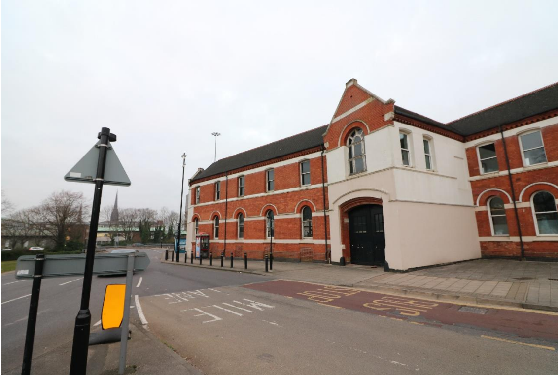
Fig 84: Surviving elements of an early 20 th century factory facing onto Mile Lane. Photograph by authors
