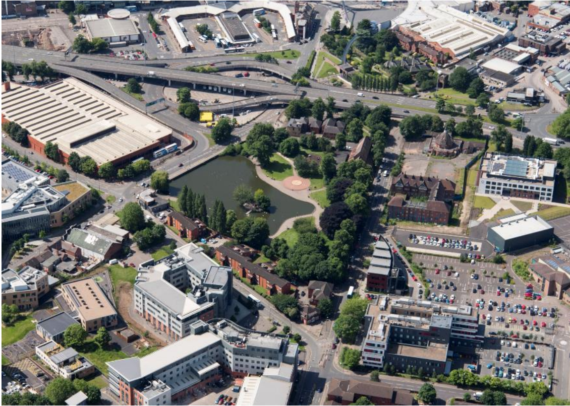
Fig 82: Aerial view from the northeast of: Swanswell Park and Pool (centre), Lady Herbert's Garden (top-right), and the remnants of the old hospital (right). Historic England (33178_019).
