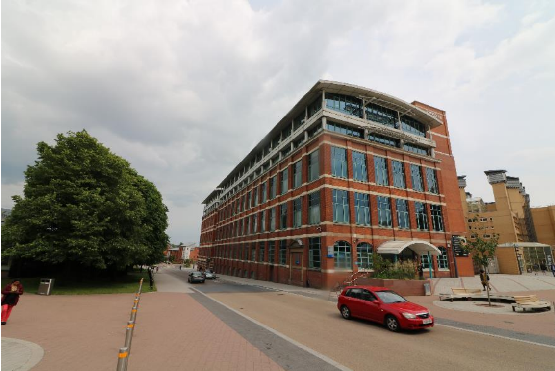
Fig 30: 90-94 Gosford Street (William Morris Building). Photograph by authors
