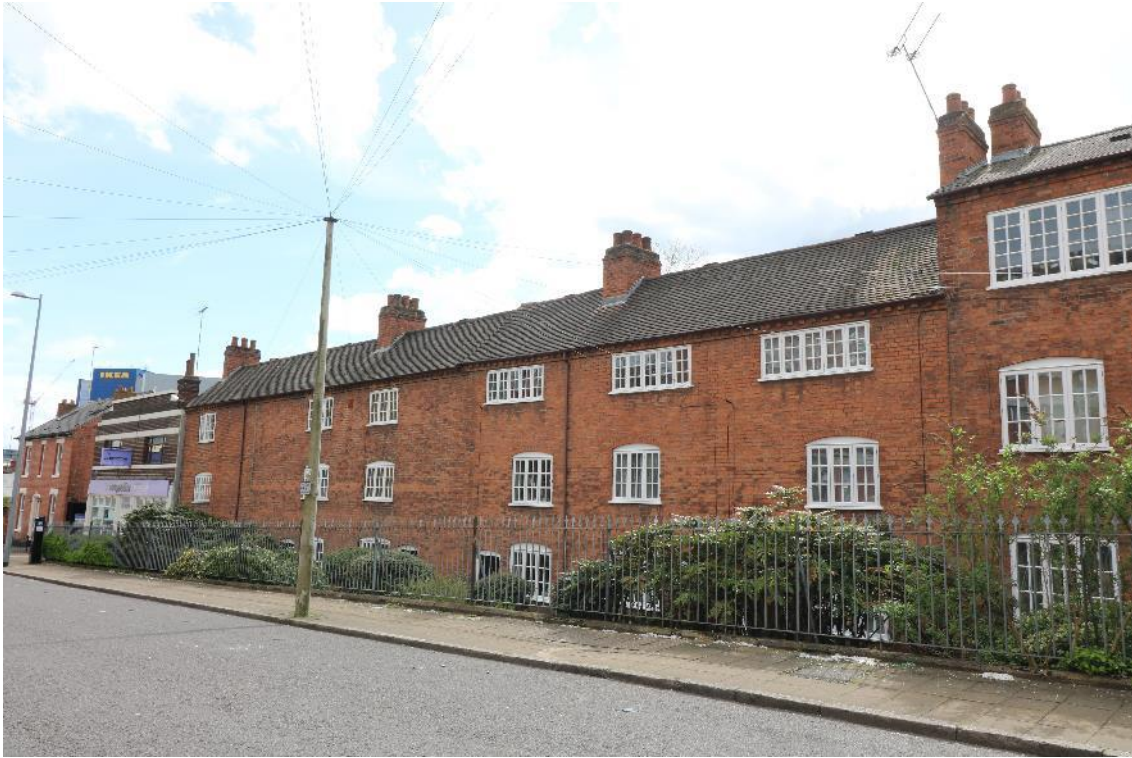
Fig 28: A small but notable collection of the mixed use 'top-shops' that were once common in the centre survive today such as 13-29 Lower Holyhead Road. Photograph by authors
