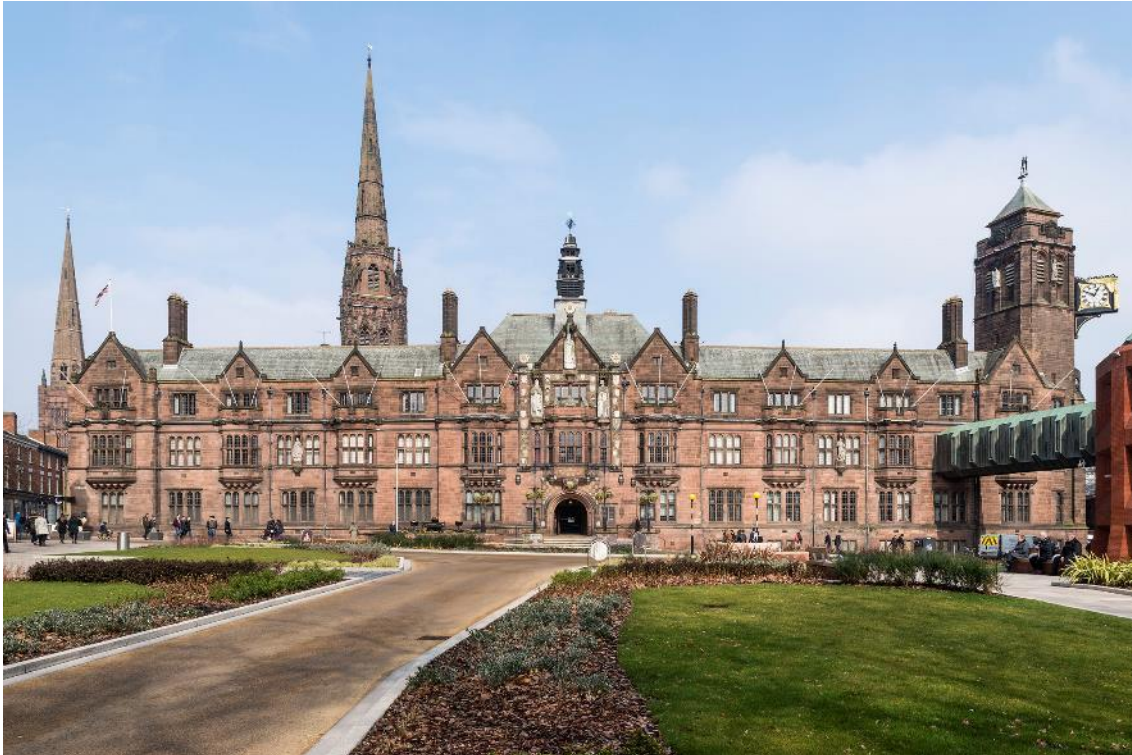
Fig 35: The Council House, Earl Street. Historic England (DPI 72629)
