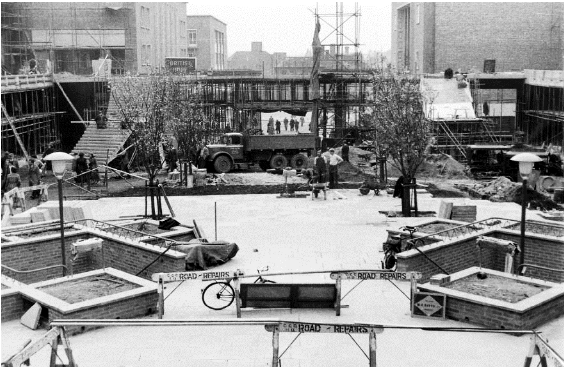
Fig 13: The Leofric Hotel (top) and Upper Precinct (bottom) under construction c.1953-55. Coventry Archive
