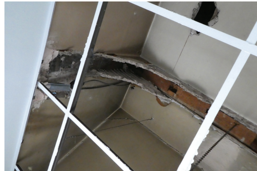
Room F2 - F_025.jpg (No. 1 Winton Square) This upwards view of the ceiling to No. 1 Winton Square reveals the remains of the original stud partition and lathe-and-plaster. Indications are that these walls were removed and the plan form altered when the suspended ceilings were first inserted in the 1980s, and not before.
