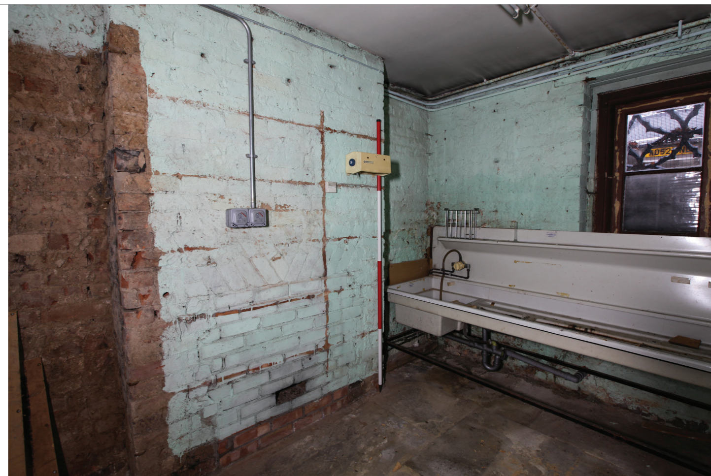
Room B8 - B_010.jpg To the right of the stairwell to No. 1 is the former scullery. The remains of a hearth have been blocked up to the chimney breast (left), although the brick wedge-lintel is still in-situ. Drainage for a sink is still in-situ, later used as a Dark Room. Stone flagged floor in-situ.
