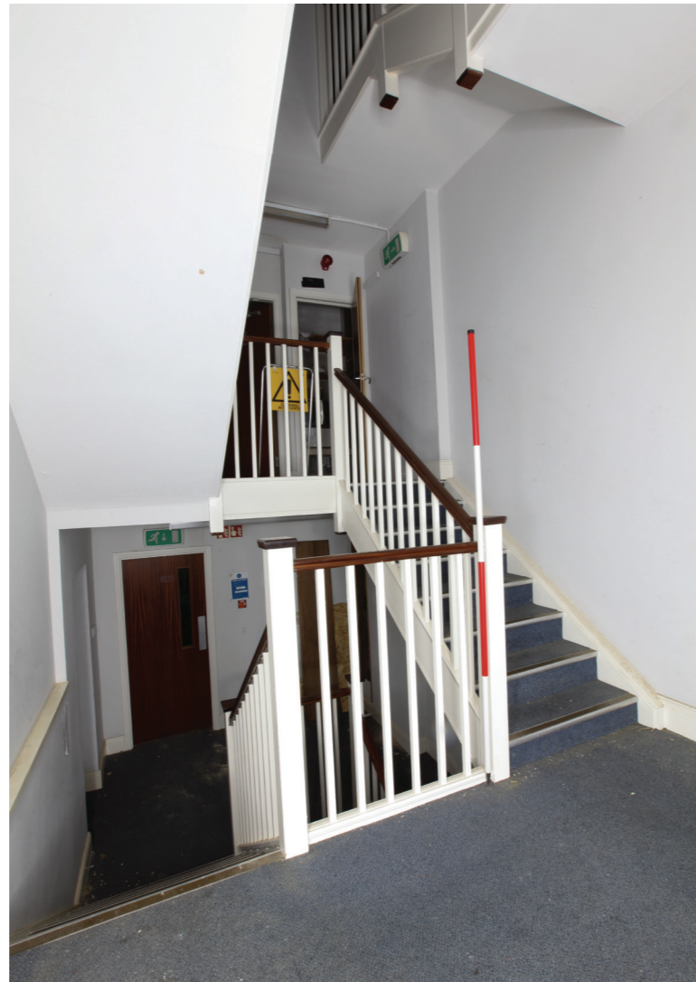
Stairwell G14 - G_032.jpg Stairwell to No. 3 Winton Square. Although it has not moved location within the building, the staircase has been altered twice, firstly when the building was extended to create mezzanine rooms and secondly in the late 20th century. The staircase may have been turned anti-clockwise when the mezzanines were added. The present staircase is entirely modern.
