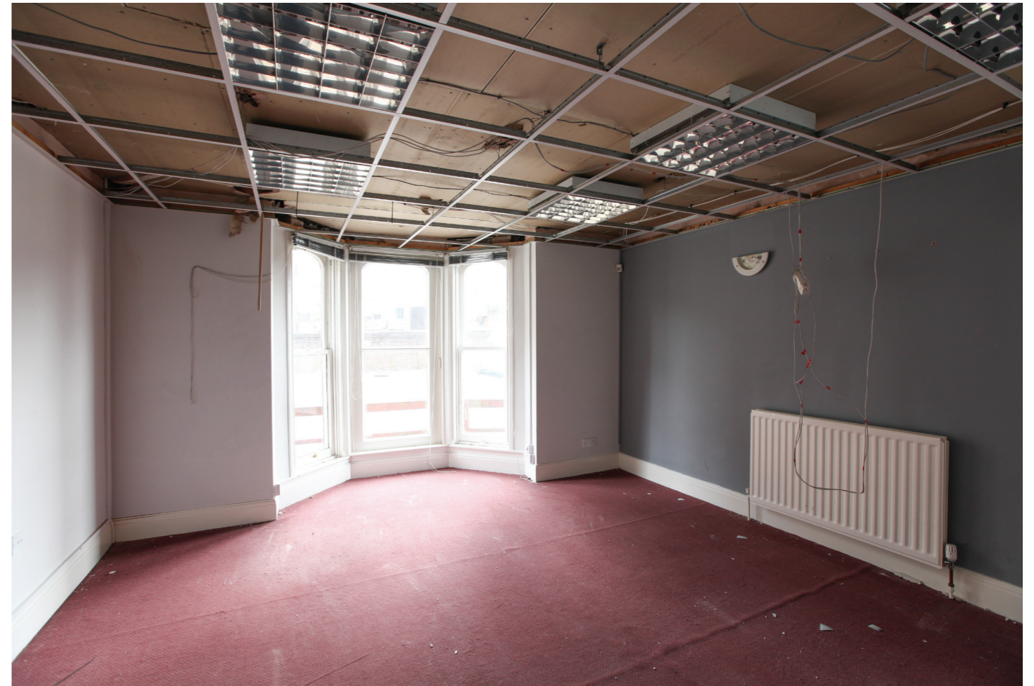
Room G13 - G_031.jpg Mezzanine reception room with full-length bay window added before 1900. There are no surviving cornices in this room and apart from the sash windows, no fixtures or fittings. The fireplace, which would have sat on the wall to the right, has also been removed and the opening blocked up.
