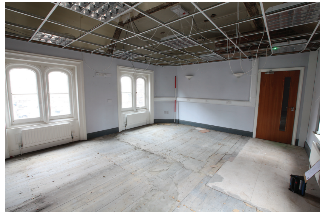
Room F1 - F_029.jpg (No. 1 Winton Square) The first floor space over the Living Room created in phase 2 was originally divided into a bedroom and smaller dressing room, with a lobby. This view of the room is looking at the main chimney breast. The right part of this had a flue serving the main bedroom. Although the fireplace has been blocked up, the hearth stone remains, as can be seen here in front of the chimney breast. The ceilings are raked, as throughout the first floor spaces, with a high level flat soffit. Here the remains of the stud partition dividing the bedroom, dressing room, and lobby can be clearly seen in the ceiling plaster, floorboards and ghosted line in the chimney breast wall. The doorway to the left is a large modern opening.
