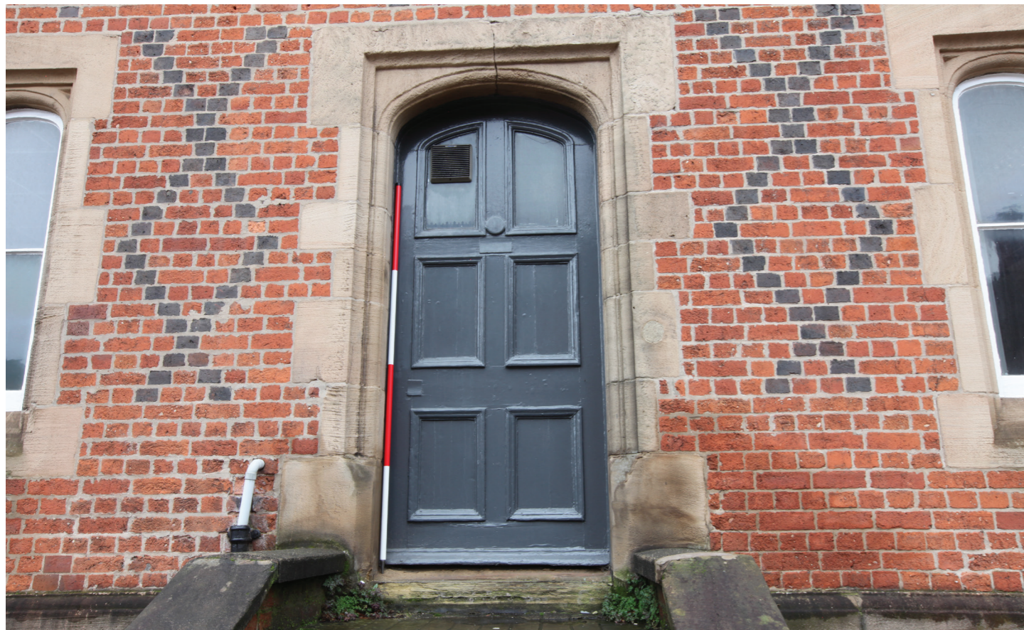
Ext_southwest_no_1_door.jpg The panelled door, with its bolection mouldings, to No. 1 may be an original one
