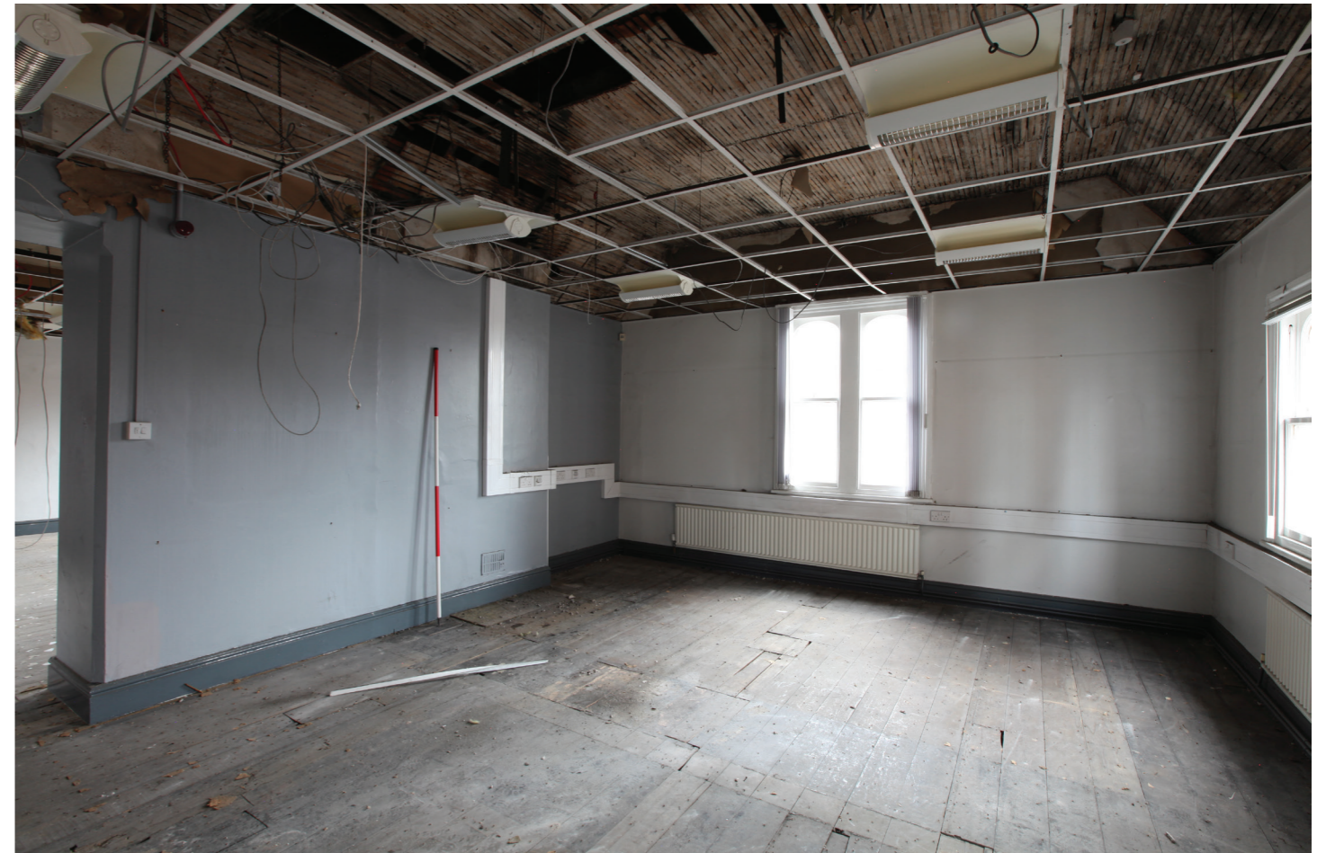
Room F1 - F_029.jpg (No. 1 Winton Square) The first floor space over the Living Room created in phase 2 was originally divided into a bedroom and smaller dressing room, with a lobby. This view of the room is looking at the main chimney breast. The right part of this had a flue serving the main bedroom. Although the fireplace has been blocked up, the hearth stone remains, as can be seen here in front of the chimney breast. The ceilings are raked, as throughout the first floor spaces, with a high level flat soffit. Here the remains of the stud partition dividing the bedroom, dressing room, and lobby can be clearly seen in the ceiling plaster, floorboards and ghosted line in the chimney breast wall. The doorway to the left is a large modern opening.
