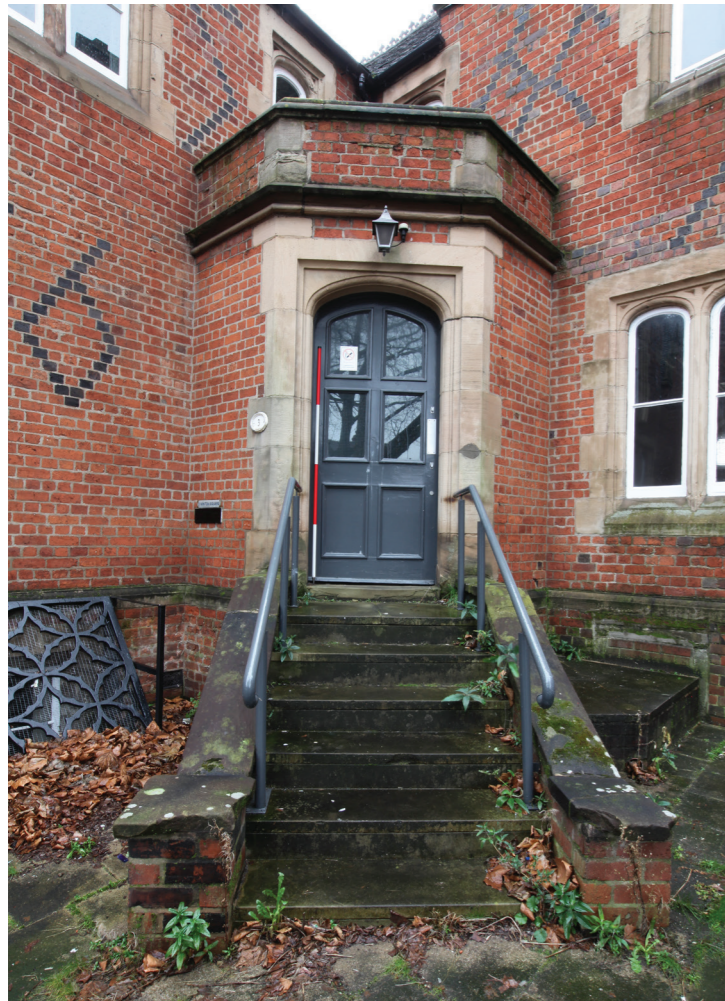
Ext_southeast_no_3_detail_porch.jpg The porch to No. 3 provided access to both No. 3 and independent access to the adjoining office, to the left.
