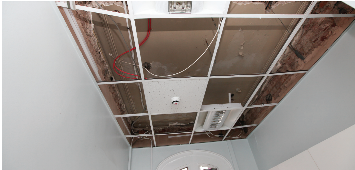
Room G3 - G_009.jpg - former staircase hall to No. 1 with inserted suspended ceiling. The doorway is still in-situ but the space is now occupied by a kitchen. The front part of the plaster cornice survives, and the outline and rake of the former staircase is evident from the ghosted plasterwork.
