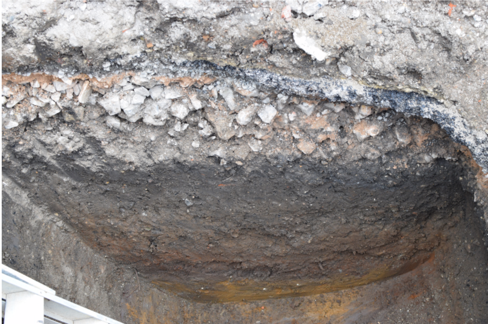
Plate 3: The north-facing section of Test Pit 3
