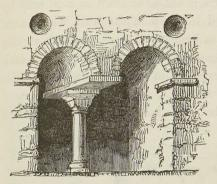
two circular-headed arches formed of radiating bricks, and having for imposts abaci of the same material, over each jamb of which, in the east and west sides, is a small, round, splayed soundhole. These have very recently been discovered and opened.
