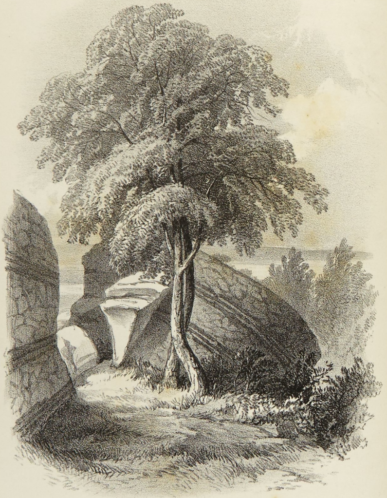
EXTERIOR. NORTH GATE .
