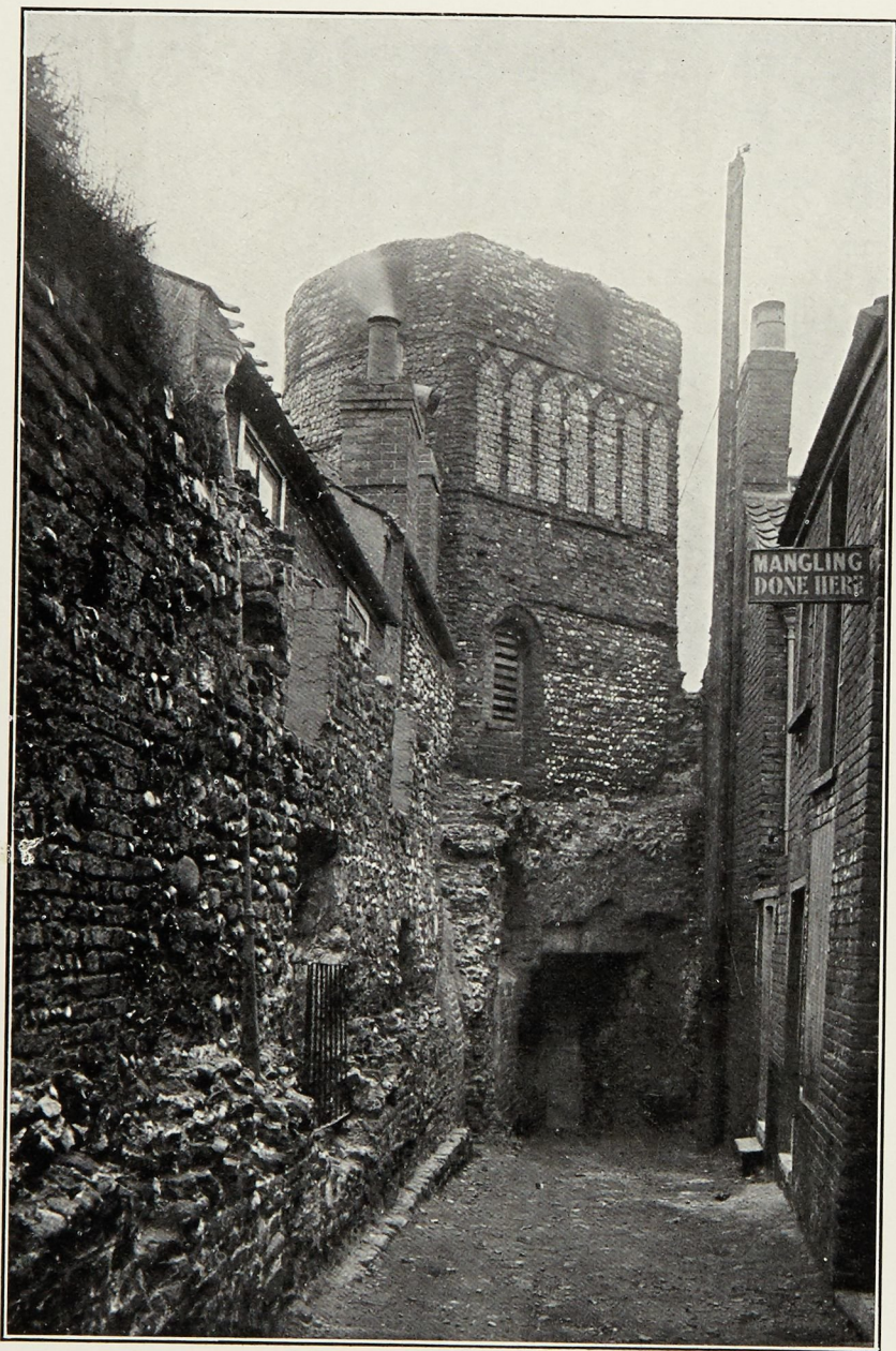
BACK OF S.E. TOWER AND WALL, GREAT YARMOUTH.
